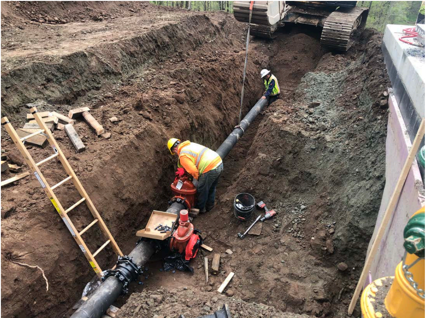
Picture 9: View of 8" water tank drain line located south of the altitude valve vault. Note that Ludlow removed the section of 6" DIP they placed temporarily between the 8" DIP water tank drain line and the altitude valve vault.
