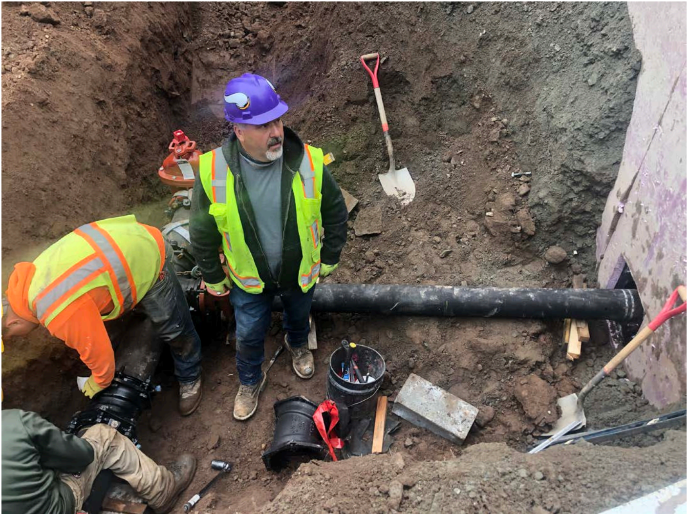
Picture 7: Section of 6" DIP that Ludlow placed temporarily between the altitude valve vault and the 8" water tank drain line to assist in the correct placement of the 6" gate valve they attached to the 8"x8"x6" M.J. TEE on the 8" drain line. View to the west.
