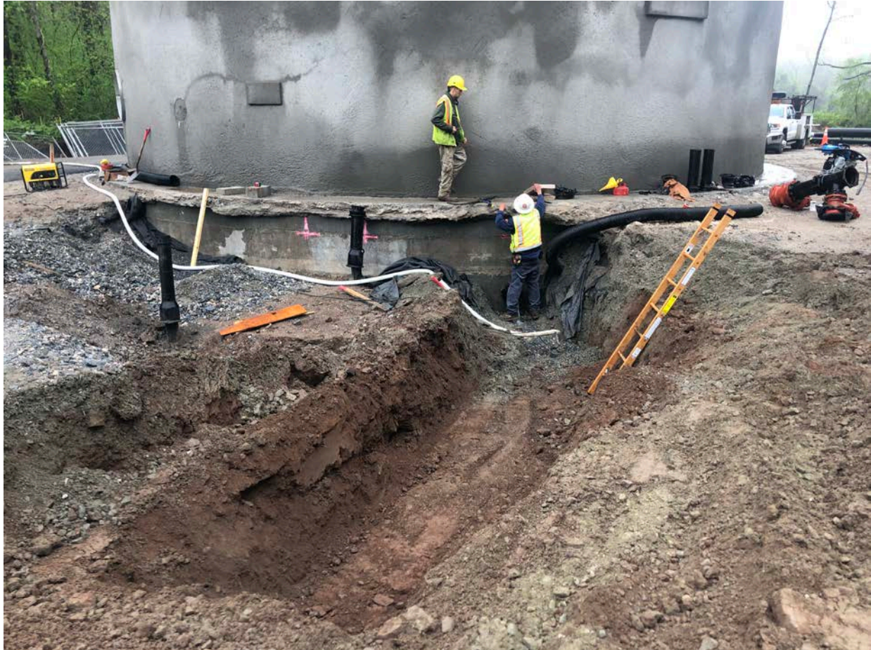
Picture 2: Trench that Ludlow excavated west of the water tank as they begin to install the tank drain line that will run south of the altitude valve vault. View to the east/northeast.
