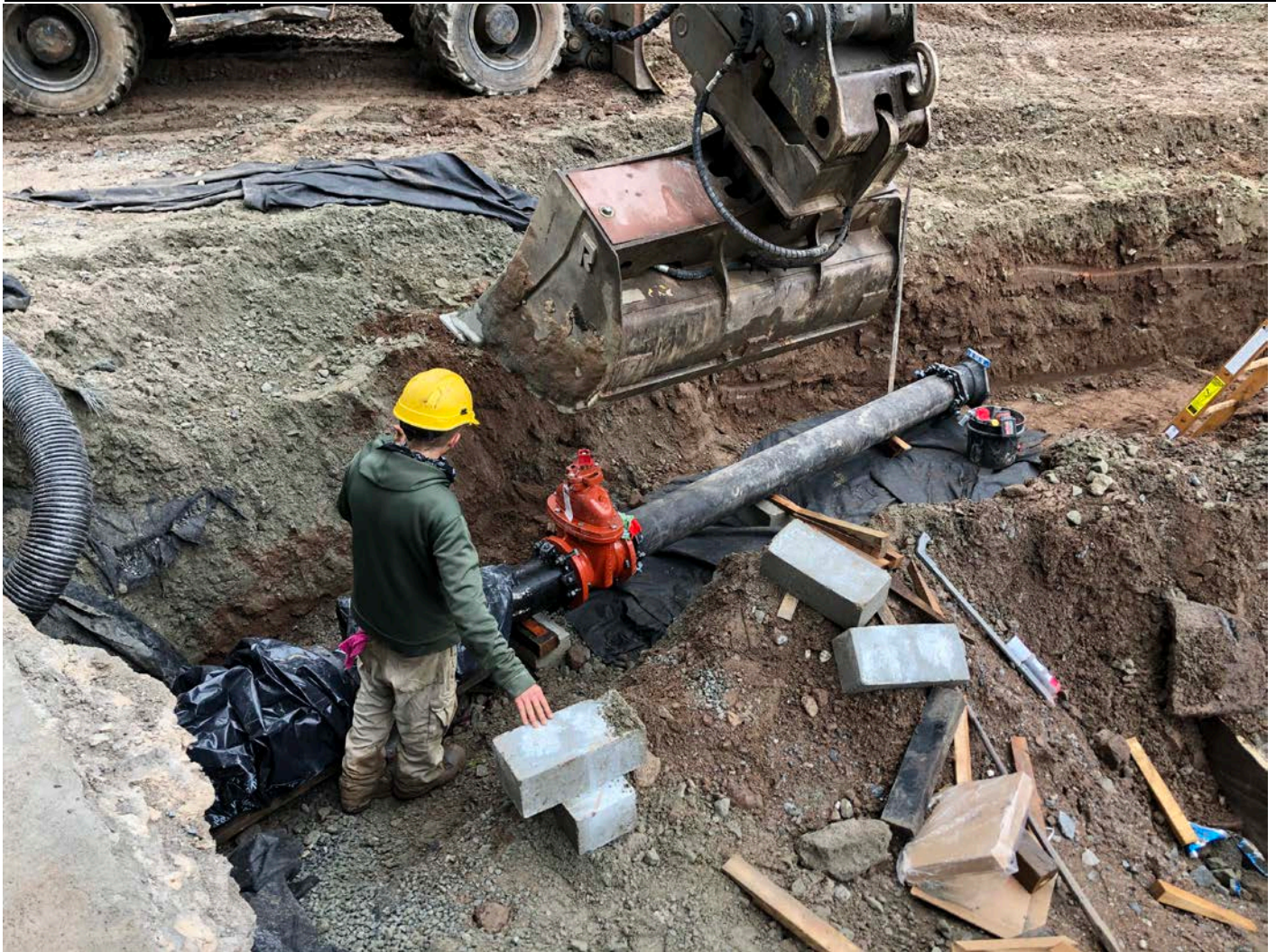
Picture 5: Ludlow in the process of installing a section of 8" DIP to the west of the 8" gate valve they just installed as part of the 8" DIP drain line that they are installing off the southwest side of the water tank. Shared Access Driveway, Middletown.
