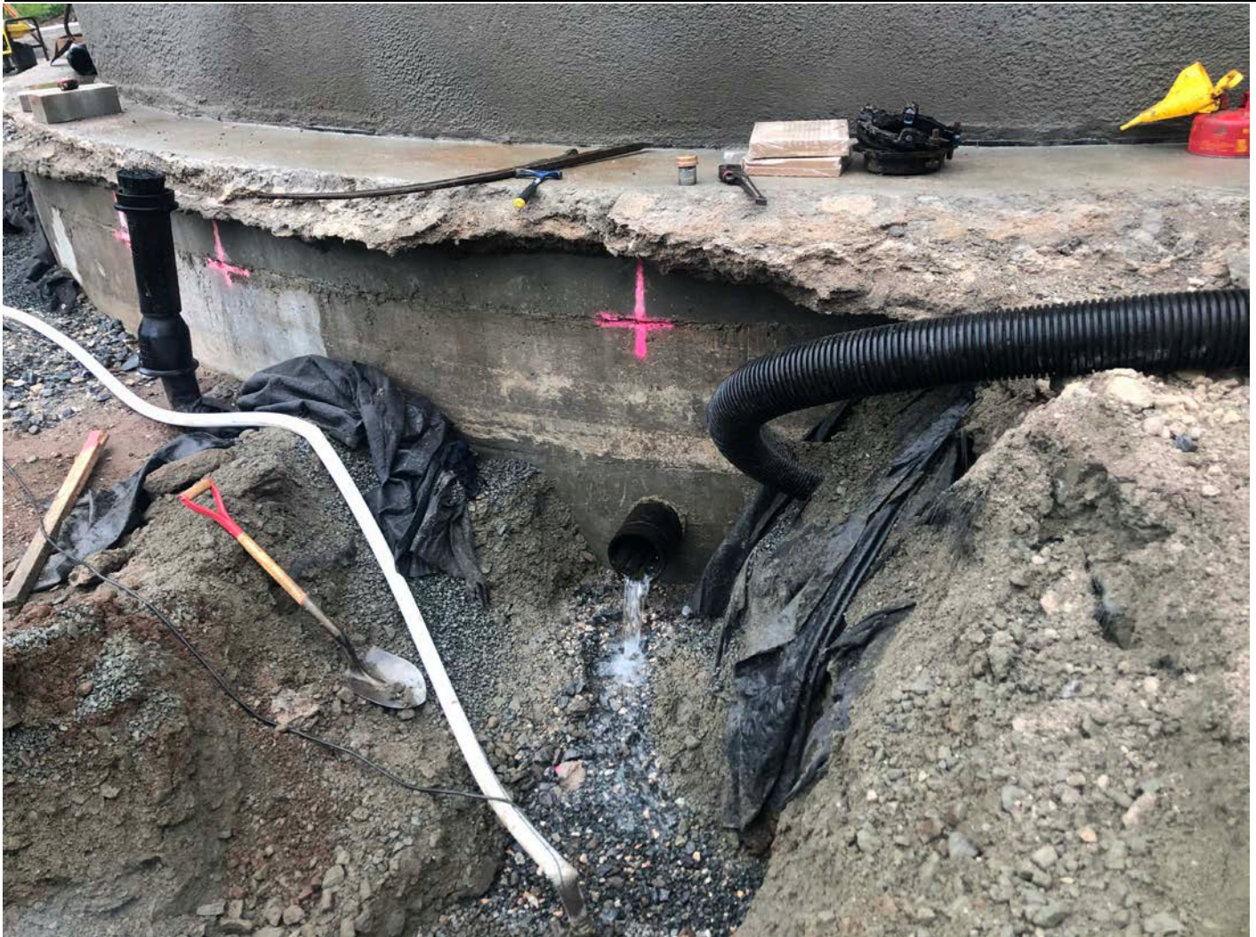
Picture 1: View of the 8" DIP water tank drain line that protrudes from the southwest side of the water tank located east of the Shared Access Driveway in Middletown. Ludlow daylighted the pipe in order to attach 8" DIP to it as they begin to install the tank drain line that will run south of the altitude valve vault. View to the east/northeast.
