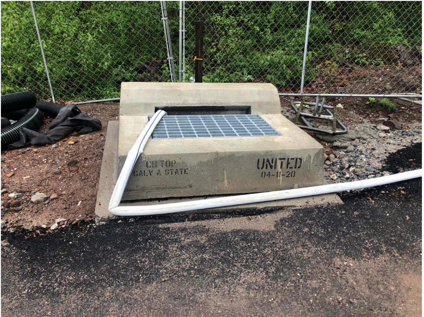
Picture 3: Catch basin that Ludlow is using to discharge water that drained out of the tank from the 8" DIP line that protrudes from the southwest side of the water tank as Ludlow installs the 8" tank drain line that will run south of the altitude valve vault. View to the north.
