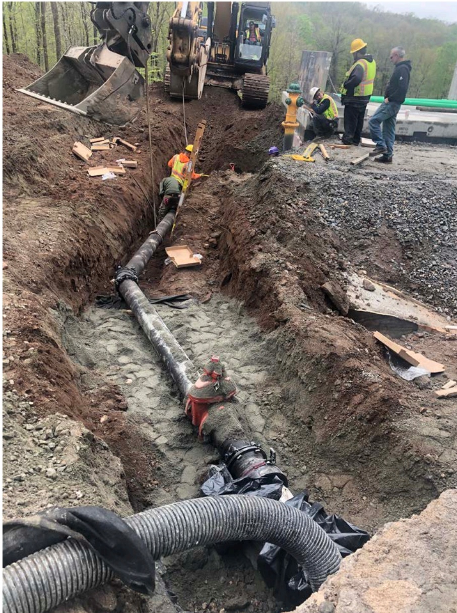
Picture 6: Overview of the 8” drain line that Ludlow is installing between the water tank and the headwall located south of the Shared Access Driveway at Station 11+70. View to the west.
