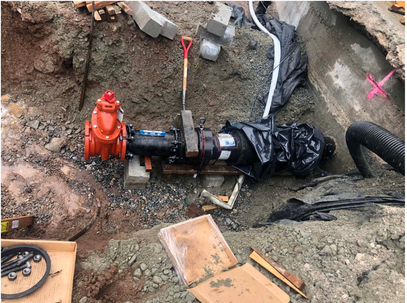
Picture 4: 8" MJ gate valve with flexible fitting that Ludlow has just connected to the 8" DIP drain line that protrudes from the water tank located east of the Shared Access Driveway in Middletown. View to the north.
