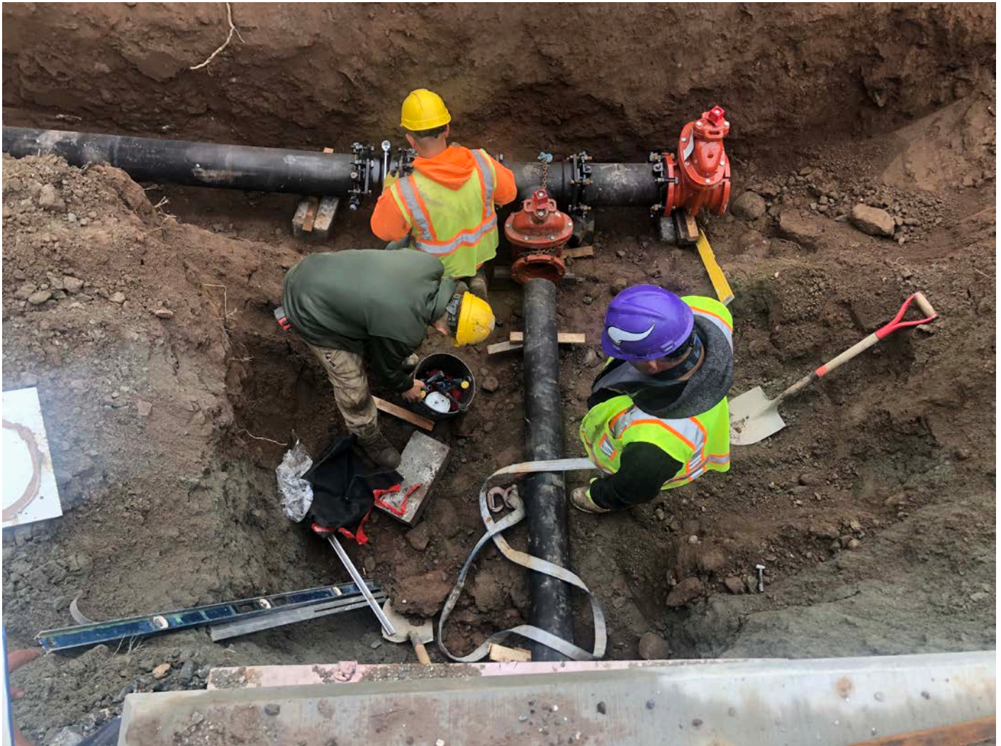
Picture 8: Another view of the 6" DIP that Ludlow placed temporarily between the altitude valve vault and the 8" water tank drain line to assist in the correct placement of the 6" gate valve they attached to the 8"x8"x6" M.J. TEE on the 8" drain line. View to the south.
