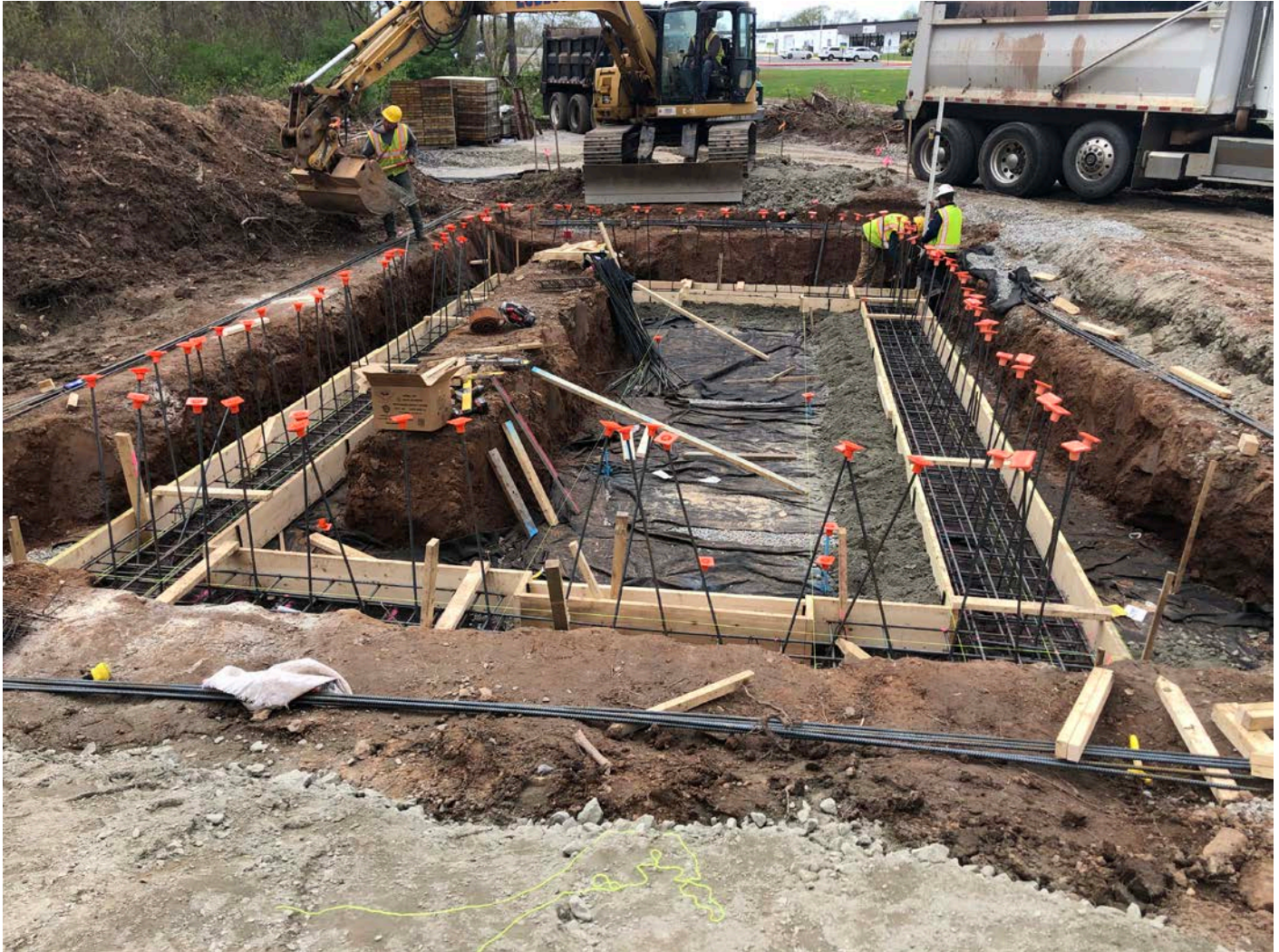
Picture 10: View of the booster station footprint as Ludlow continues to place and secure vertical pieces of rebar for the frost wall associated with the booster station. Station 750+63, Middletown. View to the west.
