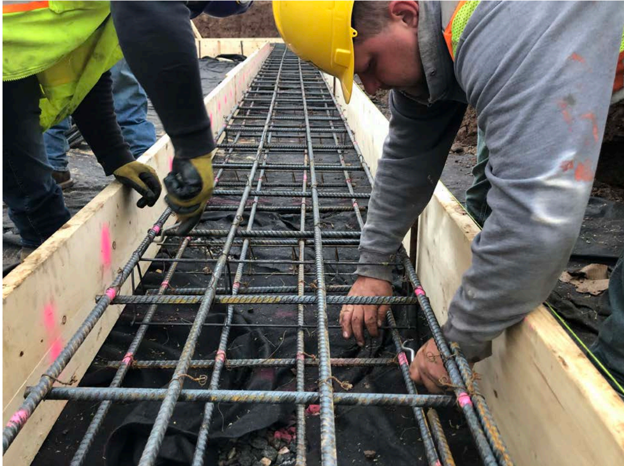
Picture 2: Ludlow twisting wire around intersecting pieces of rebar within the concrete forms for the footings of the booster station located at Station 750+63 in Middletown.
