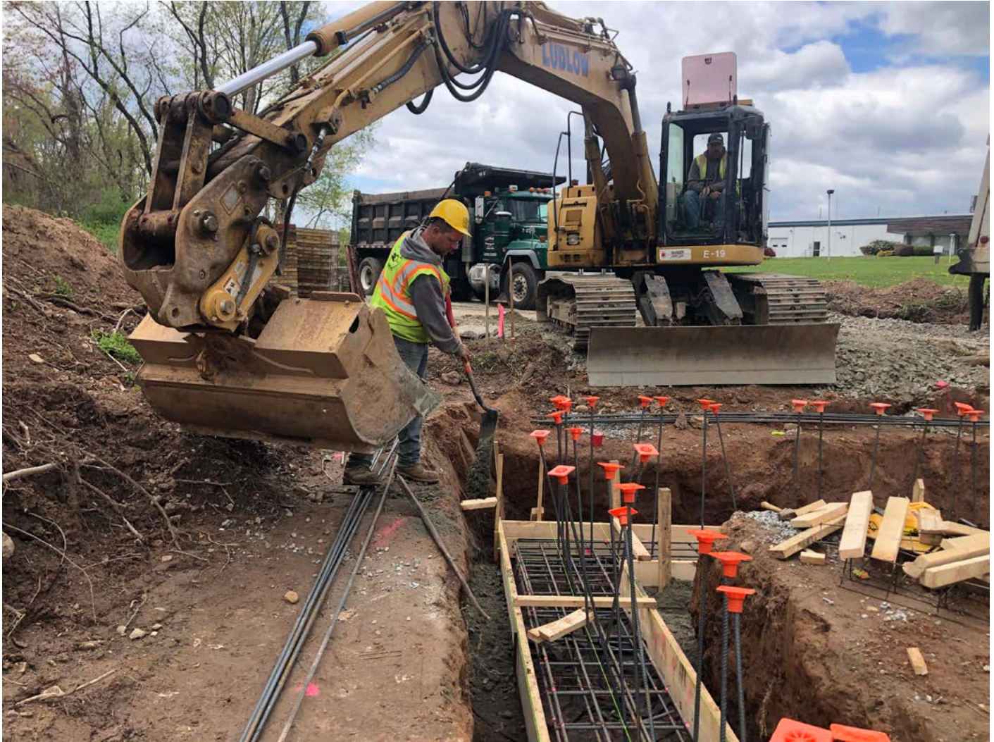
Picture 9: Ludlow placing 1.5" gravel on the exterior of the concrete forms for the booster station footings to prevent the concrete that will be poured on May 3, 2021, from blowing out from beneath the forms. Station 750+63, Middletown; view to the west.
