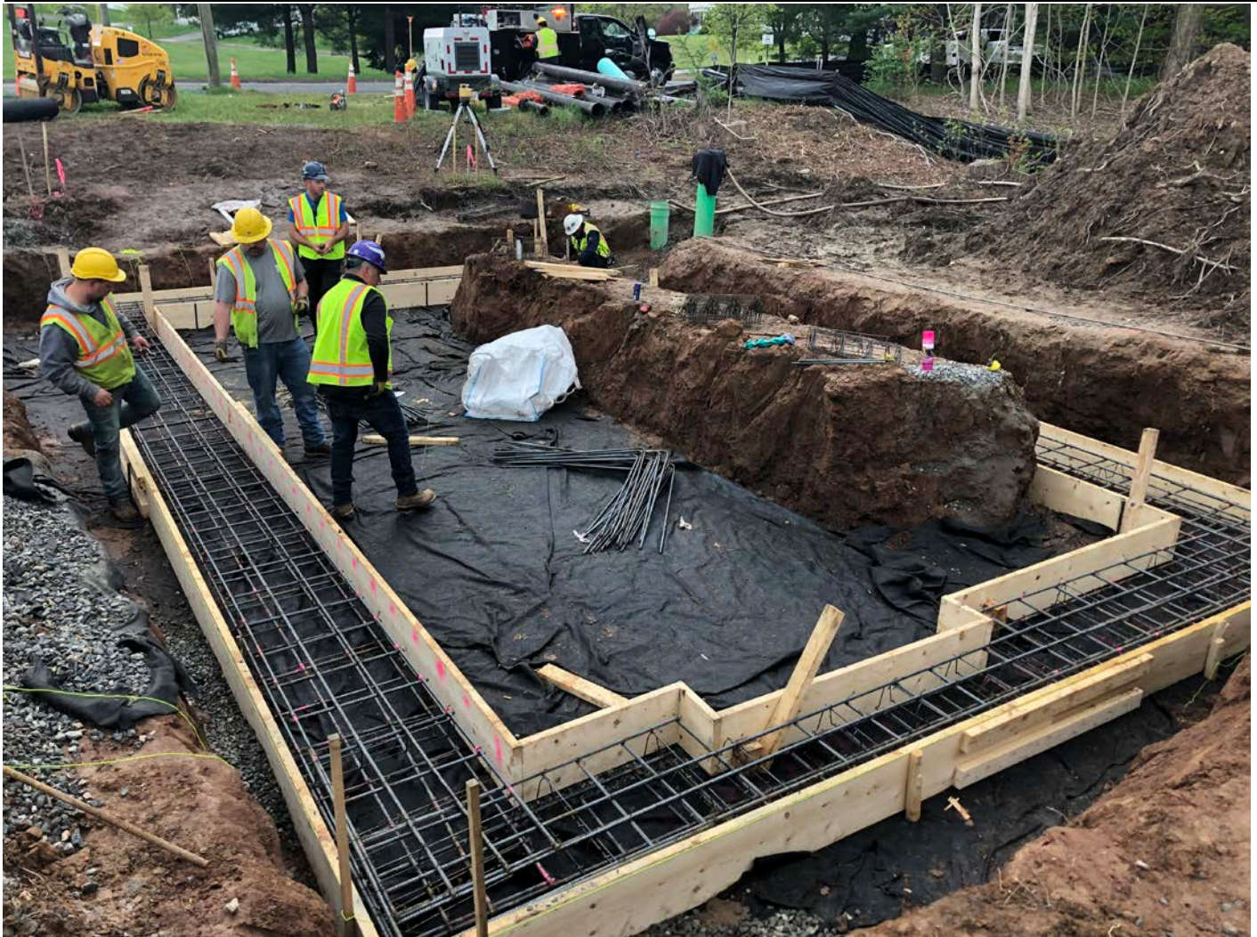
Picture 1: View of the booster station footprint as Ludlow continues to place and secure rebar within the concrete forms of the footings for the booster station located at Station 750+63 in Middletown. View to the east.
