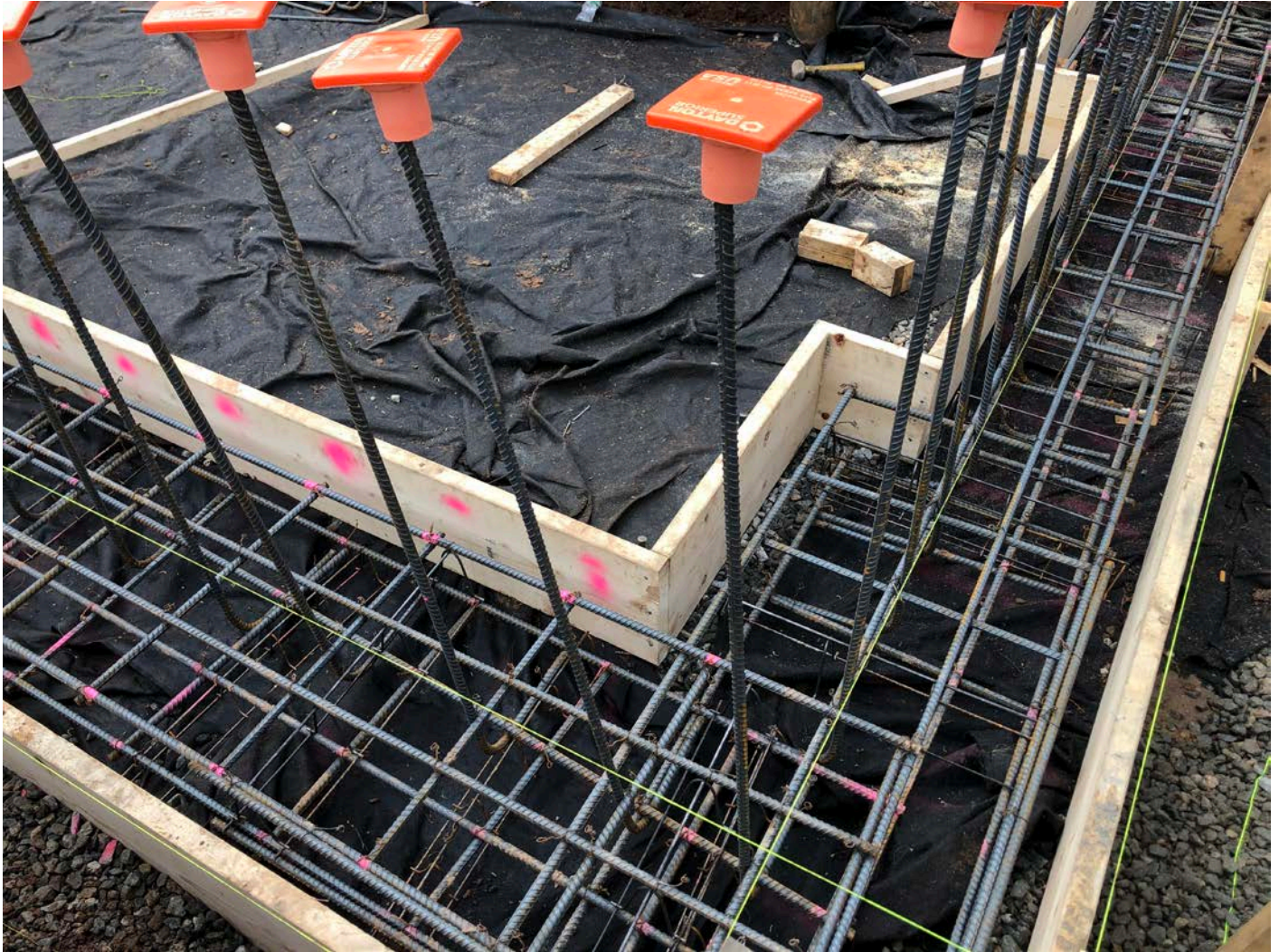
Picture 4: Vertical sections of rebar that have been placed within the concrete forms for the booster station frost wall. Station 750+63, Middletown; view to the south.
