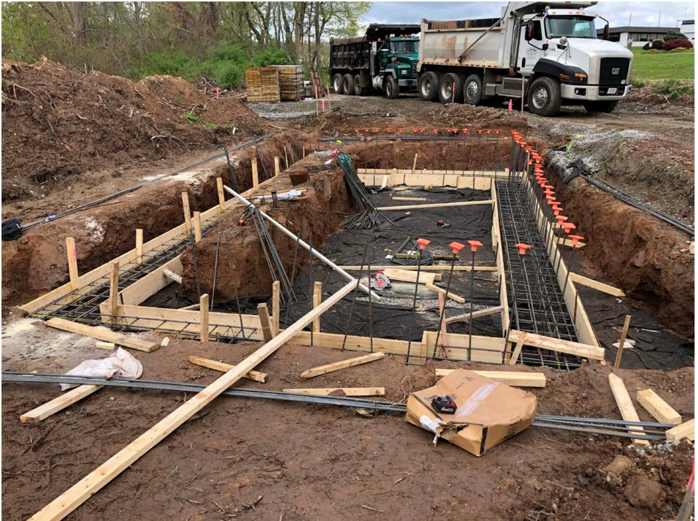
Picture 3: View of the booster station footprint as Ludlow begins to place and secure vertical sections of rebar for the frost wall associated with the construction of the booster station located at Station 750+63 in Middletown. View to the west.
