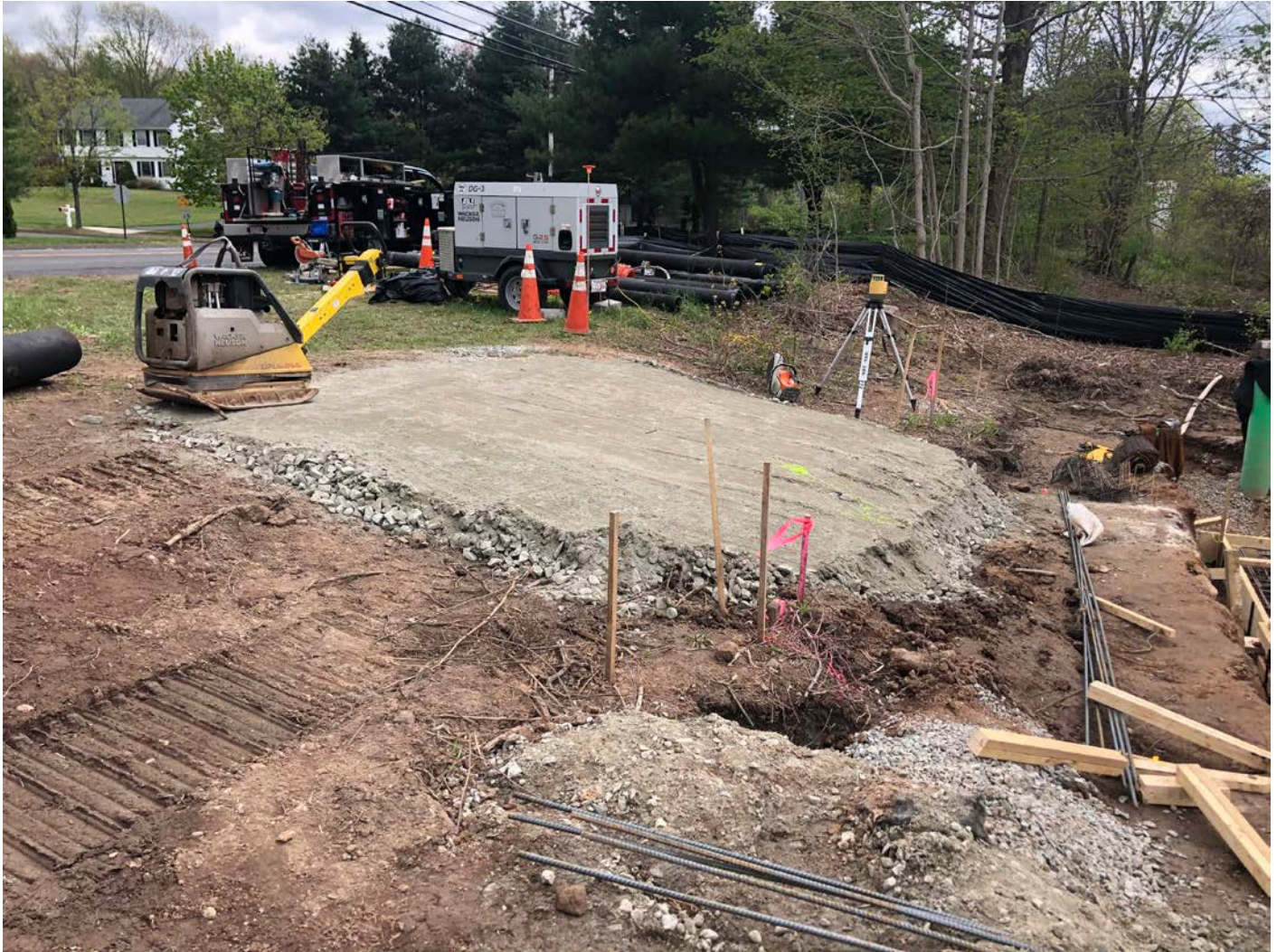
Picture 8: Pad comprised of 1.5" compacted gravel located on the east side of the booster station footprint. The pad will serve as a more stable platform for the concrete truck to stage upon when concrete gets poured into the forms for the booster station footings on Monday, May 3, 2021. Station 750+63, Middletown; view to the south.
