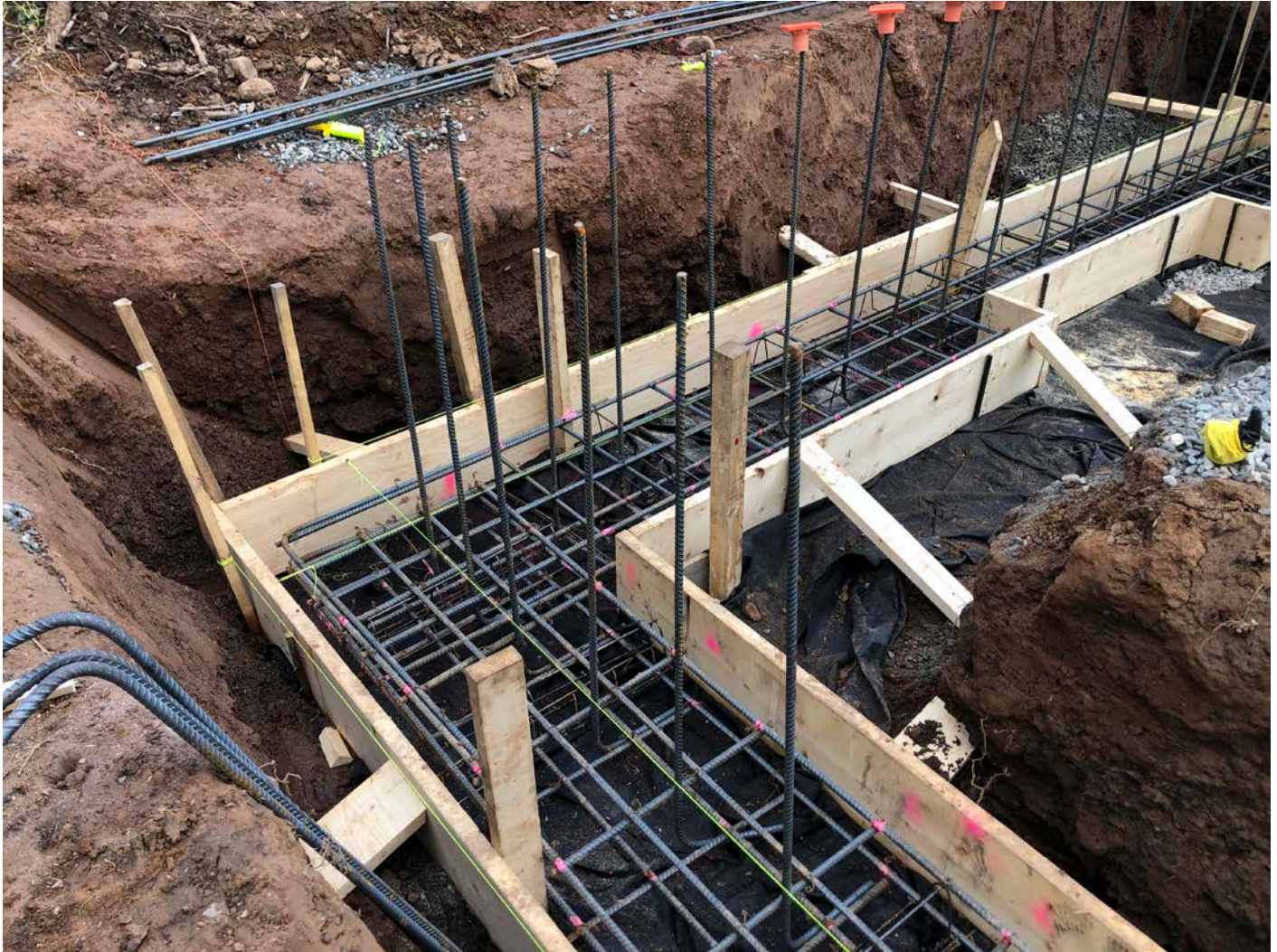
Picture 6: Vertical sections of rebar that have been placed within southeast corner of the concrete forms for the booster station frost wall. Station 750+63, Middletown; view to the southwest.
