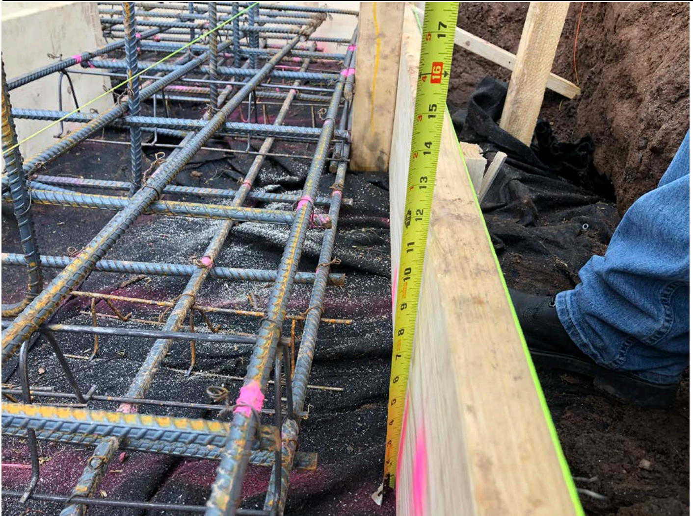
Picture 5: View of the side of one of the concrete forms for the booster station footings, showing 12" of height per specifications. Station 750+63, Middletown.
