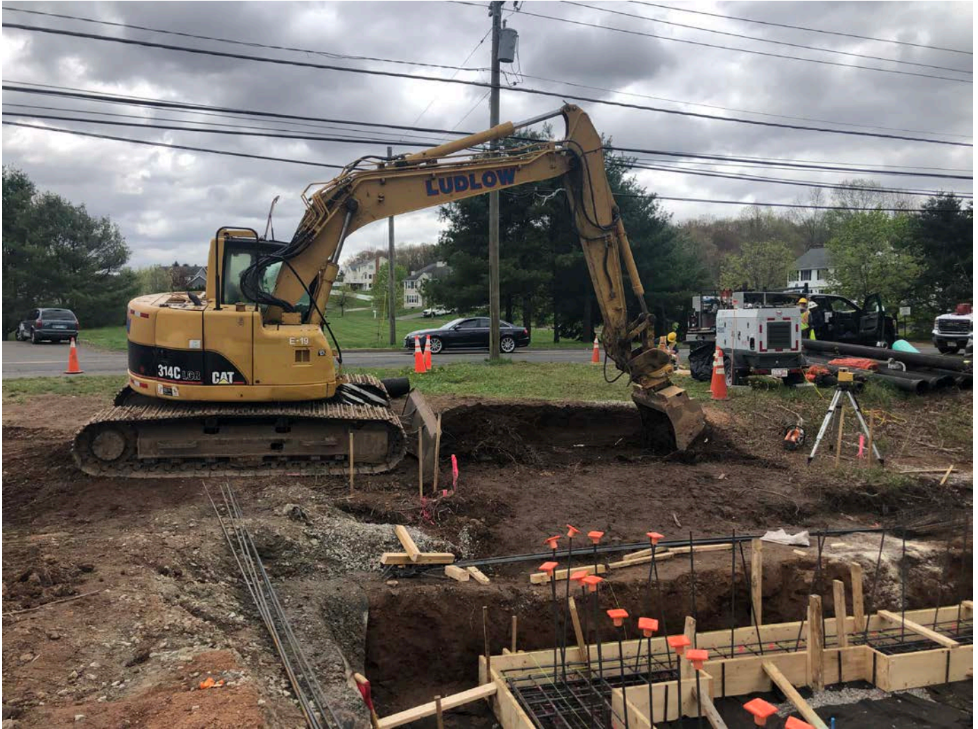
Picture 7: Ludlow excavating soil east of the booster station footprint for the placement of a compacted pad made of 1.5" gravel. Station 750+63; view to the east.
