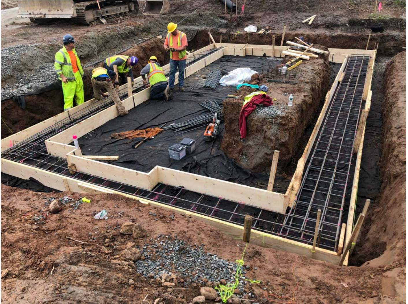
Picture 6: View of the booster station footprint where Ludlow is in the process of placing rebar within the concrete forms for the booster station footings. Station 750+63, Middletown; view to the east/southeast.
