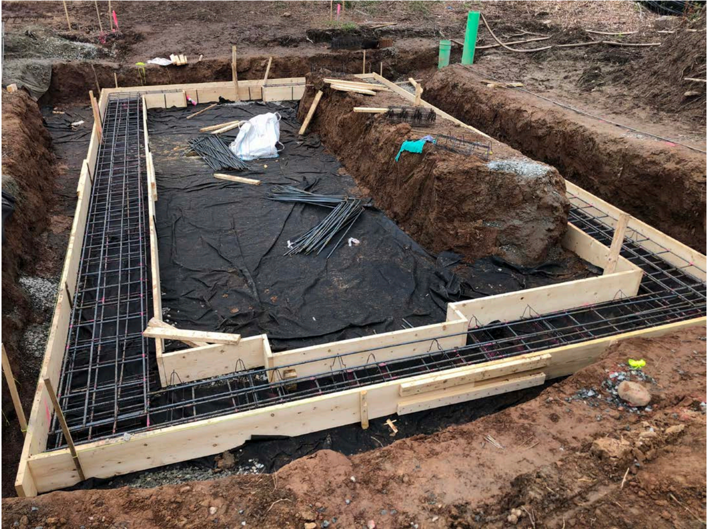
Picture 8: View of the booster station footprint depicting the progress of rebar placement within the forms for the booster station footing. Station 750+63, Middletown. View to the east.
