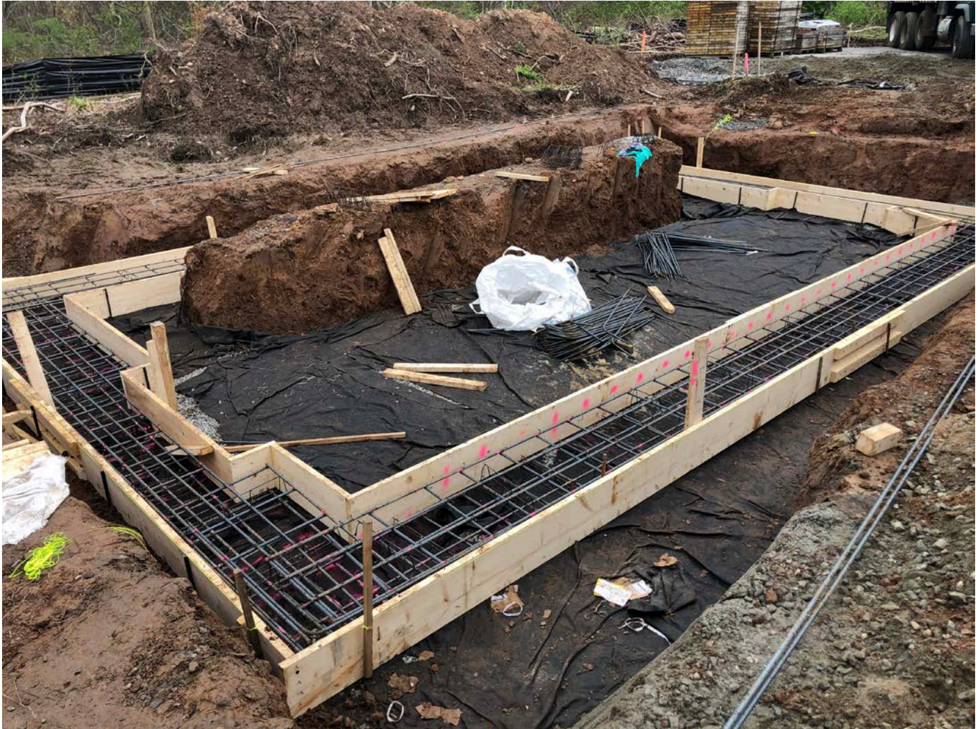
Picture 9: View of the booster station footprint depicting progress of rebar placement within the concrete forms for the booster station footing. Station 750+63, Middletown. View to the southwest.
