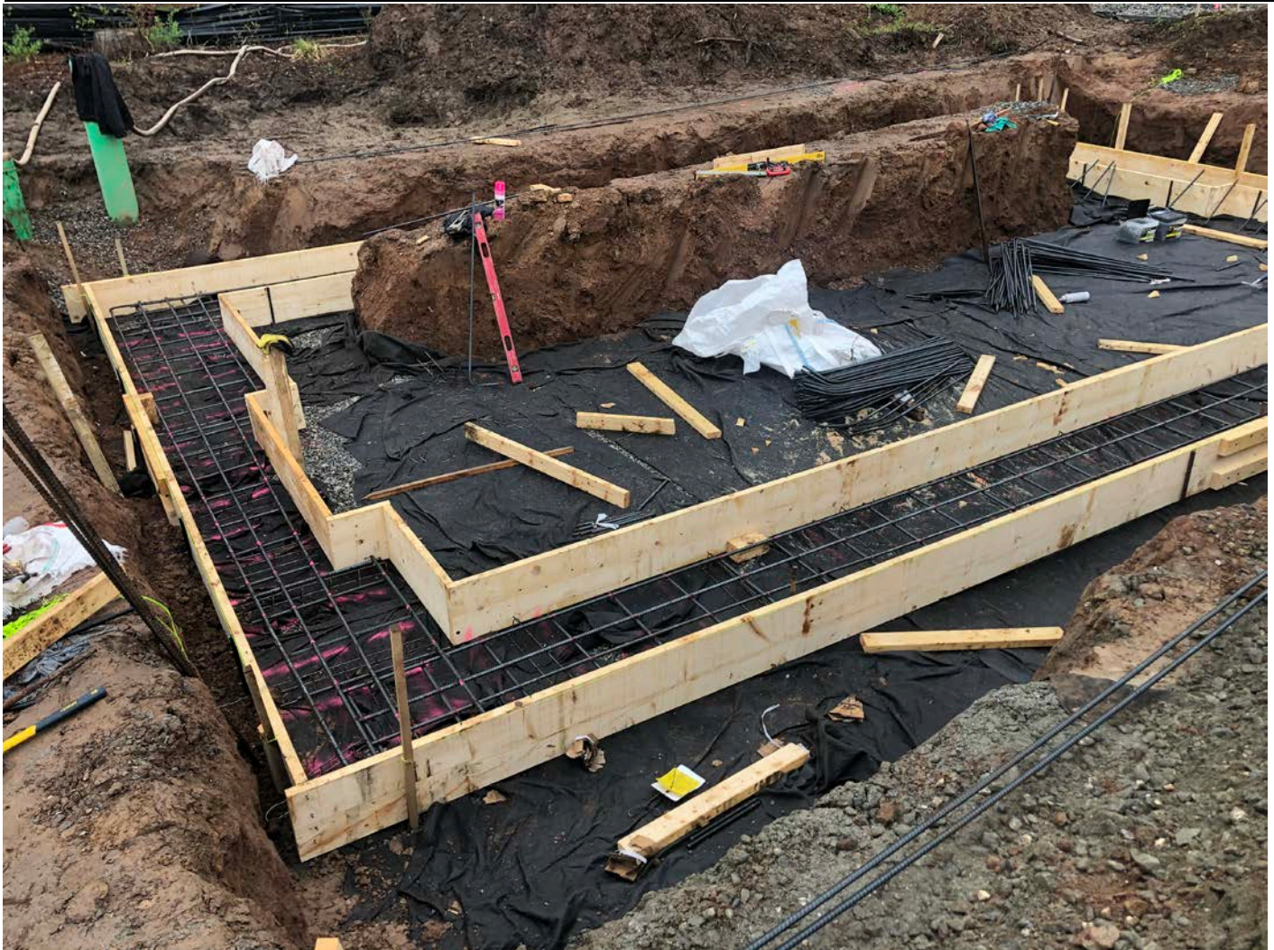
Picture 5: View of the booster station footprint where Ludlow is in the process of placing rebar within the concrete forms for the booster station footings. Station 750+63, Middletown; view to the west.
