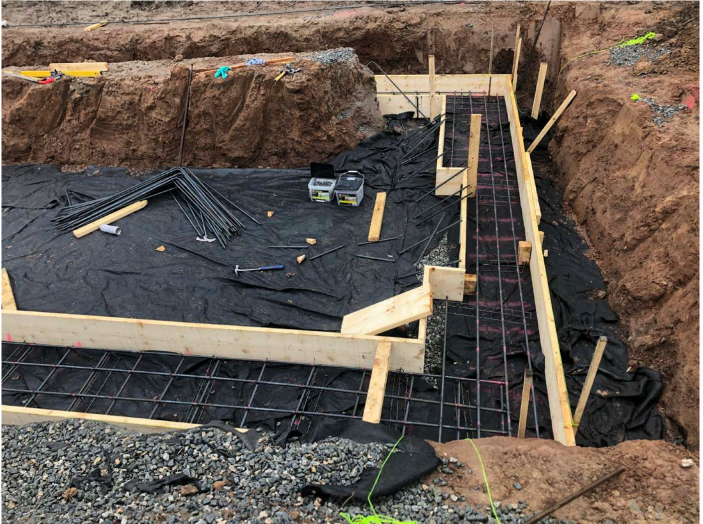
Picture 4: View of the booster station footprint where Ludlow has begun to place rebar within the concrete forms for the booster station footings. Station 750+63, Middletown; view to the south.
