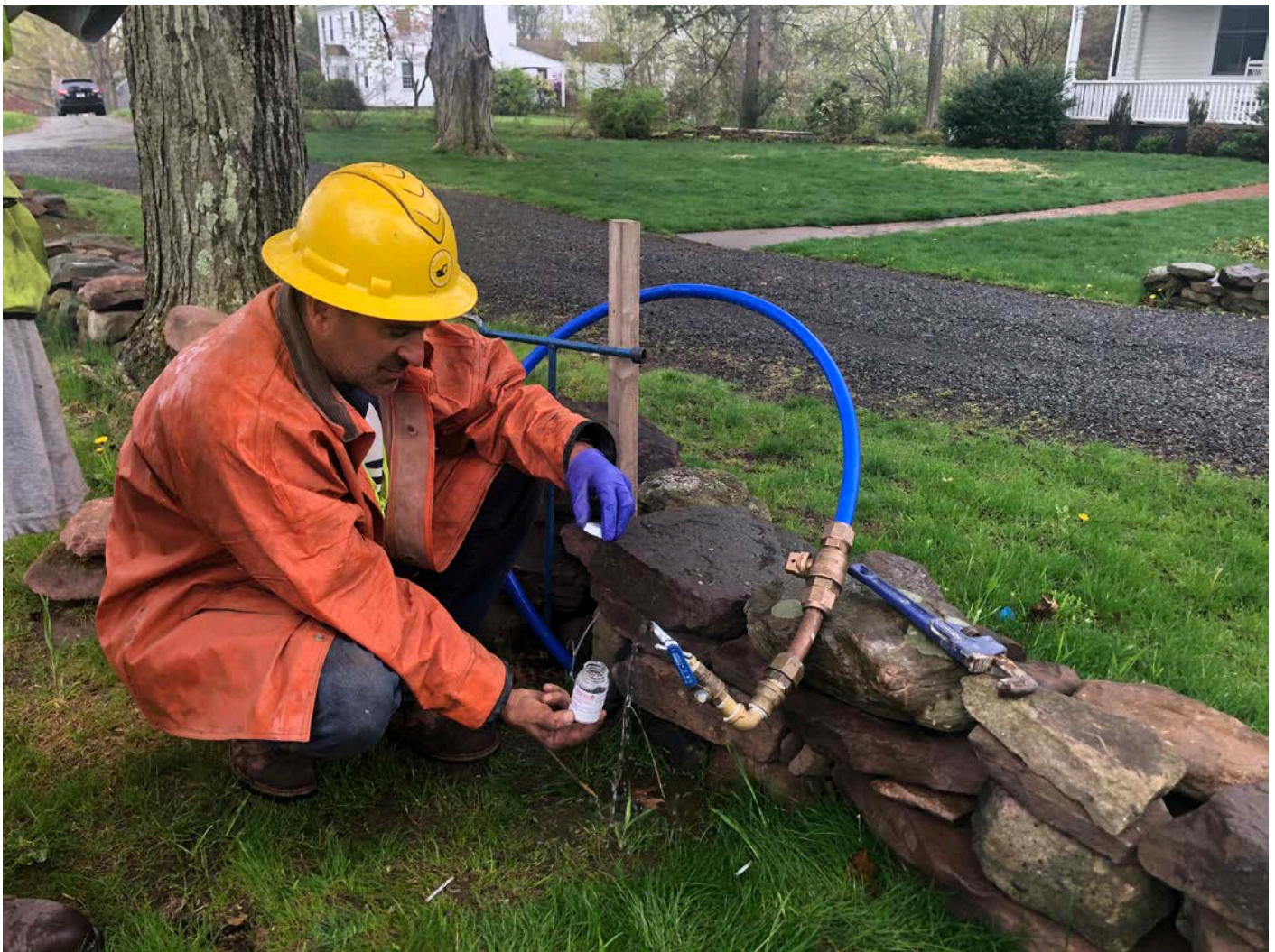
Picture 3: Ludlow collecting a water sample at 254 Maple Avenue from a 1" line attached to the 12" DIP waterline on Maple Avenue, Durham.
