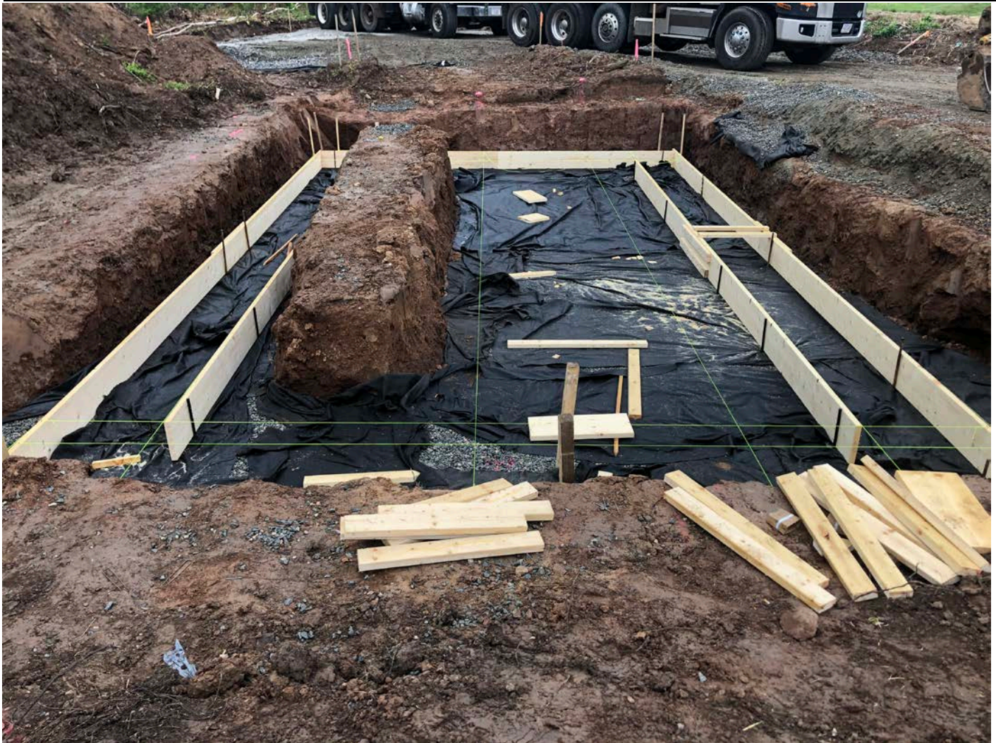
Picture 1: View of the booster station footprint at Station 750+63 in Middletown before the placement of rebar today. View to the west.
