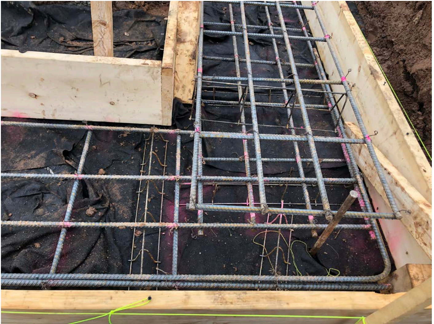
Picture 7: View of the rebar that Ludlow is placing within the concrete forms for the booster station; northeast corner of the booster station footprint. Station 750+63; view to the west.
