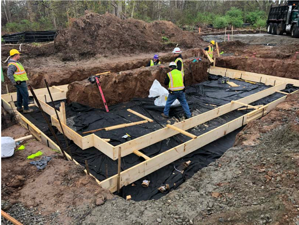
Picture 2: View of the booster station footprint as Ludlow prepares to place rebar within the concrete forms for the footings. Station 750+63 in Middletown; view to the southwest.
