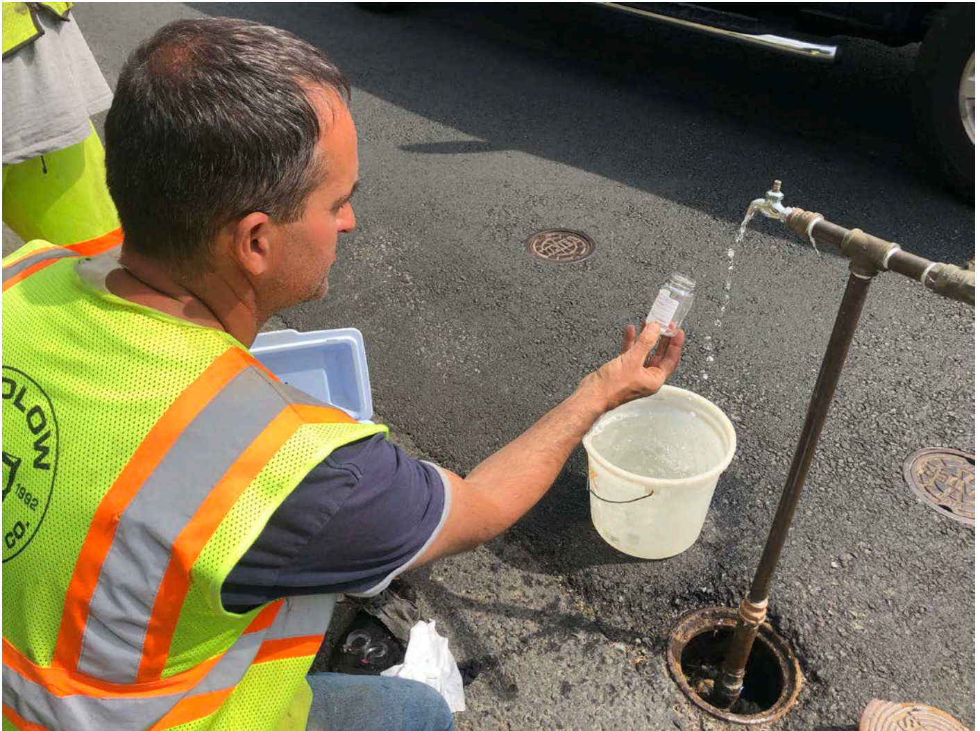
Picture 4: Ludlow collecting a water sample for submittal to a laboratory for analysis of residual chlorine from the intersection of Talcott Lane and Main Street, Durham.
