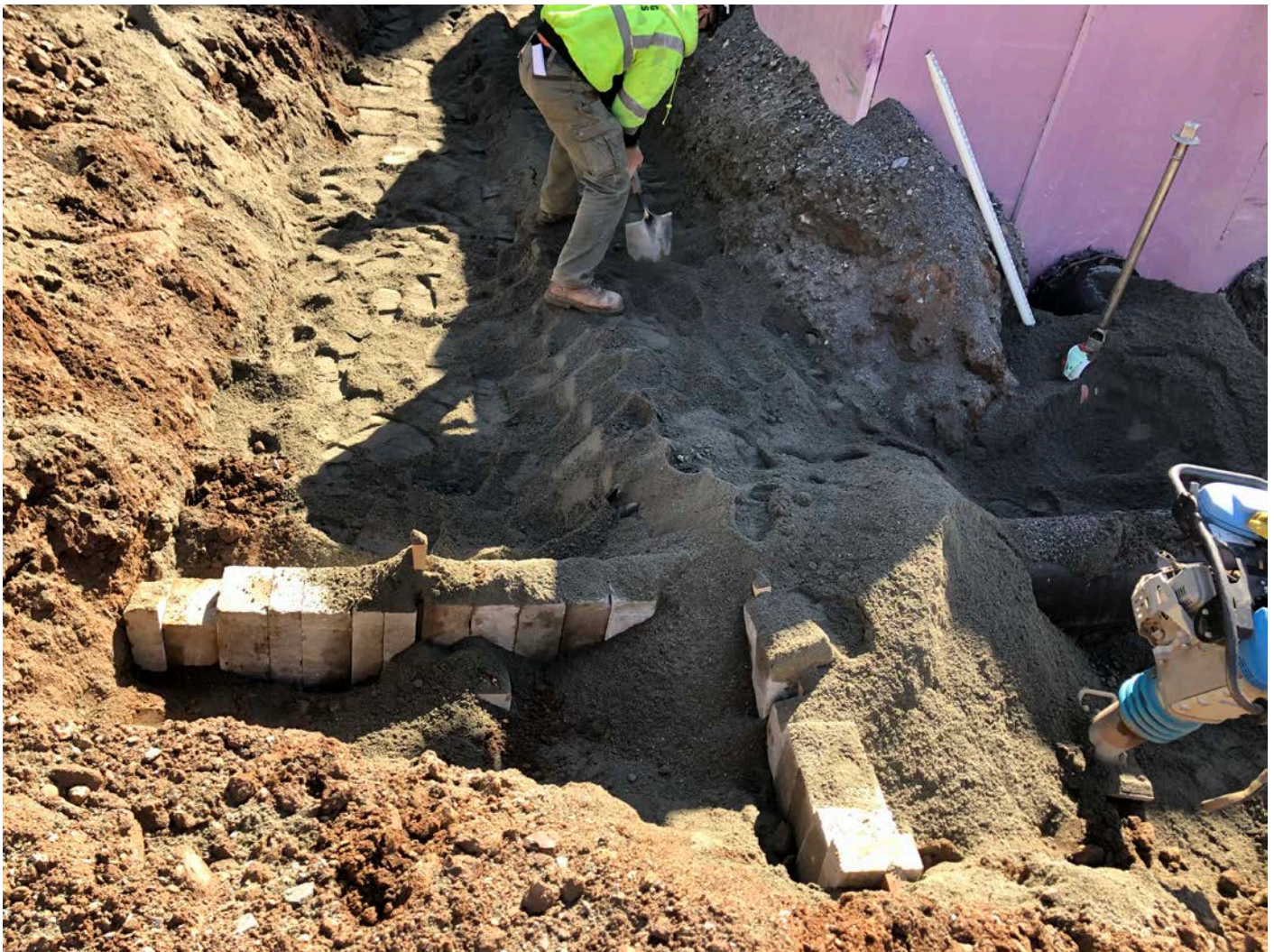
Picture 3: Thrust blocks placed on the 90° corner of the 16" DIP bypass line that is located northwest of the altitude valve vault. Shared Access Driveway in Middletown; View to the east.
