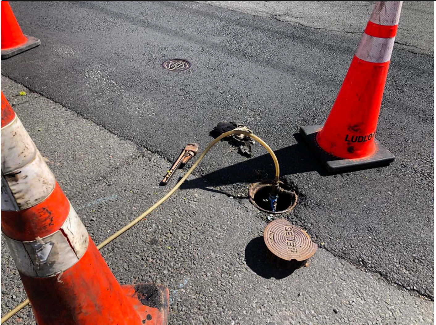
Picture 5: JMS Connections injecting sodium hypochlorite into the 16" waterline on Main street, Durham. The injection point is located at the intersection of Main Street and Talcott Lane in Durham. View to the northeast.
