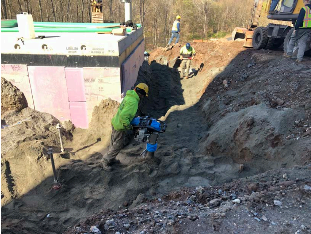
Picture 2: Ludlow compacting sand that was placed over the 16" DIP bypass line that Ludlow installed on the north side of the altitude valve vault located east of the Shared Access Driveway in Middletown. View to the west.
