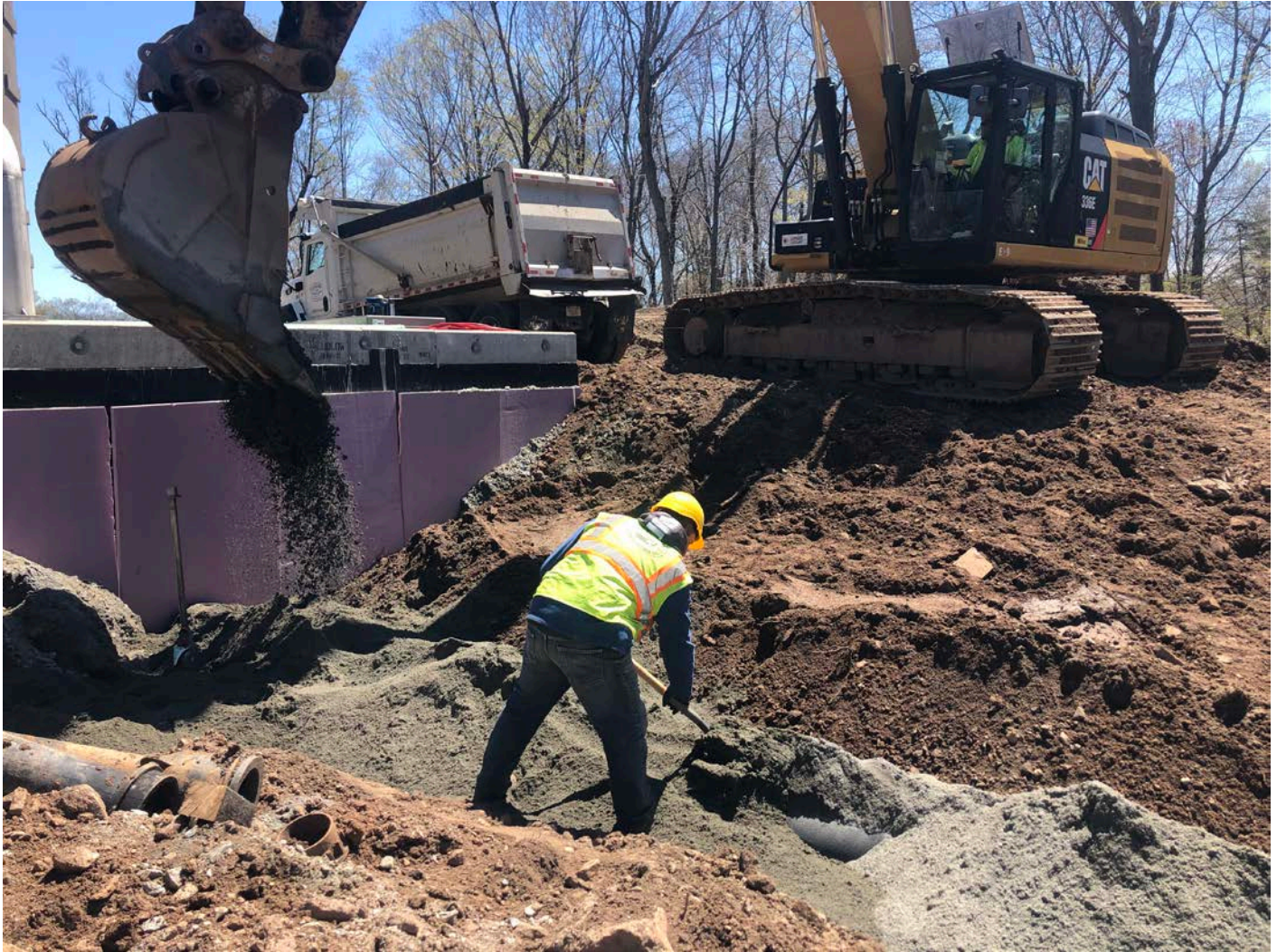
Picture 6: Ludlow placing sand over the 16" and 20" DIP° that was installed west of the altitude valve vault at the water tank work zone located east of the Shared Access Driveway in Middletown.
