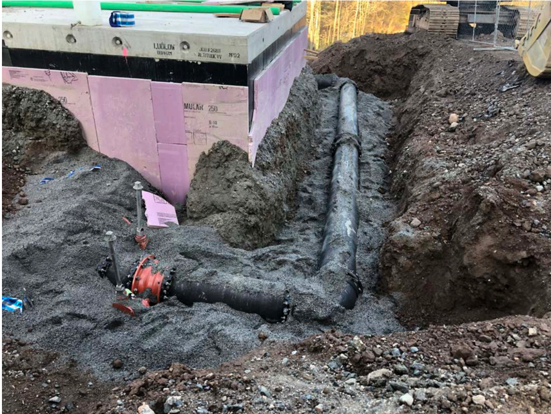
Picture 1: View of the 16" DIP bypass line that Ludlow installed on the north side of the altitude valve vault located east of the Shared Access Driveway in Middletown. View to the west.
