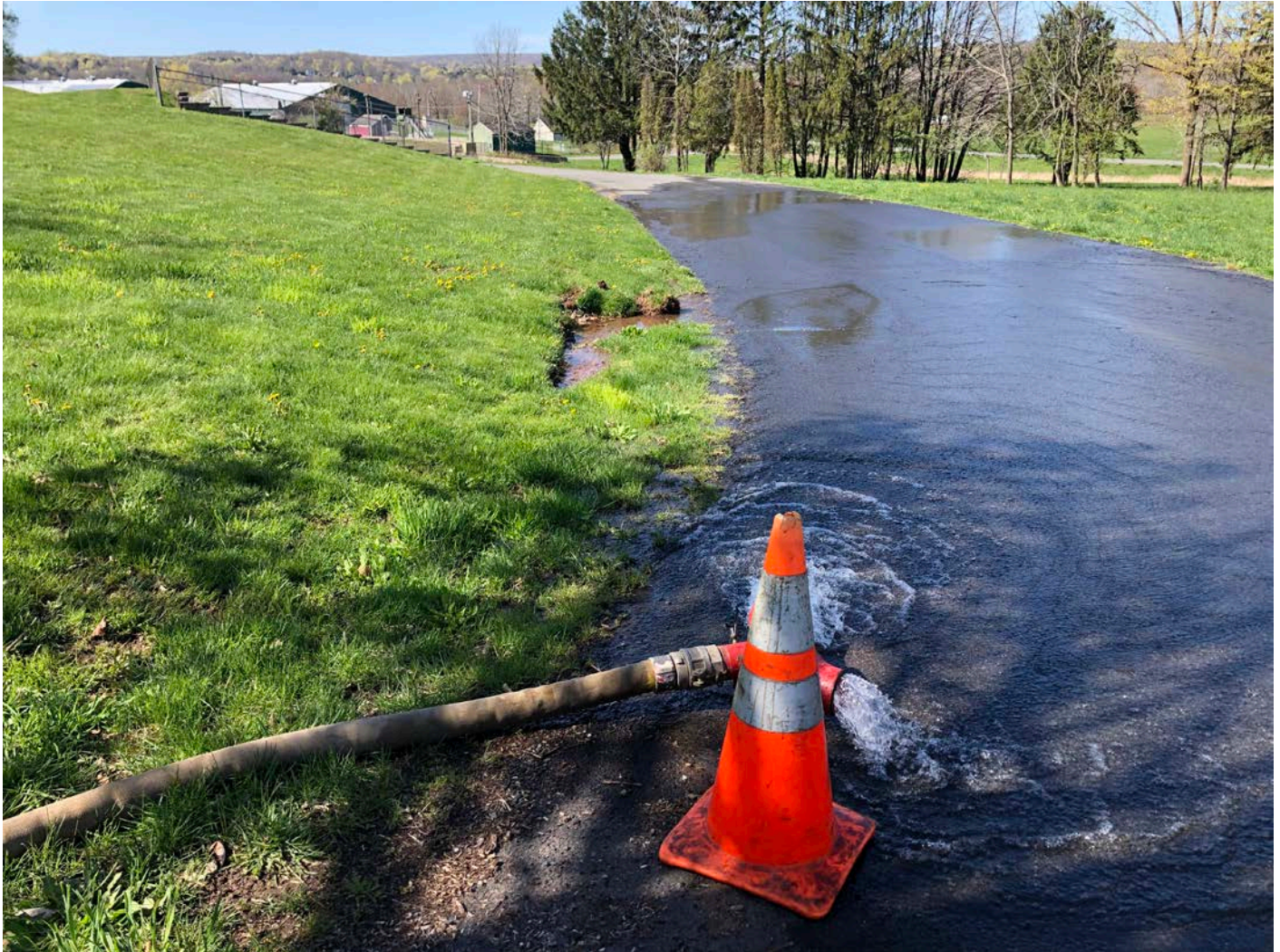
Picture 4: Ludlow discharging unchlorinated water that is being flushed onto the entrance to the Durham Fair grounds from the 12" DIP waterline on Maple Avenue as part of chlorination activities being performed by Ludlow today. View to the south/southwest.
