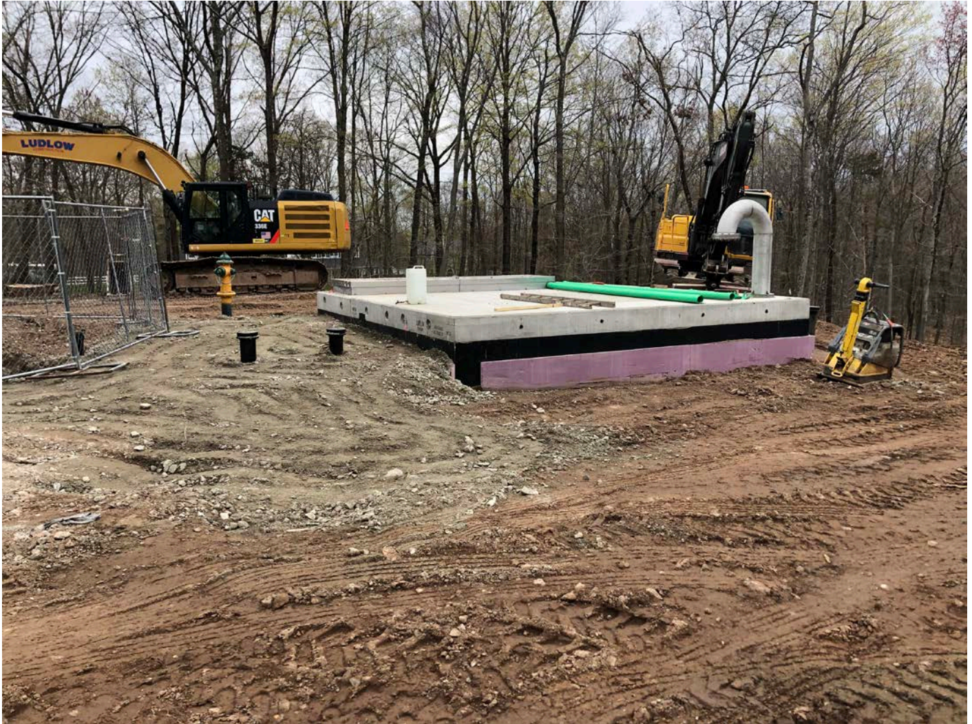
Picture 7: View of the altitude valve vault and the cover placed around its perimeter thus far. Water tank work zone located east of the Shared Access Driveway in Middletown. View to the southwest.
