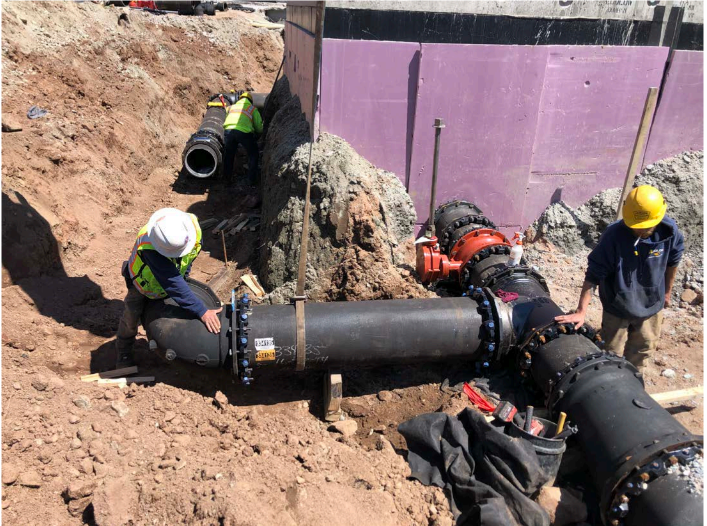
Picture 7: Ludlow working at the northwest corner of the altitude vault, installing 16" DIP for the bypass pipe that goes around the altitude valve vault to the north. Water tank work zone located east of the Shared Access Driveway in Middletown. View to the east.
