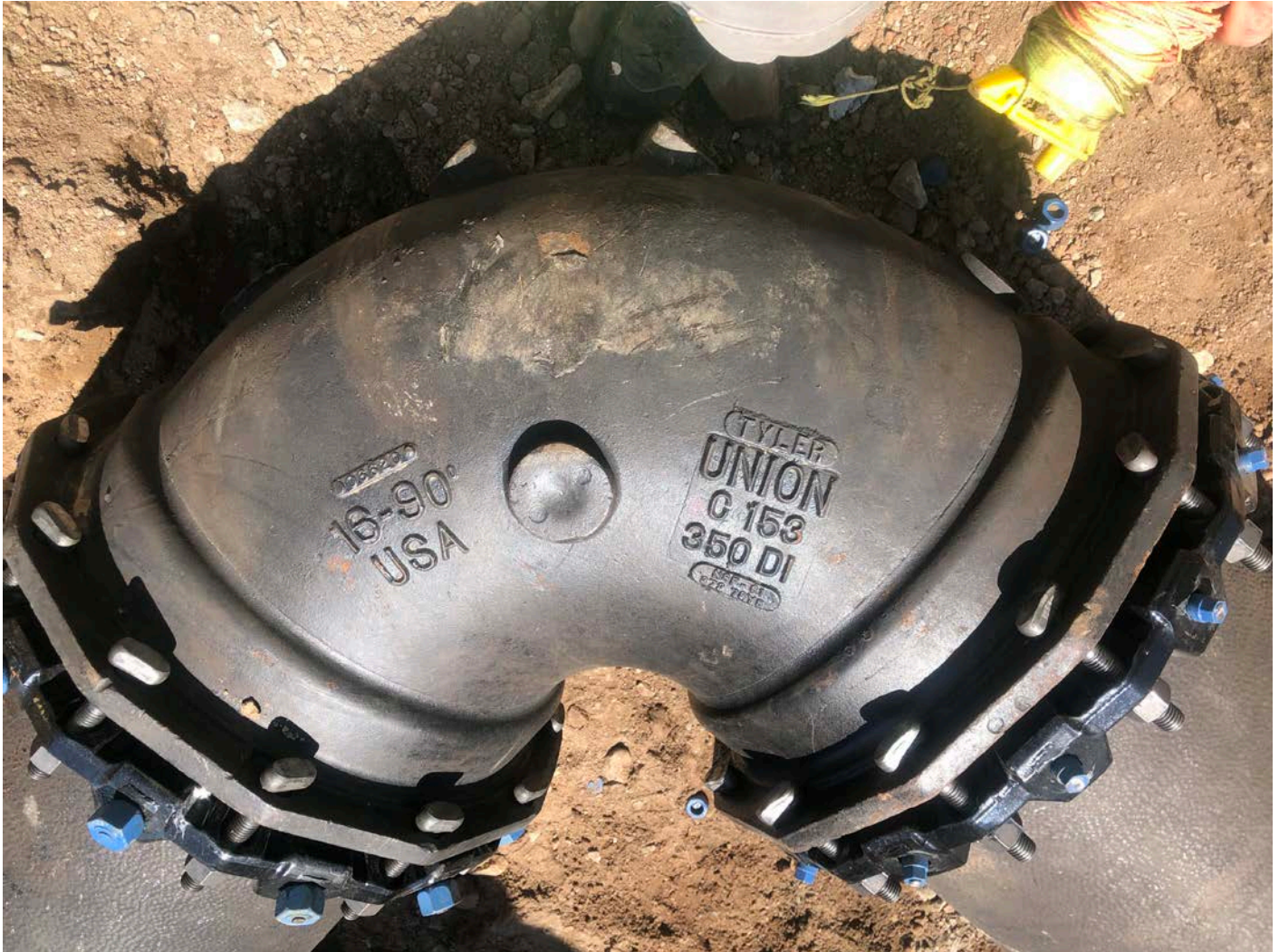
Picture 6: 90° elbow used in installing the 16" DIP used for the bypass pipe that goes around the altitude valve vault to the north. Water tank work zone located east of the Shared Access Driveway in Middletown.
