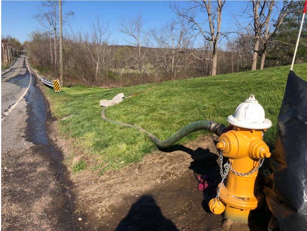
Picture 2: Ludlow flushing the 8" and 12" DIP waterline on Wallingford Road between Main Street and 47 Wallingford Road in Durham. Water is discharging into the adjoining wetland to the north of Wallingford Road. View to the west.
