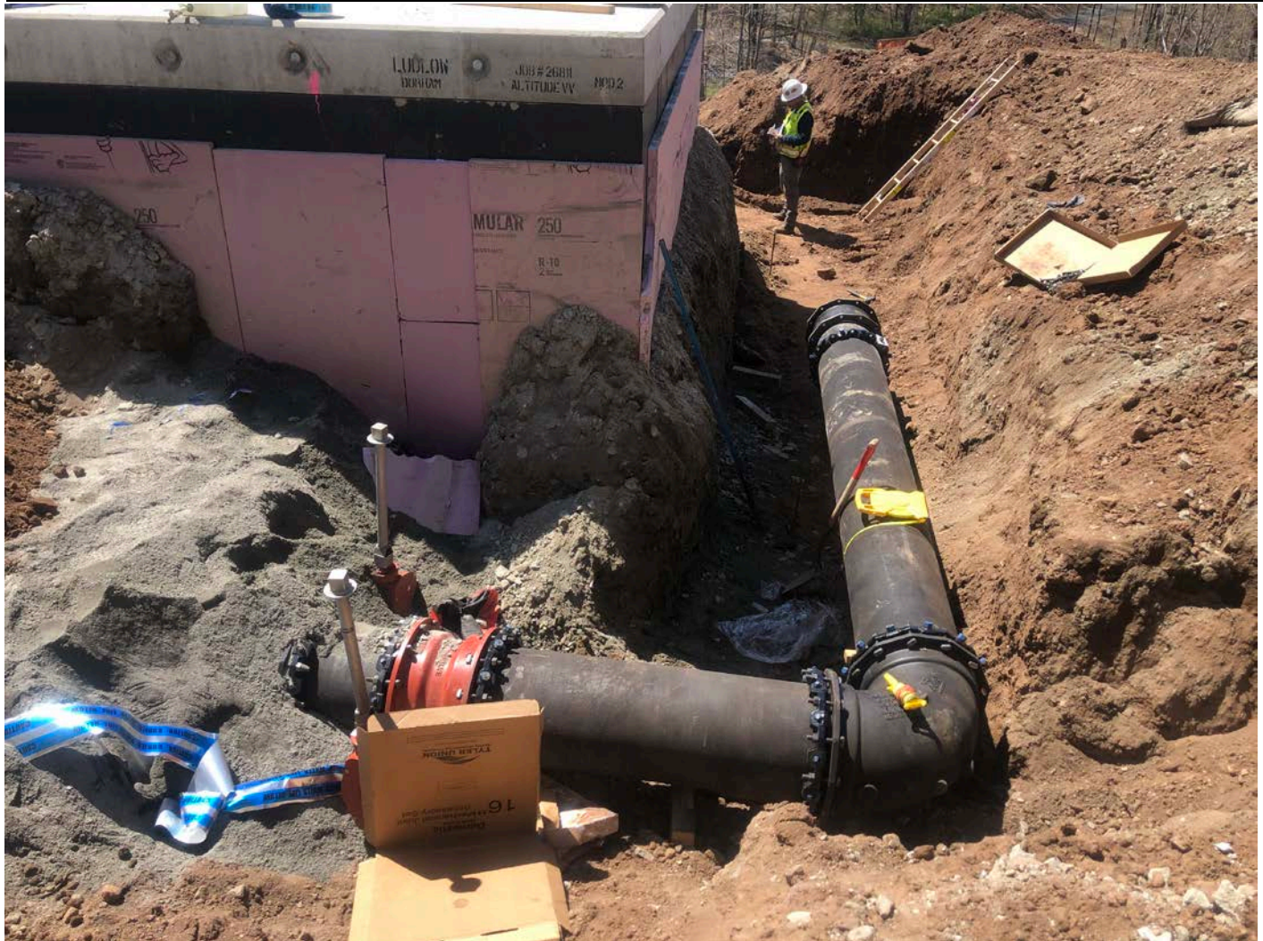
Picture 5: Ludlow in the process of installing 16" DIP for the bypass pipe that goes around the altitude valve vault to the north. Water tank work zone located east of the Shared Access Driveway in Middletown. View to the west.
