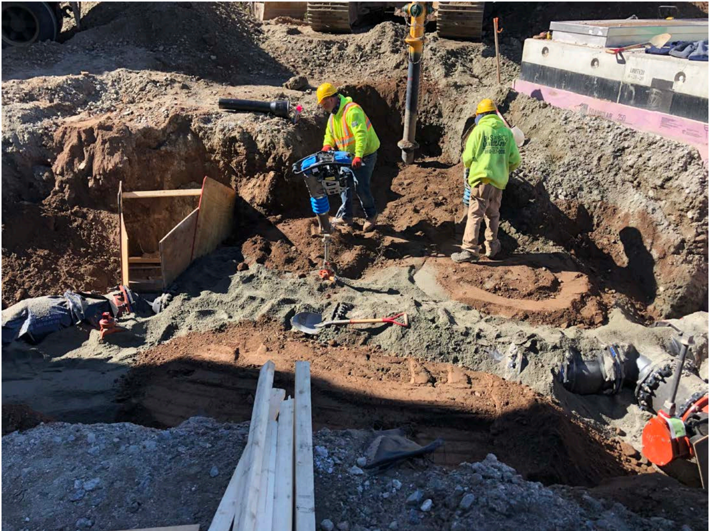
Picture 3: Ludlow compacting fill next to the hydrant they just installed with a jumping jack. Water tank work zone located east of the Shared Access Driveway in Middletown. View to the south.
