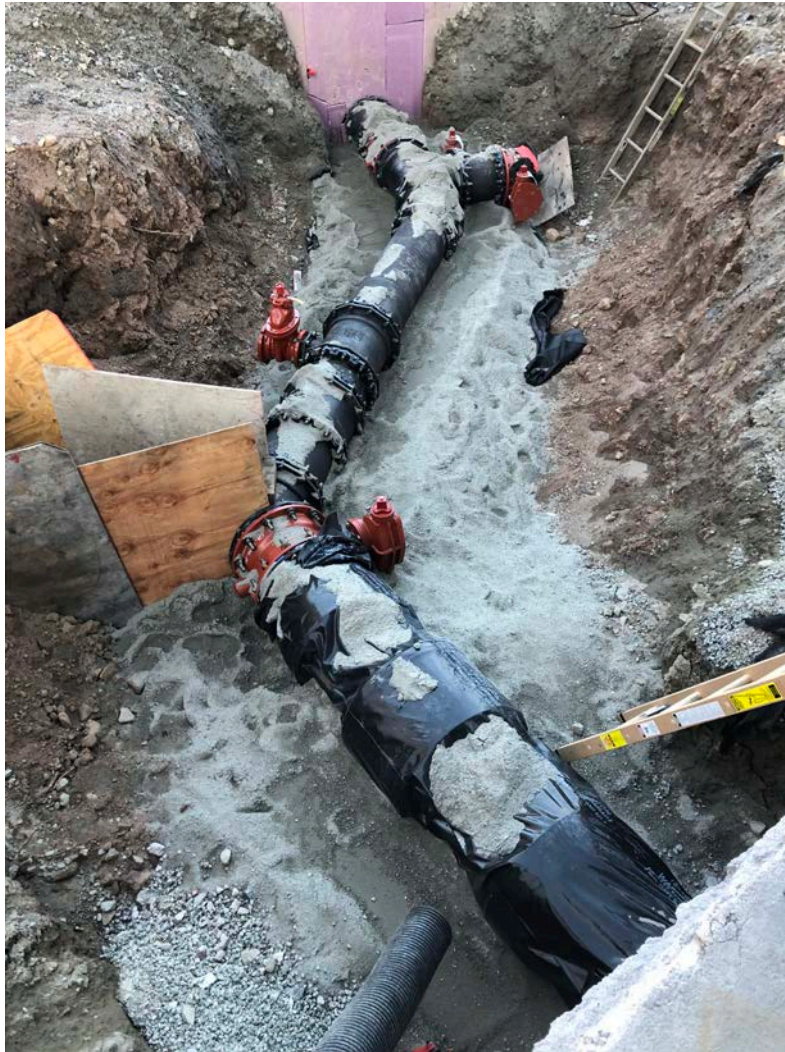
Picture 1: View of the 16" DIP that Ludlow installed between the altitude valve vault and the water tank located east of the Shared Access Driveway in Middletown. View to the west.
