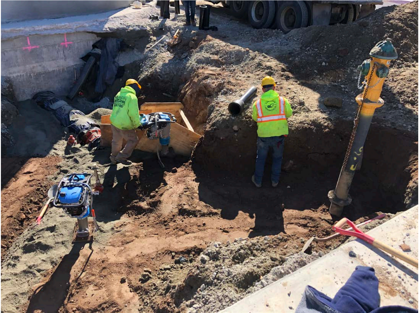
Picture 4: Ludlow compacting fill with a jumping jack next to the thrust block concrete form located between the altitude valve vault and the water tank. Water tank work zone located east of the Shared Access Driveway in Middletown. View to the southeast.
