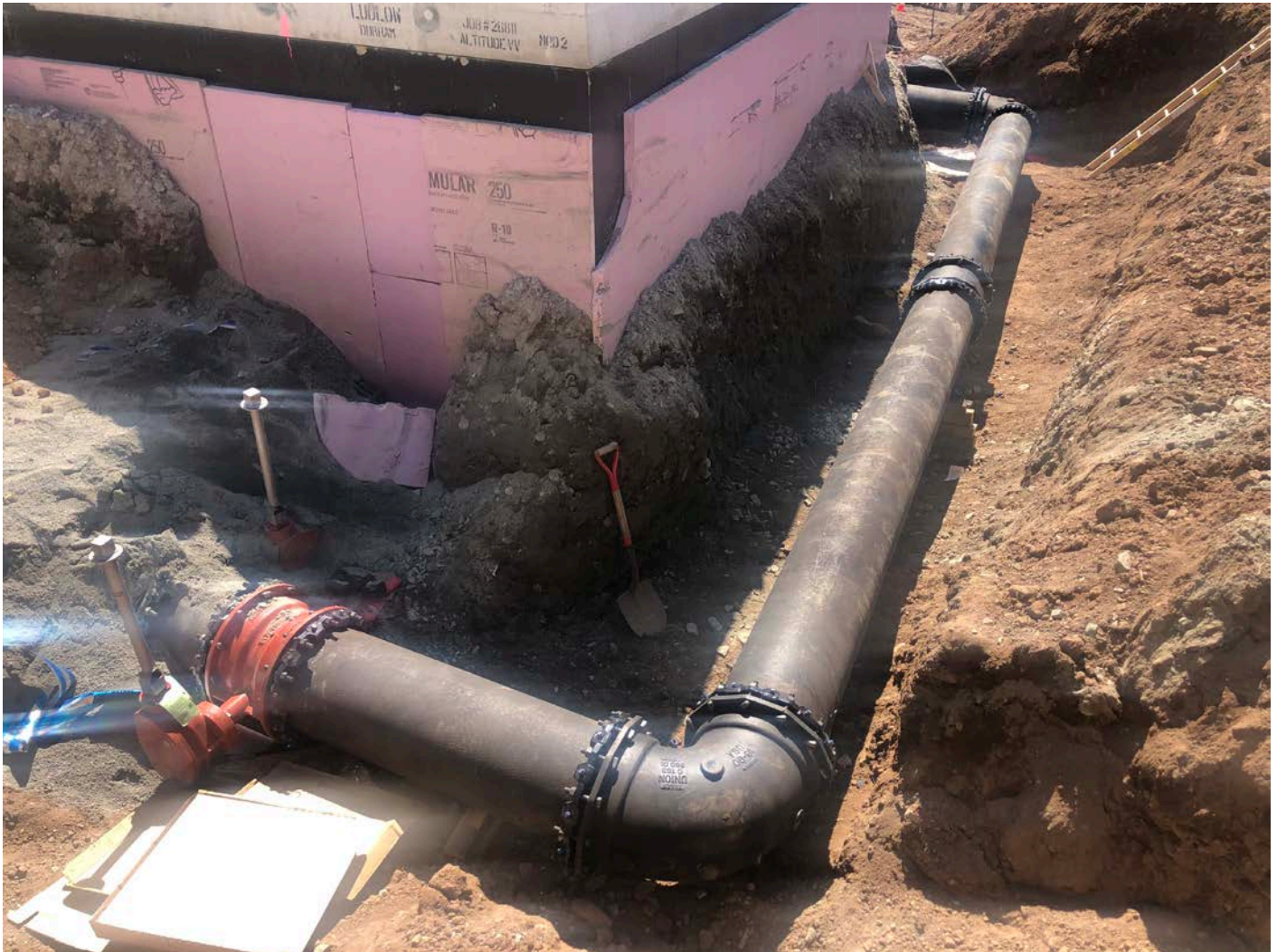
Picture 8: 16" DIP bypass pipe that Ludlow has installed around the north side of the altitude valve vault. Water tank work zone located east of the Shared Access Driveway in Middletown. View to the west.
