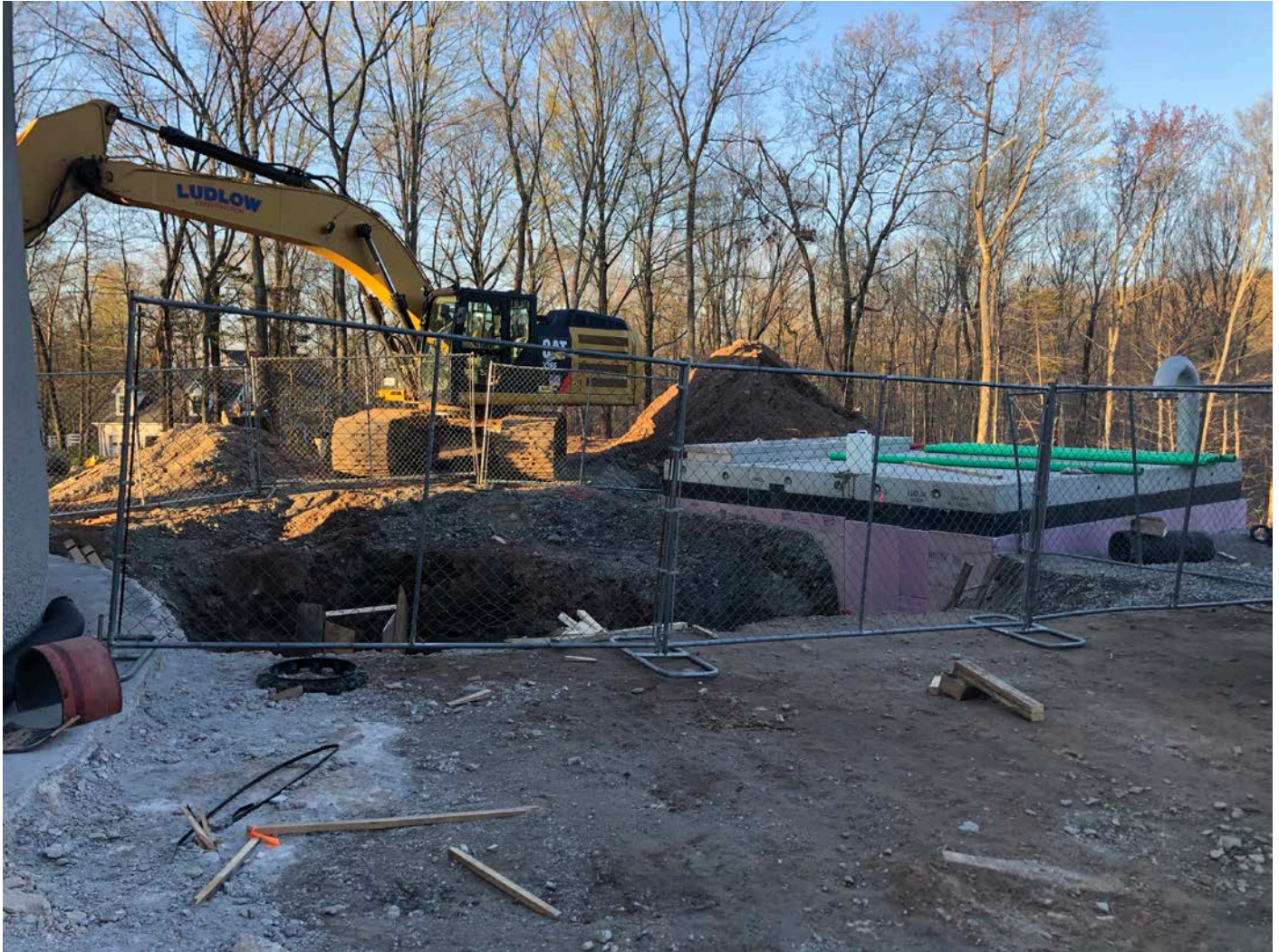
Picture 8: Excavation between the water tank to the altitude valve vault located east of the Shared Access Driveway, Middletown. Fencing was placed around the excavation at the end of the workday for security. View to the south.
