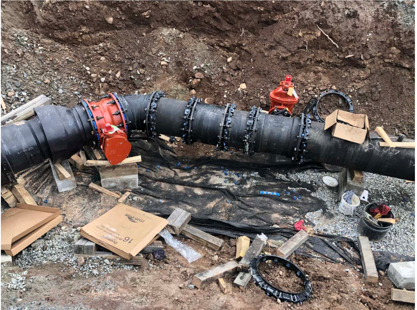
Picture 4: The last section of 16" DIP that Ludlow installed between the altitude valve vault to the water tank located to the east of the Shared Access Driveway in Middletown. View to the south.
