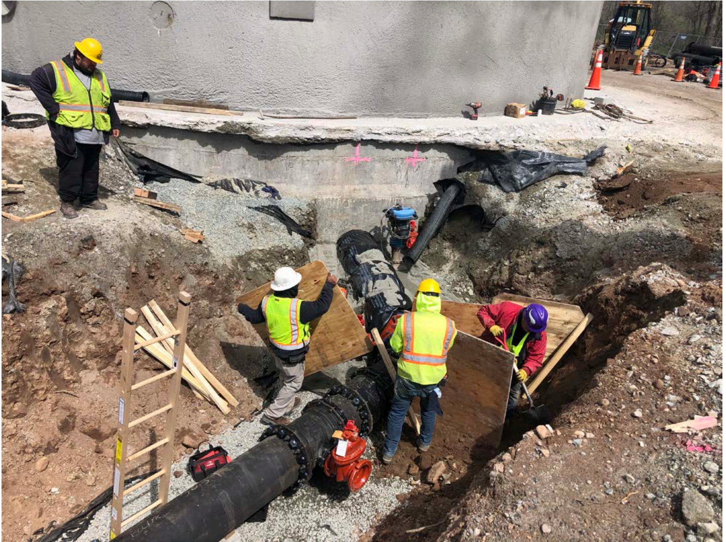
Picture 6: Ludlow building a form for concrete that will be poured to form a thrust block for the first bend of the 16" DIP located west of the 16" FLEX-TEND piping assembly. View to the east.
