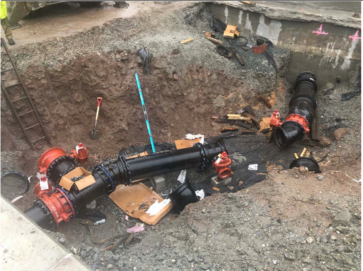
Picture 1: View of the piping that Ludlow installed yesterday between the altitude valve vault and the water tank located east of the Shared Access Driveway in Middletown. View to the northeast.
