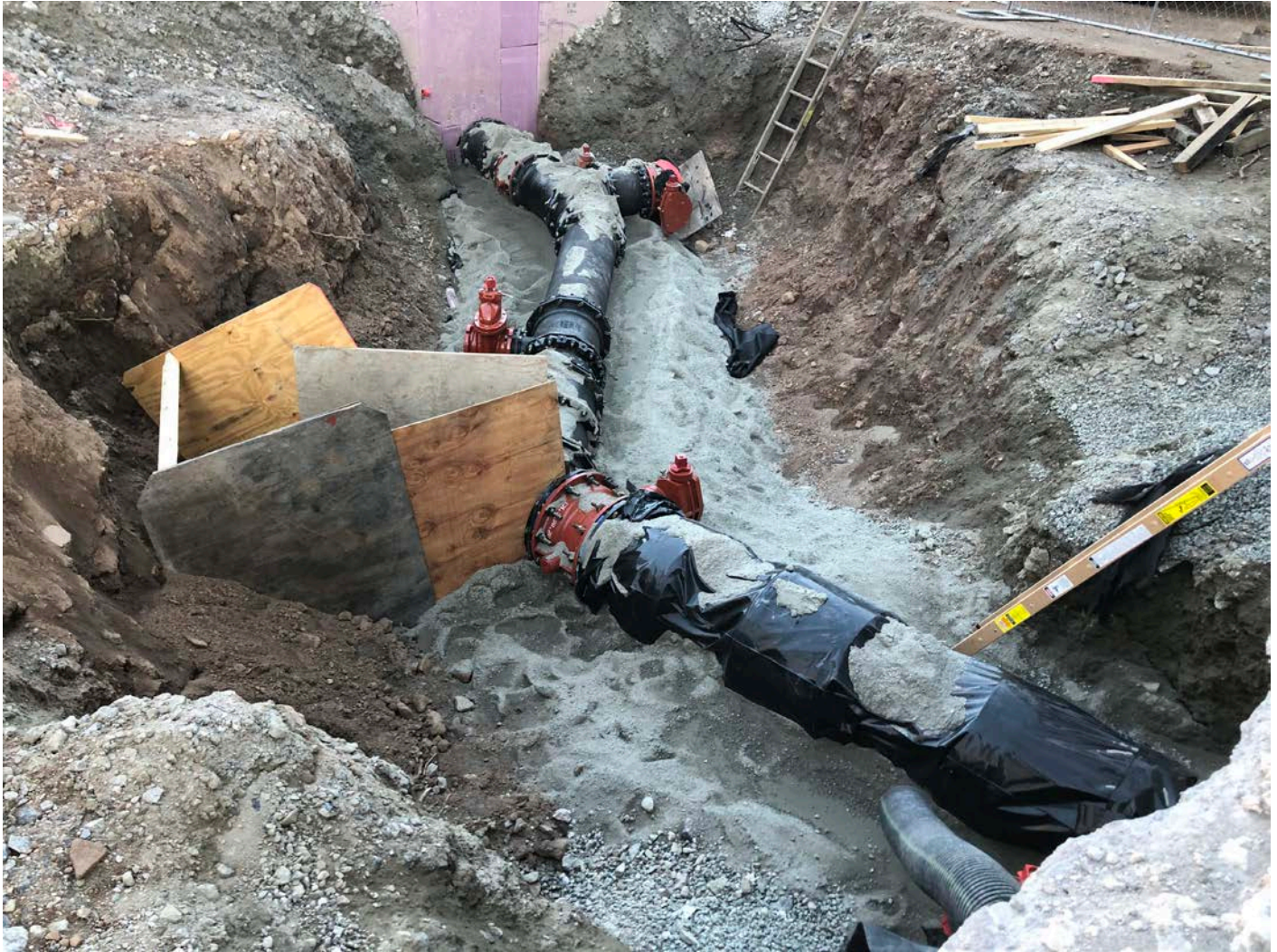
Picture 7: 16" DIP after Ludlow completed connecting the water tank to the altitude valve vault and placed geofabric, \frac{3}{4} ' gravel, and sand beneath the pipe. View to the west.
