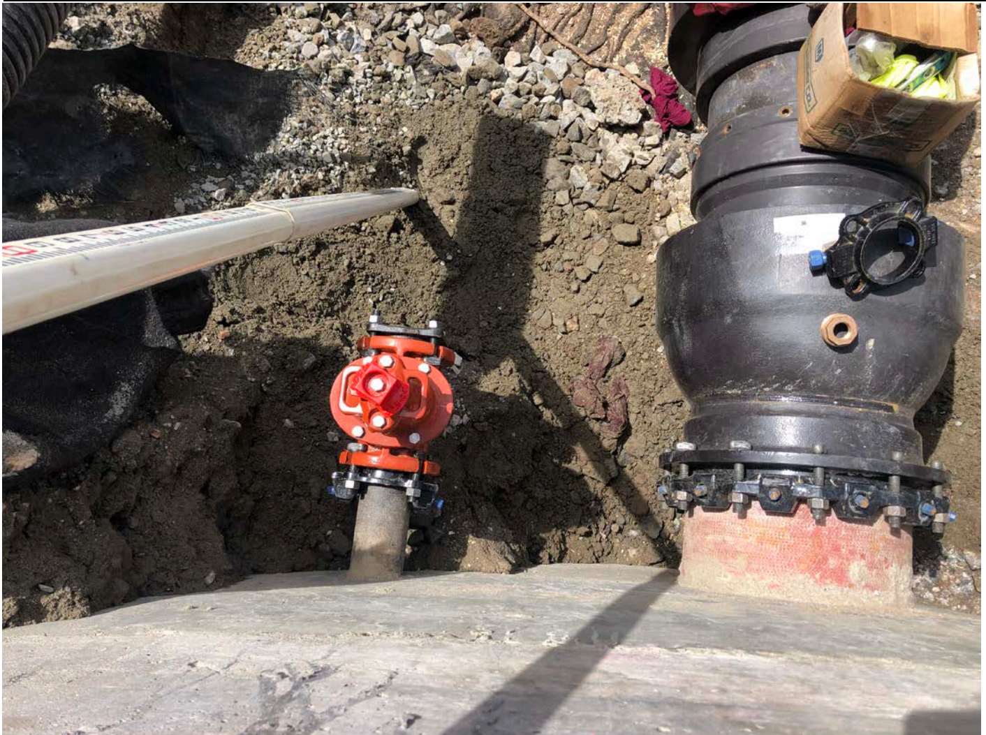
Picture 5: 3" gate valve that Ludlow has attached to the 3" DI tank level sensor line that protrudes from the west side of the water tank located east of the Shared Access Driveway in Middletown. View to the west.
