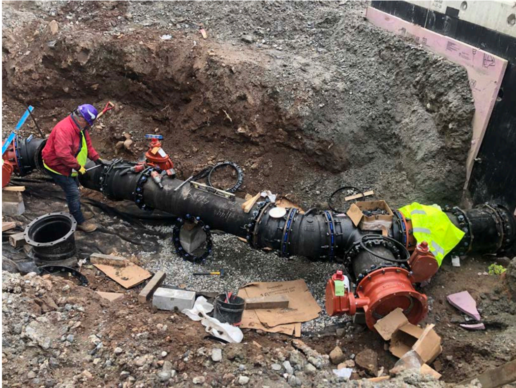
Picture 2: Ludlow tightening the bolts on a megalug restrained connection as they continue to install 16" DIP between the altitude valve vault and the water tank located east of the Shared Access Driveway in Middletown. View to the south.
