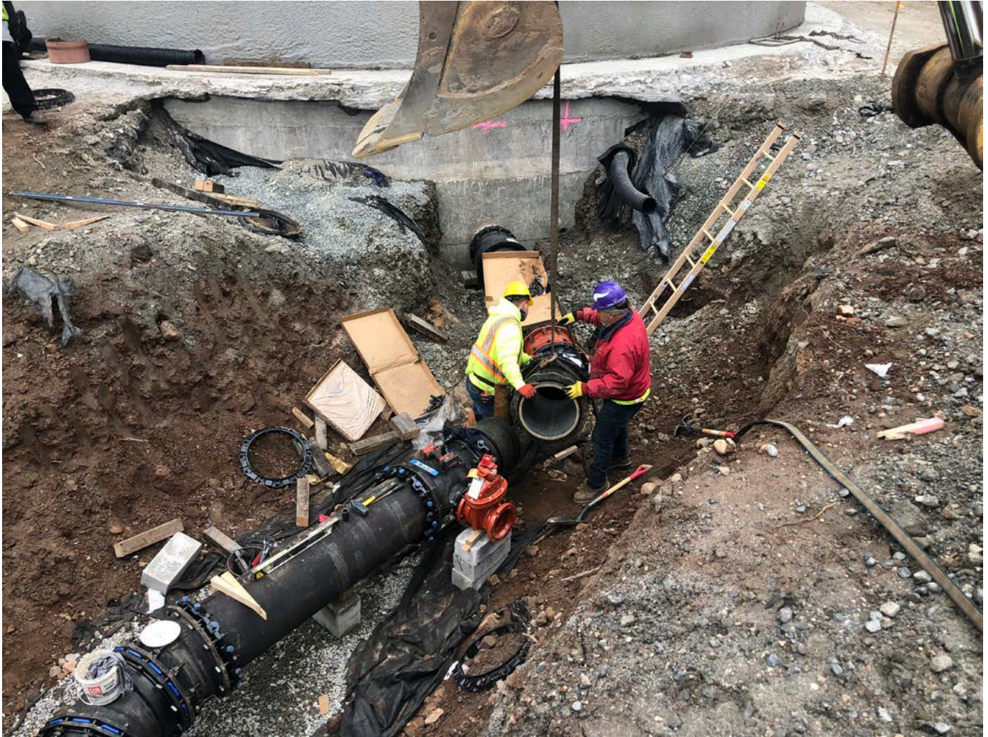
Picture 3: Ludlow continuing to install 16" DIP between the altitude valve vault and the water tank located east of the Shared Access Driveway in Middletown. View to the east.
