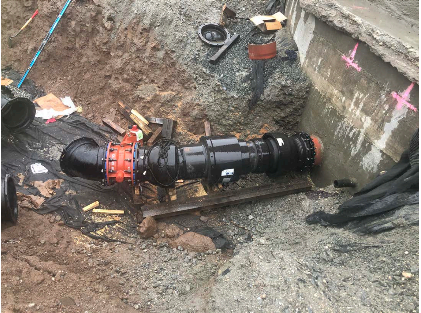
Picture 6: Final configuration of the 16" FLEX-TEND piping assembly with a foster adapter placed on either side of the 16" butterfly valve that was installed onto the 16" DIP protruding from the west side of the water tank. Water tank work zone located east of the Shared Access Driveway, Middletown. View to the north.
