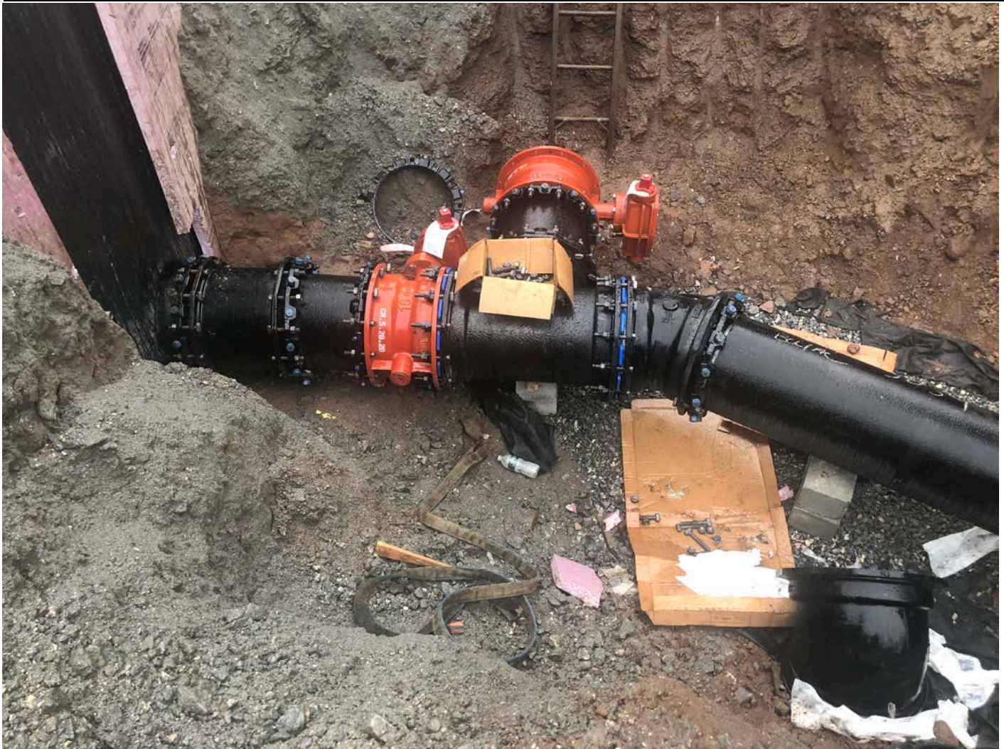
Picture 5: Final configuration of the 16" DIP that Ludlow attached to the east side of the altitude valve vault located east of the Shared Access Driveway in Middletown. Note foster adapters on either side of the 16"x16"x16" Tee. View to the north/northeast.
