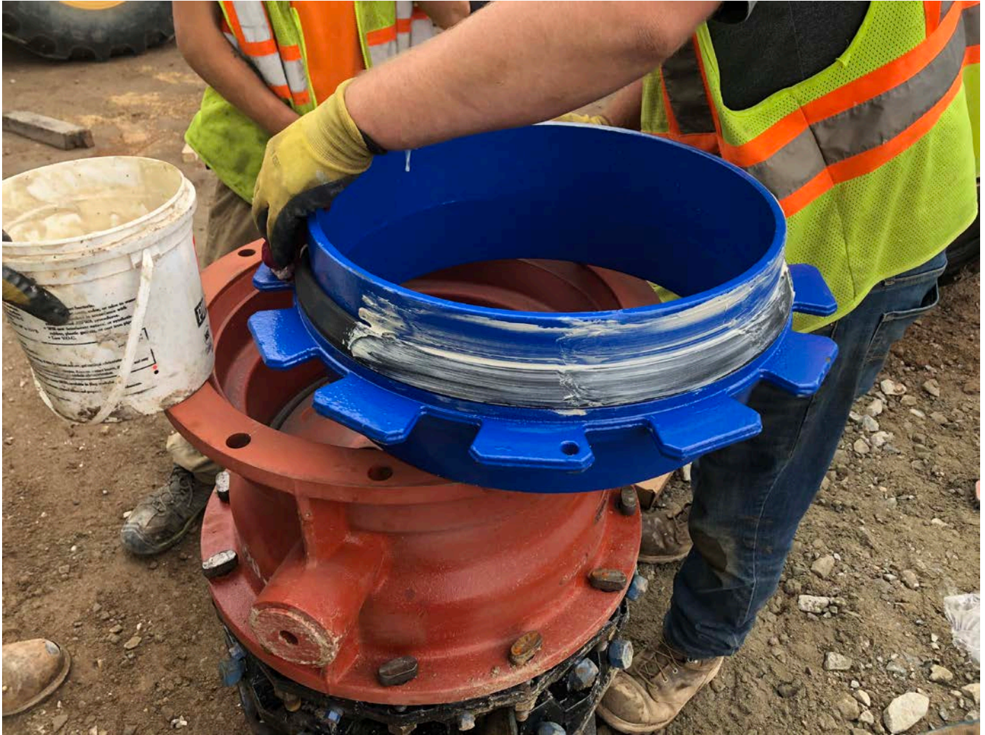
Picture 3: One of the 16" foster adapters that Ludlow used today while connecting the altitude valve vault to the water tank located east of the Shared Access Driveway in Middletown.
