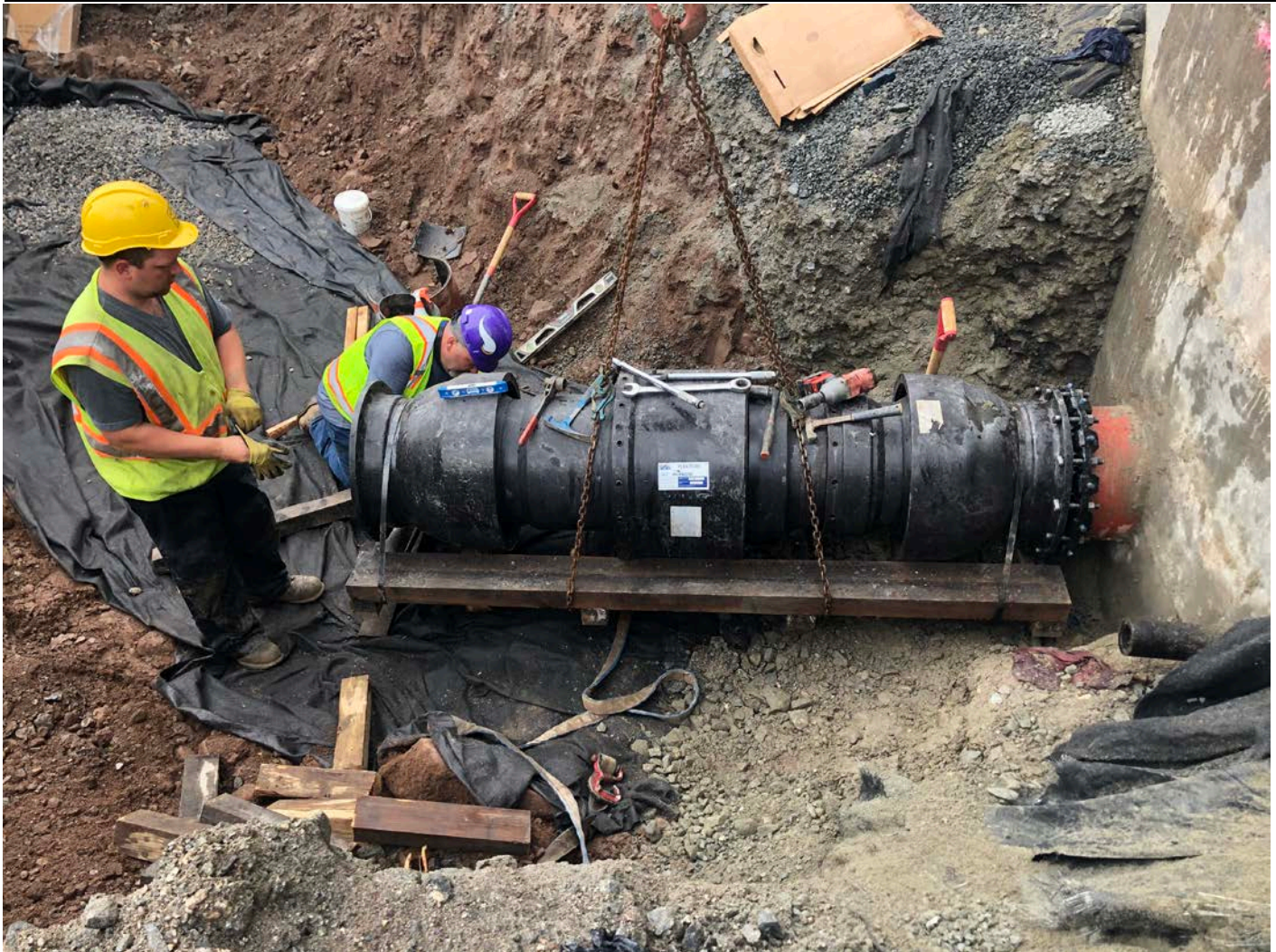
Picture 1: 16" FLEX-TEND piping assembly onto the 16" DIP protruding from the west side of the water tank located east of the Shared Access Road in Middletown. View to the north.
