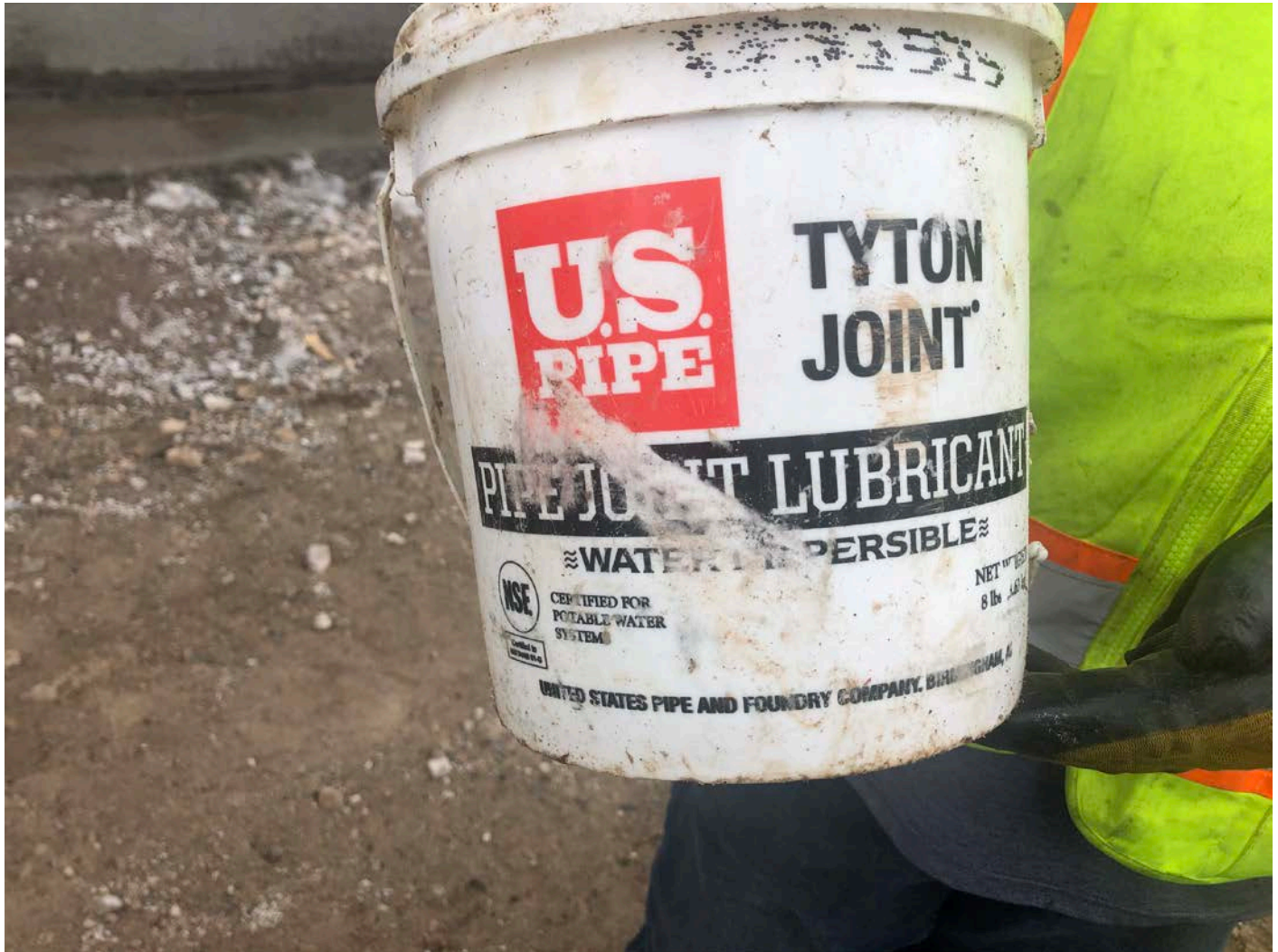
Picture 4: Pipe joint lubricant that Ludlow uses with the foster adapters and megalug connectors while connecting the altitude valve vault to the water tank located to the east of the Shared Access Driveway in Middletown.
