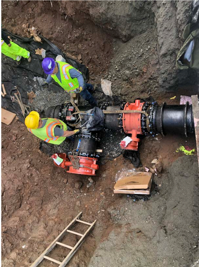
Picture 2: Ludlow dry-fitting 16" DIP and associated appurtenances on the east side of the altitude valve vault located east of the Shared Access Driveway in Middletown. Ludlow subsequently reconfigured this section using foster adapters.
