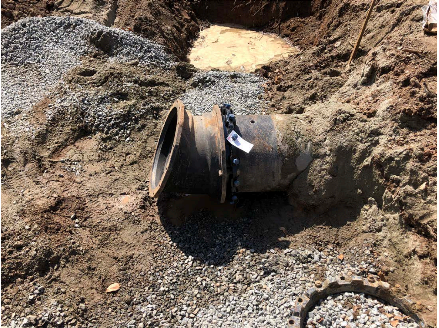
Picture 3: A 20", 22.5° MJ bend that Ludlow has attached to the east end of the 20" DIP that they installed last year at the water tank work zone. Location is west of the altitude valve vault and east of the Shared Access Driveway in Middletown. View to the south.
