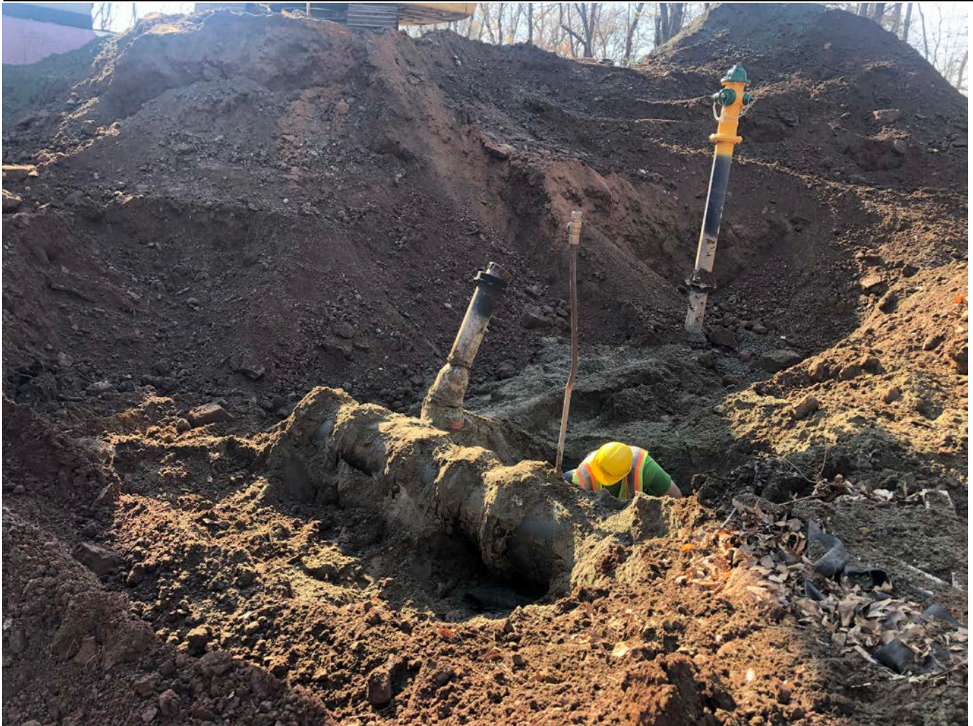
Picture 1: Section of 16" DIP (foreground) and 6" DIP (attached to the hydrant) that Ludlow daylighted as they prepare to remove the daylighted pipe. Location is west of the altitude valve vault and east of the Shared Access Driveway in Middletown. View to the south/southeast.
