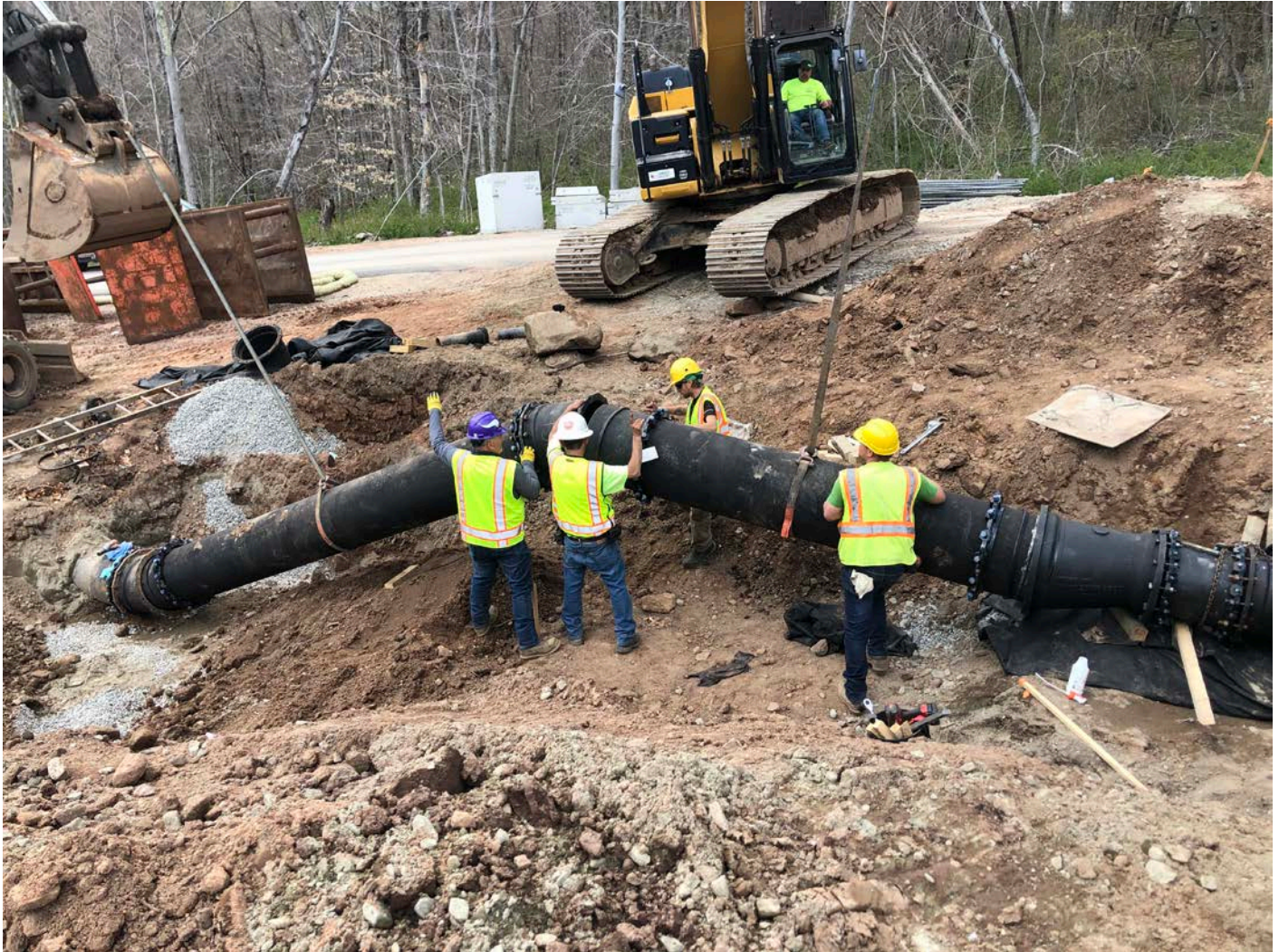
Picture 8: Ludlow finishing the connection between the previously-installed 20" DIP and the altitude valve vault with ~10' section of 20" DIP. View to the north/northwest.
