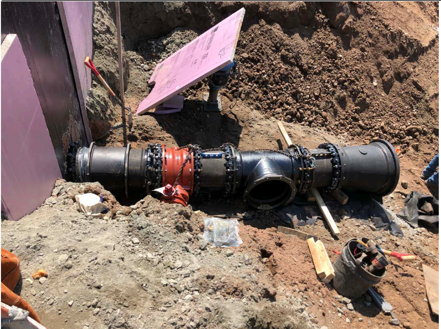
Picture 5: 16" DIP with a butterfly valve, a 16"x16"x16" TEE, and a 20"-to-16" reducer. that Ludlow connected to the 16" DIP protruding from the west side of the altitude valve vault located east of the Shared Access Driveway in Middletown. View to the south.
