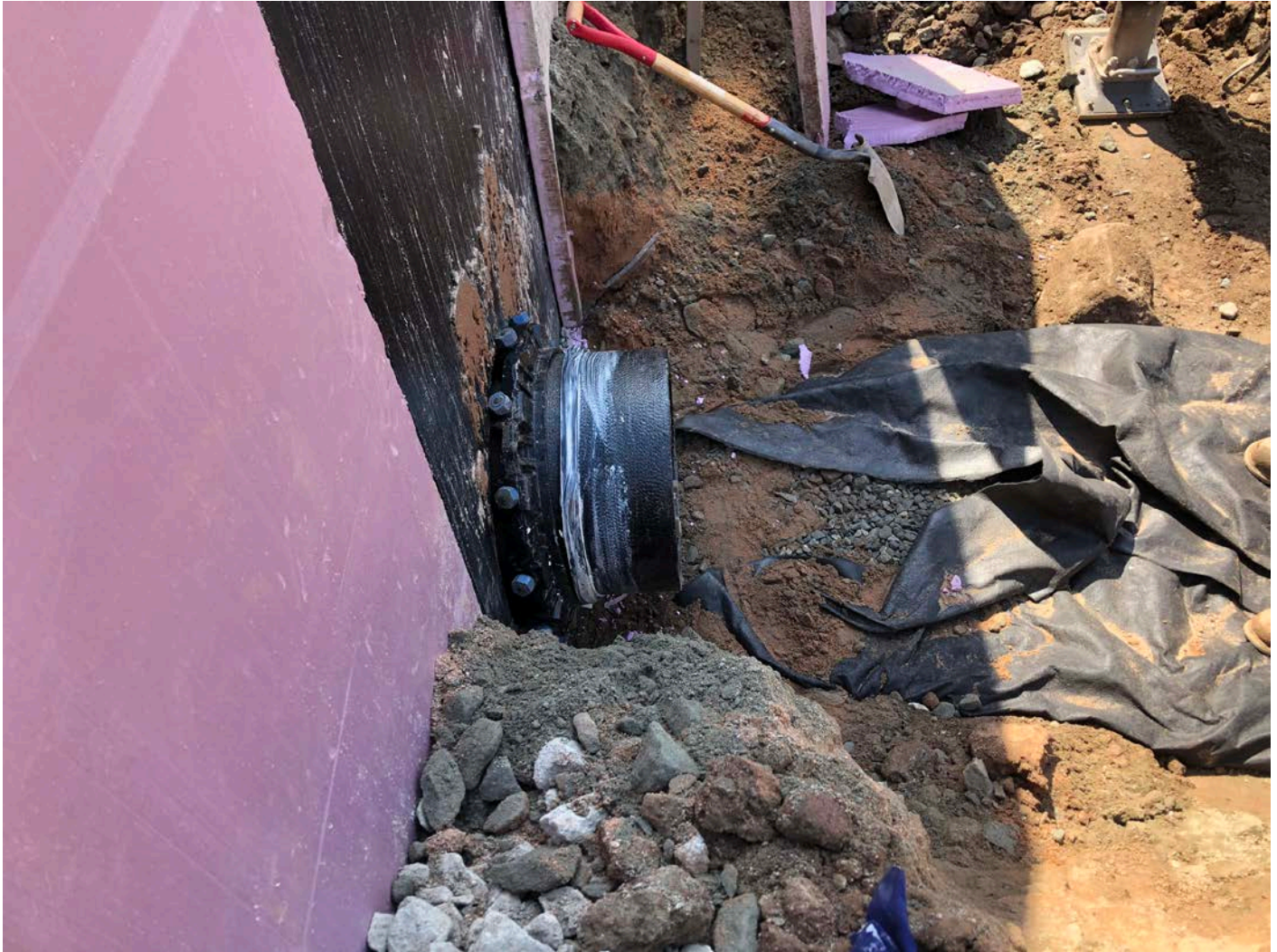
Picture 2: 16" DIP protruding from the west side of the altitude valve vault located east of the Shared Access Driveway in Middletown. Ludlow has placed a MJ gasket and a Megalug restrained gland onto the 16" DIP. View to the south.
