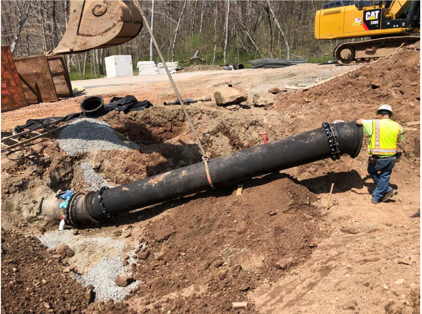
Picture 7: Ludlow connecting a section of 20" DIP (with a 22.5° DI MJ bend) to the previously-installed 20" DIP located west of the altitude valve vault at the water tank work zone located east of the Shared Access Driveway in Middletown.
