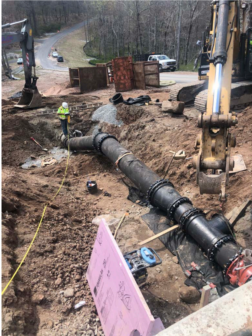
Picture 9: Overview of the 16" and 20" DIP that Ludlow installed today to connect the previously-installed 20" DIP to the altitude valve vault. View to the west.
