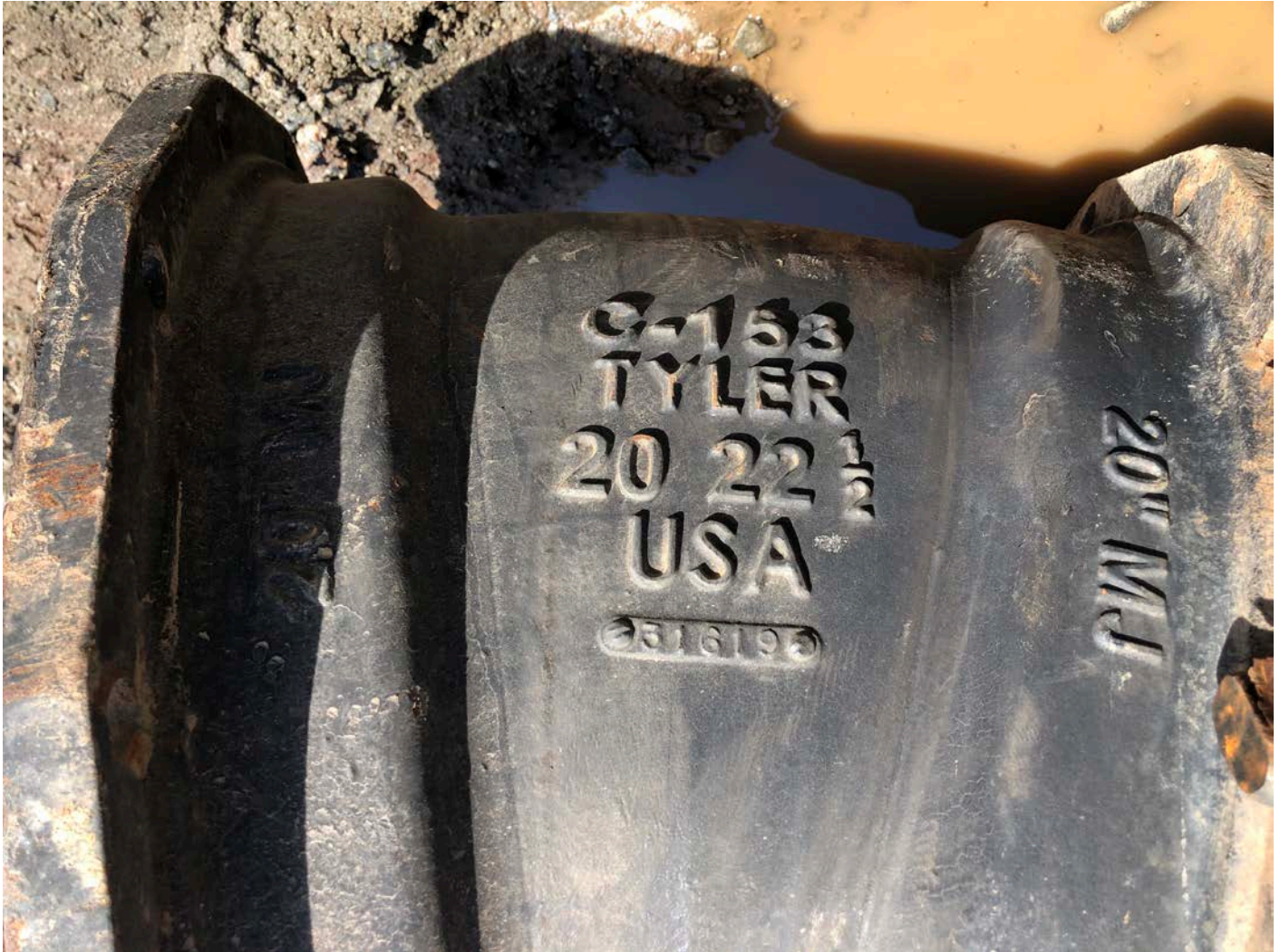
Picture 4: Close-up of the 20", 22.5° MJ DI bend that Ludlow attached to the east end of the 20" DIP they installed last year at the water tank work zone.
