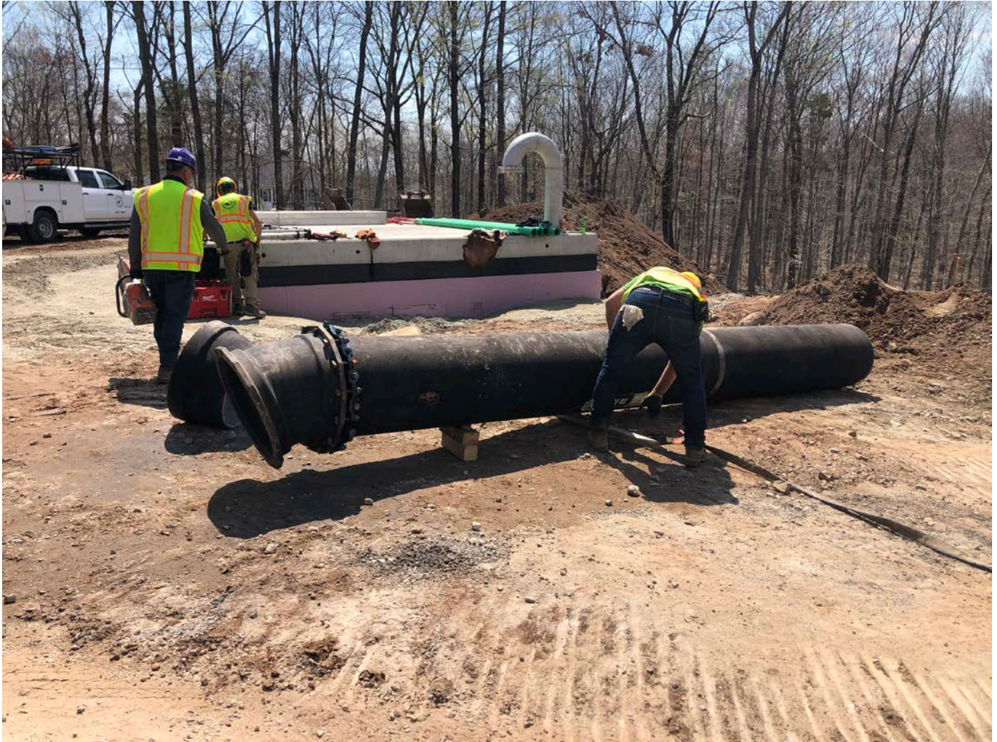
Picture 6: Ludlow placing lift strap on a section of 20" DIP, to which they connected a 22.5° DI MJ bend. Water tank work zone; view to the southwest.
