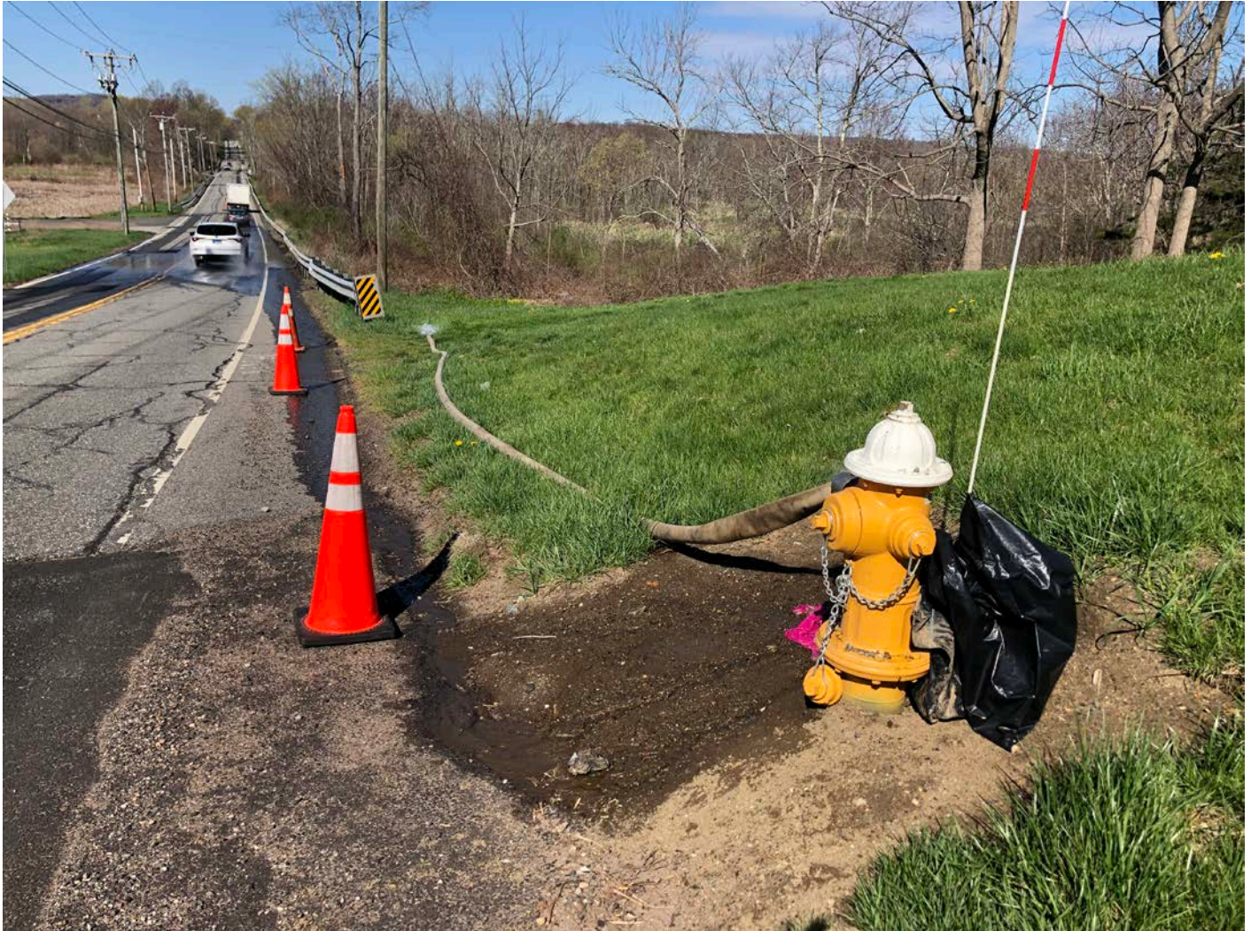
Picture 6: Ludlow in the process of flushing the 8" and 12" DIP waterlines located on Wallingford Road, Durham. Hydrant is located at Station 609+46. View to the west.
