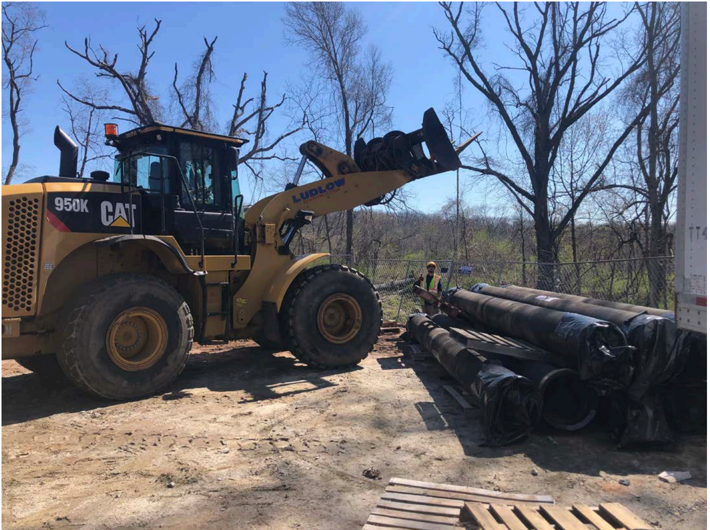
Picture 7: Ludlow staging 16" DIP at the southeast corner of the water tank work zone located east of the Shared Access Driveway in Middletown.
