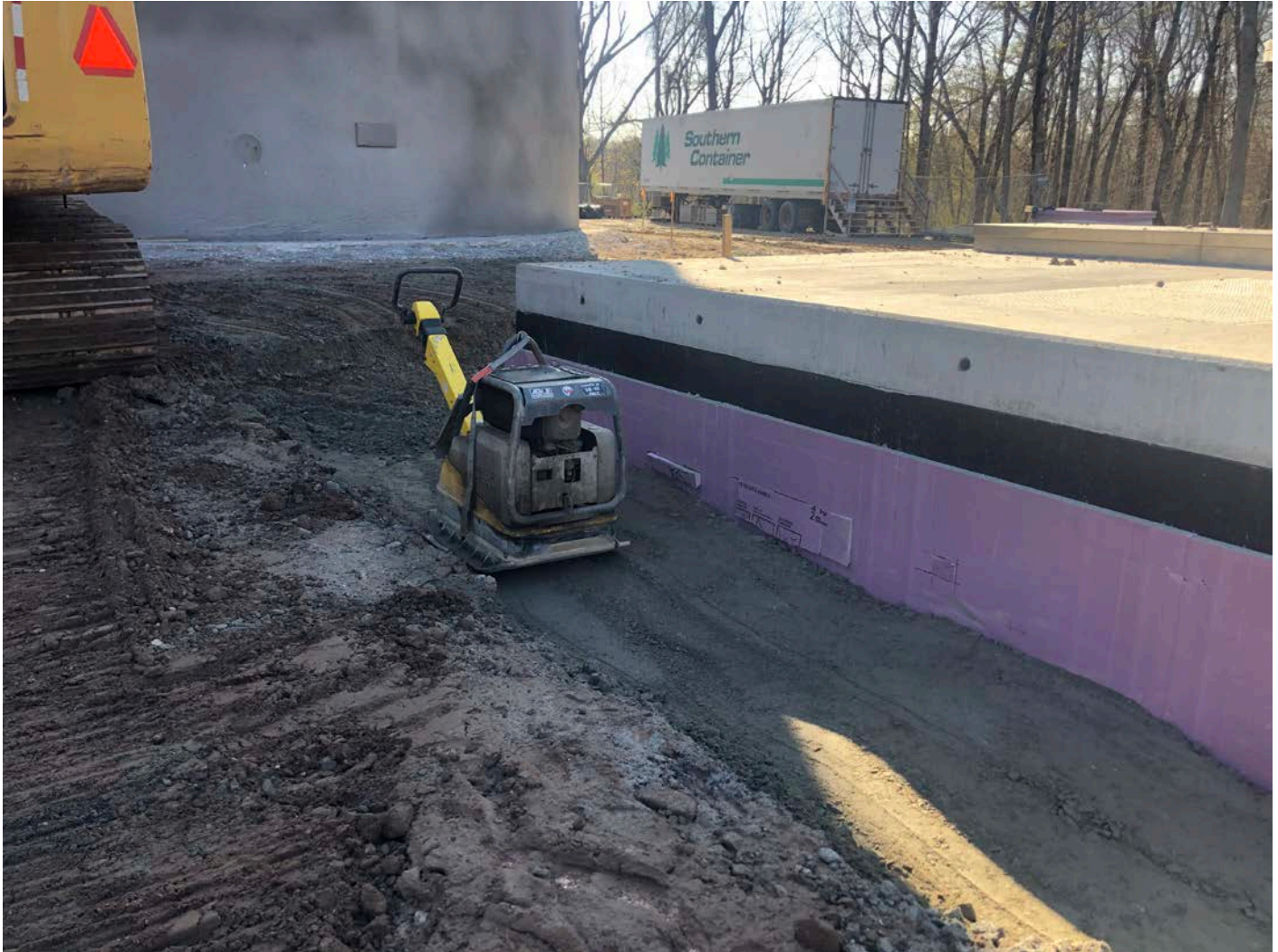
Picture 2: Ludlow compacting -3.5" gravel fill with a plate compactor that was placed around the north side of the altitude valve vault located east of the Shared Access Driveway in Middletown.
