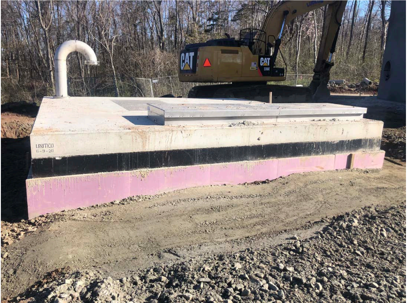
Picture 3: 3.5" gravel fill that has been placed and compacted around the south side of the altitude valve vault located east of the Shared Access Driveway in Middletown. View to the north.
