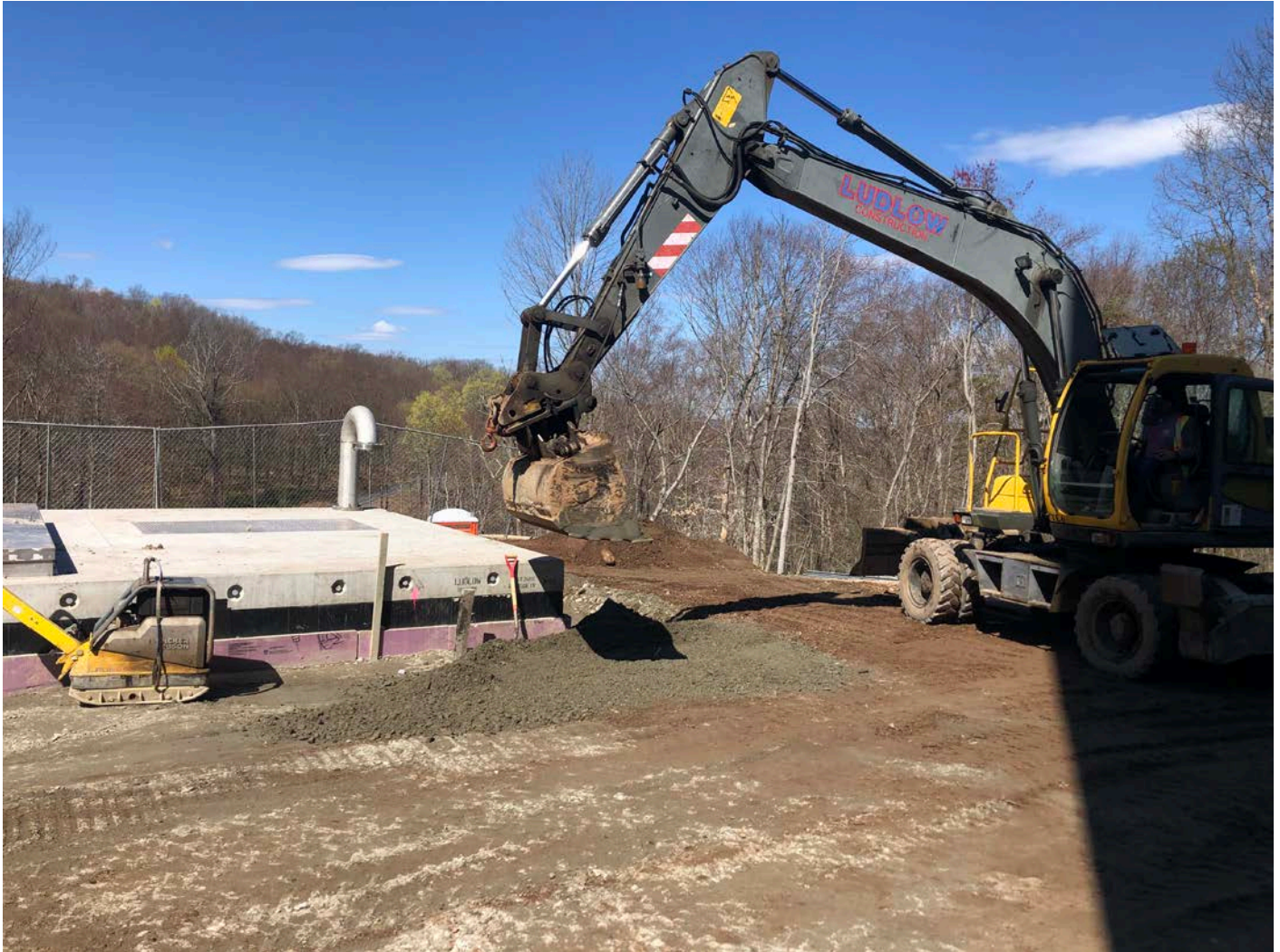
Picture 8: Ludlow placing and compacting -3.5" gravel on the east side of the altitude valve vault exterior. View to the northwest.
