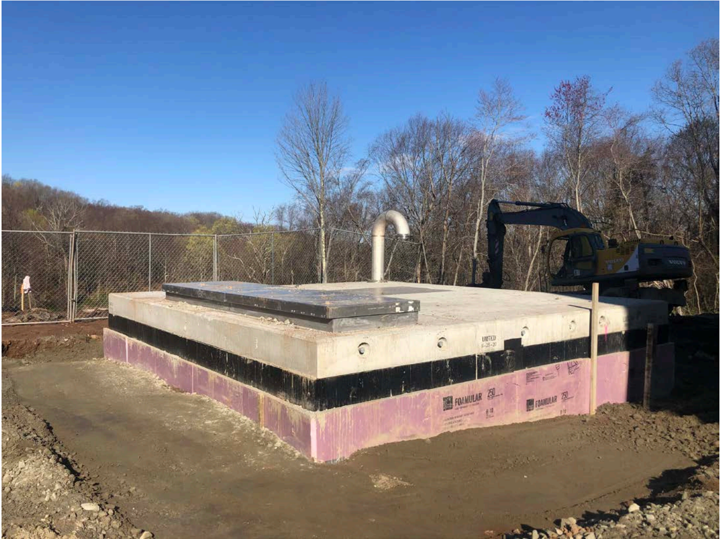
Picture 4: 3.5" gravel fill that has been placed and compacted around the south and east side of the altitude valve vault located east of the Shared Access Driveway in Middletown. View to the northwest.
