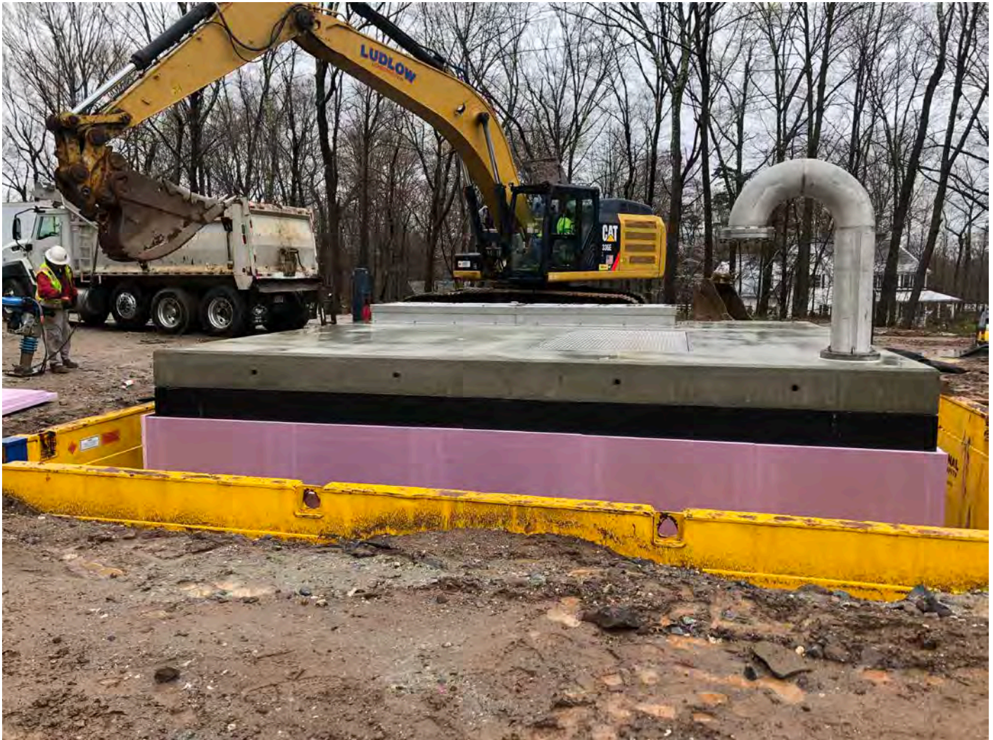
Picture 1: Ludlow having just placed 2" thick Owens Corning Foamular 250 XPS around the foundation of the altitude vault east of the Shared Access Driveway in Middletown. View to the south.
