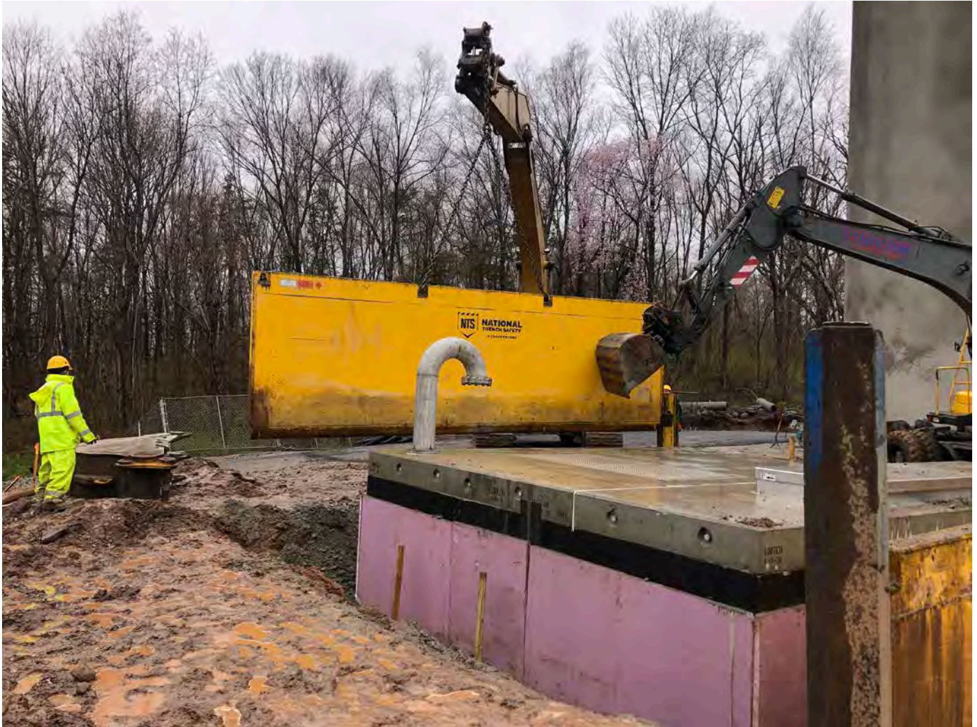
Picture 7: Ludlow in the process of raising the northern side panel on the trench box surrounding the altitude valve vault as they place and compact -3.5" gravel around the exterior of the vault. East of the Shared Access Driveway, Middletown. View to the north.
