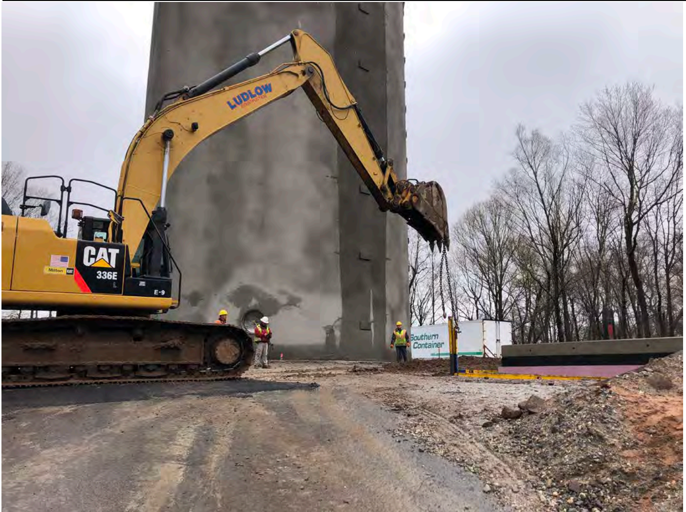
Picture 5: Ludlow removing the northeast slide rail post from the trench box surrounding the altitude valve vault as they backfill around east of the Shared Access Driveway in Middletown; view to the southeast.
