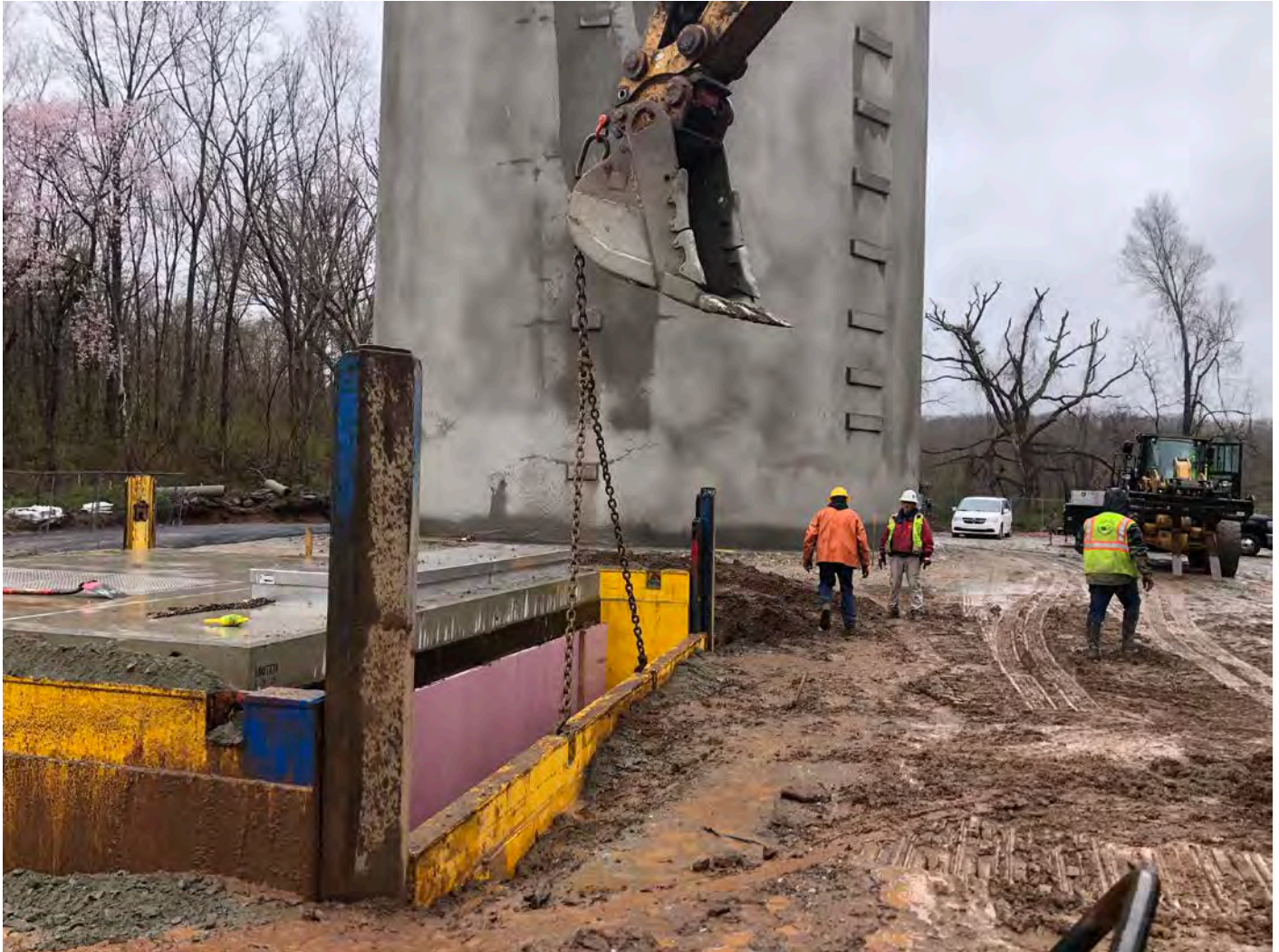
Picture 6: Ludlow in the process of raising the southern side panel on the trench box surrounding the altitude valve vault as they place and compact -3.5" gravel around the exterior of the vault. East of the Shared Access Driveway, Middletown. View to the east.
