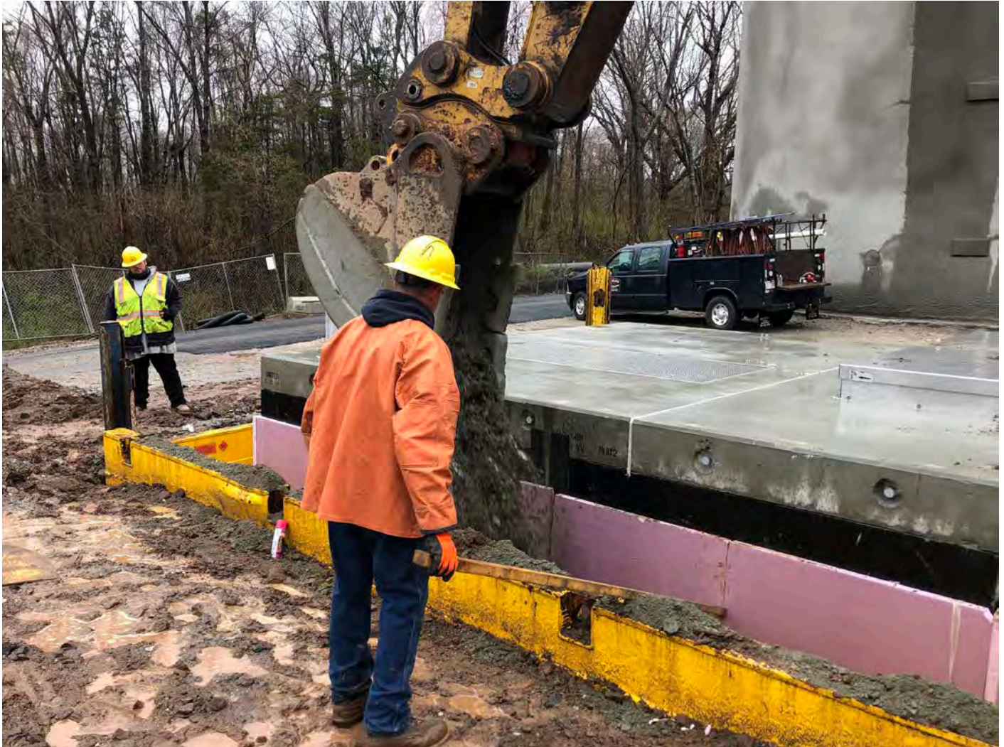
Picture 3: Ludlow placing -3.5" gravel fill around the outside of the altitude valve vault located east of the Shared Access Driveway in Middletown. View to the southeast.
