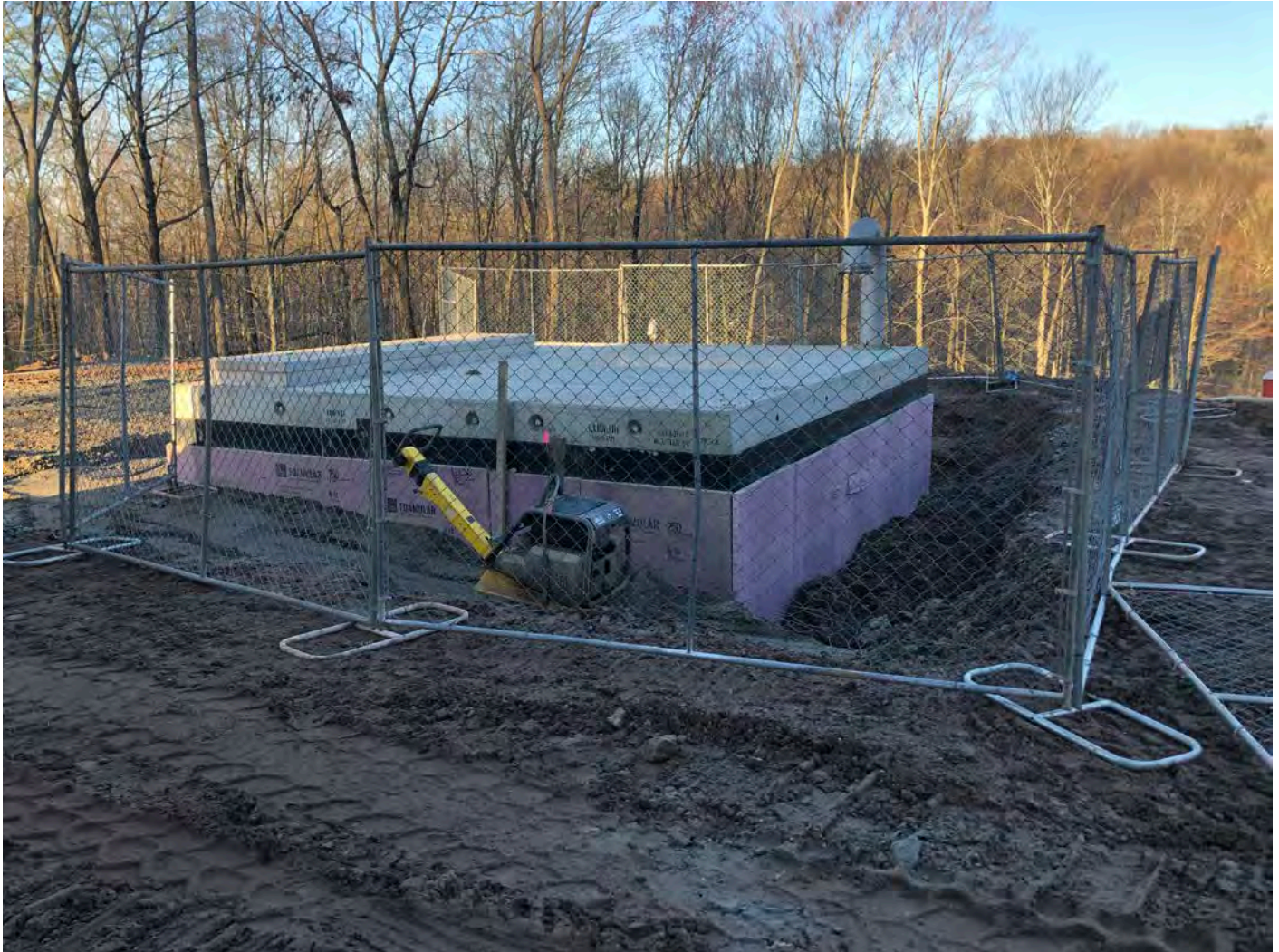
Picture 8: Altitude valve vault after Ludlow placed and compacted fill around the vault exterior. Ludlow secured the vault at the end of the day with temporary fencing. East of the Shared Access Driveway, Middletown. View to the southwest.
