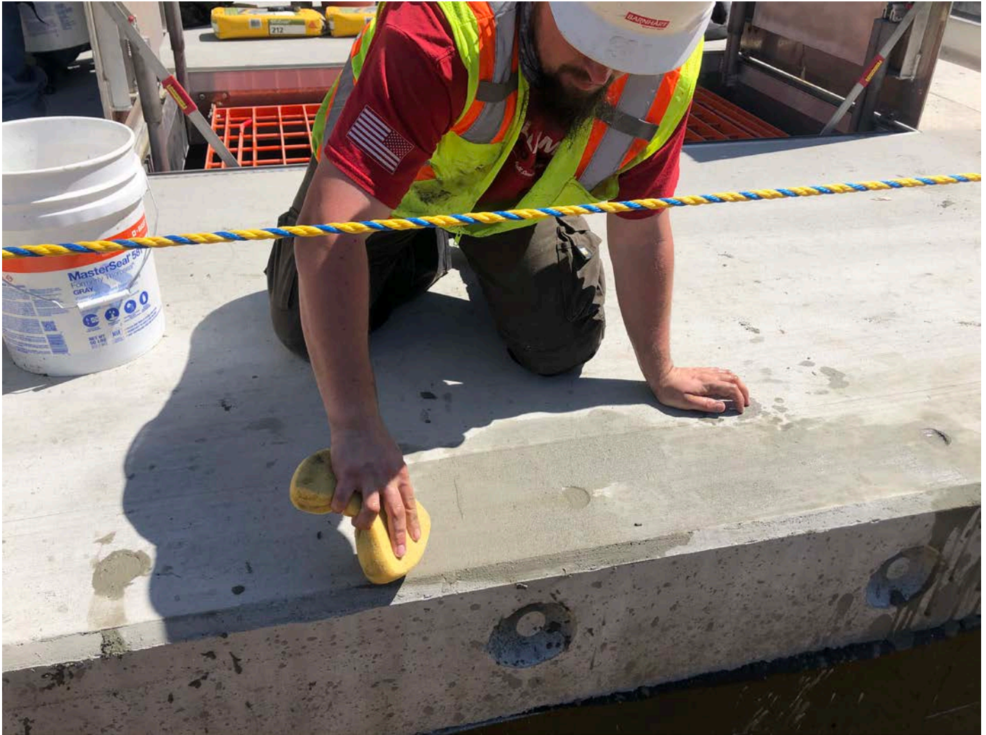
Picture 10: United Concrete cleaning away excess grout that was poured over the rebar sections that were secured with Hilti epoxy on the altitude valve vault located east of the Shared Access Driveway, Middletown.
