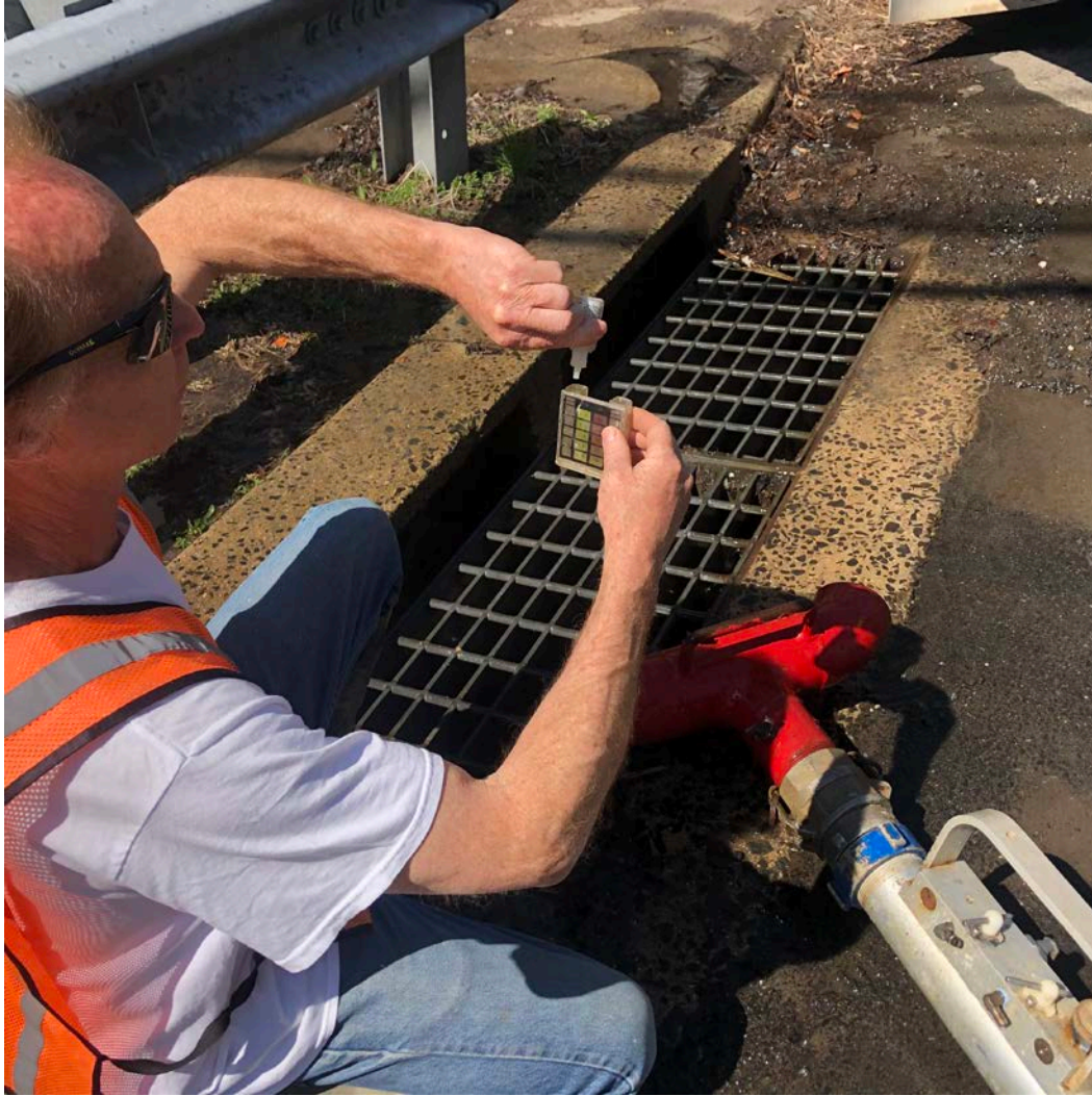
Picture 7: JMS is dechlorinating water that is being purged from the Main Street water line with calcium thiosulphate prior to discharging it and is testing the water frequently for residual chlorine.
