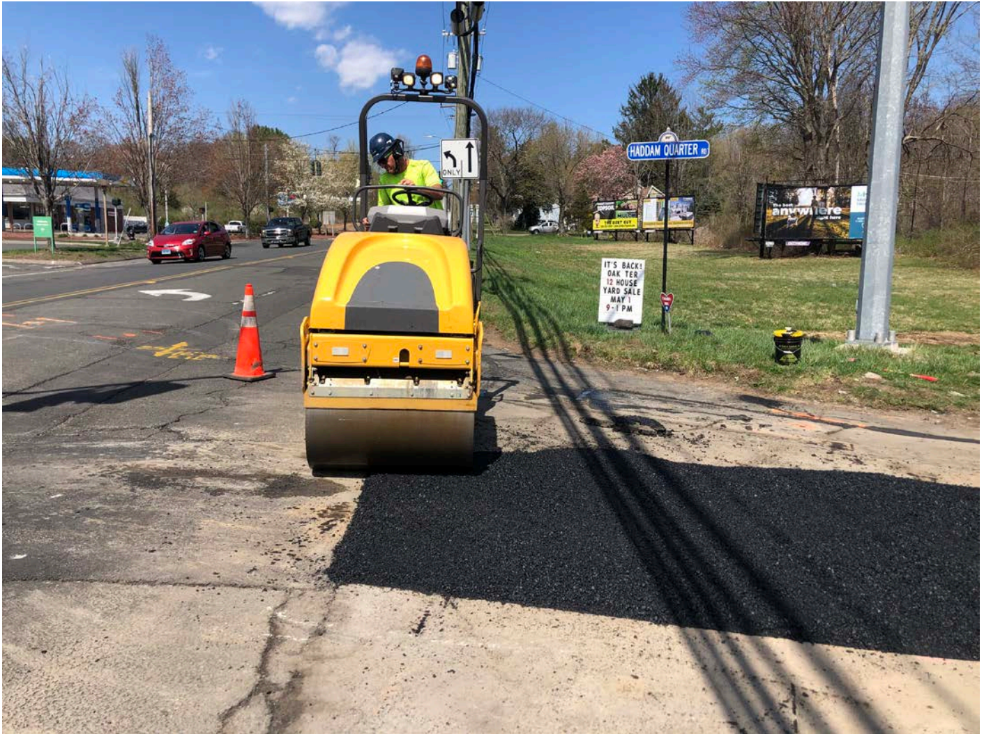
Picture 12: Ludlow compacting asphalt on the trench overcut on Haddam Quarter Road in Durham as part of permanent paving activities. View to the north.
