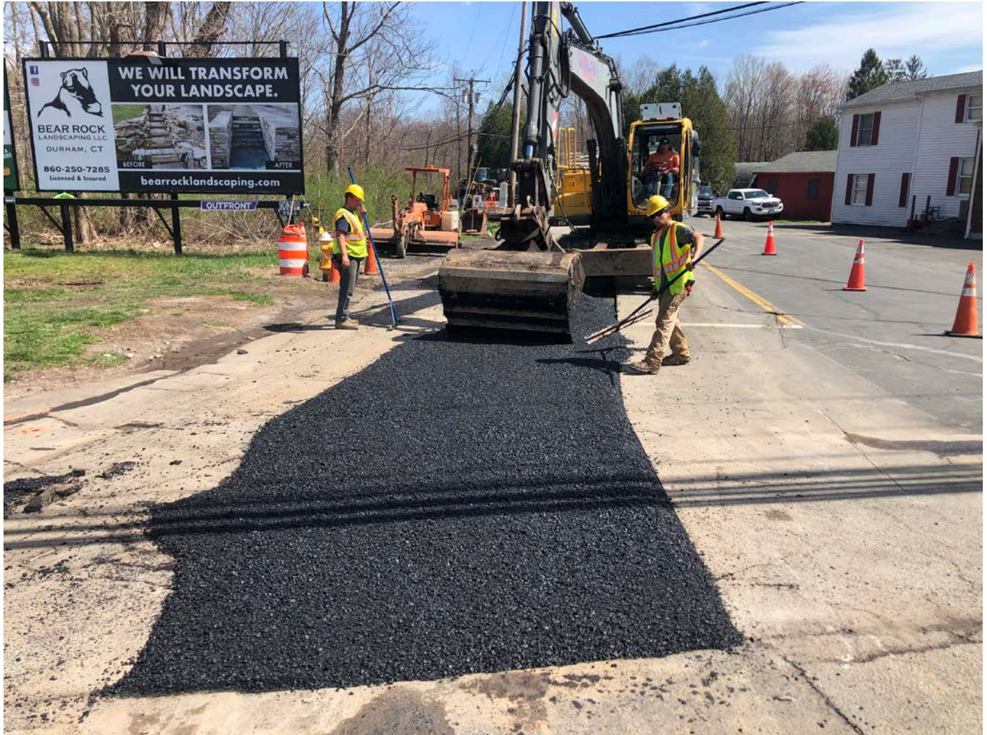
Picture 11: Ludlow placing asphalt on trench overcut on Haddam Quarter Road in Durham as part of permanent paving activities. View to the east.
