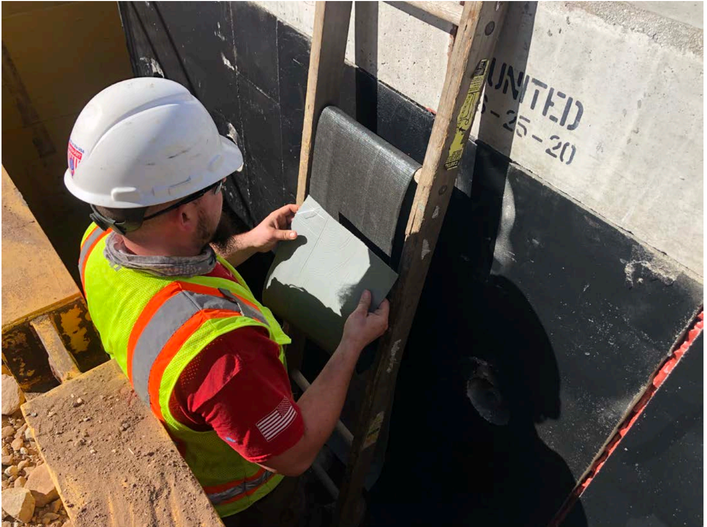
Picture 4: United Concrete applying Boa tape to the side joints of the altitude valve vault walls. East of the Shared Access Driveway, Middletown. View to the southwest.
