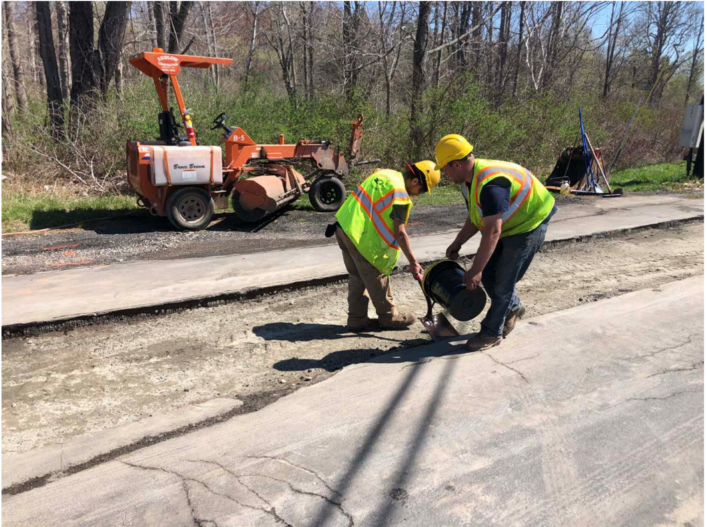
Picture 8: Ludlow placing tack coating on the cut edges of pavement as part of permanent paving activities on Haddam Quarter Road, Durham. View to the northeast.
