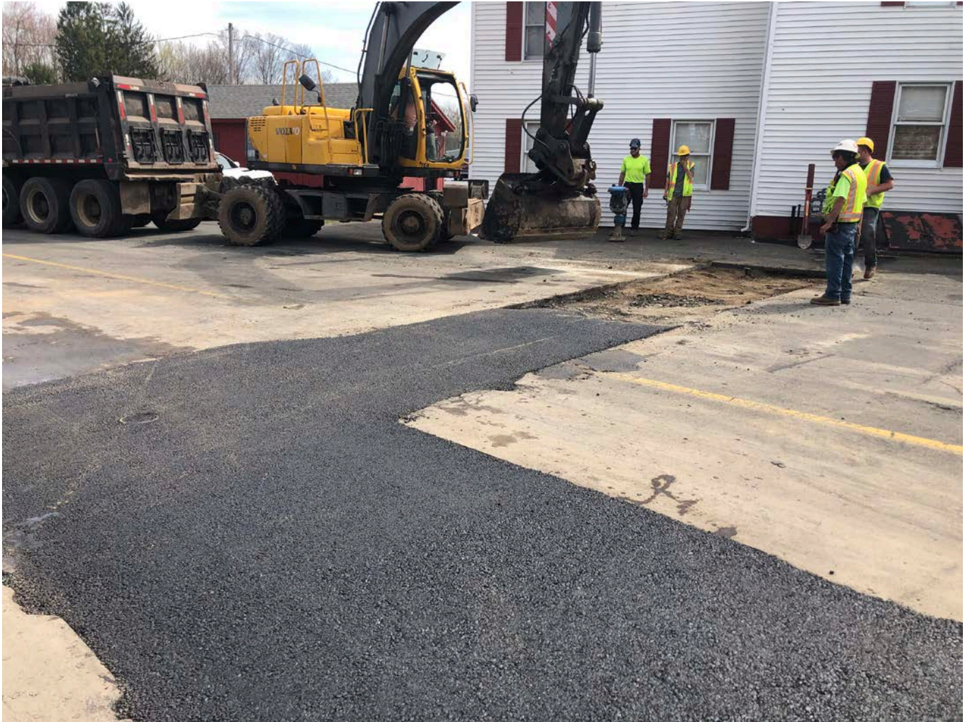
Picture 13: Ludlow placing asphalt on the curb stop trench overcut on Haddam Quarter Road in Durham as part of permanent paving activities. Rooster Liquors visible in the rear. View to the southeast.
