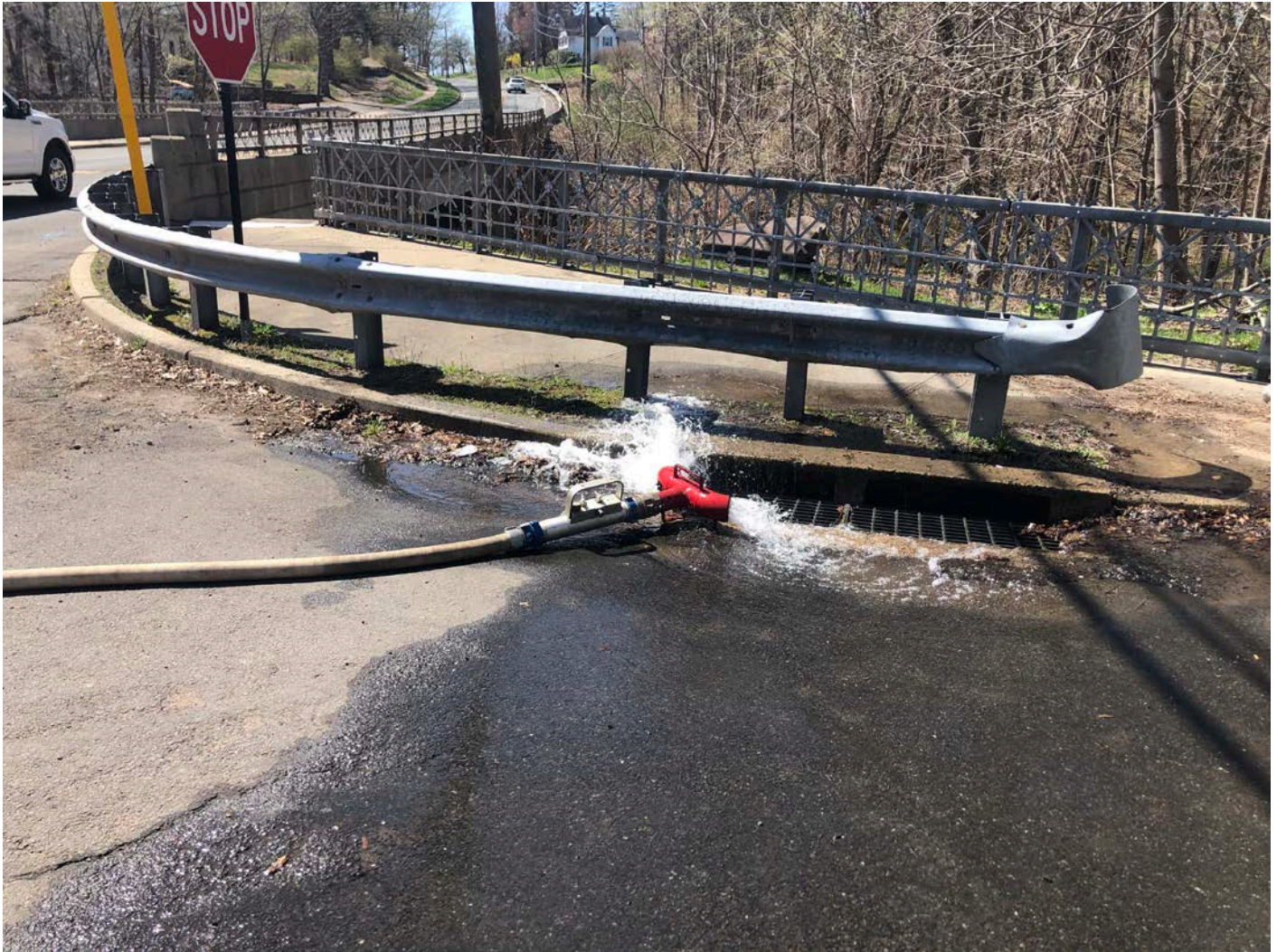
Picture 6: Ludlow and JMS discharging water that they are flushing from the 16" DIP waterline from 327 Main Street to the intersection of Main Street and Old Cemetery Road, Durham. View to the south.
