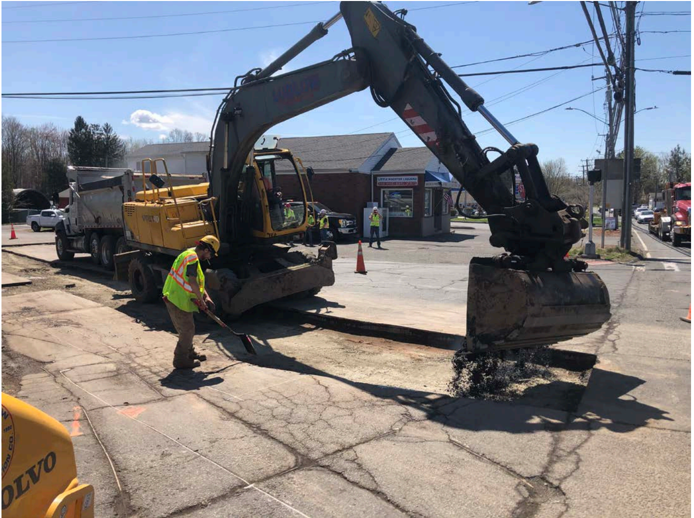
Picture 9: Ludlow placing the first lift of asphalt as part of permanent paving activities on Haddam Quarter Road, Durham. View to the southeast.
