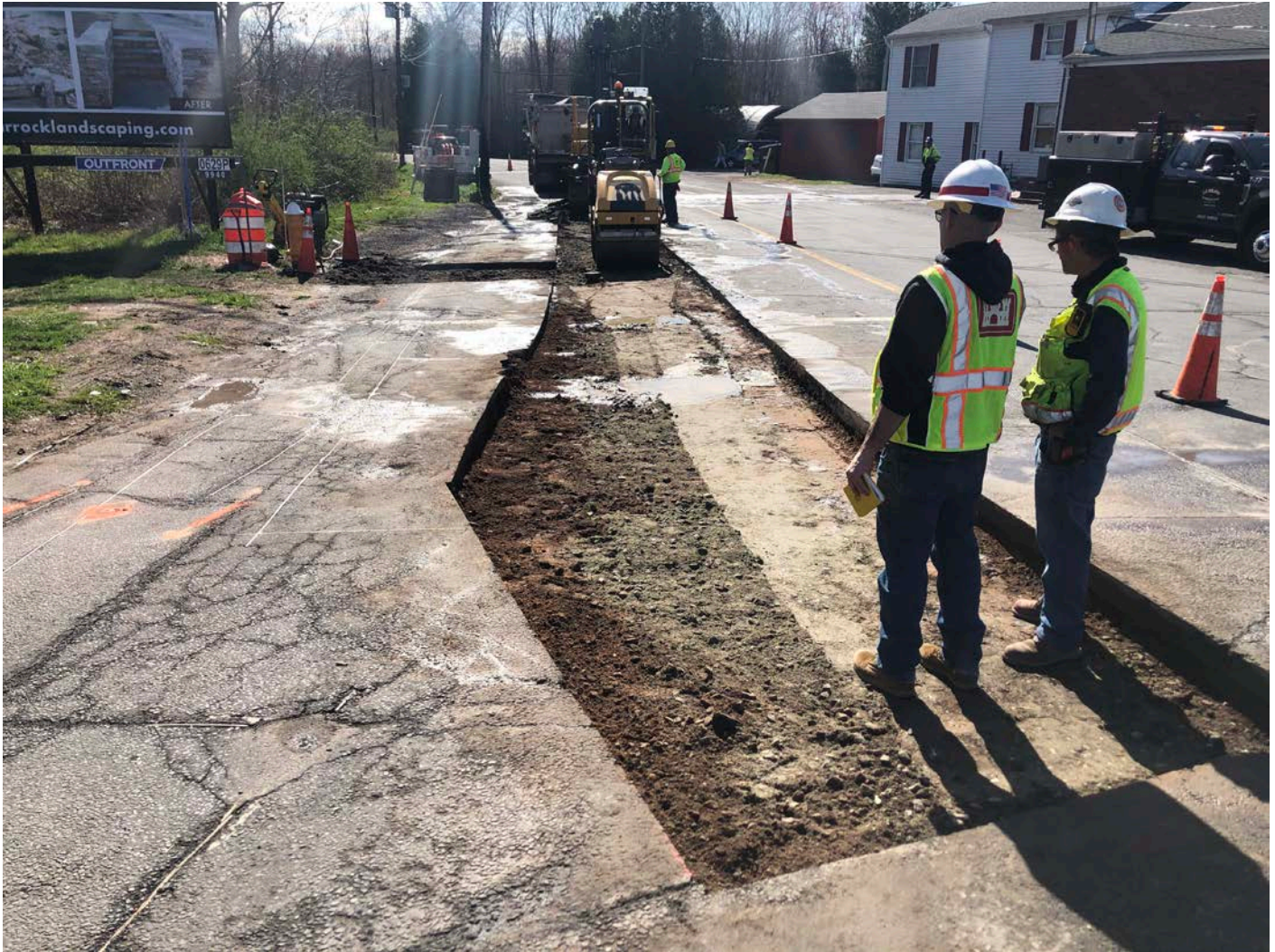
Picture 5: Asphalt that Ludlow stripped away on Haddam Quarter Road, Durham, as part of permanent paving activities. View to the east.
