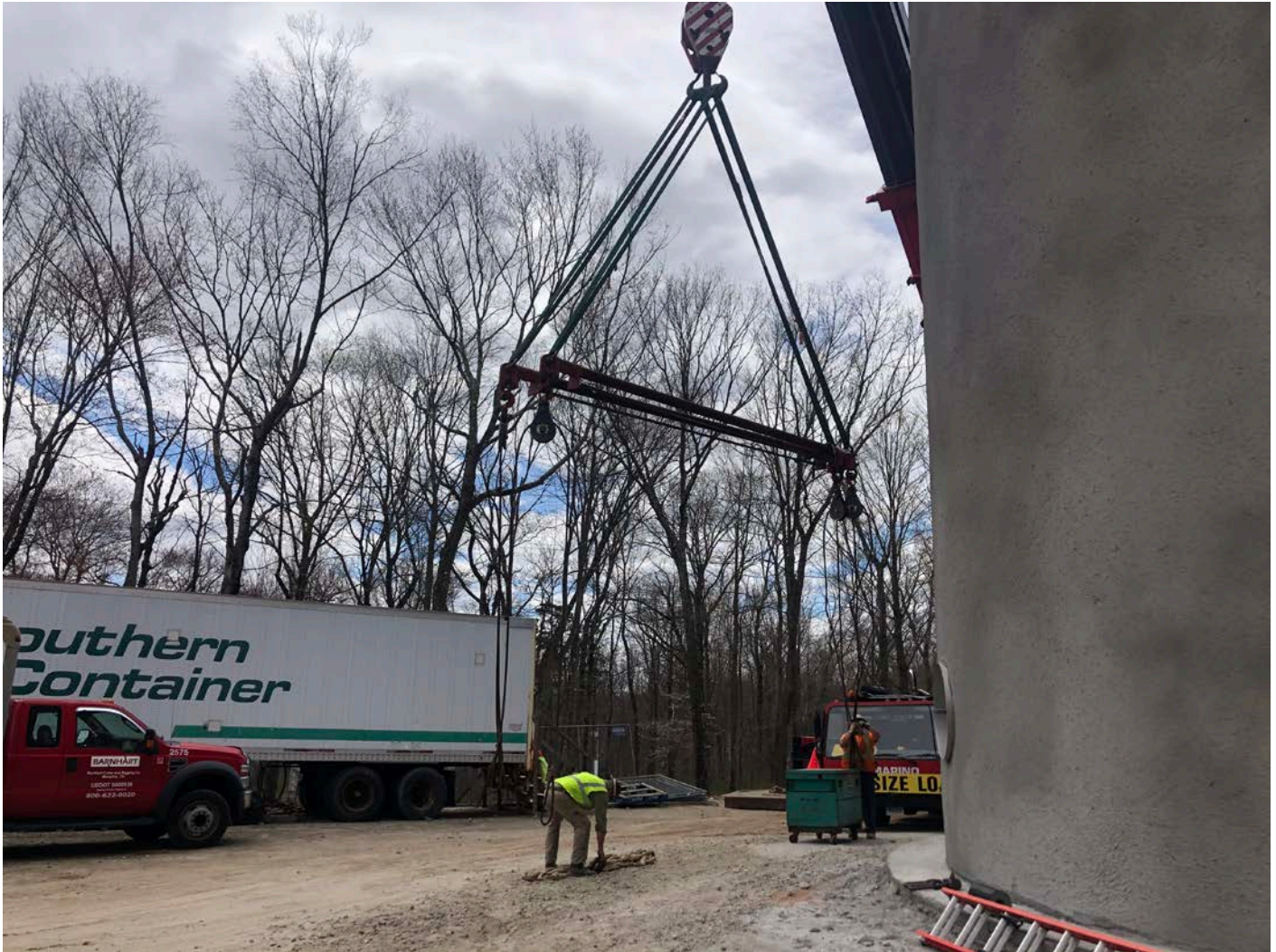
Picture 6: Barnhart adding lift hardware to the lift sling that will be used to hoist pieces of the altitude valve vault into place during the vault installation to the east of the Shared Access Driveway. View to the southwest.
