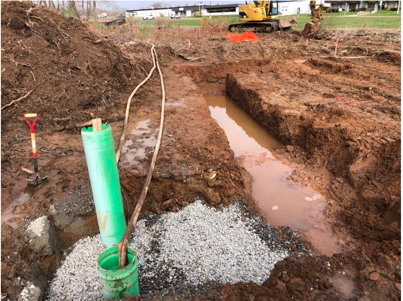
Picture 1: Two dewatering wells that Ludlow placed at the southeast corner of the booster station footprint.
