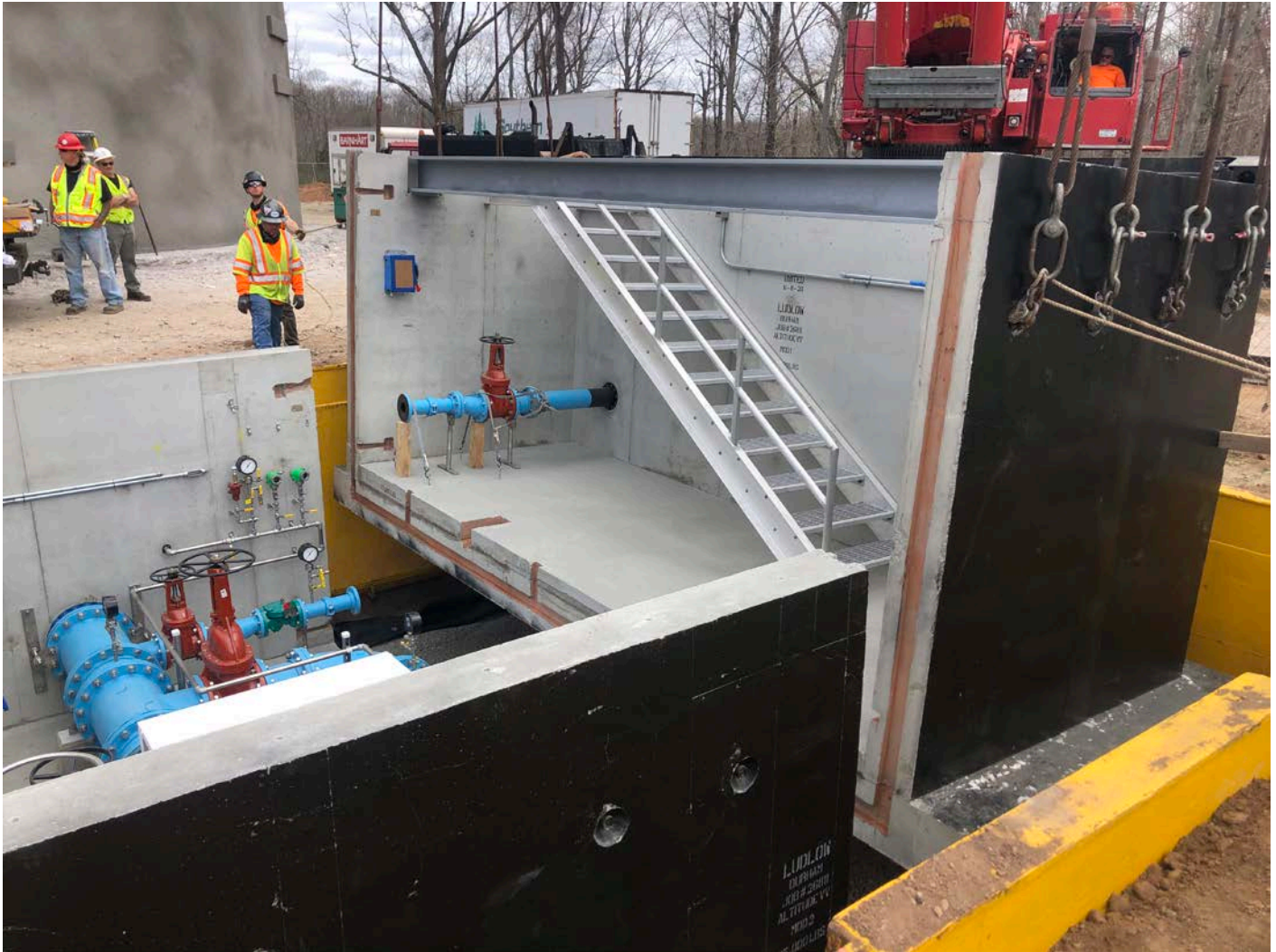
Picture 9: Barnhart lowering the second of the two halves of the altitude vault into place; east of the Shared Access Driveway, Middletown. View to the southeast.
