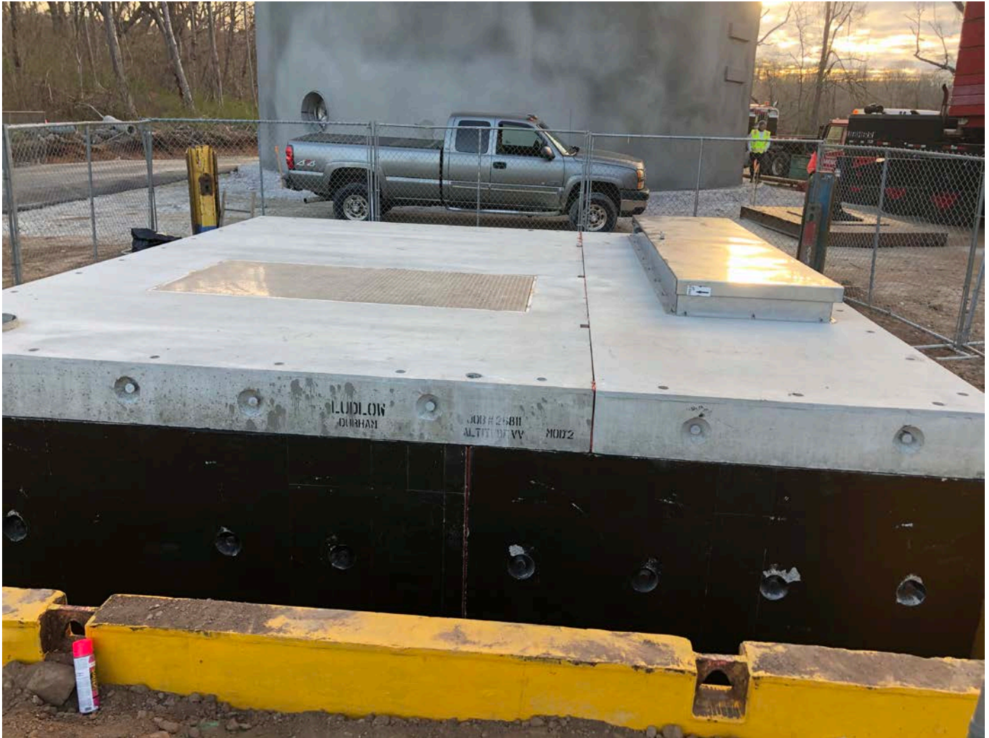
Picture 10: View of the altitude valve vault with both sections of the roof installed; east of the Shared Access Driveway, Middletown. View to the east.
