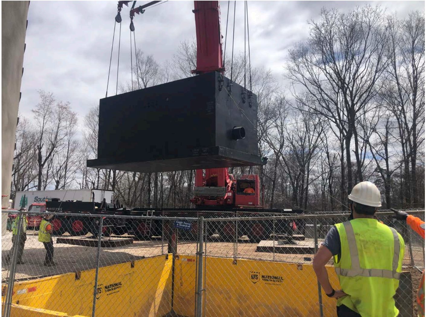
Picture 7: Barnhart lifting the first of the two halves of the altitude valve vault as they prepare to lower it into the trench box. East of the Shared Access Driveway, Middletown. View to the southeast.
