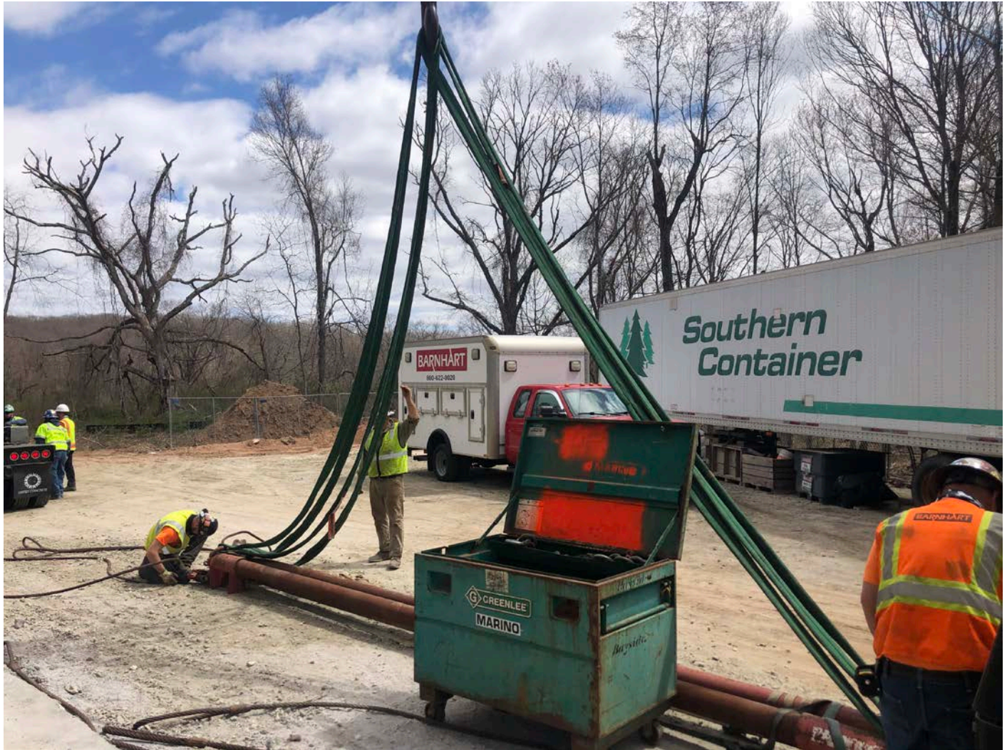
Picture 4: Barnhart preparing the sling that will be used to hoist pieces of the altitude valve vault into place during the vault installation to the east of the Shared Access Driveway. View to the southeast.
