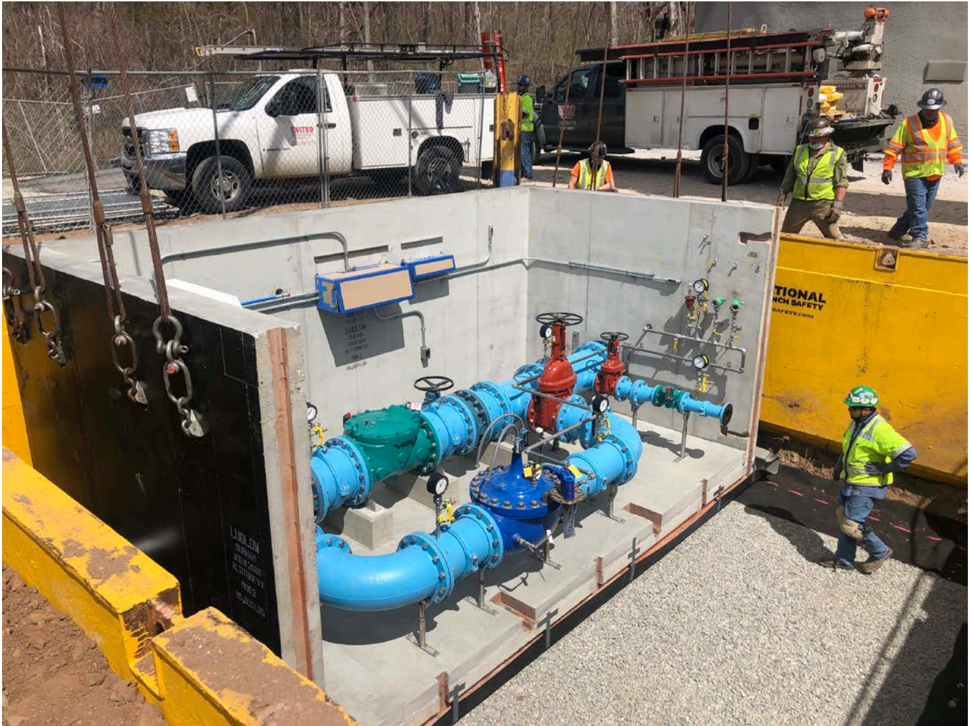
Picture 8: The project field team fine-tuning the placement of the first of the two halves of the altitude valve vault east of the Shared Access Driveway, Middletown. View to the southeast.
