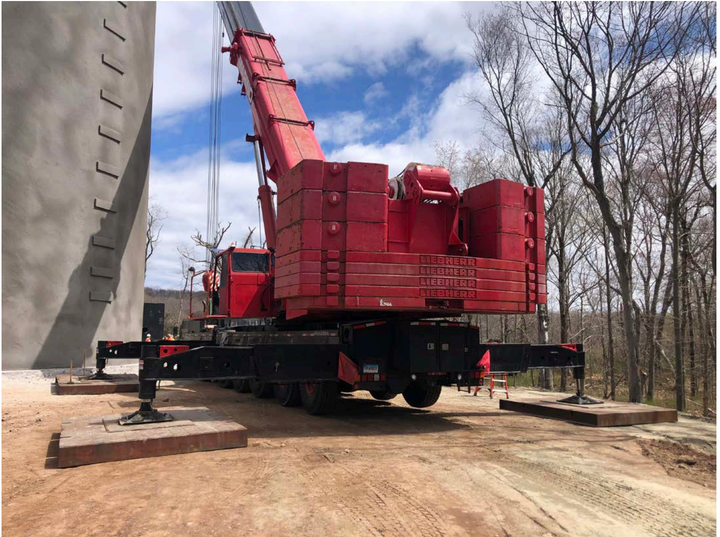
Picture 3: Barnhart/Marino crane staged on the southwest side of the water tank located east of the Shared Access Driveway as they prepare to lift the pieces of the altitude valve vault as they prepare to install them. View to the east.
