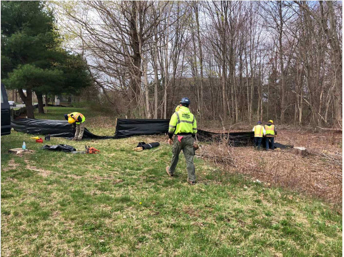
Picture 3: Ludlow placing and fixing silt fence south, and proximal to, the booster station at Station 750+63. View to the south.
