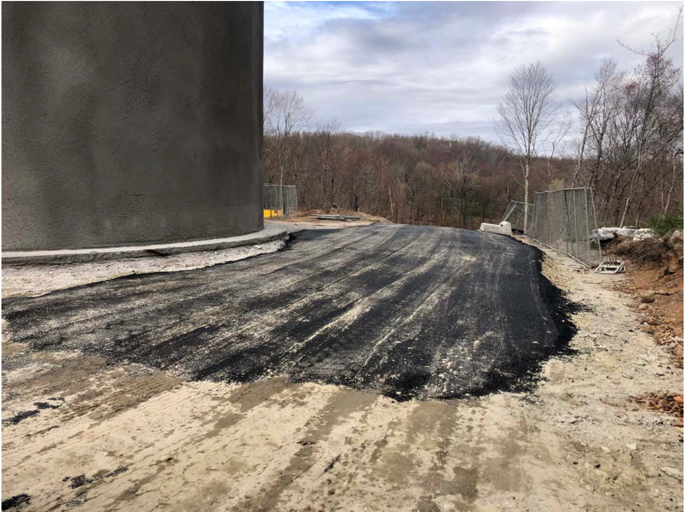
Picture 2: Ludlow has placed asphalt at the northwest corner of the water tank work zone located east of the shared access driveway in preparation for the heavy vehicles that will be at the site tomorrow for the installation of the altitude vault. View to the west.
