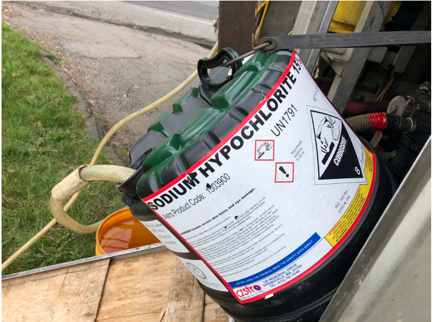
Picture 5: The sodium hypochlorite that JMS Connections in the process of introducing into the 16" water main at 327 Main Street, Durham.
