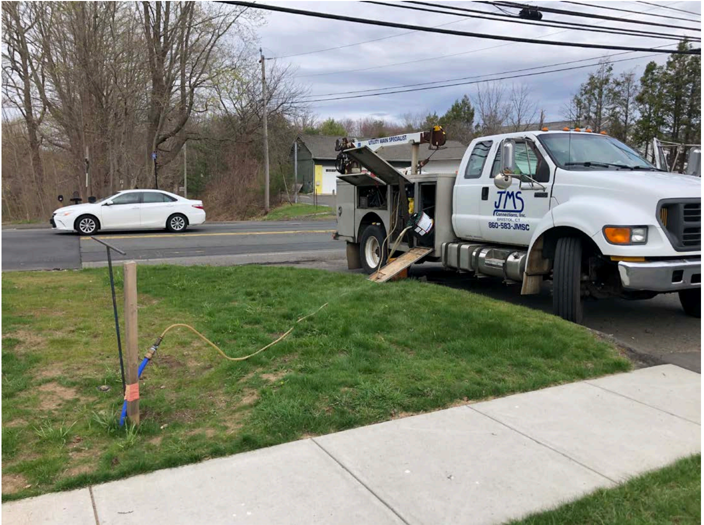
Picture 4: JMS Connections in the process of introducing sodium hypochlorite into the 16" water main at 327 Main Street, Durham. View to the west.
