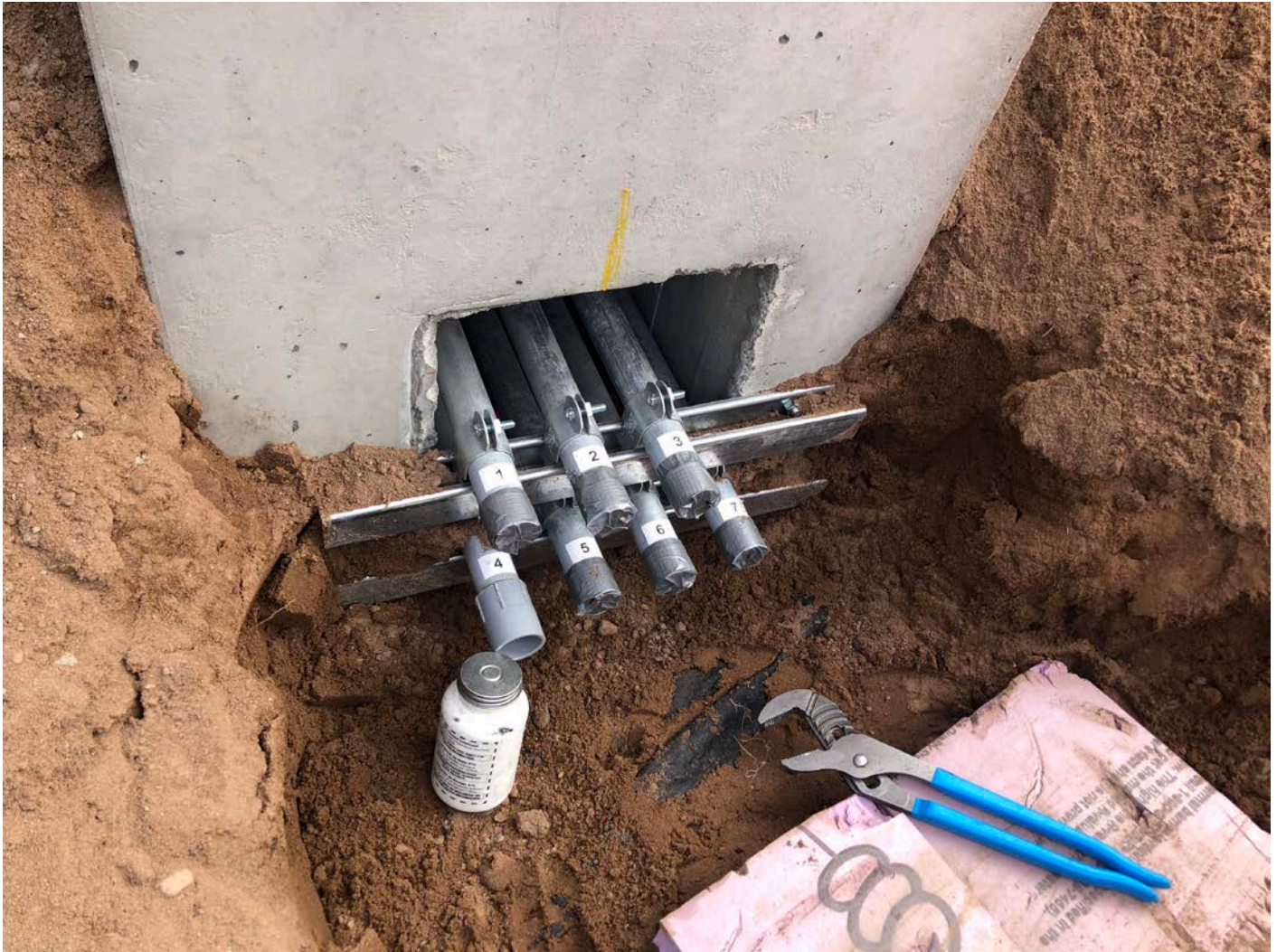
Picture 4: View of the electrical enclosure at the pressure reducing valve vault at Station ~161+40 as United Concrete is in the process of installing PVC conduits. View to the northeast.
