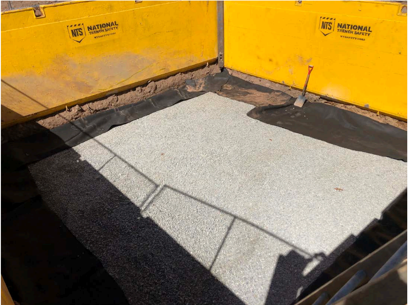
Picture 5: View of the altitude valve vault excavation at the water tank work zone located east of the Shared Access Driveway, Middletown. View to the southwest.
