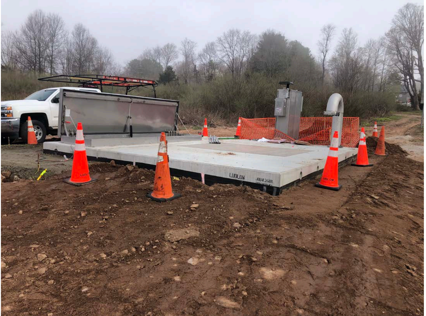
Picture 2: View of the fill that has been placed around the walls of the pressure reducing valve vault at Station ~161+40. View to the northwest.
