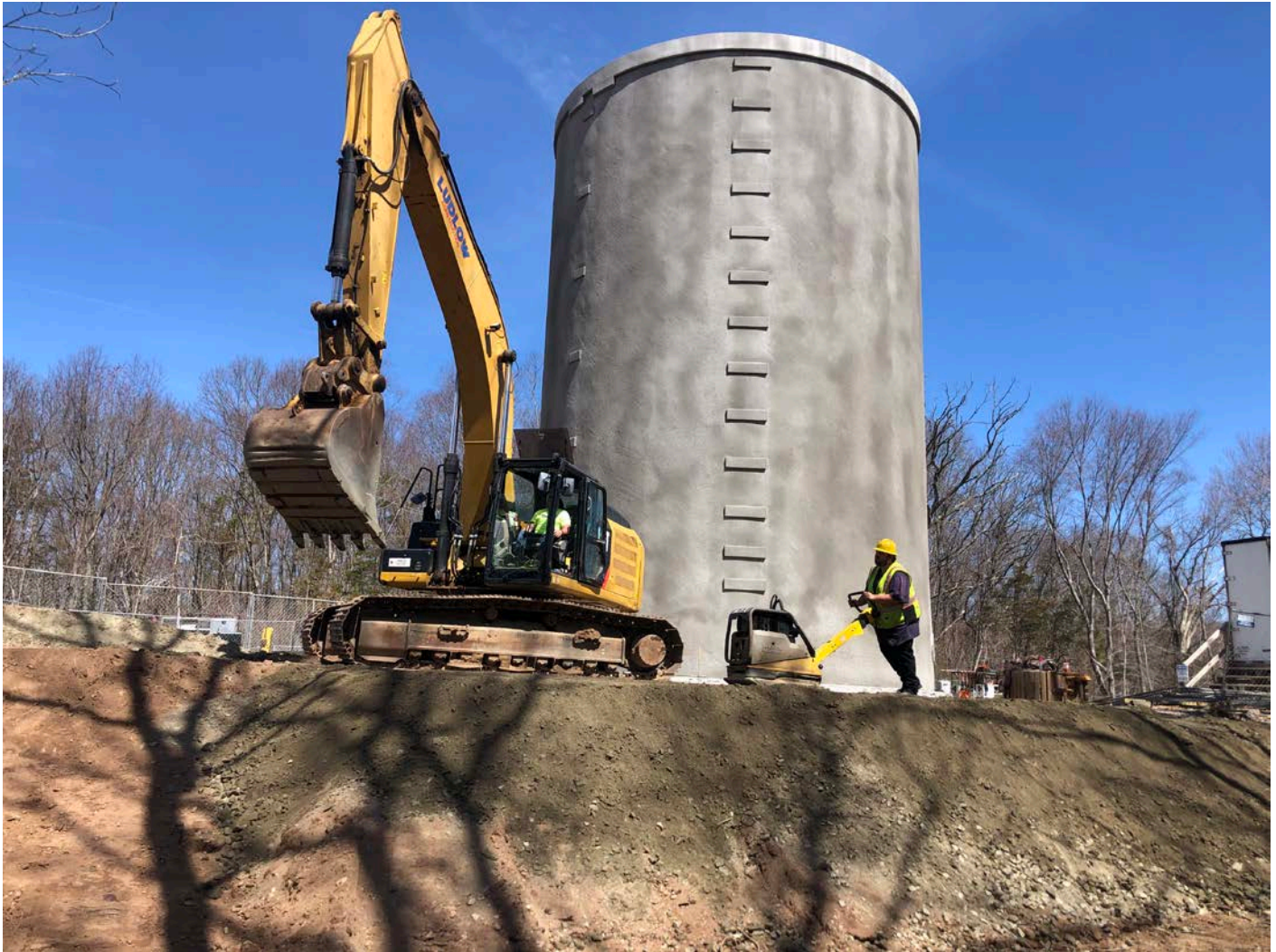
Picture 6: Ludlow placing and compacting fill at the southwest corner of the water tank work zone in order to create a staging pad for a crane outrigger. View to the northeast.
