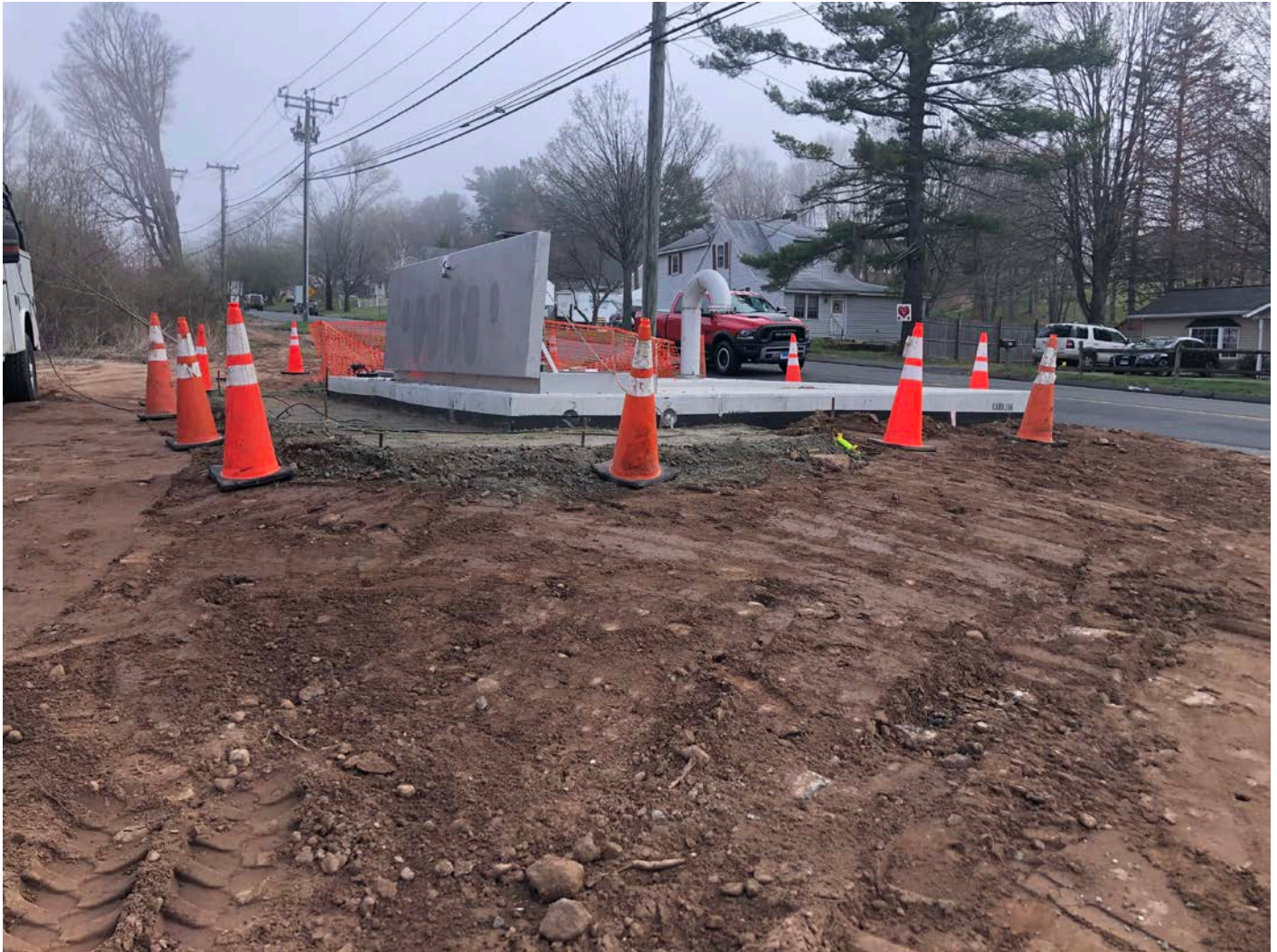
Picture 1: View of the fill that has been placed around the walls of the pressure reducing valve vault at Station ~161+40. View to the northeast.
