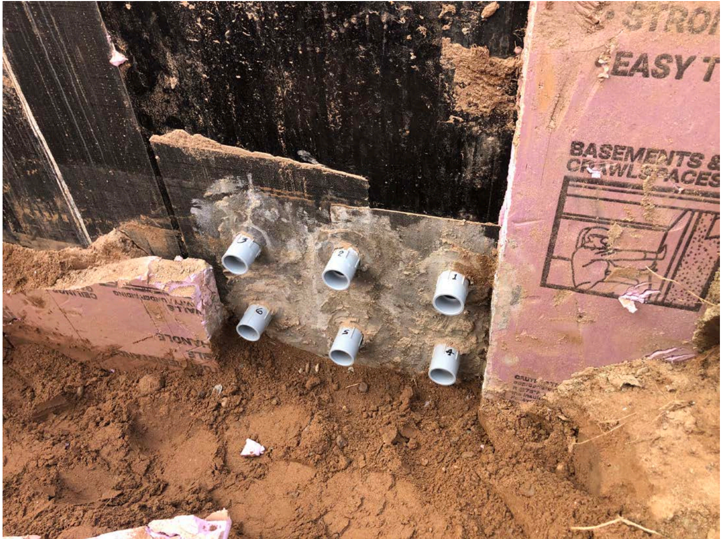
Picture 3: PVC fittings that United Concrete has installed on the north side of the pressure reducing valve vault at Station ~161+40. View to the south.
