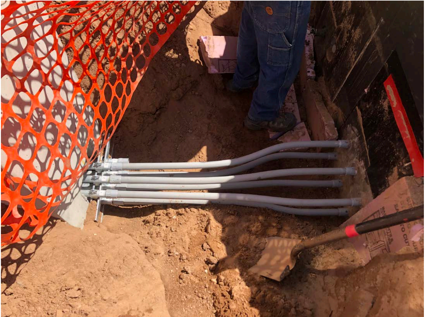
Picture 7: PVC conduit that United Concrete installed between the electrical enclosure and the pressure reducing valve vault at Station ~161+40.
