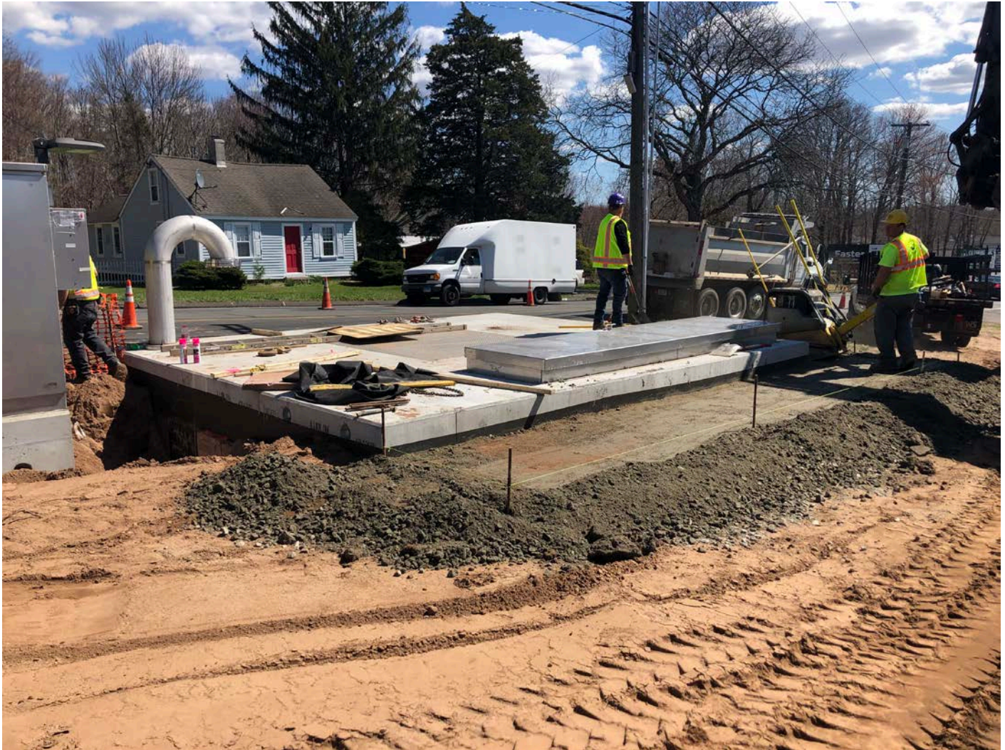
Picture 8: View of the pressure reducing valve vault at Station ~161+40 as Ludlow places and compacts fill around the perimeter of the vault. View to the southeast.
