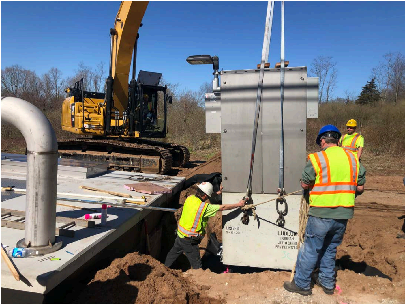
Picture 3: Ludlow and United Concrete positioning the electrical enclosure for the pressure reducing valve vault at Station ~161+40. View to the west.
