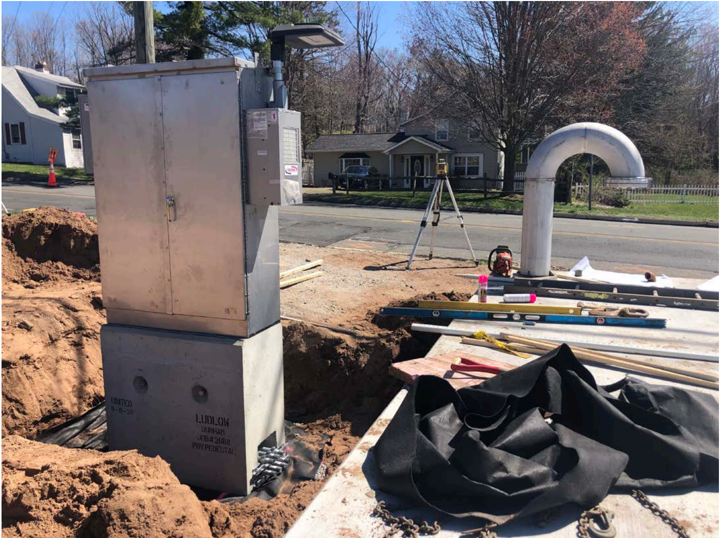
Picture 4: View of the electrical enclosure at Station ~161+40 as Ludlow is in the process of installing it. View to the east.
