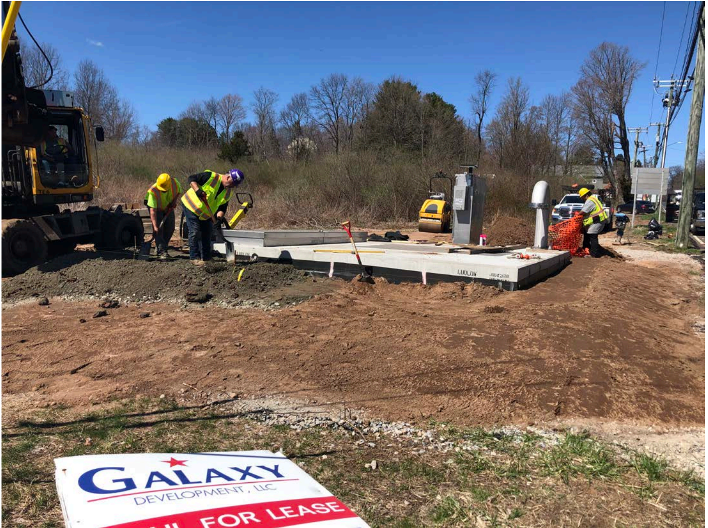
Picture 7: View of the pressure reducing valve vault at Station ~161+40 as Ludlow places and compacts fill around the perimeter of the vault. View to the north.
