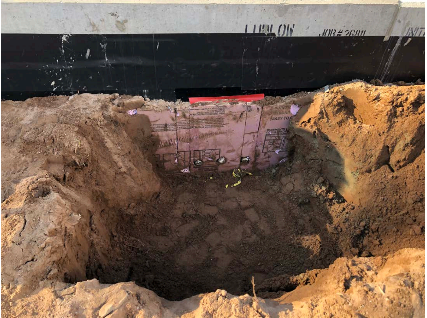
Picture 1: View of the north side of the pressure reducing valve vault that has been daylighted so that Ludlow can install the electrical enclosure at Station ~161+40. View to the south.
