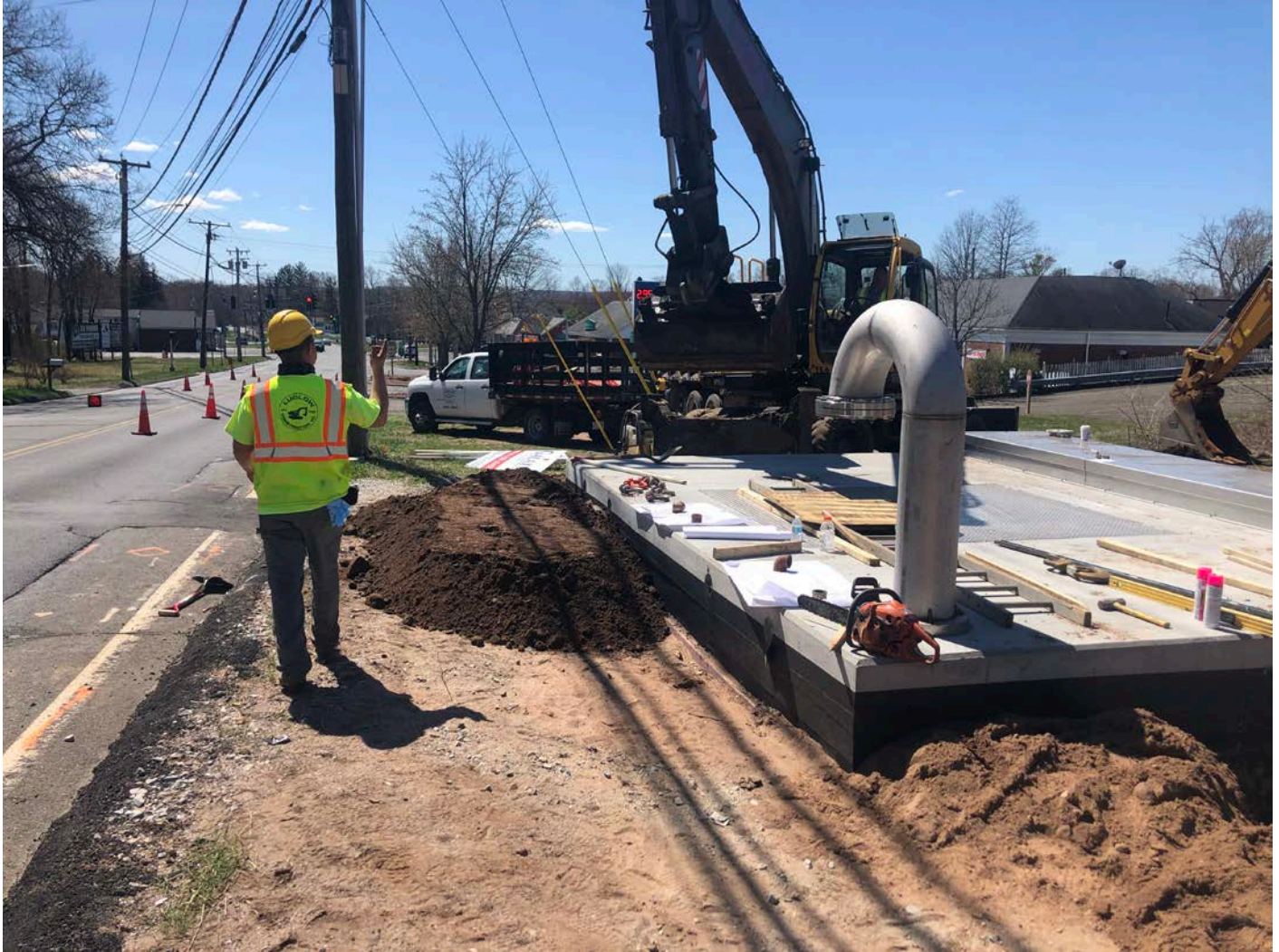
Picture 6: Ludlow placing fill around the perimeter of the pressure reducing valve vault at Station ~161+40 in Durham. View to the south.
