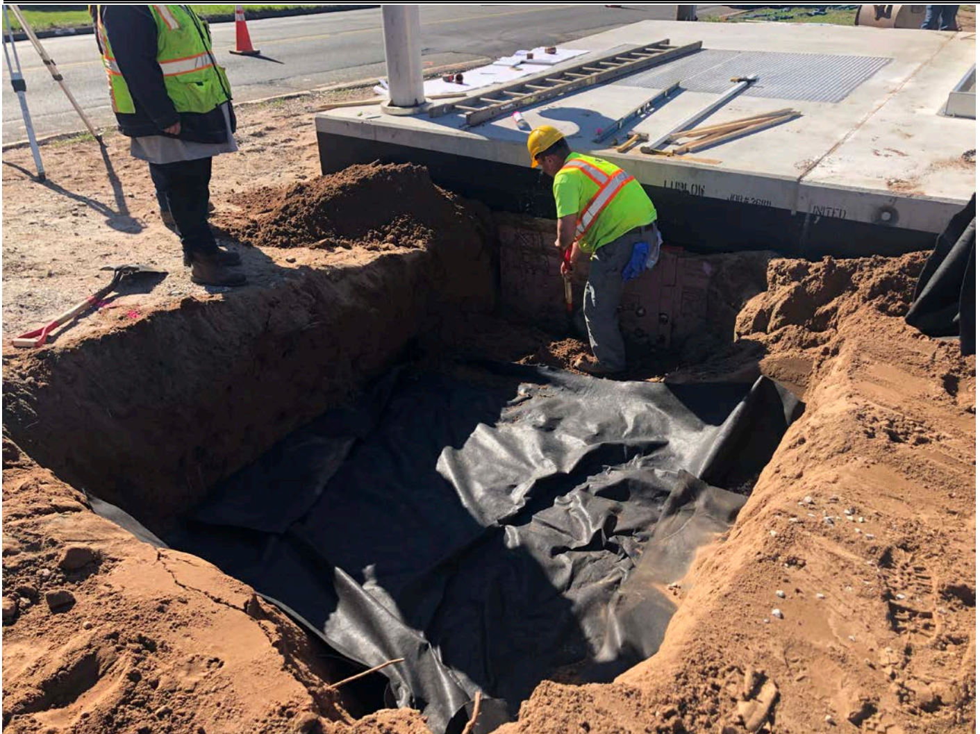
Picture 2: View of the north side of the pressure reducing vault that has been daylighted so that Ludlow can install the electrical enclosure for the pressure reducing valve vault at Station ~161+40, with geofabric placed over \frac{3}{4} " stone at the bottom of the excavation. View to the southeast.
