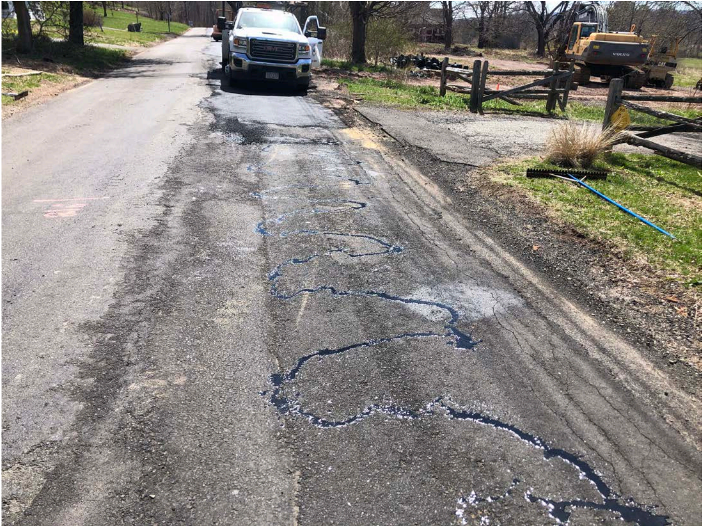
Picture 6: Tack coat that Ludlow applied to the west side of Maple Avenue as they shim coat sections of Maple Avenue between Old Cemetery Road and Route 68. View to the south.
