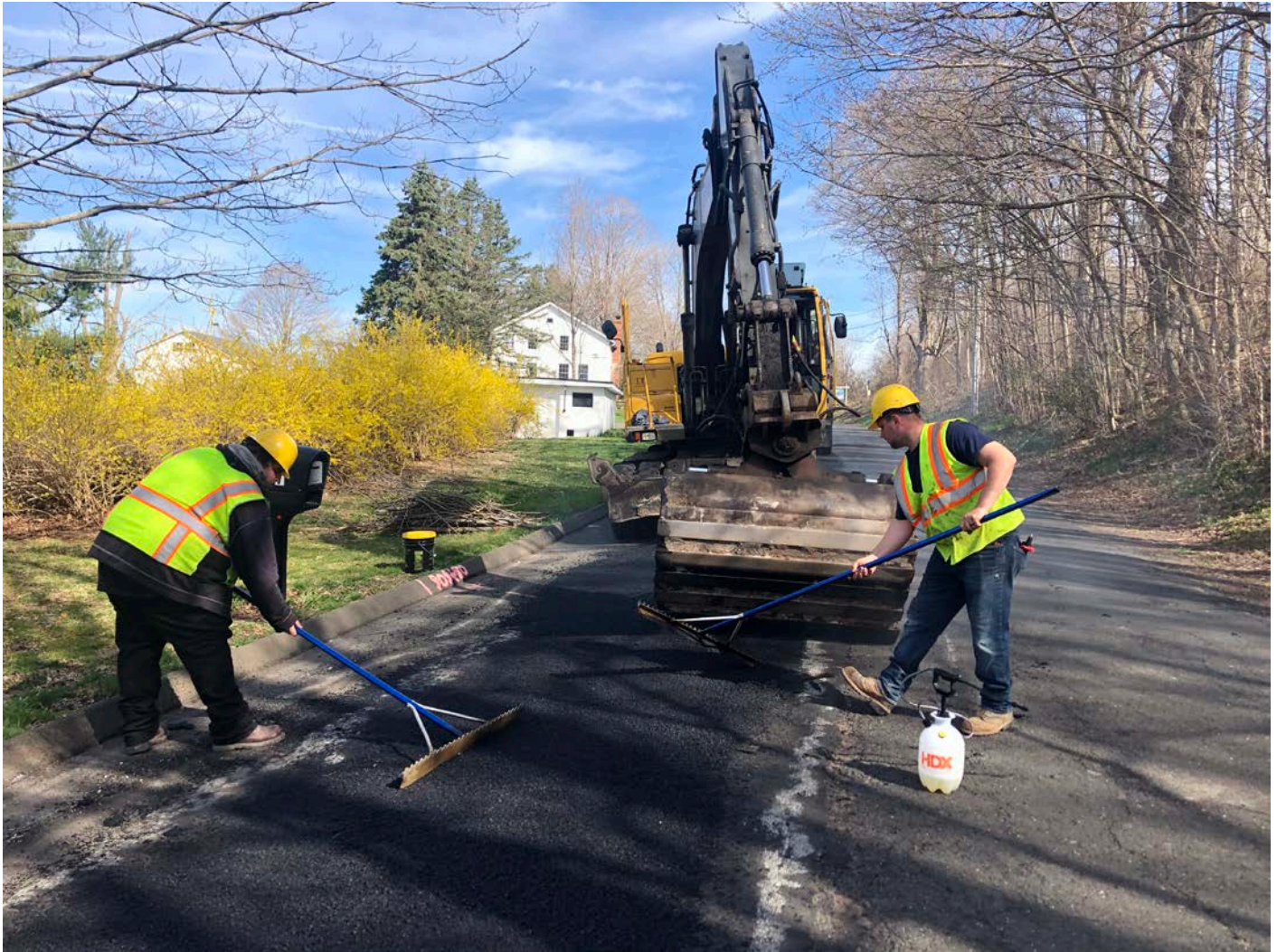
Picture 5: Ludlow grading freshly-placed asphalt as they shim coat on the west side of Maple Avenue between Old Cemetery Road and Route 68. View to the north.
