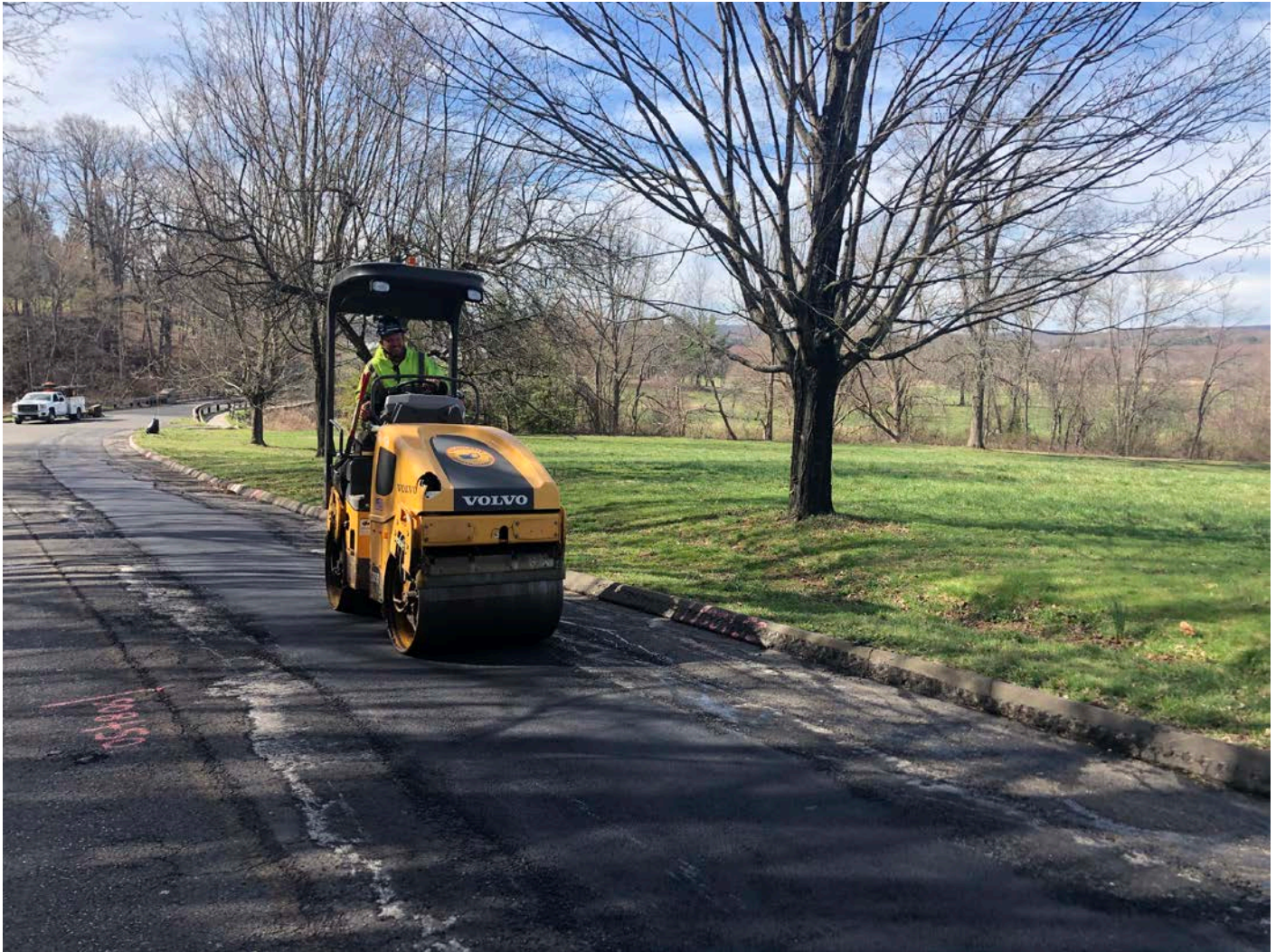
Picture 4: Ludlow rolling freshly-placed asphalt as they shim coat sections of Maple Avenue between Old Cemetery Road and Route 68. View to the south.
