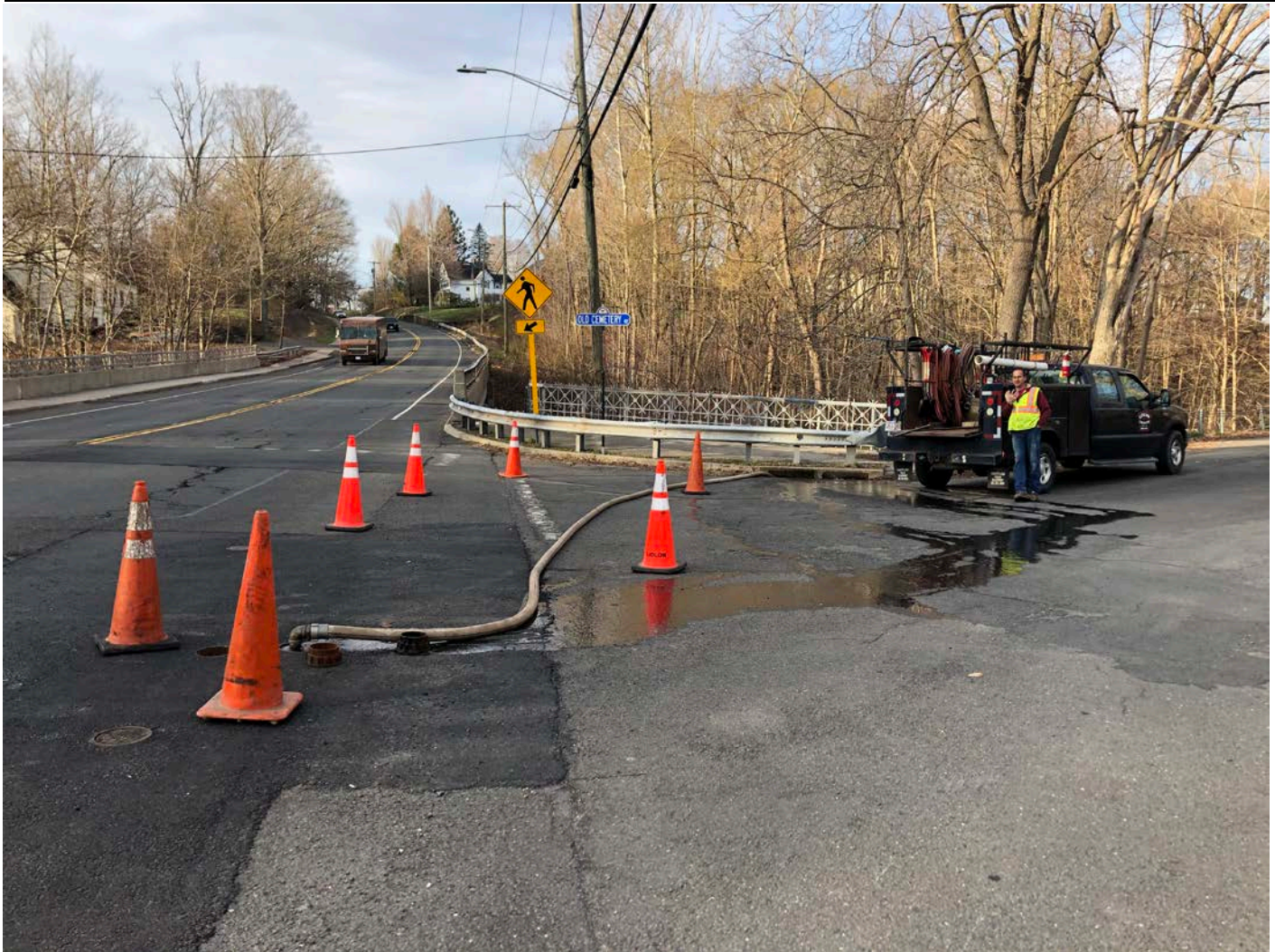
Picture 1: Ludlow directing water purged from the 16" water line on Main Street from Talcott Lane to Cemetery Road, Durham. View to the south.
