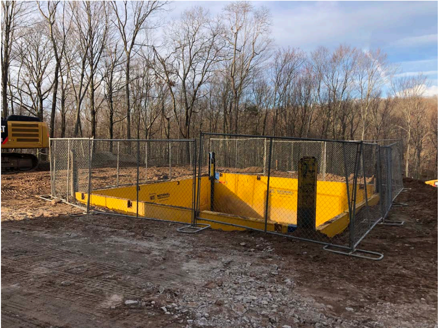
Picture 2: Trench box for the altitude valve vault with security fencing placed around it for security. East of the Shared Access Driveway, Middletown. View to the southwest.
