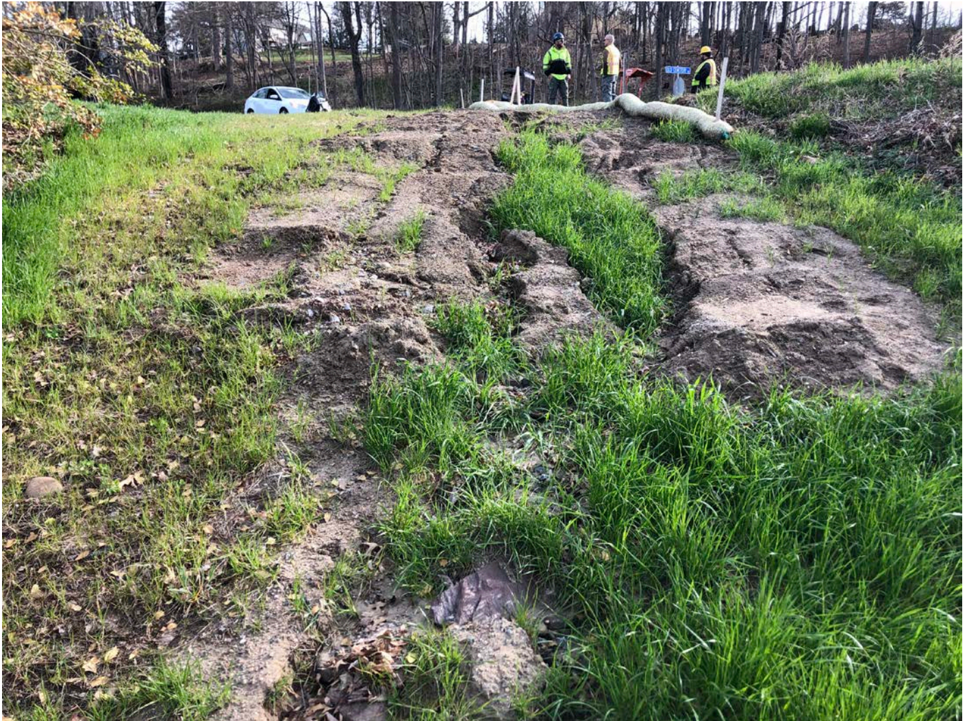
Picture 3: Several deep rills were observed on the slope north of, and adjacent to, the bridge that crosses Allyn Brook on the west side of Maple Avenue. View to the northeast.
