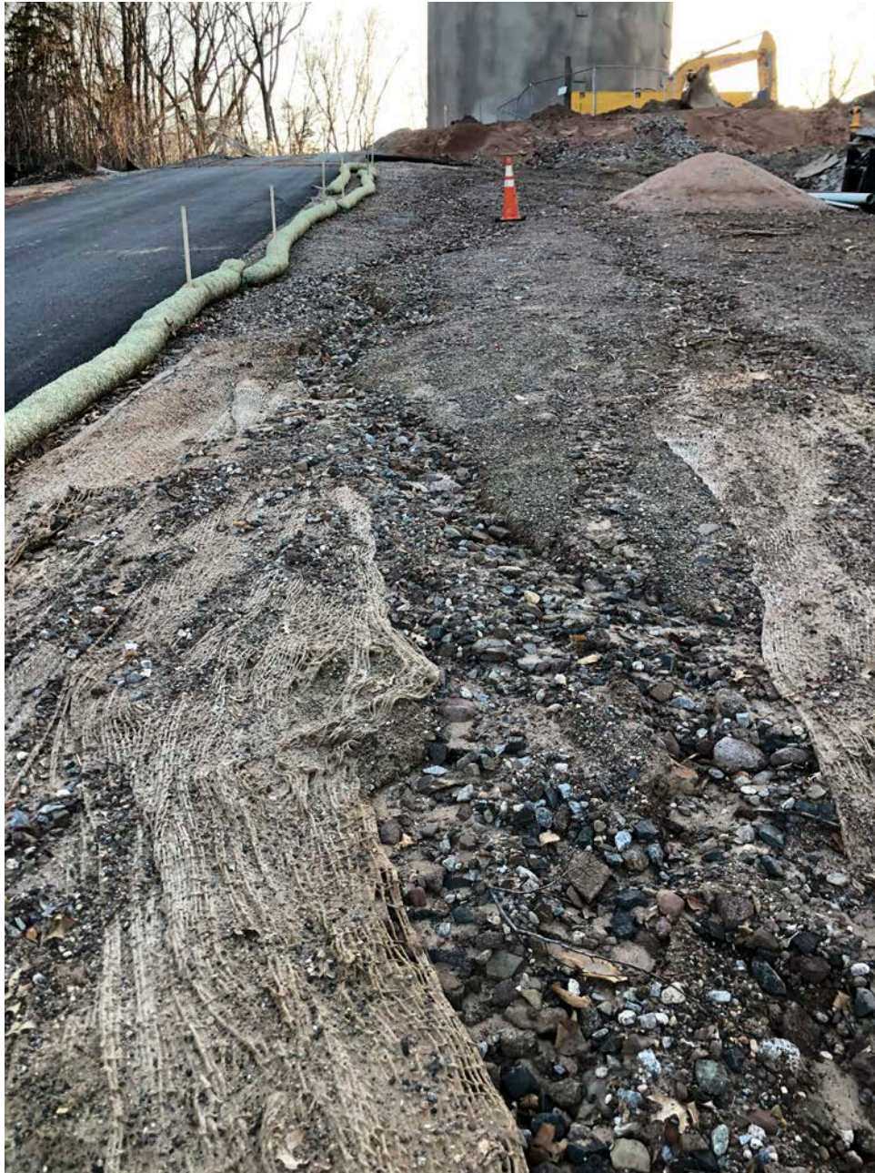
Picture 2: Minor erosion observed south of the straw wattles placed by Ludlow on the southern/upslope side of the Shared Access Driveway. View to the east.
