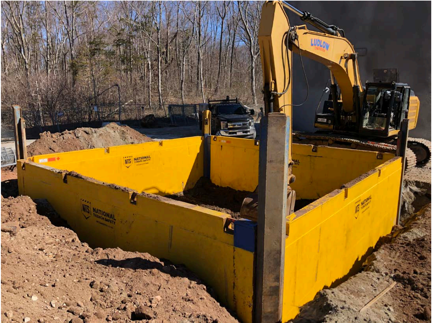
Picture 5: Trench box that Ludlow installed around the Altitude Valve Vault excavation, east of the Shared Access Driveway, Middletown. View to the south.
