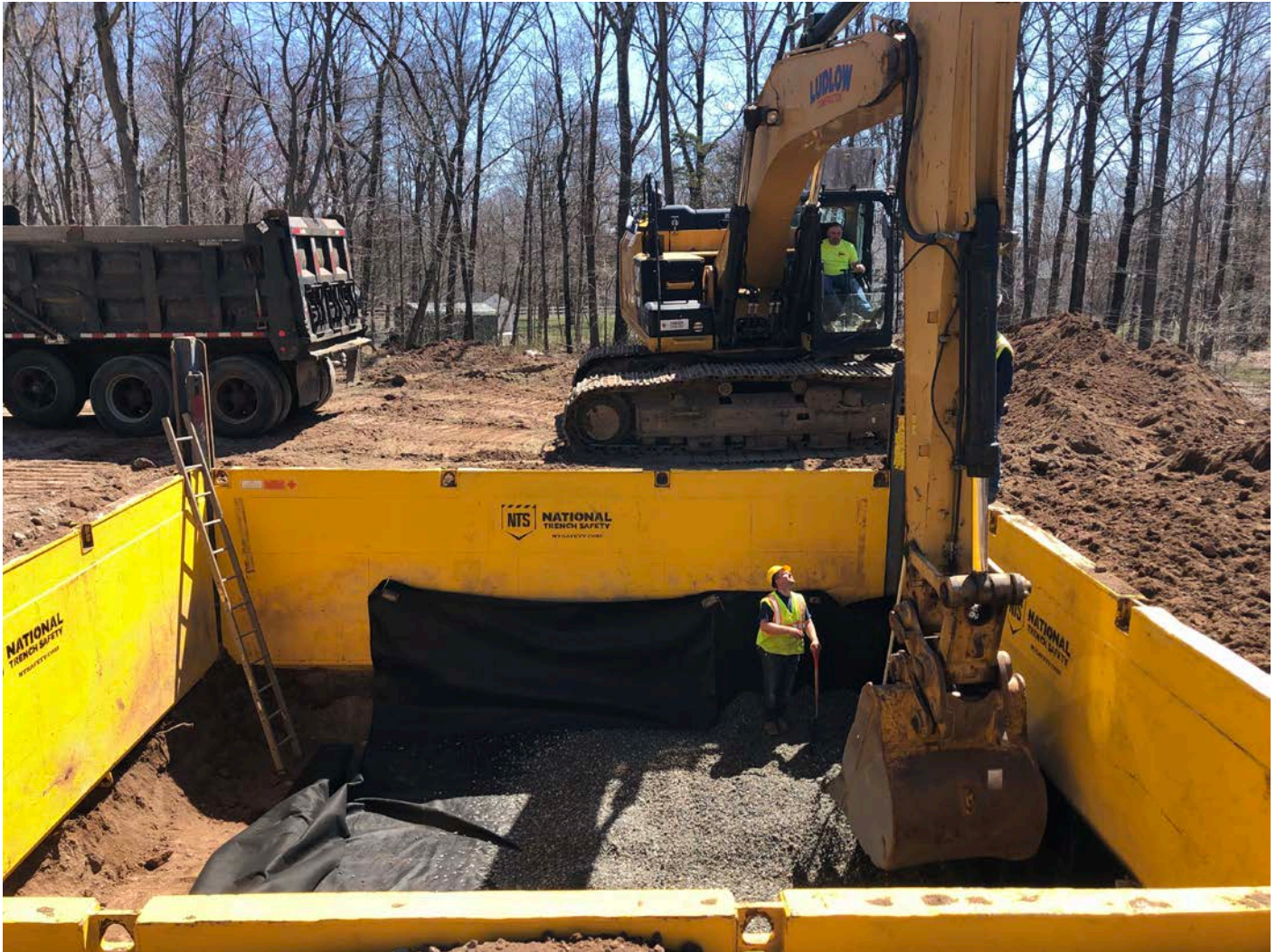
Picture 7: Ludlow placing ¾" stone on top of black geofabric at the bottom of the altitude valve vault excavation. View to the south.
