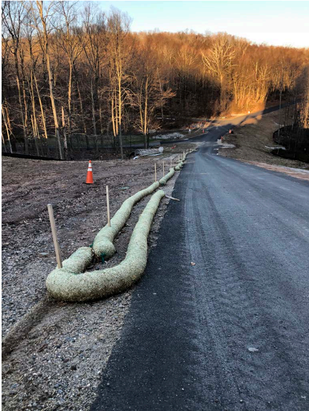
Picture 1: Straw wattles that Ludlow placed for erosion control on the southern/upslope side of the Shared Access Driveway. View to the west.
