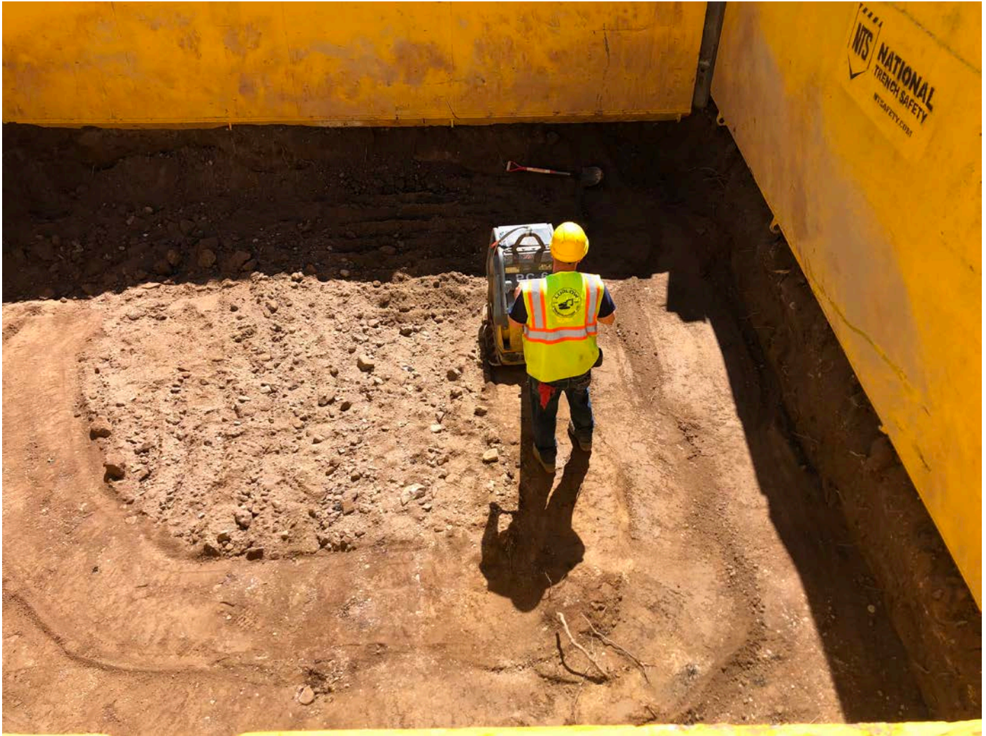
Picture 6: Ludlow compacting native earth at the bottom of the altitude valve vault excavation using a plate compactor. View to the south.
