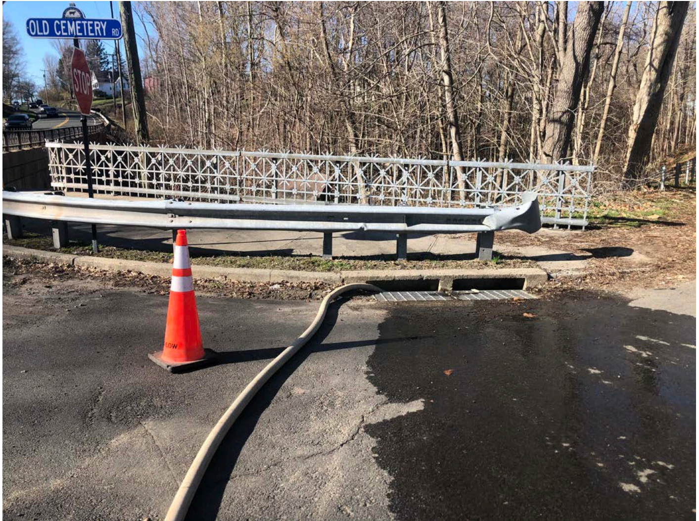
Picture 4: Ludlow directing water purged from the 16" water line on Main Street from Talcott Lane to Cemetery Road, Durham. View to the south.
