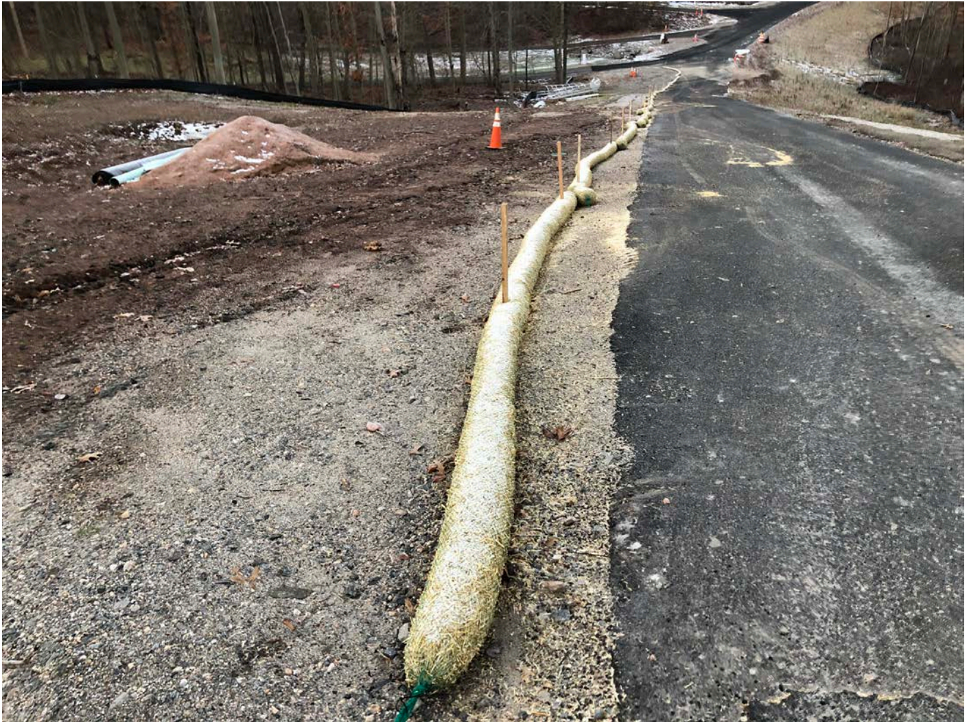
Picture 1: Straw wattles that Ludlow placed for erosion control on the southern/upslope side of the shared access driveway. View to the west.
