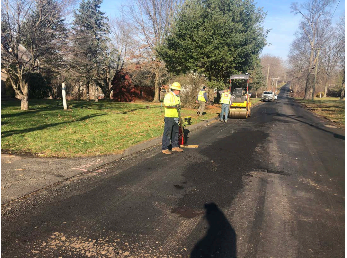
Picture 3: Ludlow shim coating on the southbound lane of Maple Avenue in the vicinity of Station 927+50. View to the north.
