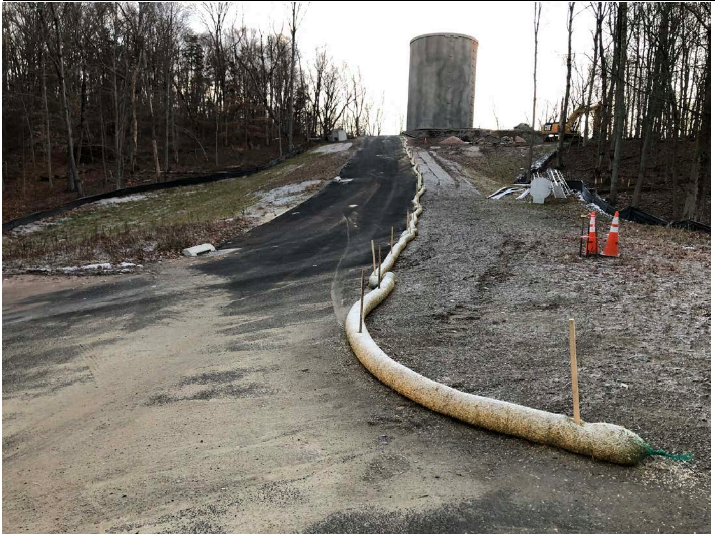
Picture 2: Straw wattles that Ludlow placed for erosion control on the southern/upslope side of the shared access driveway. View to the east.
