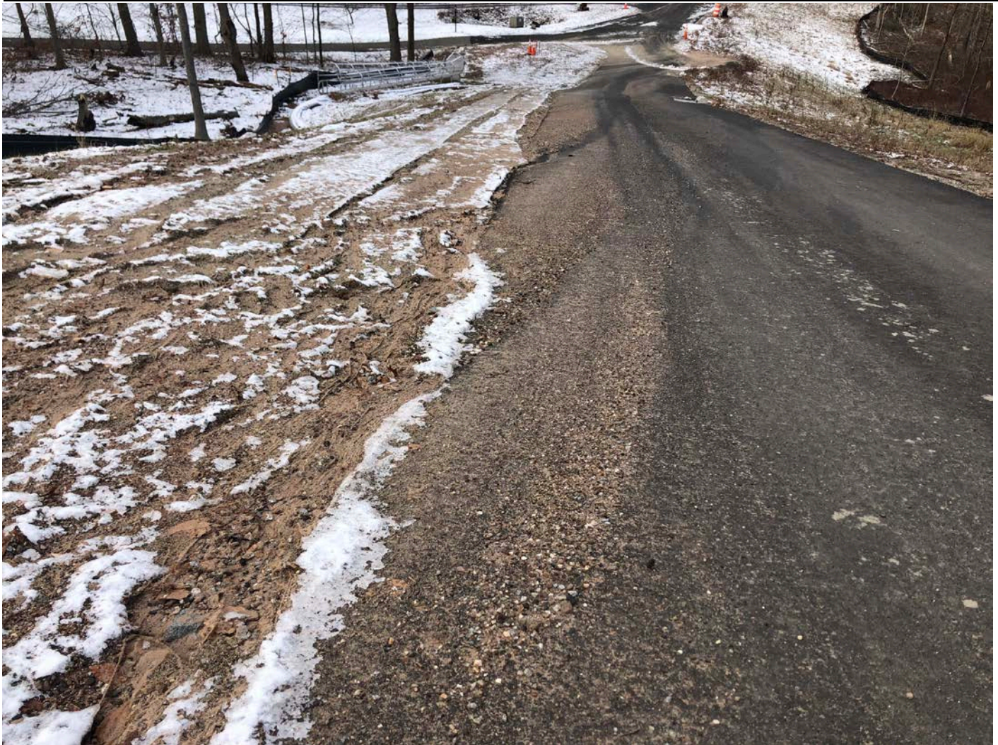
Picture 5: Gravel that has been washed onto the eastern end of the Shared Access Driveway from recent rain events. View to the west.
