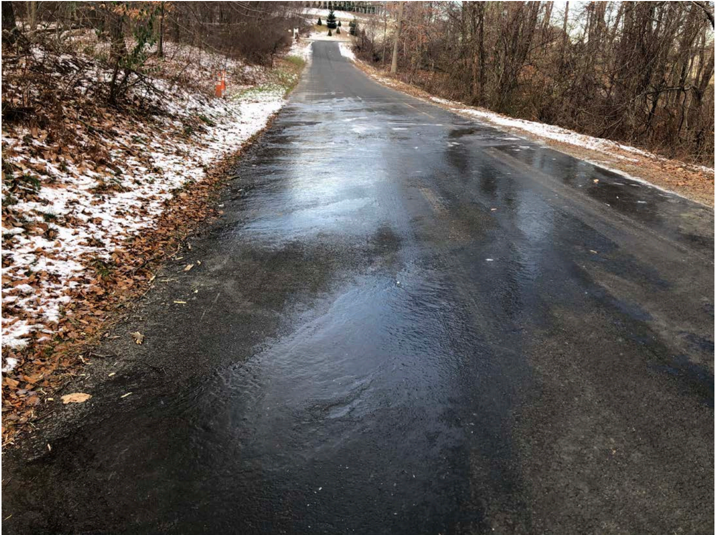
Picture 3: Area on the Shared Access Driveway at ~Station 19+50 where water has moved from south to north across the road and froze in place (just east of the plunge bowl located on the south side of the road at ~Station 19+80; visible just past the traffic cone on the rear left of the photograph). View to the northwest.
