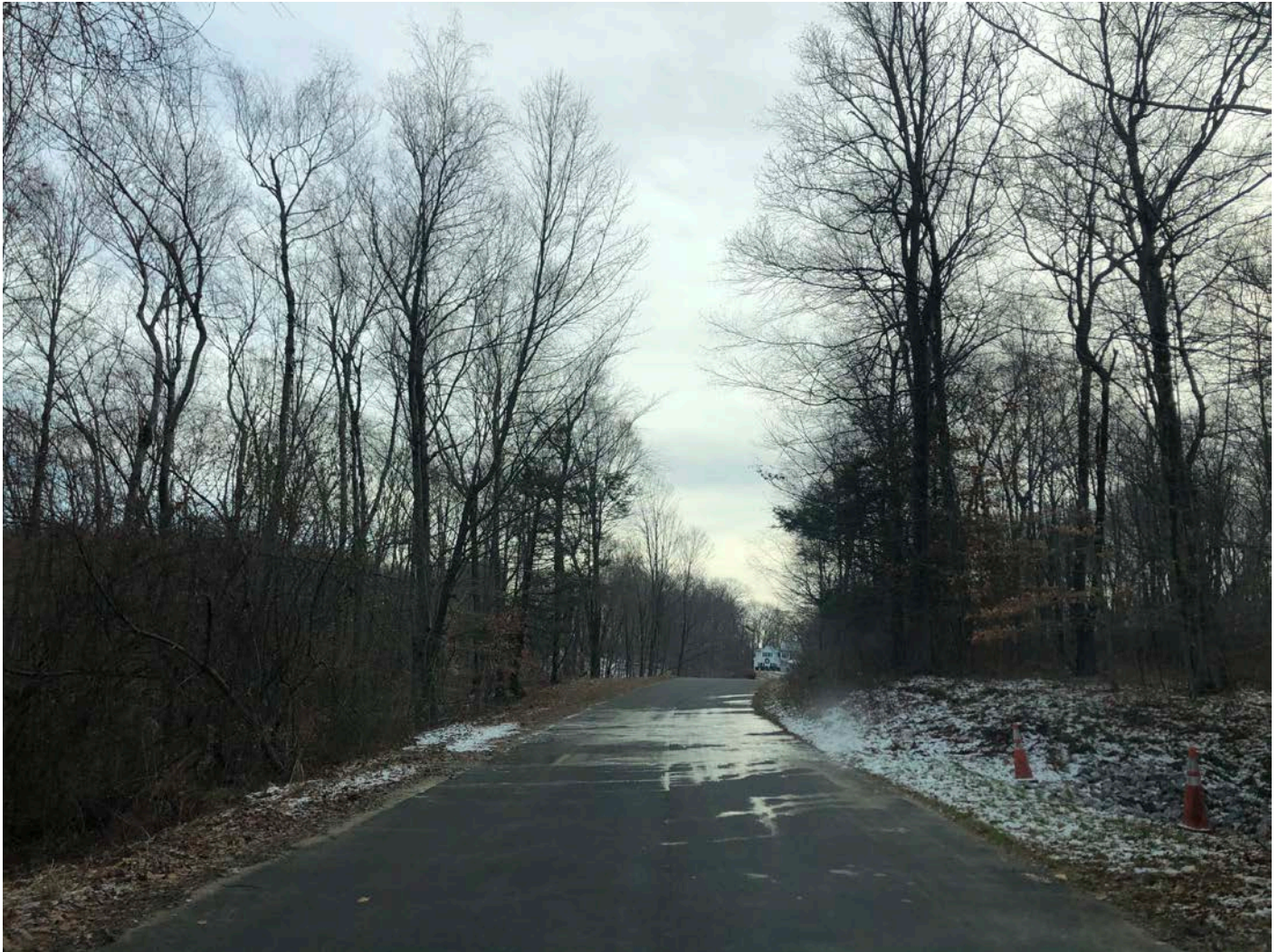
Picture 2: Area on the Shared Access Driveway at ~Station 19+50 where water has moved from south to north across the road and froze in place (just east of the plunge bowl located on the south side of the road at ~Station 19+80). View to the southeast.
