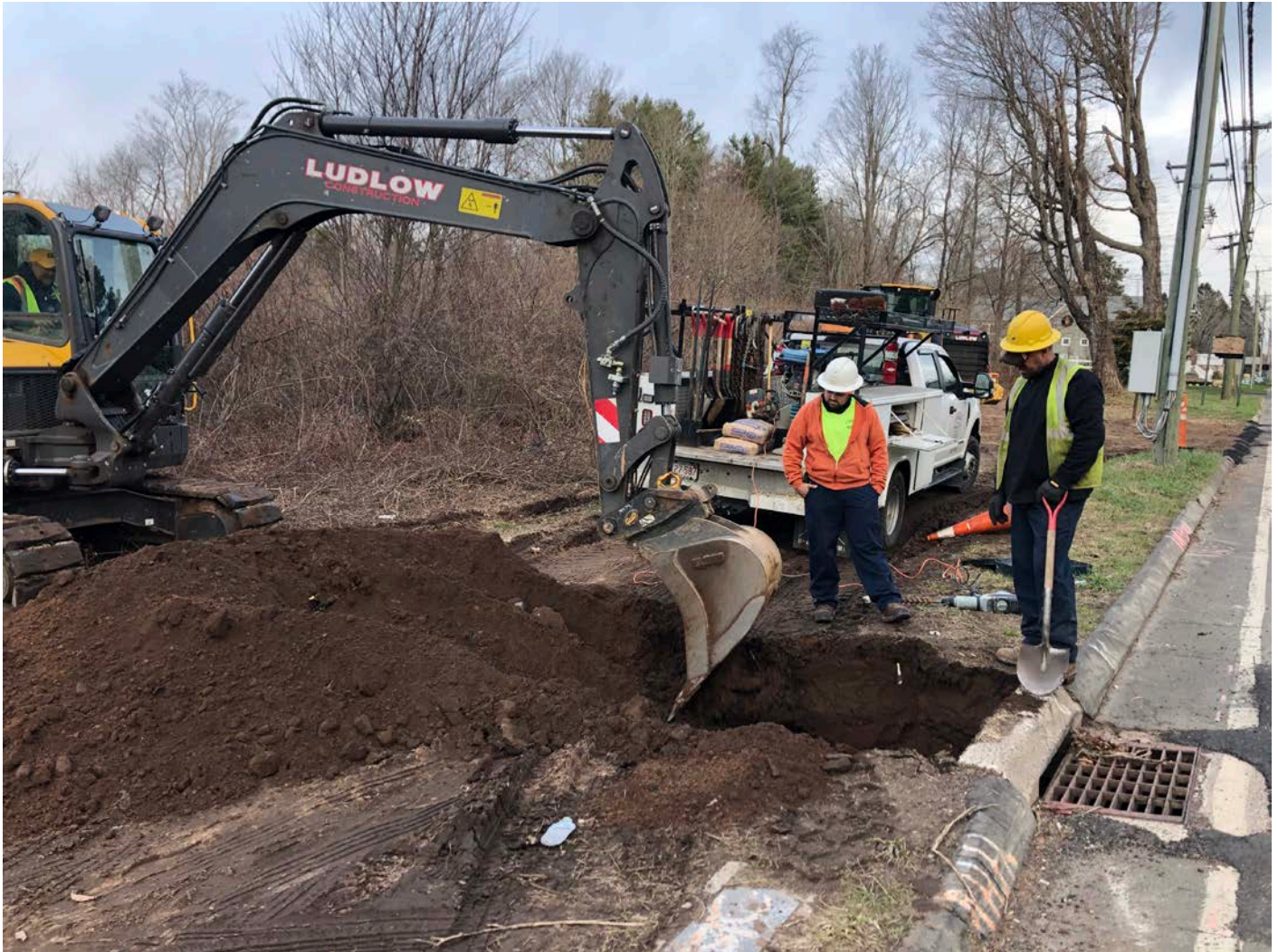
Picture 2: Ludlow excavating at ~Station 161+20 as they begin the installation of a 2" PVC drain line that will connect the PRV vault sump to the storm drain line that is connect to the catch basin depicted above. View to the north.
