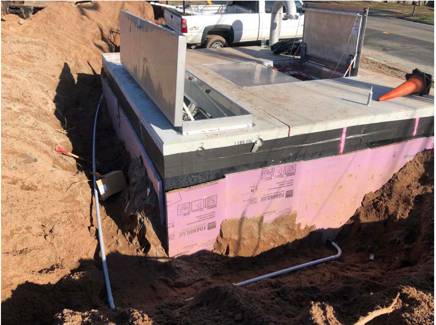
Picture 7: PVC drain line that has been connected to the south side of the PRV vault located at ~161+30 to the west of Main Street, Durham. View to the northeast.
