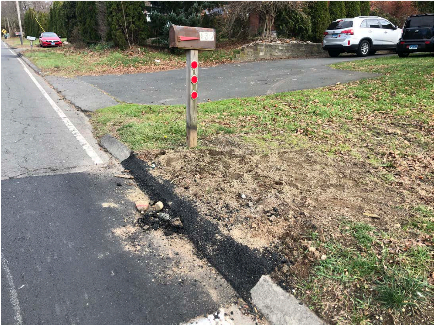
Picture 6: Temporary curb patch located at 435 Main Street, Durham that was the subject of a complaint. Ludlow removed the asphalt that was pushed into the road and added additional loam to the east of the curb. View to the northeast.
