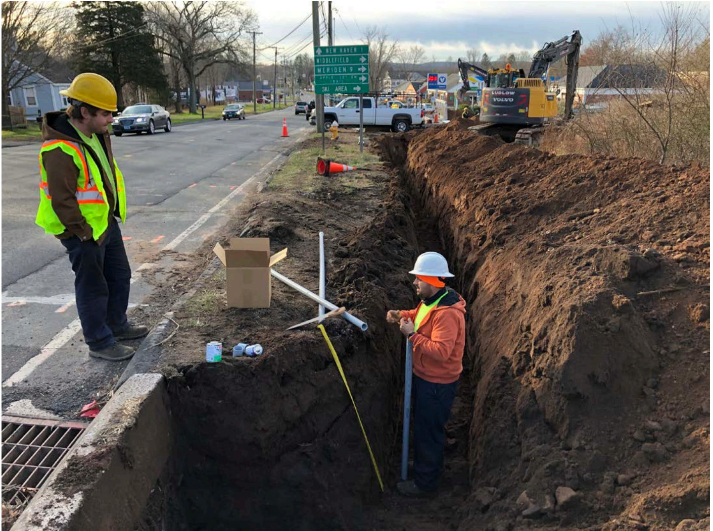
Picture 4: Ludlow in the process of installing a 2" PVC drain line that will connect the PRV vault sump to the storm drain line located at Station 161+20 on the west side of Main Street. View to the south.
