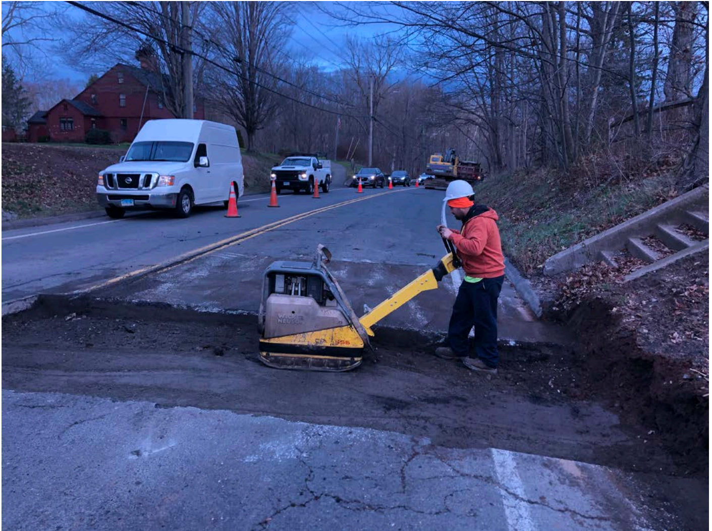
Picture 1: Ludlow compacting 1.5" processed gravel at the curb stop overcut on the northbound lane at 127 Main Street, Durham. View to the north.
