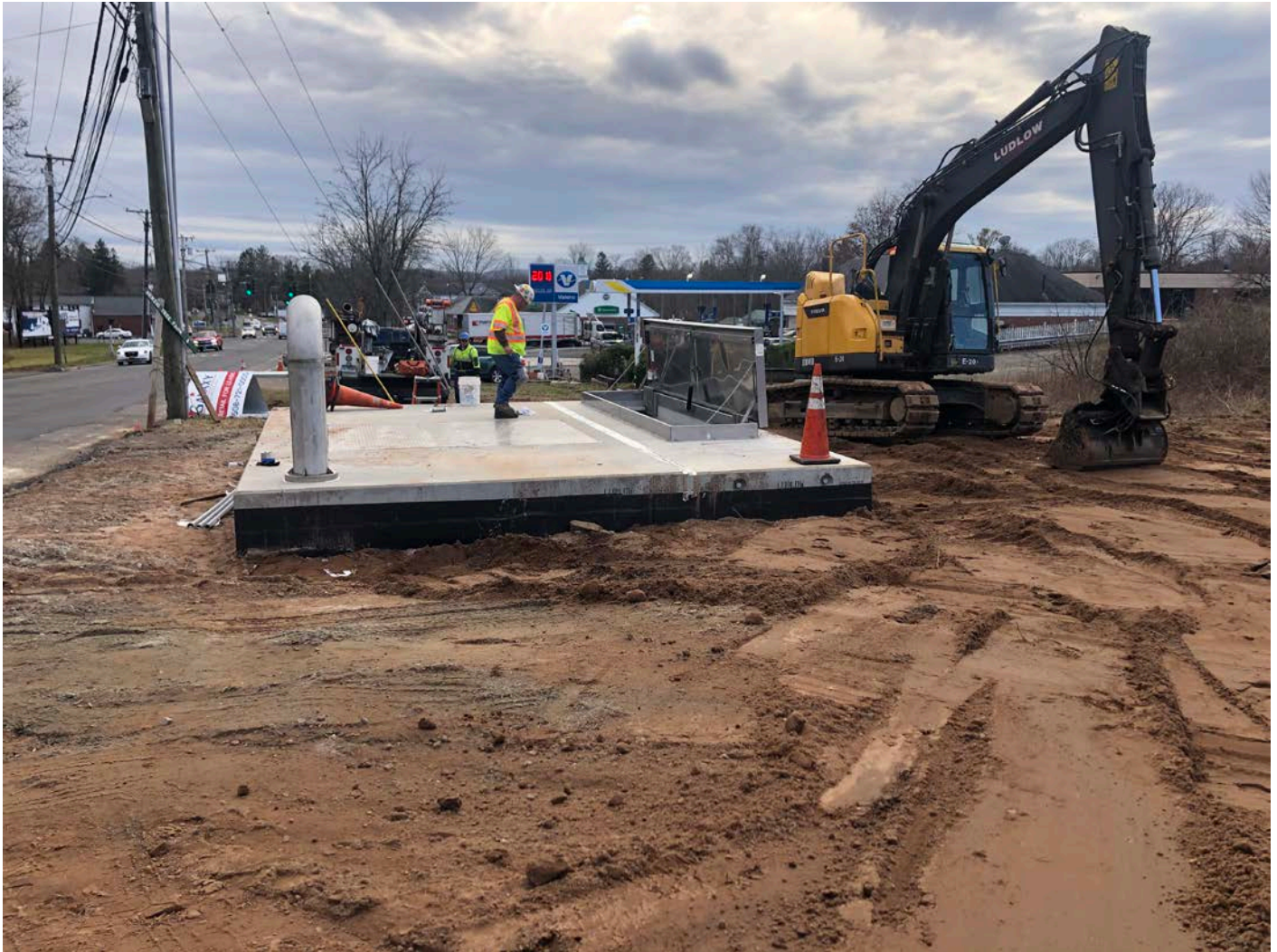
Picture 10: PRV vault after Ludlow backfilled around it after installing a PVC drain line from the vault to a storm drain located at Station ~161+20. View to the south.
