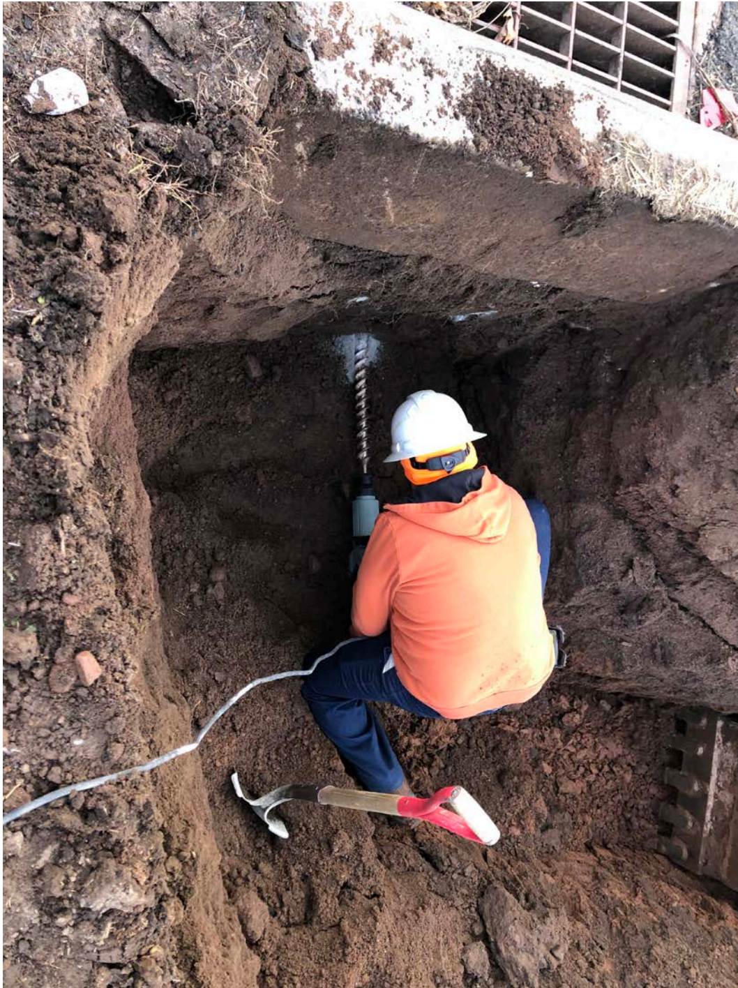
Picture 3: Ludlow drilling into the storm drain line located at Station 161+20 as they prepare to install a 2" PVC drain line that will connect the PRV vault sump to the storm drain line. View to the east.
