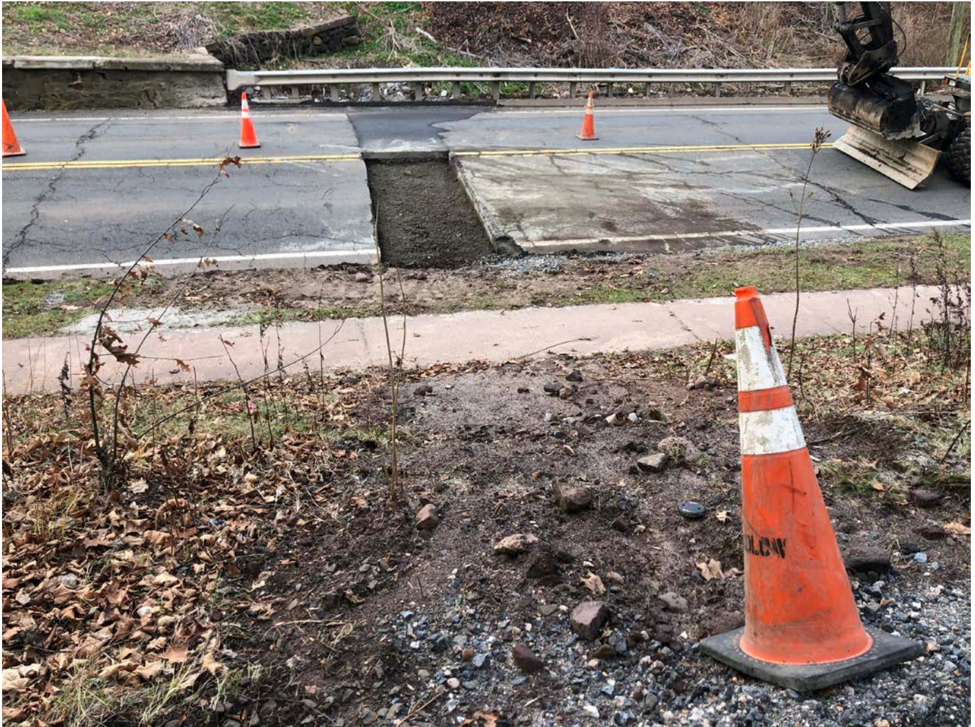
Picture 5: Curb stop overcut that is ready for permanent paving, located at 119 Main Street, Durham. View to the west.
