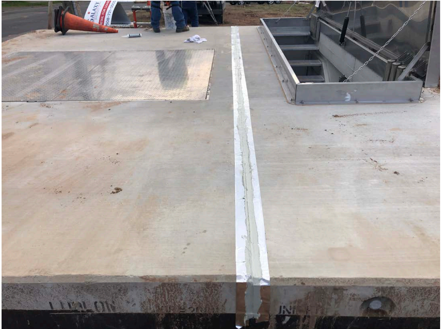
Picture 9: Seam between PRV vault roof sections that United Concrete sealed today (tape was removed once caulk set). View to the south.
