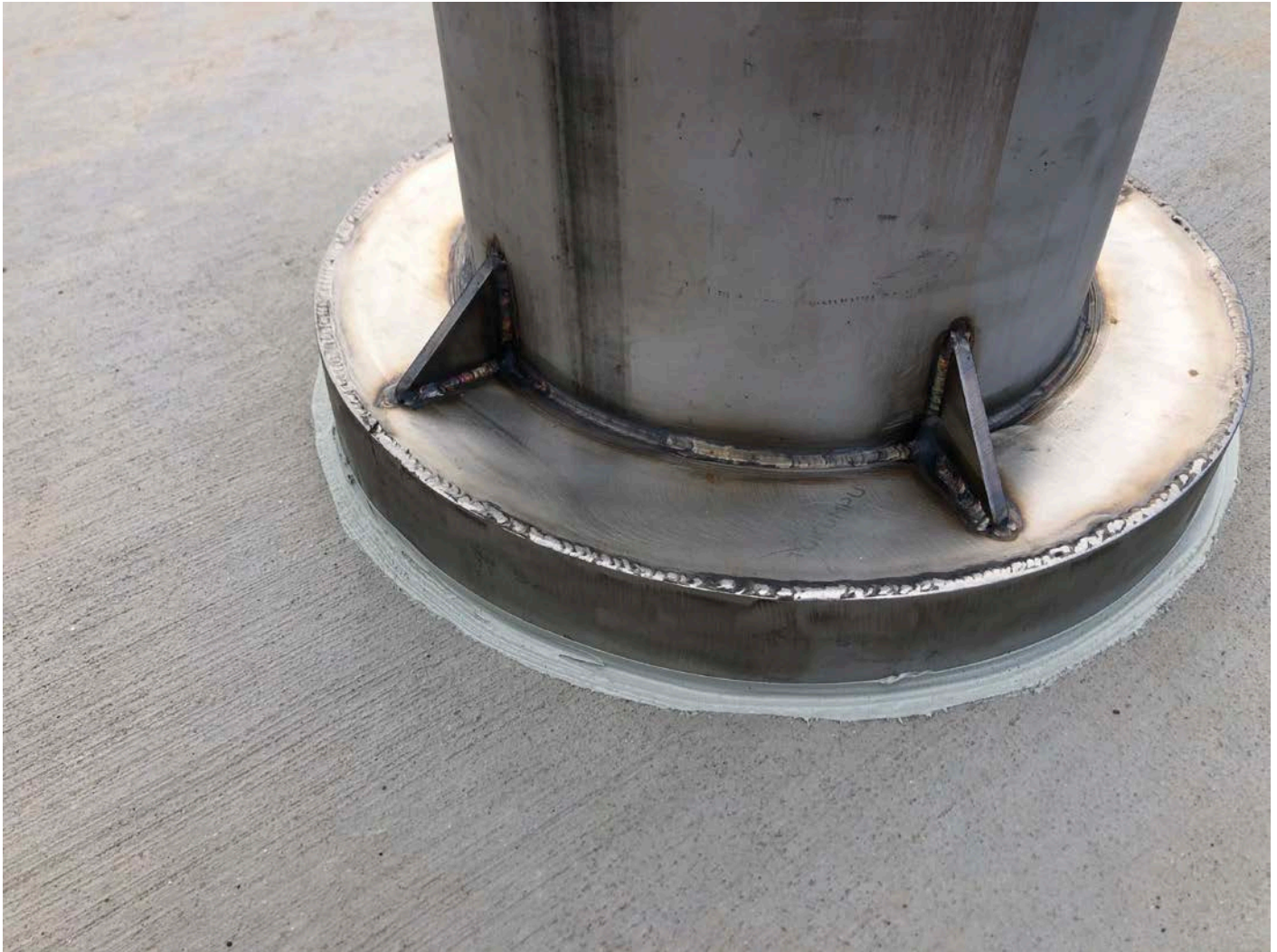
Picture 8: Seam between the PRV vault roof and the vent pipe located on the northeast corner of the vault that United Concrete sealed today. View to the southwest.
