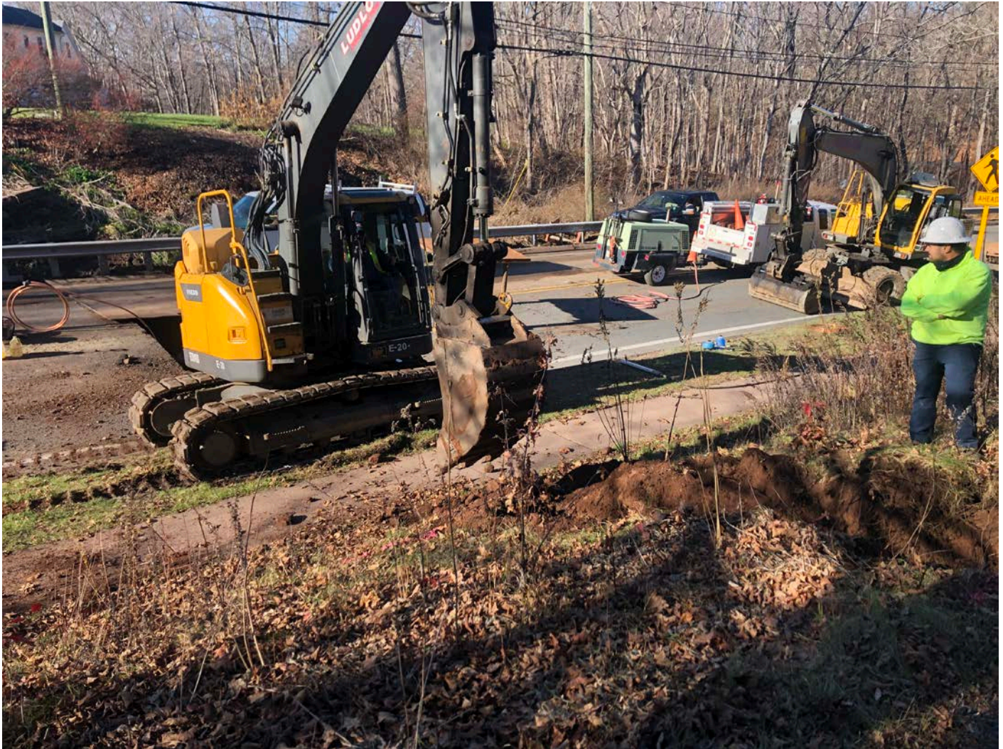
Picture 7: Ludlow excavating on the 127 Main Street, Durham property for the installation of a curb stop. View to the northwest.
