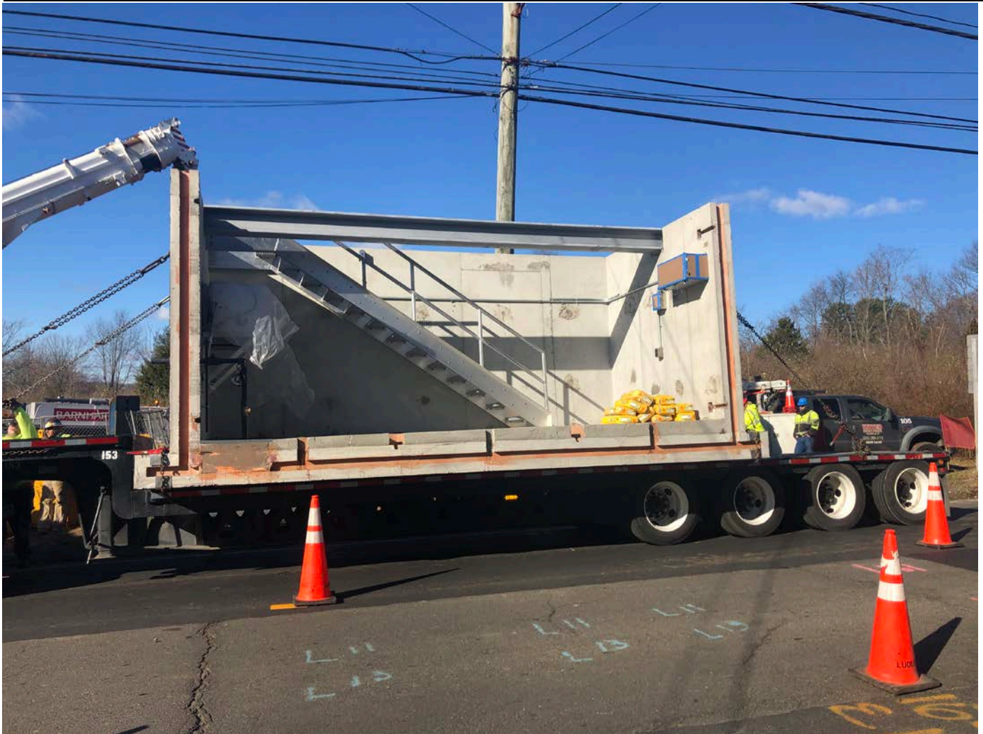
Picture 4: One of the sections of the PRV vault that was installed at Station 161+30 to the west of Main Street, Durham today.
