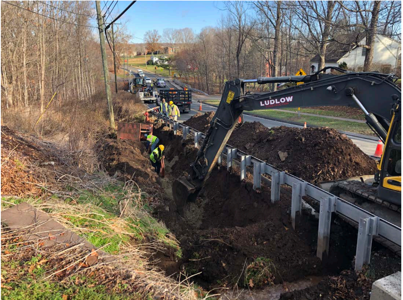
Picture 1: Ludlow excavating to the west of Main Street as part of installation activities for a curb stop at 127 Main Street, Durham. View to the northeast.
