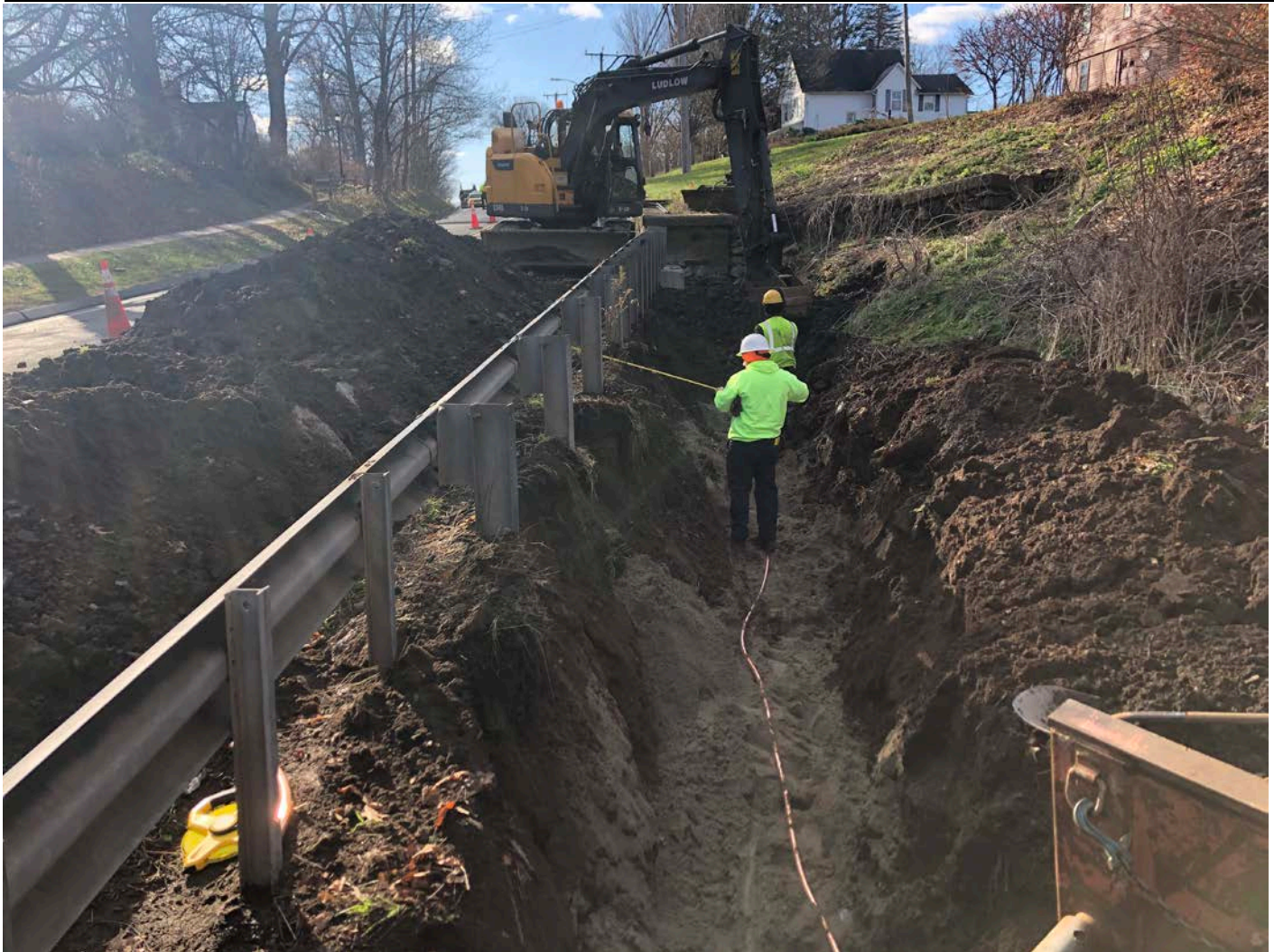
Picture 3: Ludlow installing 1" copper service line 6.5' to the west of Main Street, Durham for the installation of a curb stop at 127 Main Street. View to the south.
