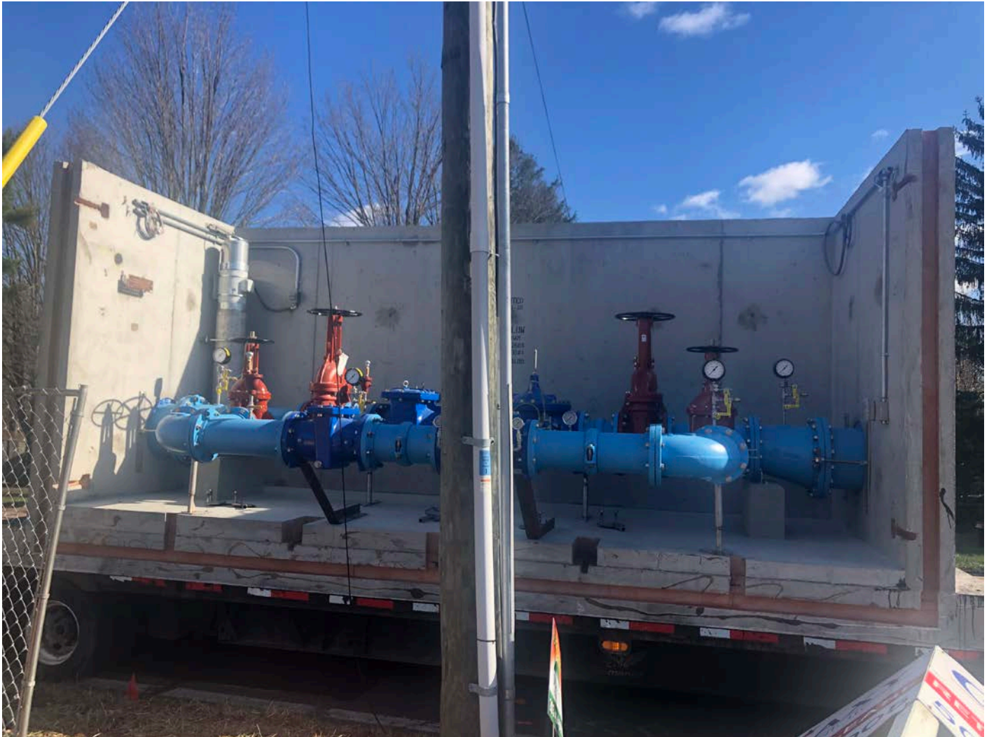
Picture 5: The second section of the PRV vault that was installed at Station 161+30 to the west of Main Street, Durham today.
