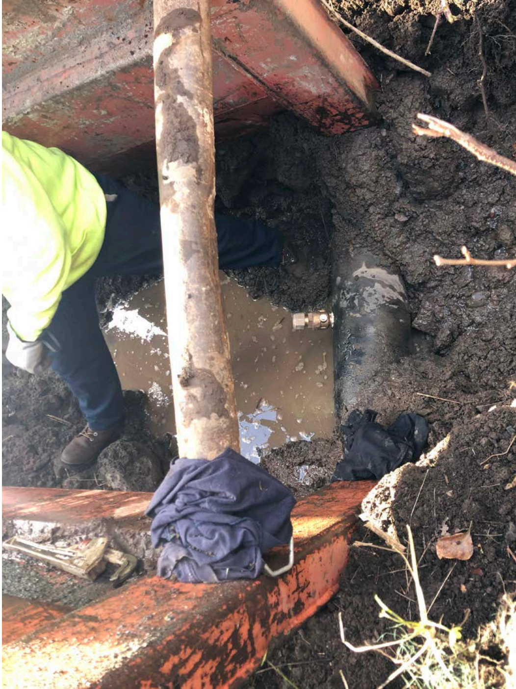
Picture 2: Corporation stop that Ludlow installed on the existing Town waterline as part of curb stop installation activities for 127 Main Street, Durham.
