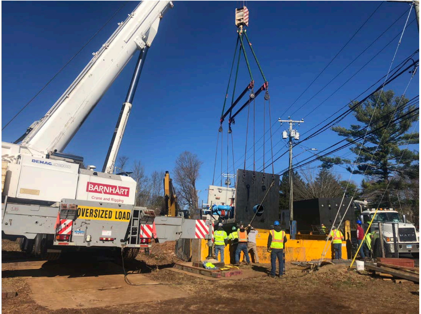
Picture 6: United hoisting the first of two sections of the PRV vault at Station 161+30, to the west of Main Street, Durham. View to the north.
