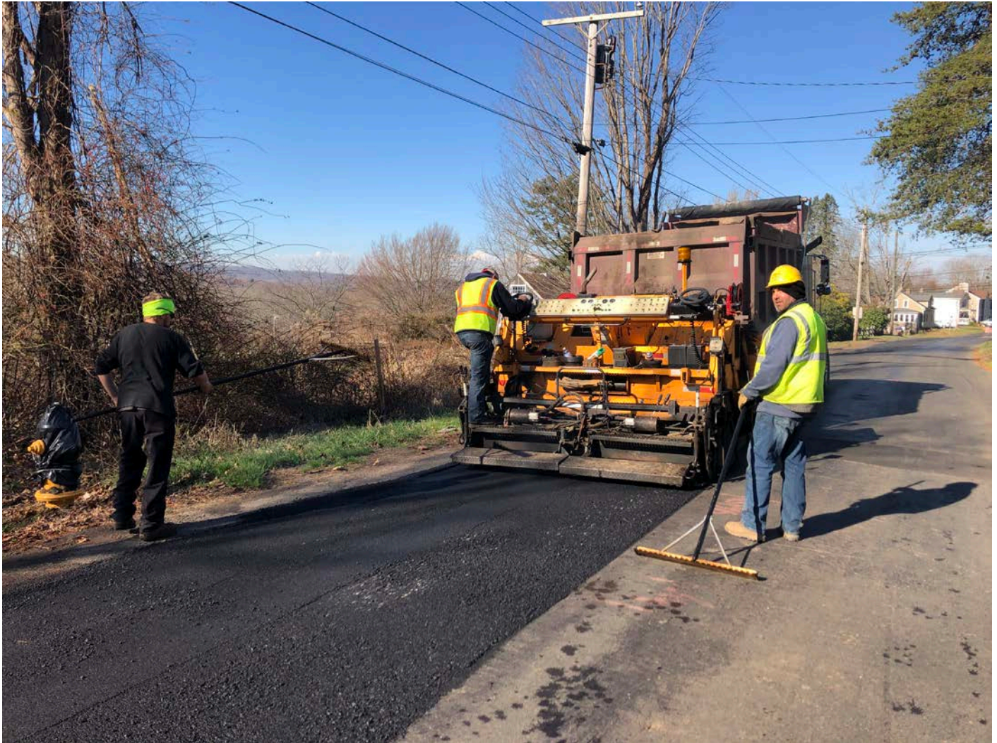
Picture 5: Ludlow shim coating over temporary trench pavement on the southbound lane of Maple Avenue, Durham at Station 913+50. View to the northwest.
