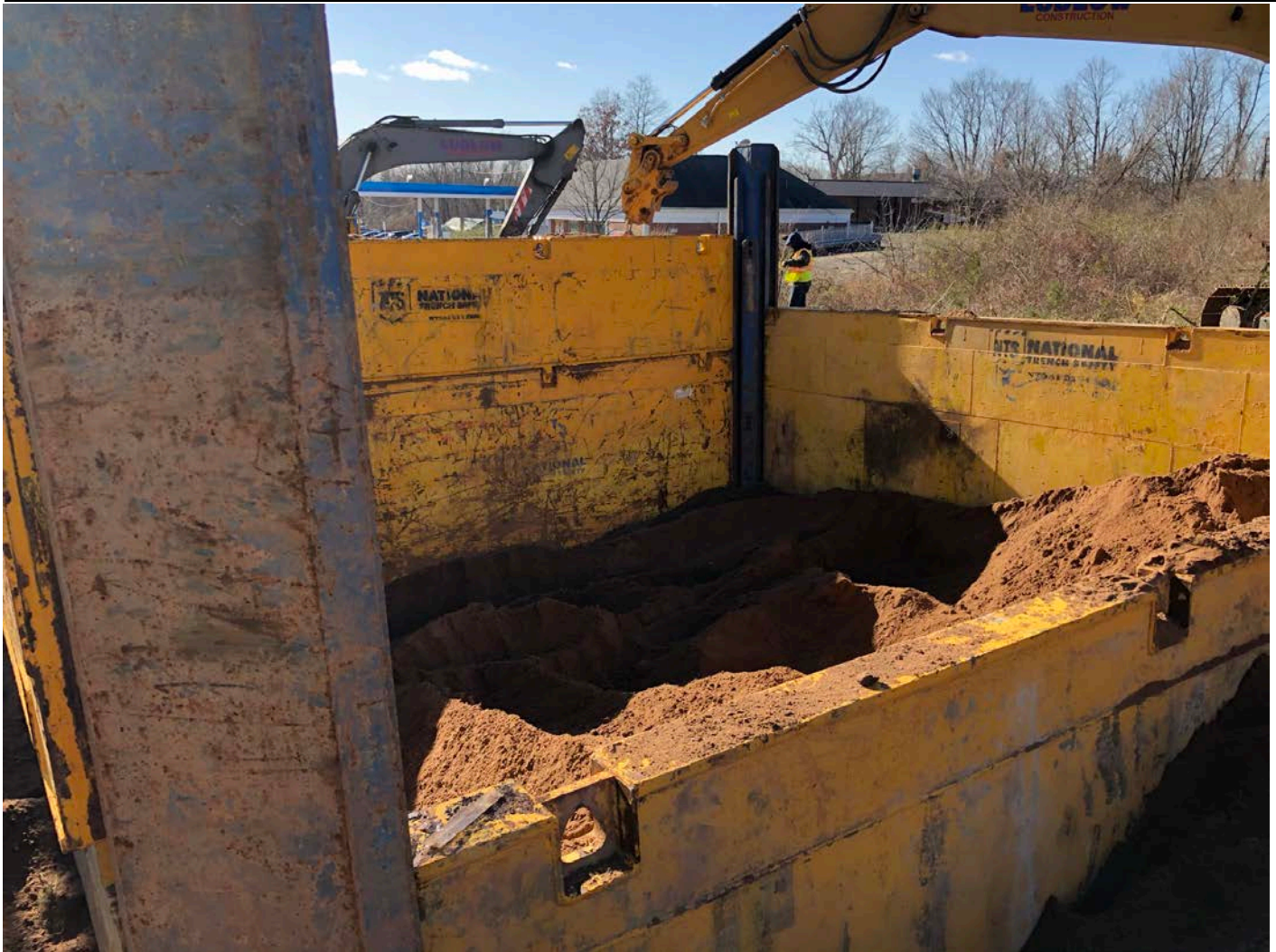
Picture 3: Ludlow excavating the site for the Pressure Reducing Valve Vault.
