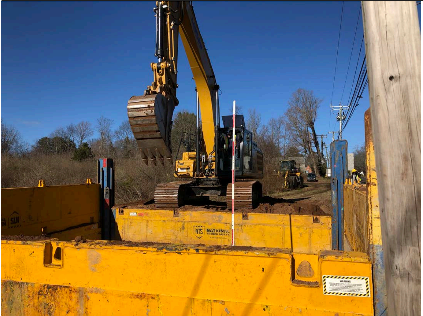
Picture 4: Ludlow confirming the depth of the valve vault.
