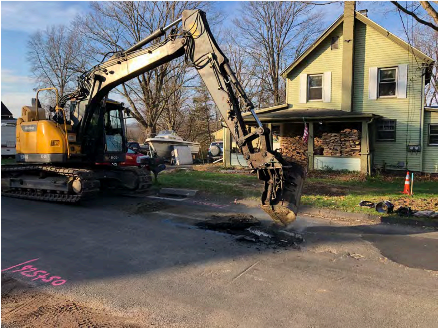
Picture 3: Ludlow beginning to excavate on the southbound lane of Maple Avenue, Durham at Station 925+55 to install a gate valve to help isolate a leak in the 8" DIP water line they installed earlier in the year. View to the west.
