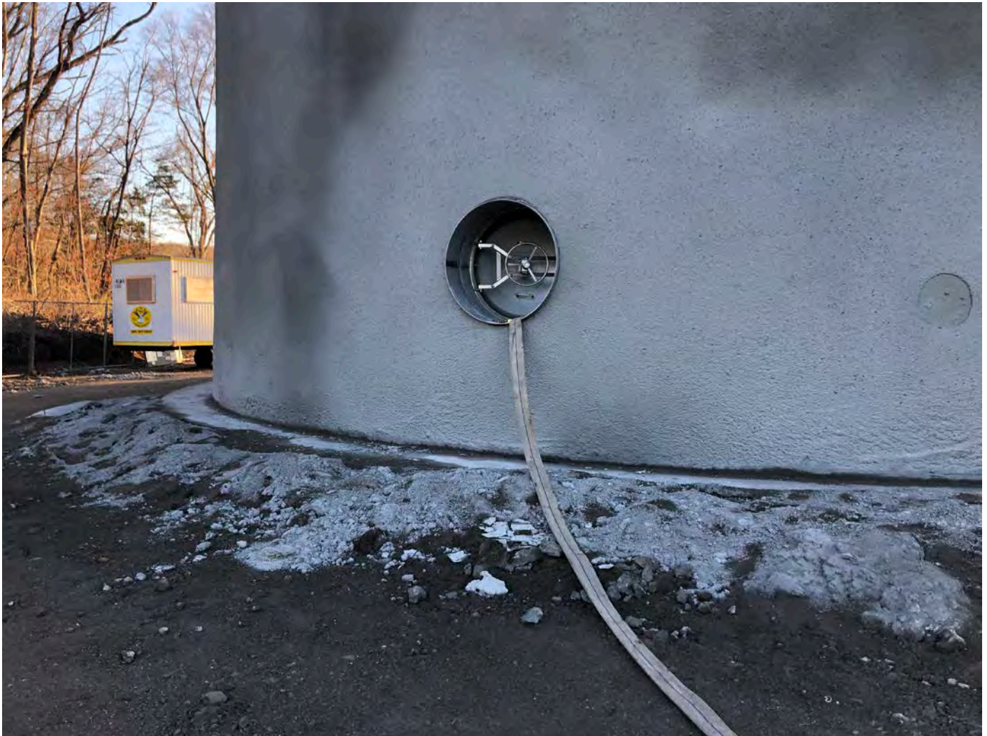
Picture 1: Hose that Ludlow connected to a nearby hydrant and placed into the water tank located to the east of the Shared Access Driveway, Middletown. DN Tanks would later continue placing water into the tank until the level was brought up just below the bottom of the manway hatch. View to the east.
