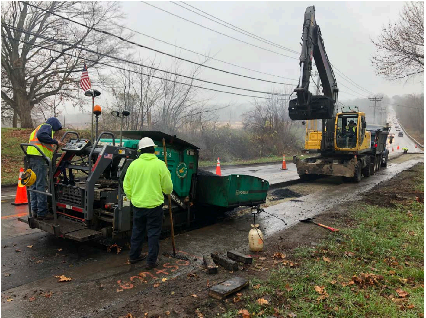
Picture 3: Ludlow excavating pavement for trench overcuts on the westbound lane of Main Street, Durham between Stations 607+50 and 609+60 as part of permanent paving activities. View to the southwest.
