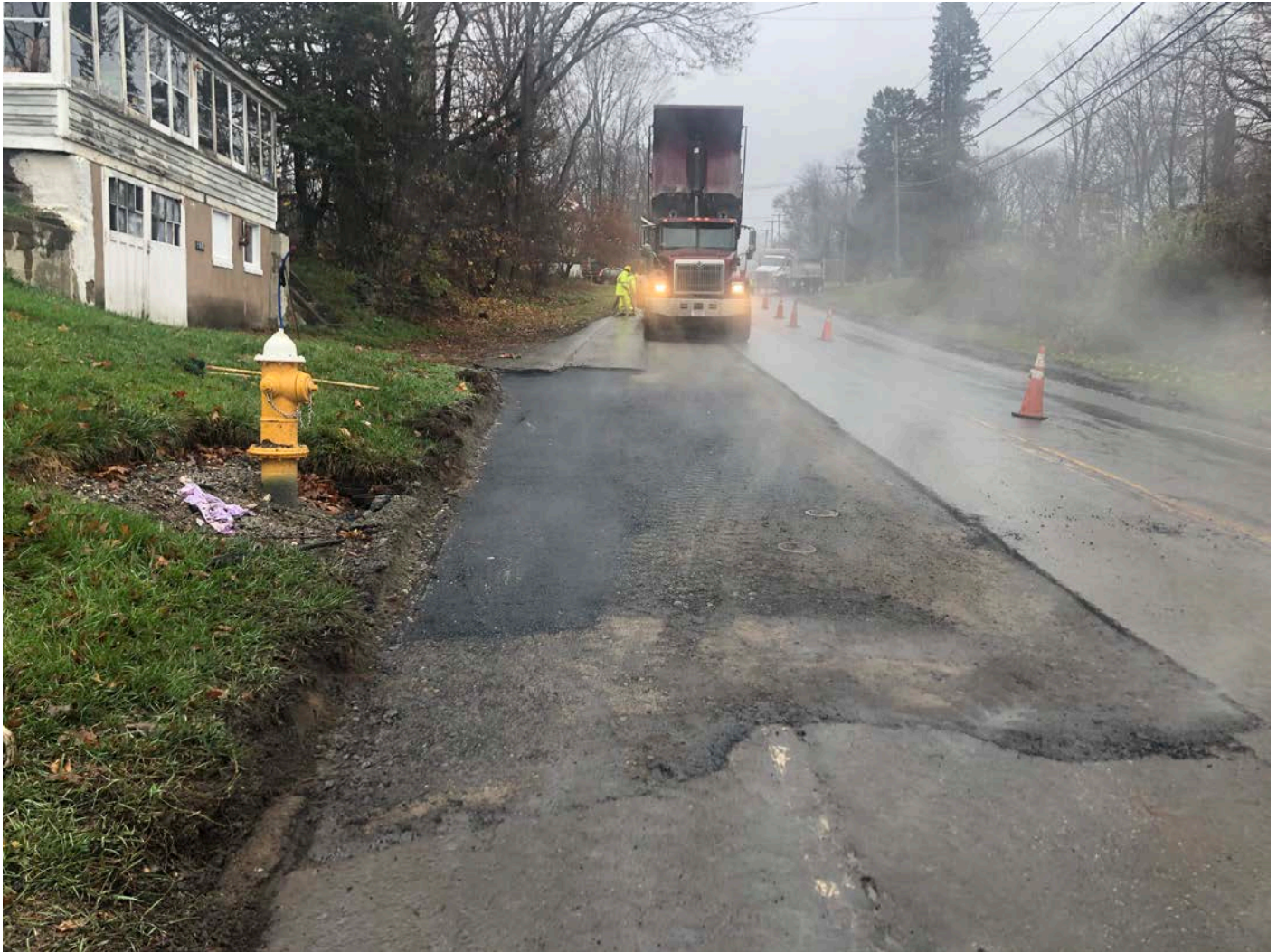
Picture 8: Second lift of asphalt placed and compacted on the westbound lane of Route 68, Durham as part of permanent pavement activities on trench overcuts. View to the east.
