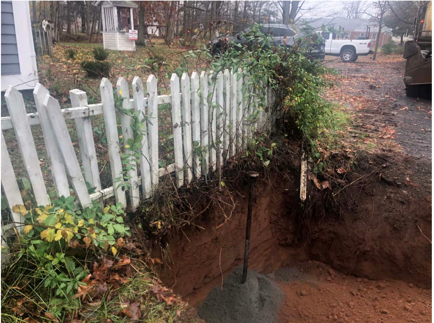
Picture 9: Curb stop that Ludlow installed at 119 Main Street, Durham. View to the north.
