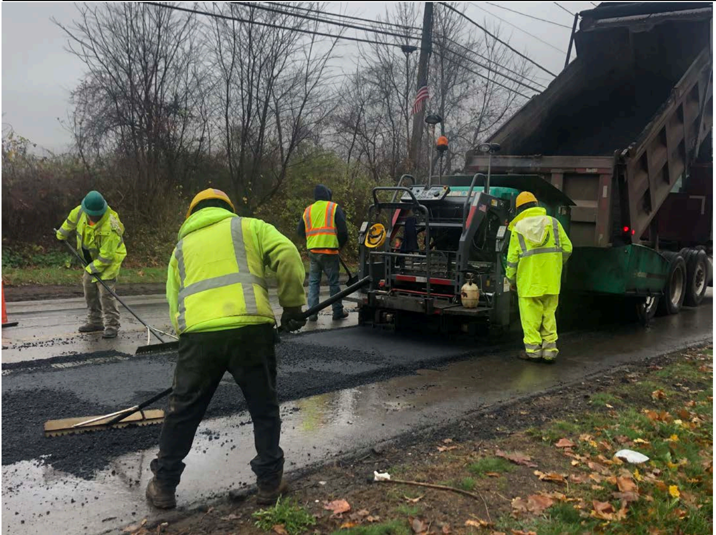
Picture 7: Ludlow placing asphalt on the westbound lane of Route 68, Durham as part of permanent pavement activities on trench overcuts. View to the southwest.
