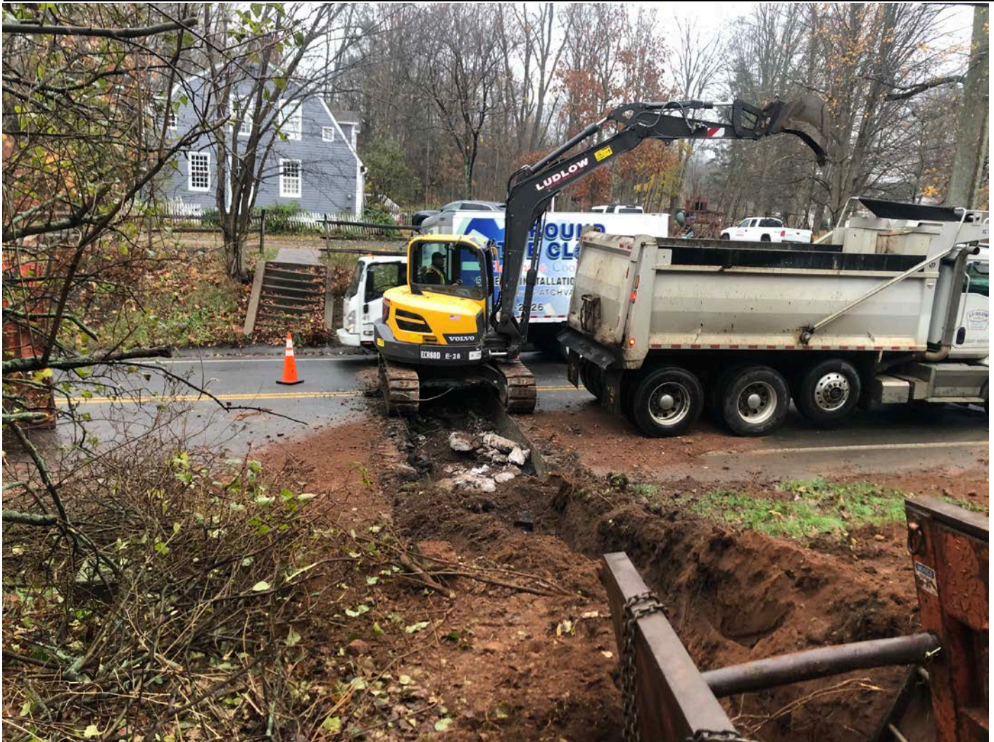
Picture 1: Ludlow excavating from the 120 Main Street residence (where the Town water line is located) to the 119 Main Street residence as part of installation activities for the placement of a water service to 119 Main Street. Main Street, Durham; view to the east.
