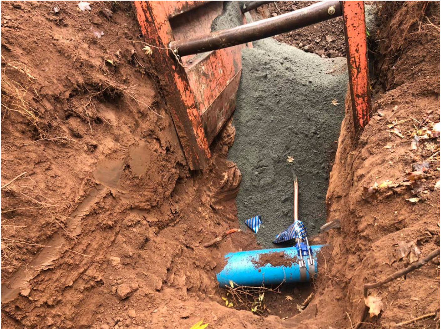
Picture 4: 1" copper water service line that Ludlow just installed on the corporation stop they installed on the 8" PVC Town water line on the 120 Main Street property for the installation of a curb stop at 119 Main Street, Durham. View to the east.
