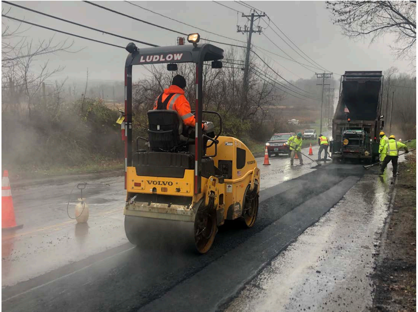
Picture 6: Ludlow compacting pavement on the westbound lane of Route 68, Durham as part of permanent pavement activities on trench overcuts. View to the southwest.
