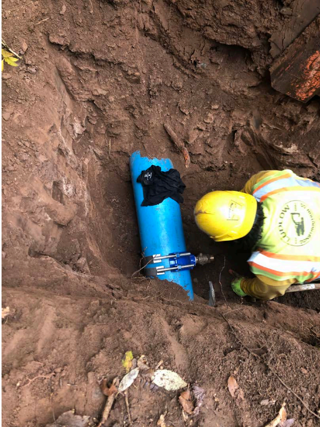
Picture 2: Ludlow installing a saddle and a corporation stop on the 8" PVC Town water line located on the 120 Main Street property for the installation of a curb stop at 119 Main Street, Durham.
