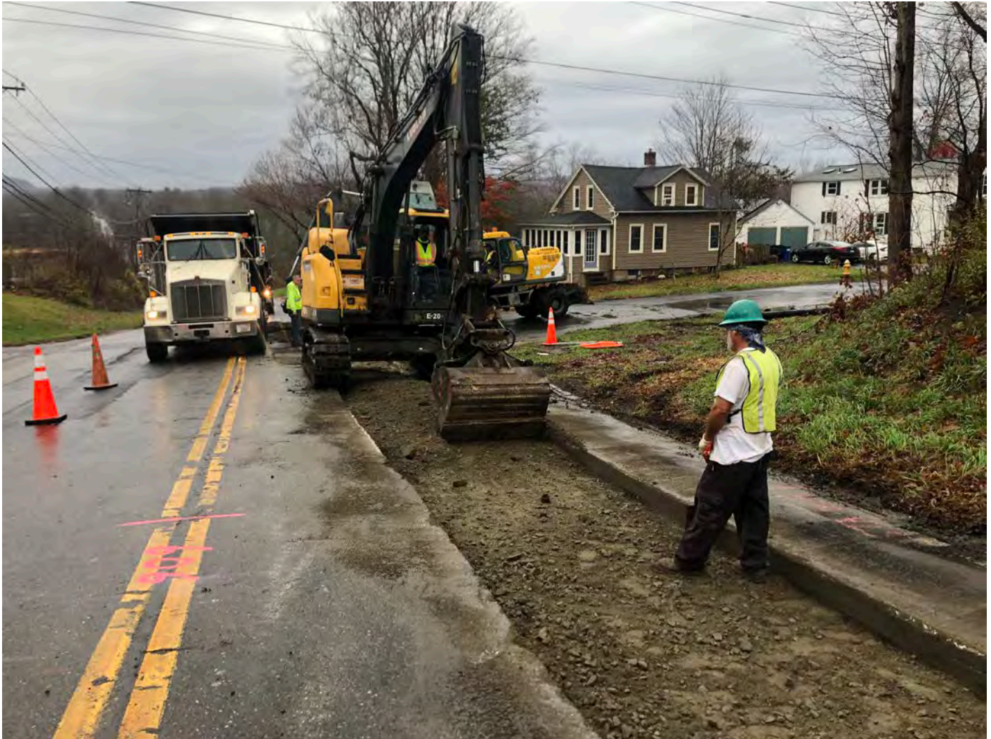
Picture 1: Ludlow grading 1.5" gravel between Stations 604+75 to 607+50 on the westbound lane of Route 68, Durham as part of permanent paving activities. View to the west.
