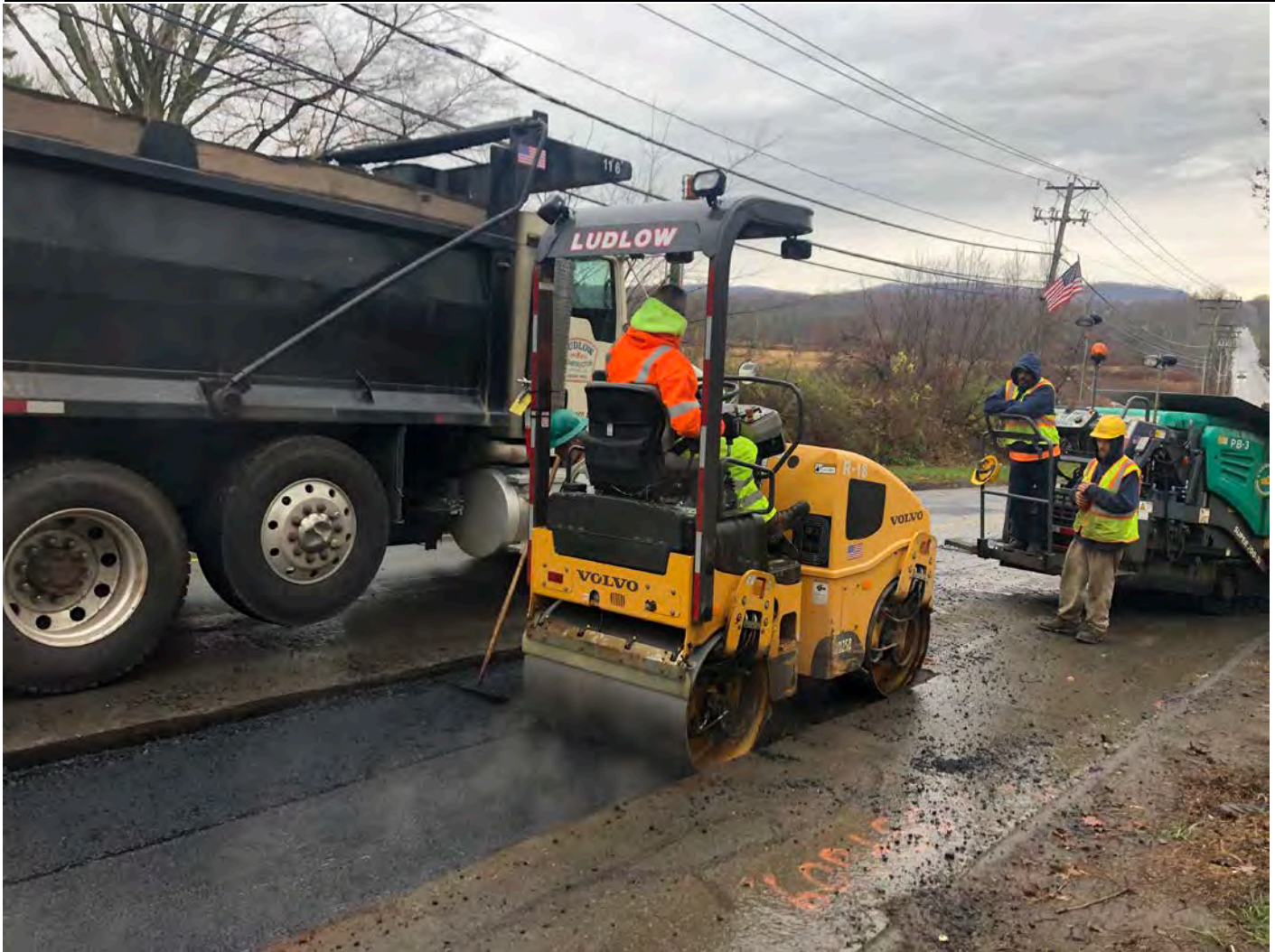
Picture 3: Ludlow compacting asphalt between Stations 604+75 to 607+50 on the westbound lane of Route 68, Durham as part of permanent paving activities. View to the southwest.
