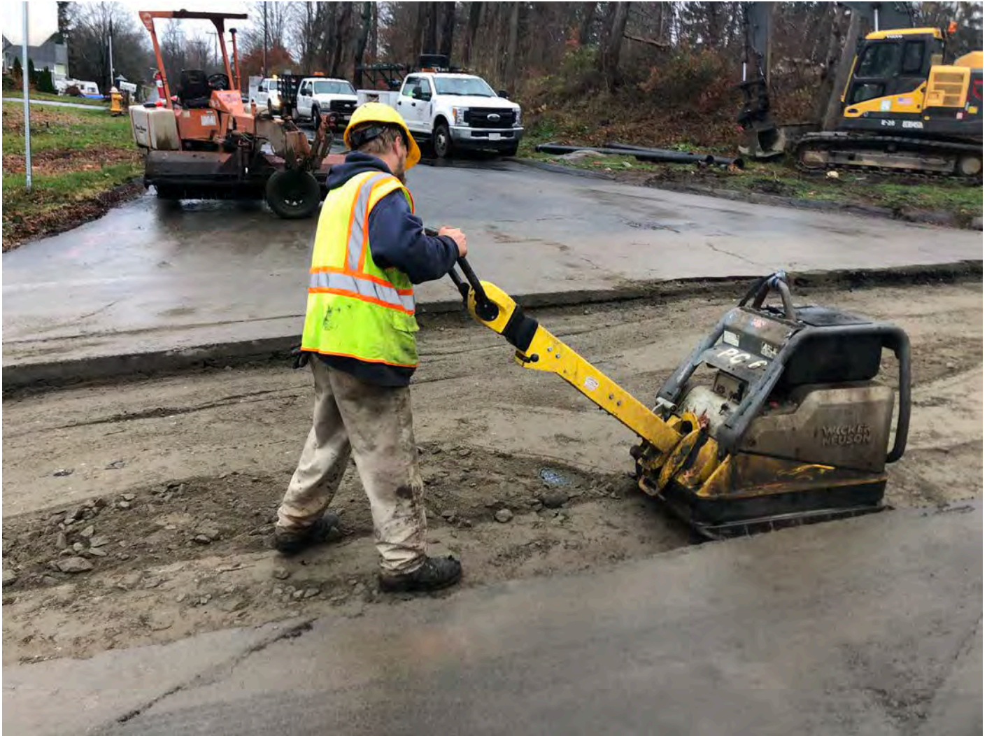
Picture 2: Ludlow compacting 1.5" gravel between Stations 604+75 to 607+50 on the westbound lane of Route 68, Durham as part of permanent paving activities. View to the north.
