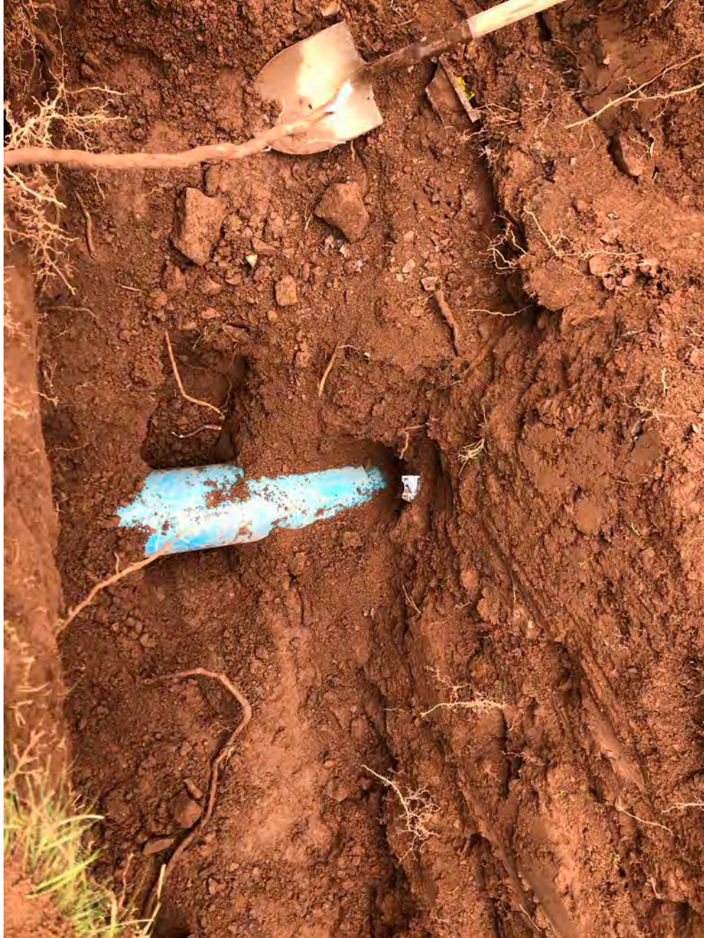
Picture 7: Ludlow daylighted an 8" blue PVC line (believed to be a Town water main) located 29.5' west of the edge of Main Street while excavating for the installation of a curb stop at 120 Main Street, Durham. View to the east.
