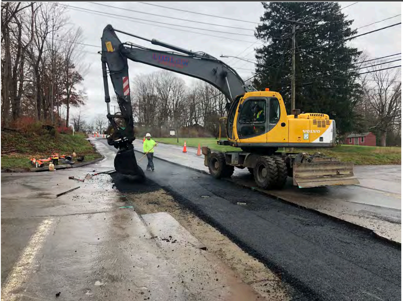
Picture 4: Ludlow placing asphalt in sliver slab cutout on the westbound lane of Route 68, Durham as part of permanent paving activities. View to the east.
