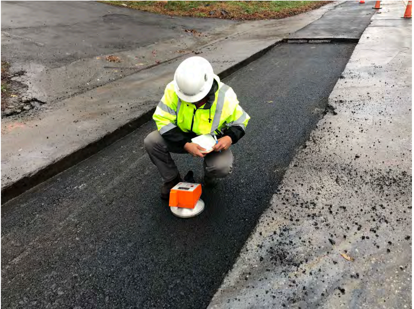
Picture 5: JTC collecting compaction data from asphalt placed and compacted between Stations 604+75 to 607+50 on the westbound lane of Route 68, Durham as part of permanent paving activities. View to the southwest.
