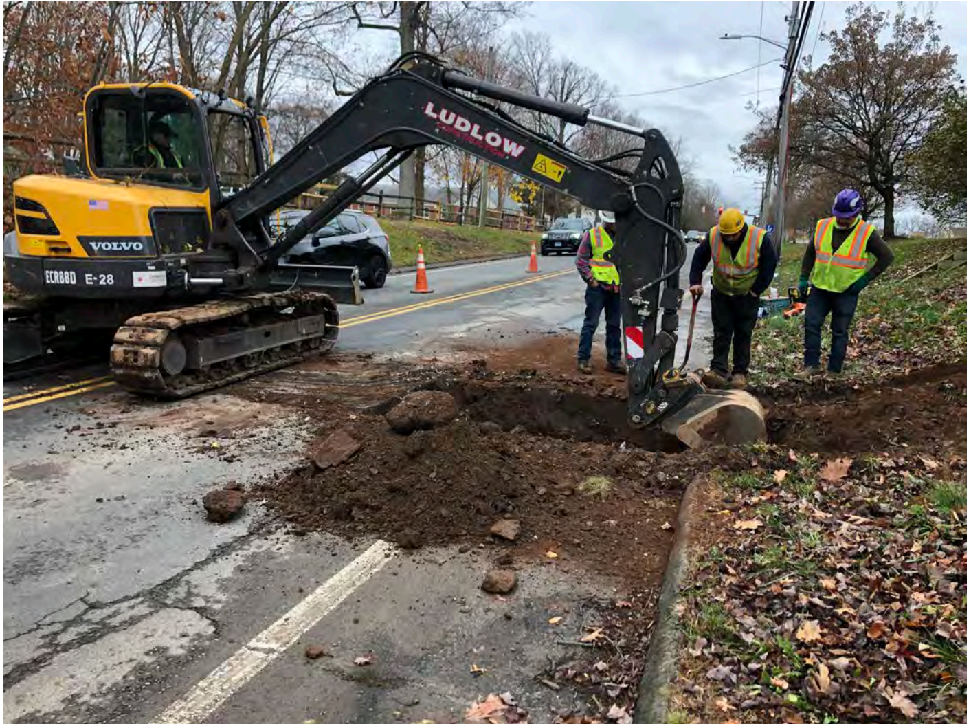
Picture 8: Ludlow excavating a test pit in front of 120 Main Street to further investigate the location of the Town water line that services Main Street, Durham. View to the south.
