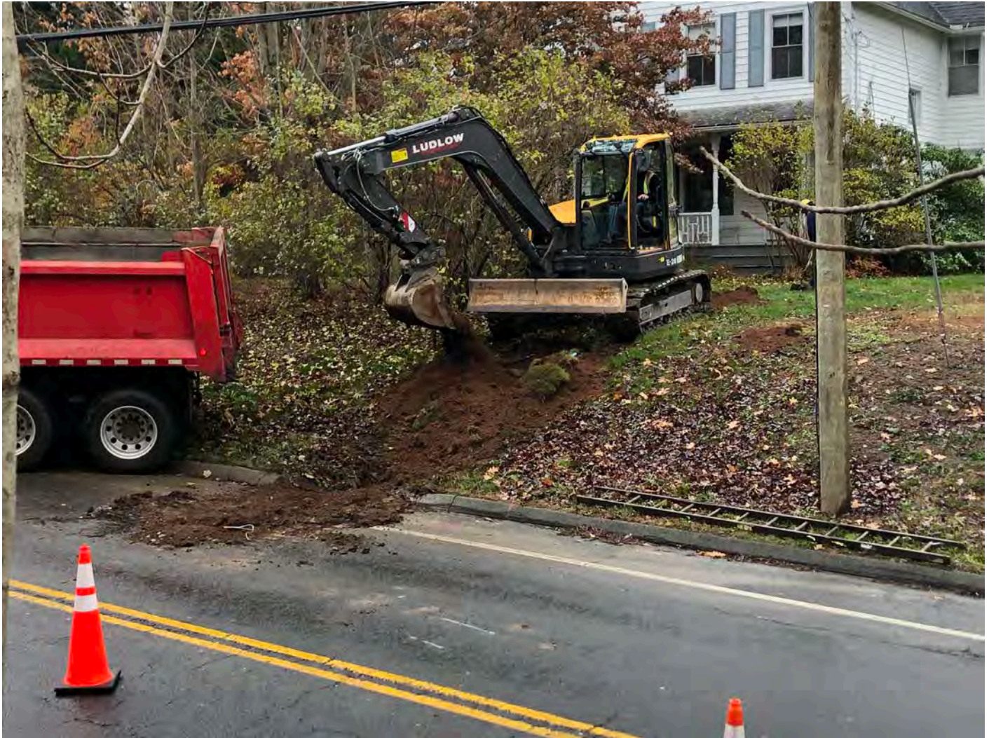
Picture 6: Ludlow excavating for the installation of a curb stop and corporation stop at 120 Main Street, Durham. View to the southwest.
