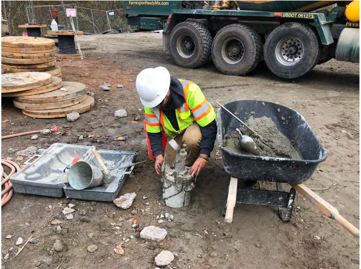
Picture 9: JTC preparing an air entrainment test from the first load of shotcrete delivered to the water tank work zone today, east of the Shared Access Driveway, Middletown. View to the northeast.
