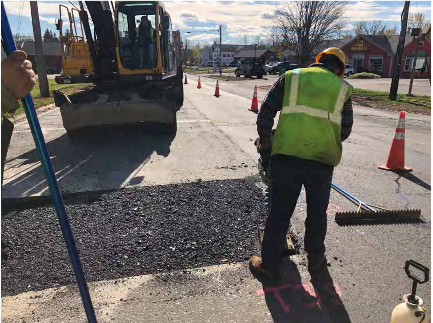
Picture 8: Ludlow compacting a second lift of asphalt on a curb stop overcut located on the northbound lane of Main Street, Durham as part of permanent paving activities. View to the south.
