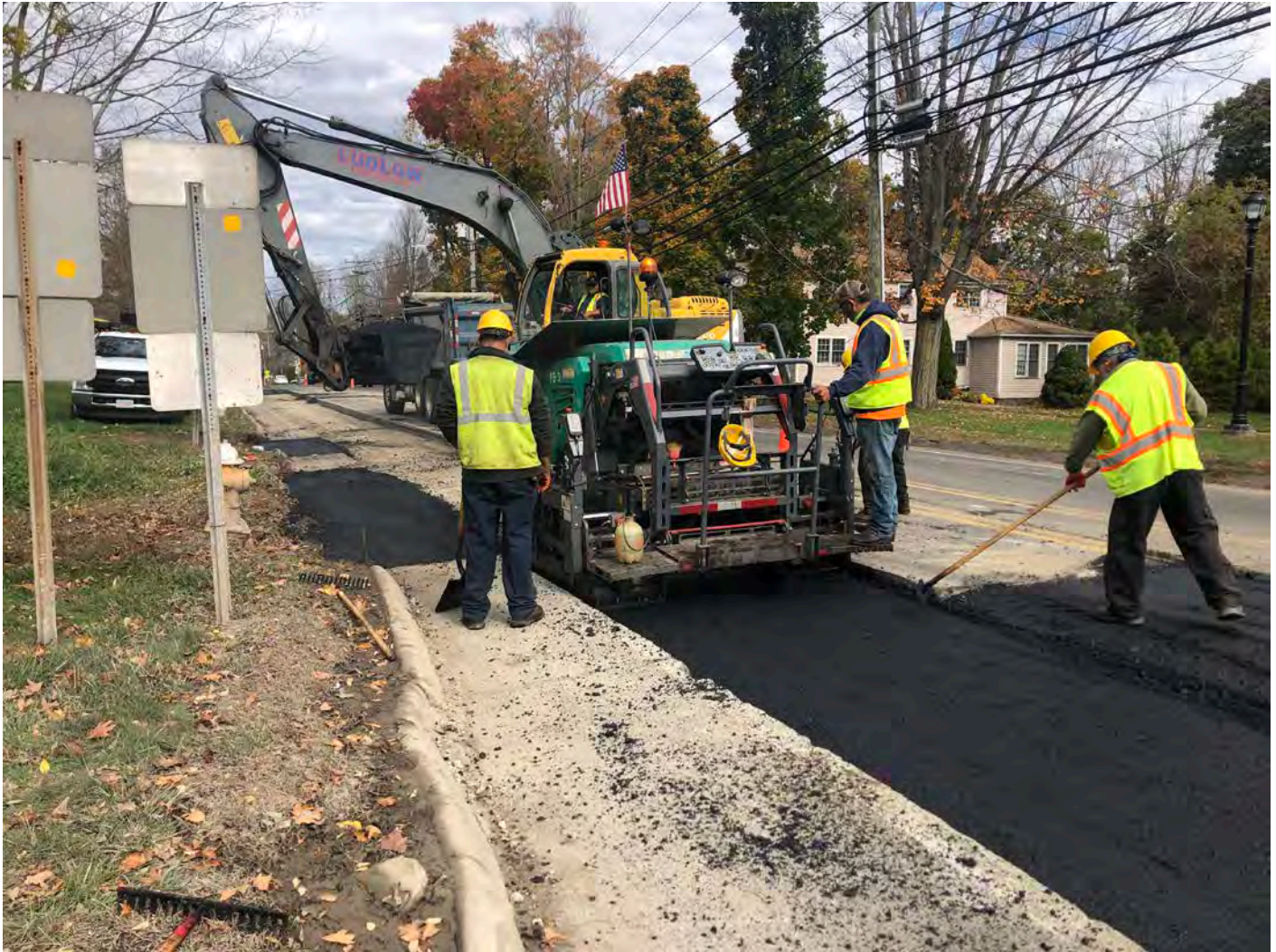
Picture 6: Ludlow applying the first lift of asphalt between Stations 192+70 and 195+30 on the southbound lane of Main Street, Durham as part of permanent paving activities. View to the northeast.
