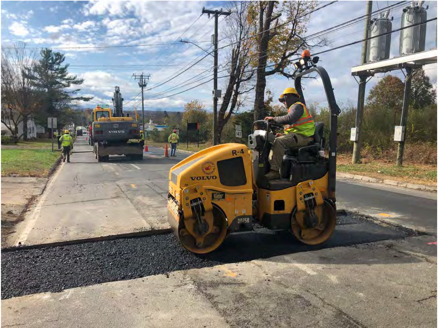
Picture 7: Ludlow compacting a second lift of asphalt on a curb stop overcut located on the northbound lane of Main Street, Durham as part of permanent paving activities. View to the south.
