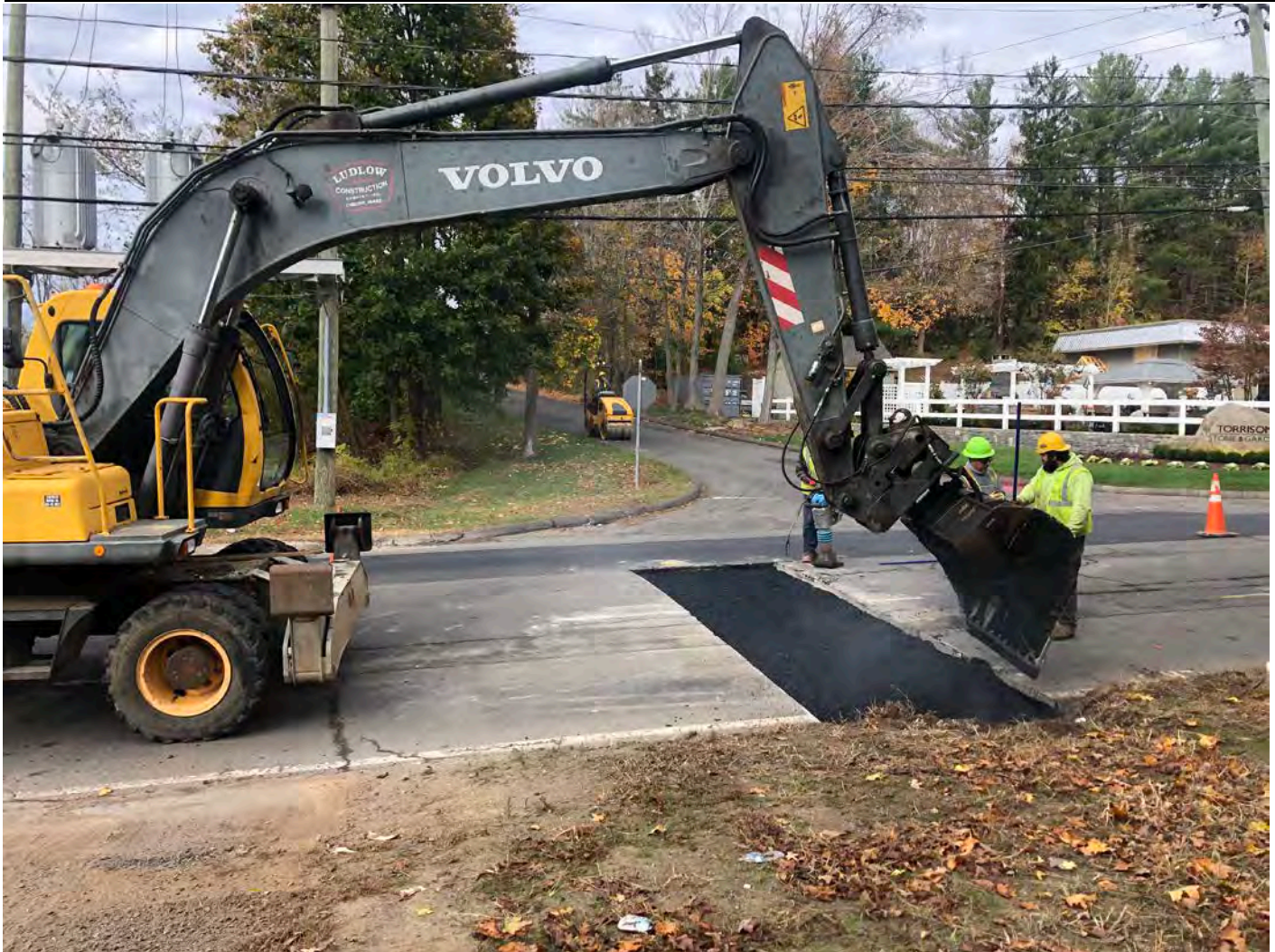
Picture 4: Ludlow applying a second lift of asphalt on a curb stop overcut on the northbound lane of Main Street, Durham, as part of permanent paving activities. View to the west.
