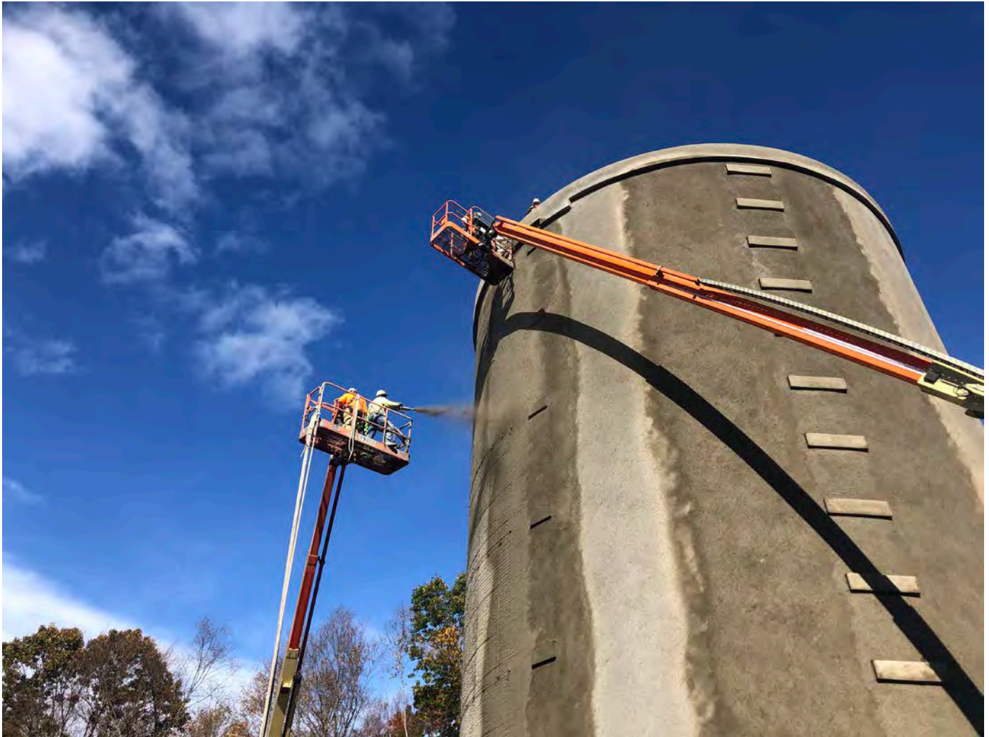
Picture 10: DN Tanks applying shotcrete to the west side of the water tank, east of the Shared Access Driveway, Middletown. View to the north.
