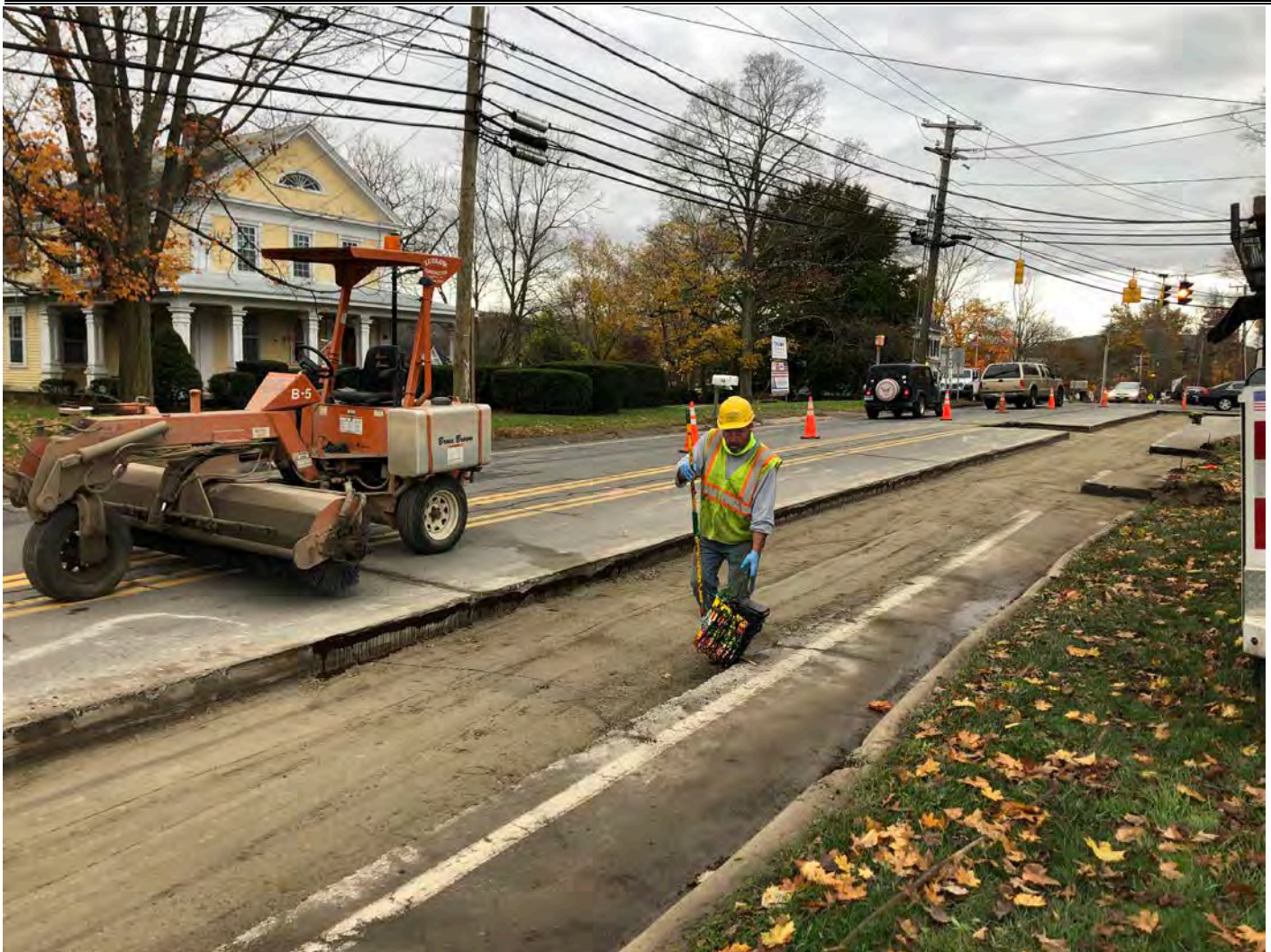
Picture 3: Ludlow applying tack coat to the edge of cut pavement between Stations 192+70 and 195+30 as part of permanent paving activities on the southbound lane of Main Street, Durham. View to the southeast.
