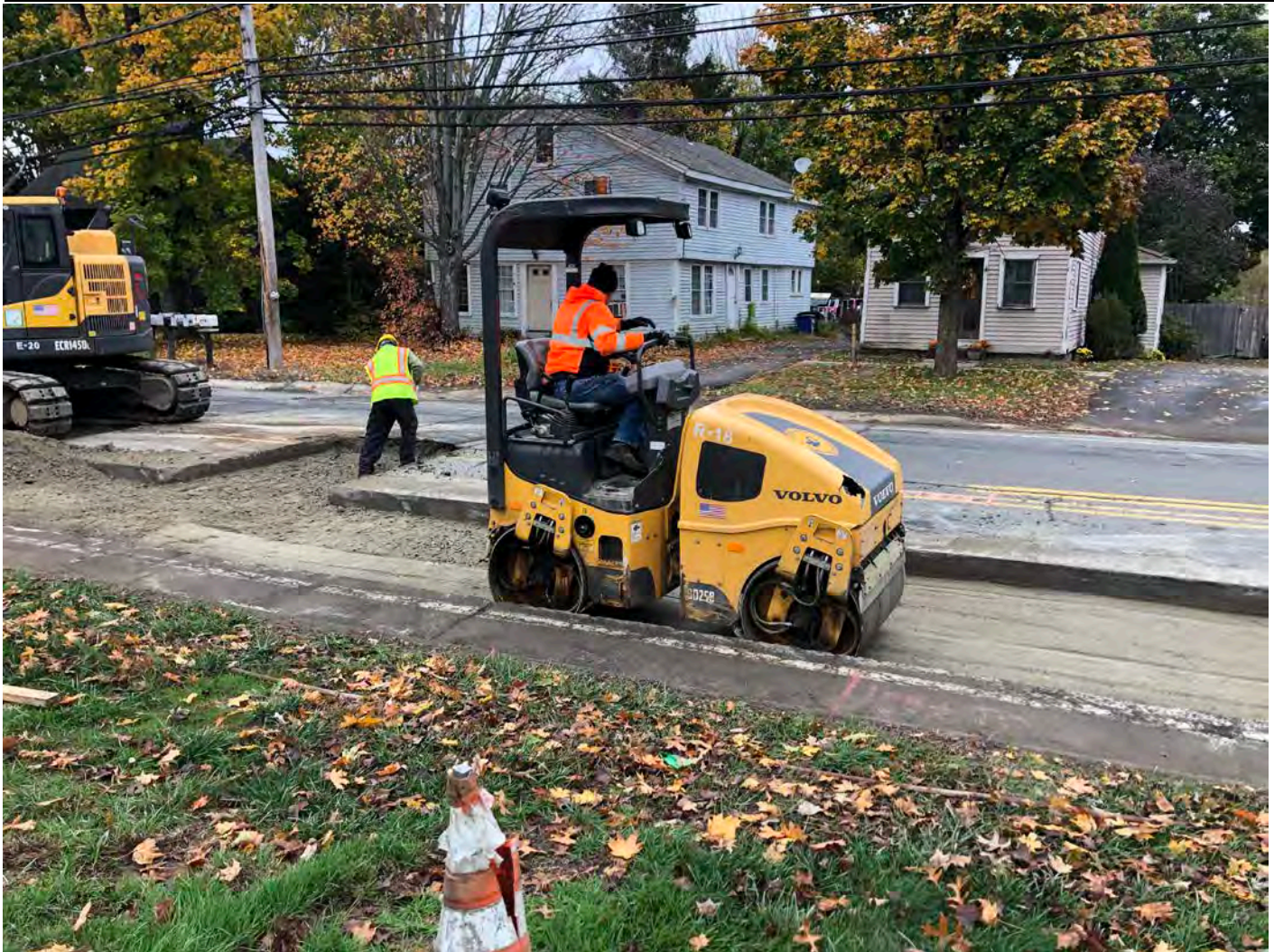
Picture 1: Ludlow compacting 1.5" processed gravel on the southbound lane of Main Street, Durham, as part of permanent paving activities. View to the west.
