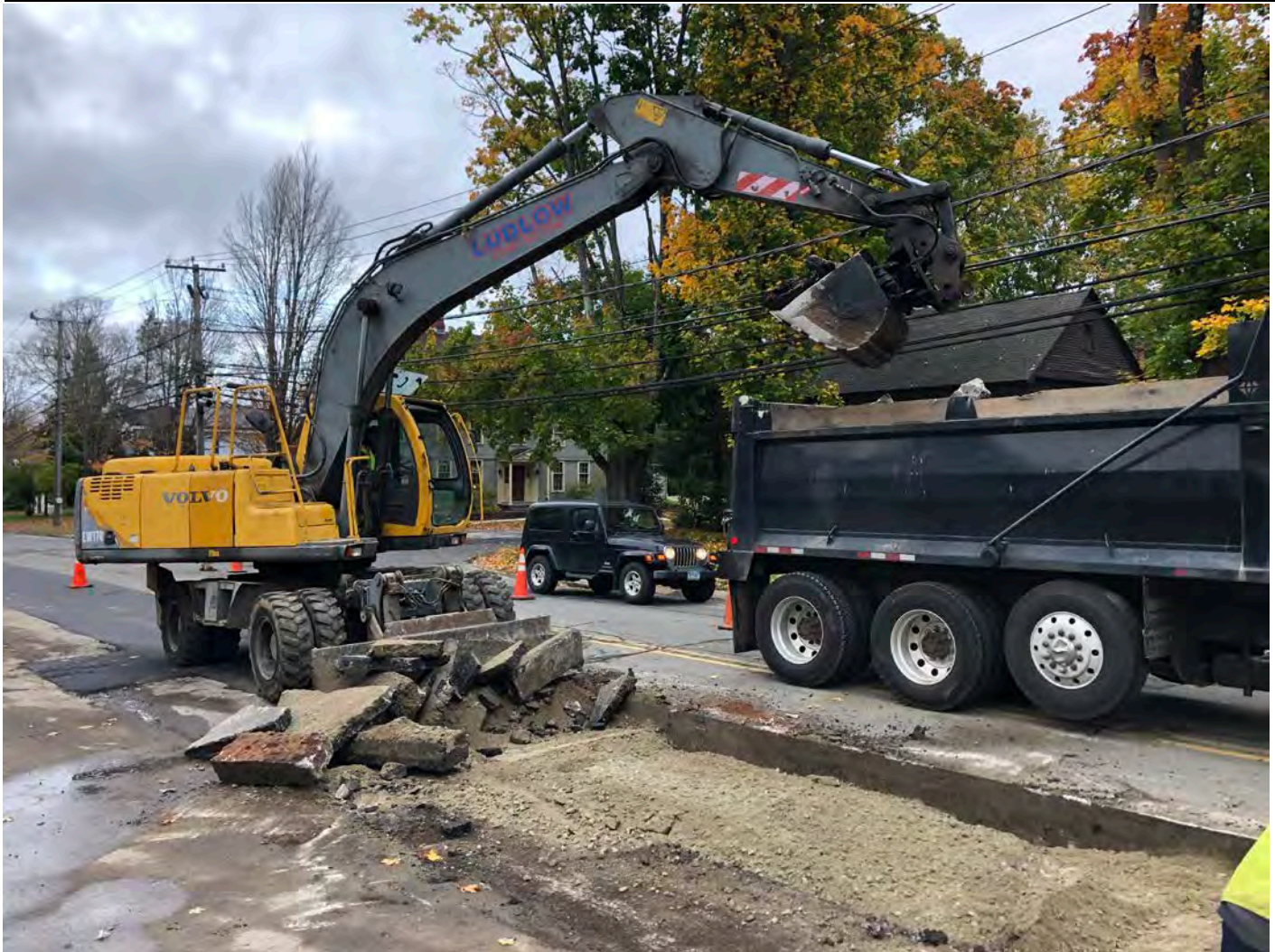
Picture 2: Ludlow stripping pavement away from trench overcuts between Stations 192+70 and 195+30 on the southbound lane of Main Street, Durham, as part of permanent paving activities. View to the northeast.
