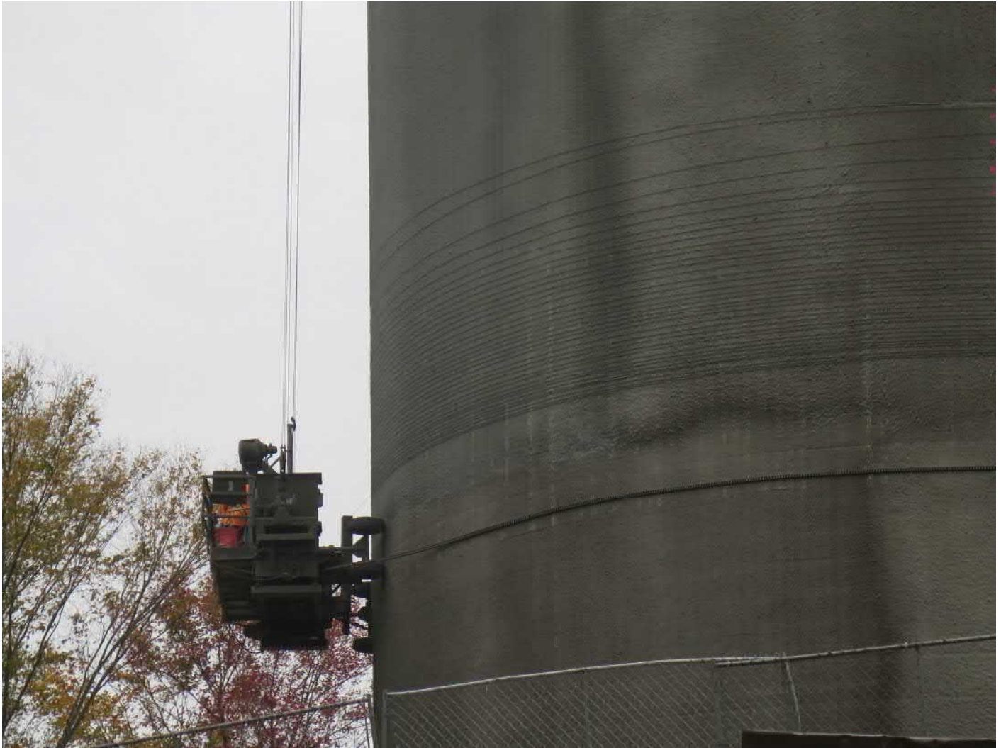
Picture 4: Close-up of wire application on tank wall. Water tank work zone located to the east of the Shared Access Driveway, Middletown. View to the east.
