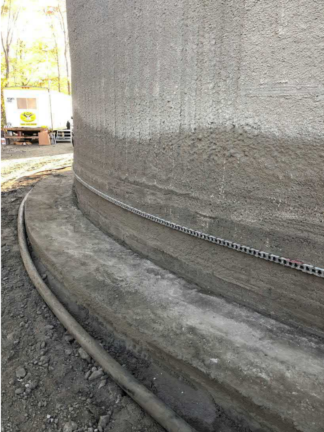
Picture 2: The base of the water tank after shotcrete was applied to it yesterday. Water tank work zone located east of the Shared Access Driveway, Middletown. View to the east.
