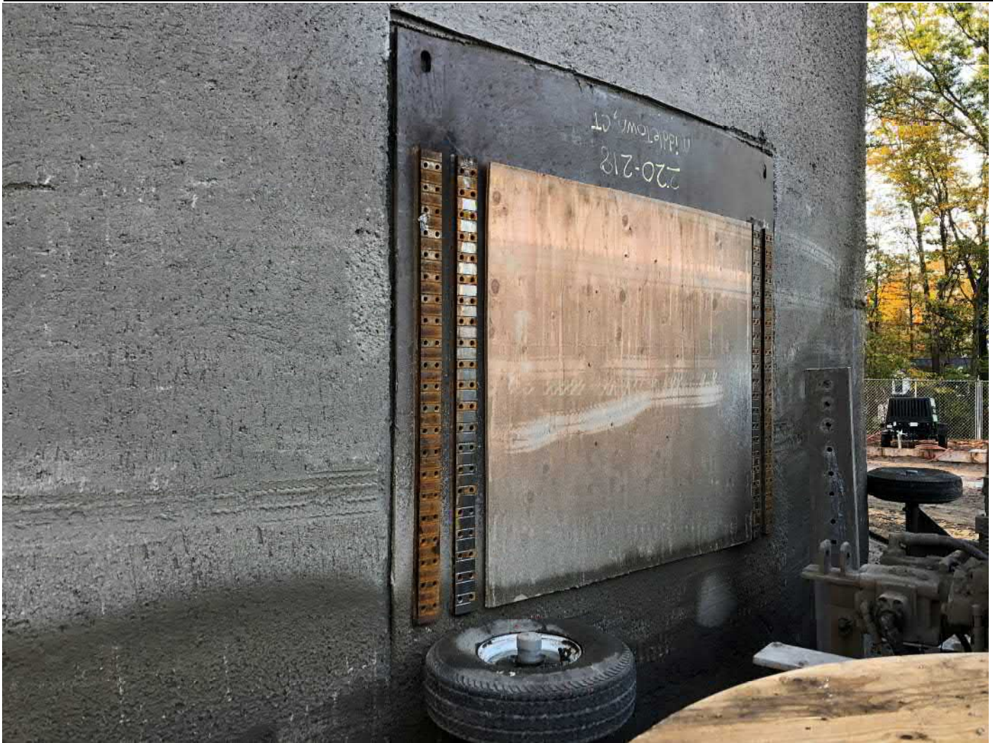
Picture 1: Stress plate that DN Tanks installed on the manways located on the west side of the water tank. Water tank work zone located east of the Shared Access Driveway, Middletown. View to the southeast.
