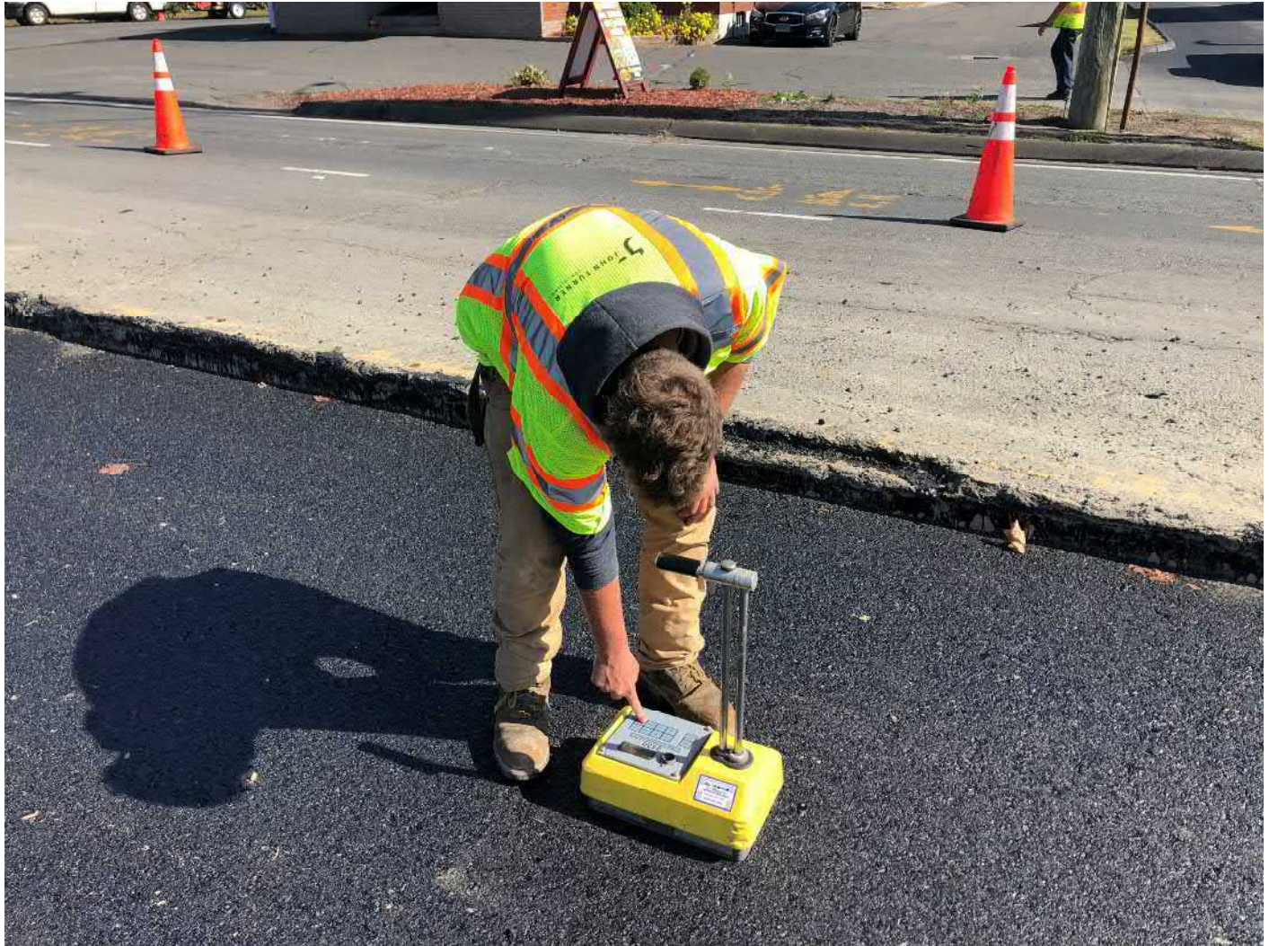
Picture 10: JTC collecting compaction data from the first 3" lift of asphalt as part of trench overcut paving activities on the southbound lane of Main Street, Durham, between Stations 167+30 and 171+00. View to the northeast.
