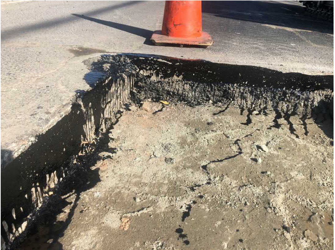
Picture 5: Tack coat that Ludlow has applied to the edge of cut pavement on the trench overcuts for permanent paving on the southbound lane of Main Street, Durham, between Stations 167+30 and 171+00.
