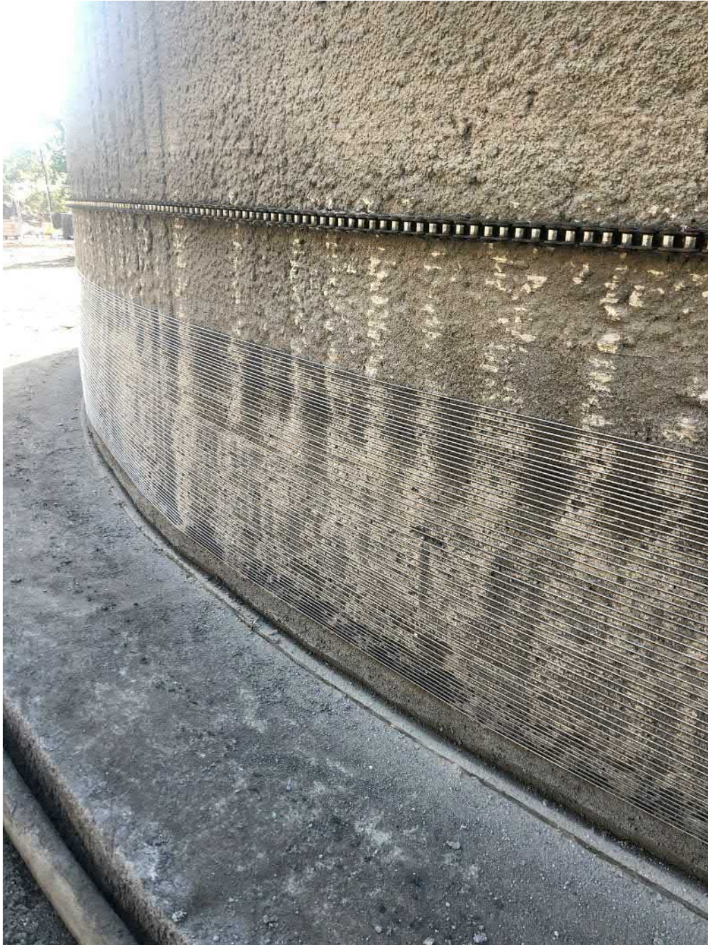
Picture 8: DN Tanks started to place a second layer of prestressed wire on the base of the water tank after shotcrete was applied to it yesterday. Water tank work zone located east of the Shared Access Driveway, Middletown. View to the east.
