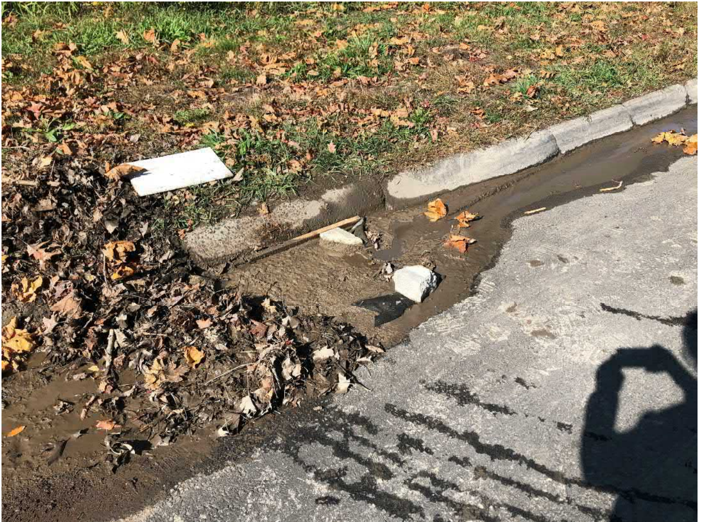
Picture 4: Silt fabric placed over the catch basin located at Station 206+20, which is located downgradient of pavement saw cutting activities. Main Street, Durham; view to the northwest.
