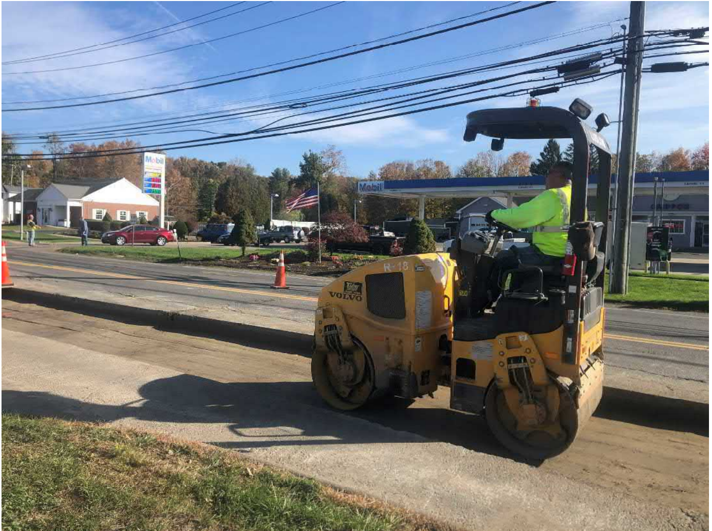
Picture 7: Ludlow compacting 1.5" processed gravel as part of trench overcut paving activities on the southbound lane of Main Street, Durham, between Stations 167+30 and 171+00.
