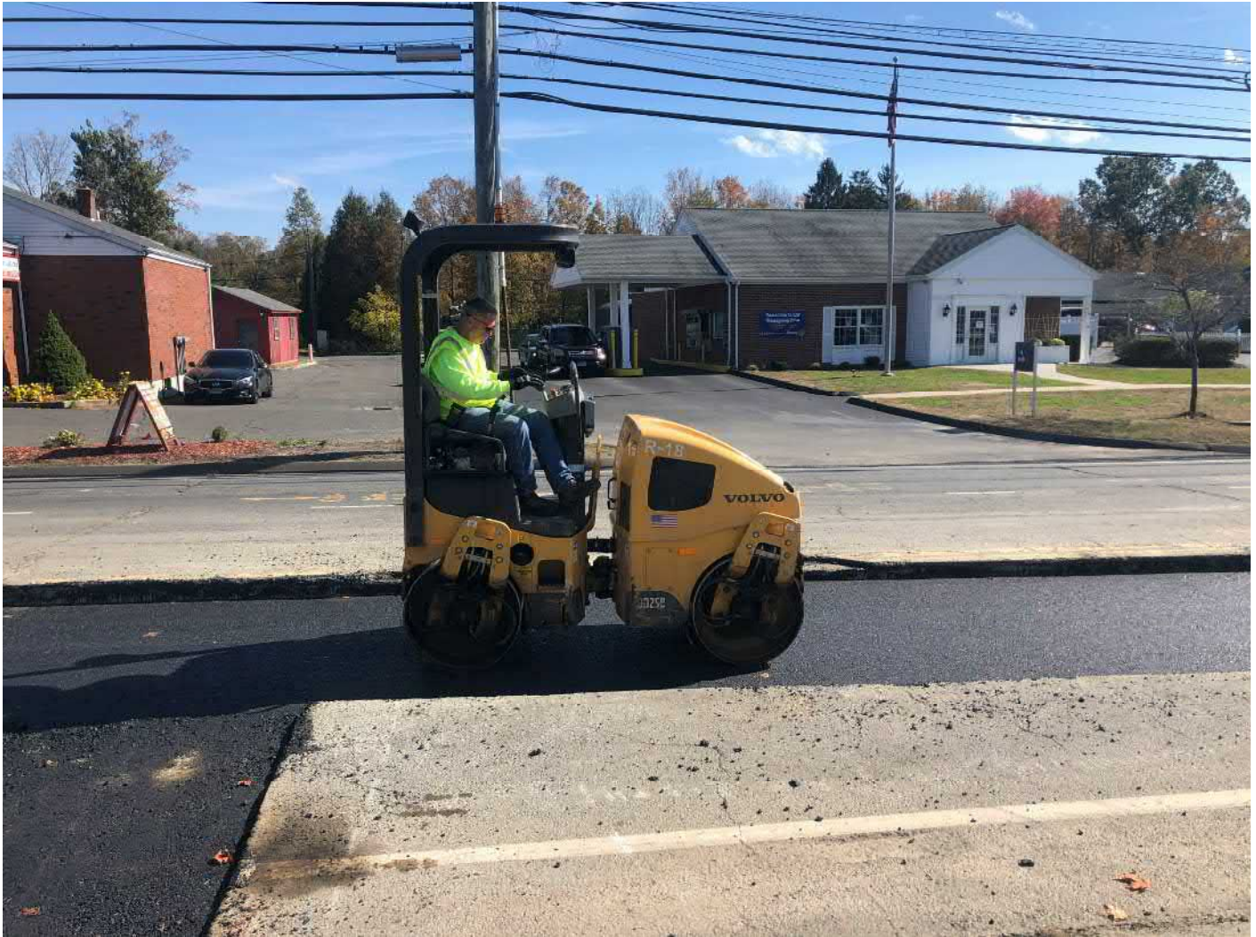
Picture 9: Ludlow compacting first 3" lift of asphalt as part of trench overcut paving activities on the southbound lane of Main Street, Durham, between Stations 167+30 and 171+00. View to the east.
