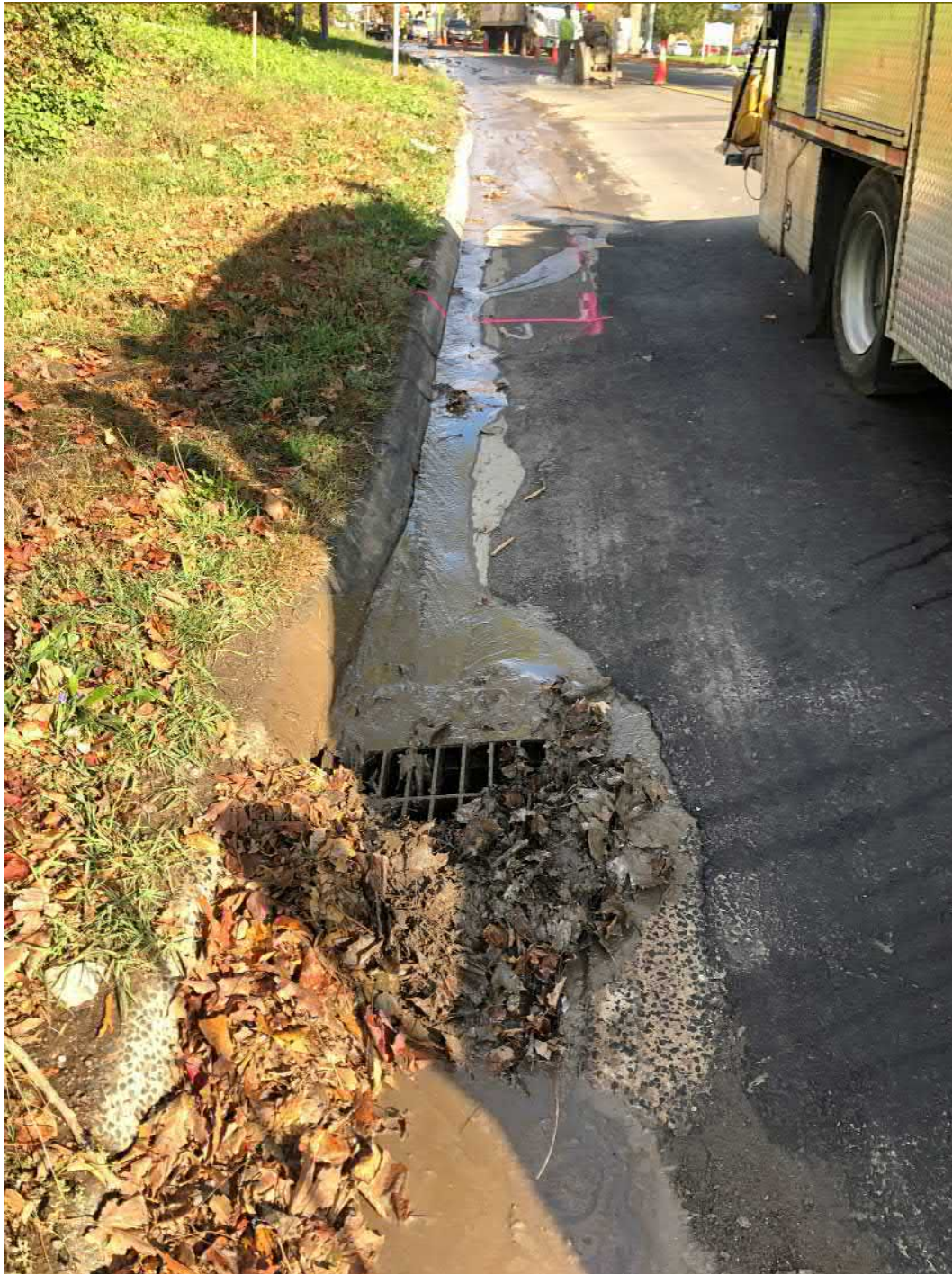
Picture 3: Water and silt from saw cutting operations on the southbound lane of Main Street, Durham entering the catch basin located at Station 206+20. View to the north.
