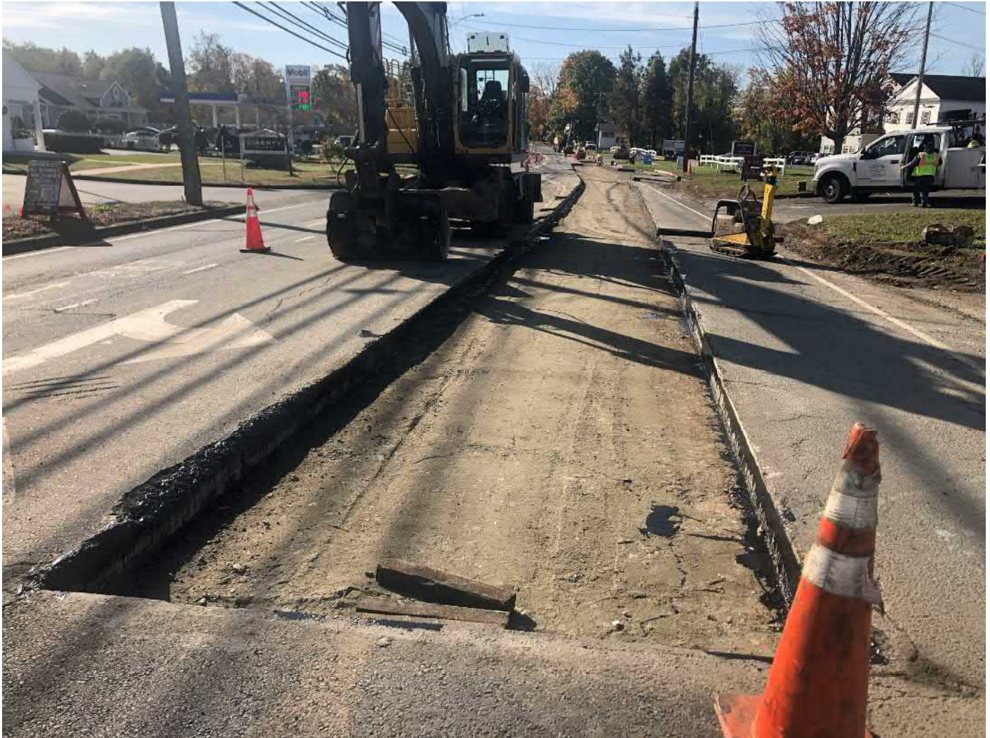
Picture 6: Asphalt stripped away from trench overcuts paving work zone located on the southbound lane of Main Street, Durham, between Stations 167+30 and 171+00.
