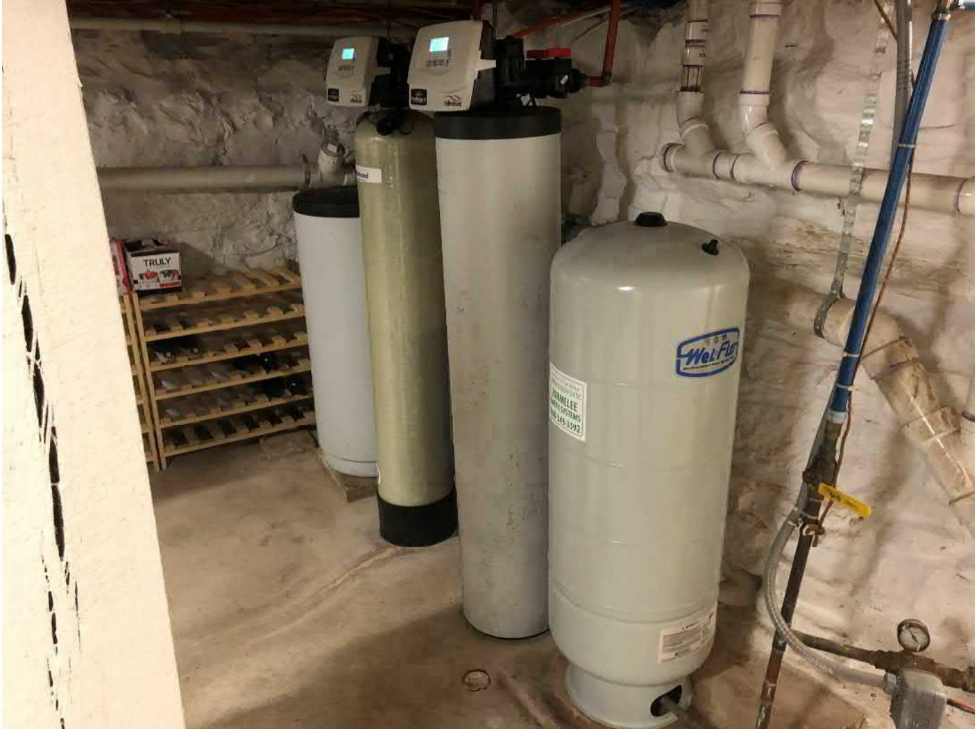
Picture 3: Water treatment system owned by the residents of 13 Maple Avenue, Durham. The water service brought into the house today by the Ludlow plumbing contractor was connected to this system at the request of the residents.
