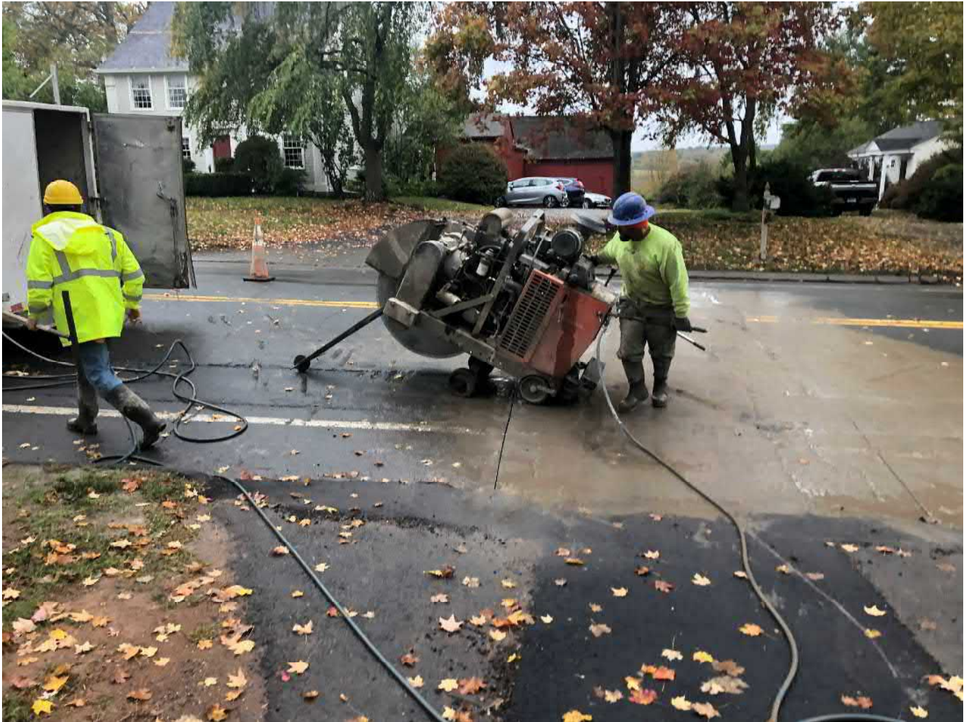
Picture 7: Veilleux saw cutting curb stop cutbacks on the northbound lane of Main Street. View to the southeast.
