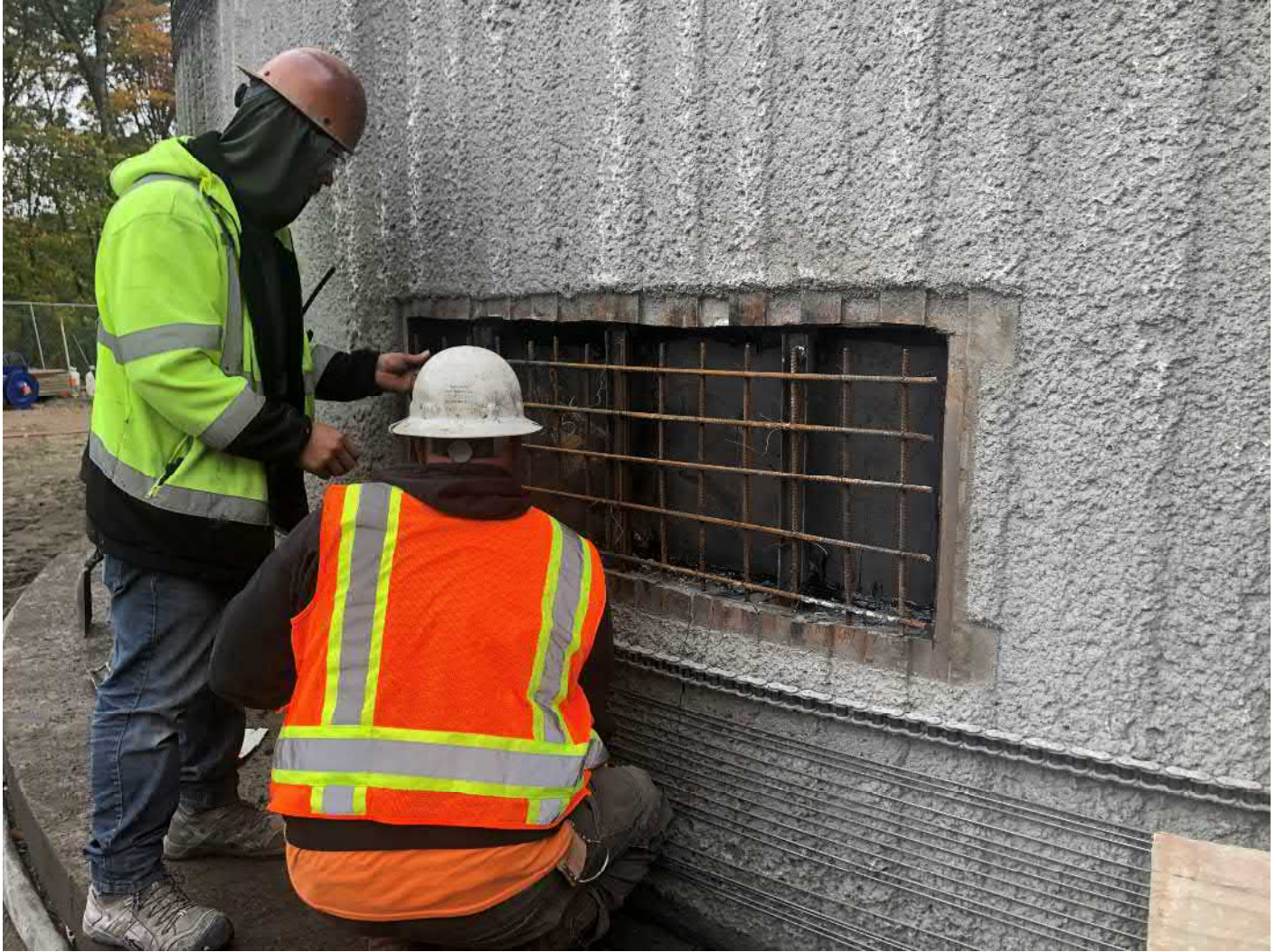
Picture 8: DN Tanks preparing to seal off a temporary entrance to the water tank. Water tank work zone located to the east of the Shared Access Driveway, Middletown.
