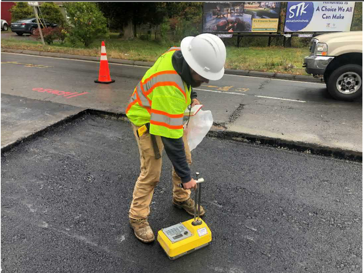
Picture 5: JTC collecting compaction data from permanent paving at trench cutbacks at Station 163+60 on the southbound lane of Main Street, Durham. View to the northeast.
