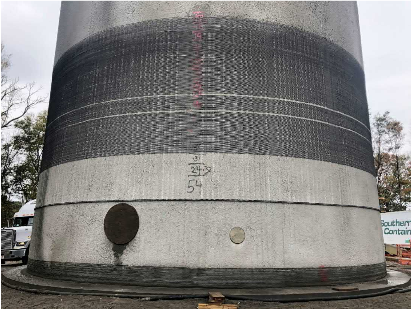
Picture 1: Prestressed wire that DN Tanks has wrapped around the exterior of the water tank located to the east of the Shared Access Driveway, Middletown. View to the east.
