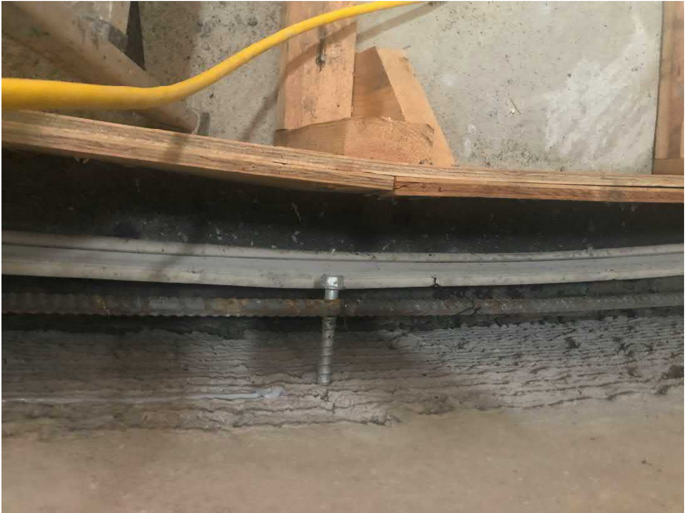
Picture 3: Concrete form for the C.I.P cove on the inside of the water tank with rebar set in place. Water tank work zone located to the east of the Shared Access Driveway, Middletown.
