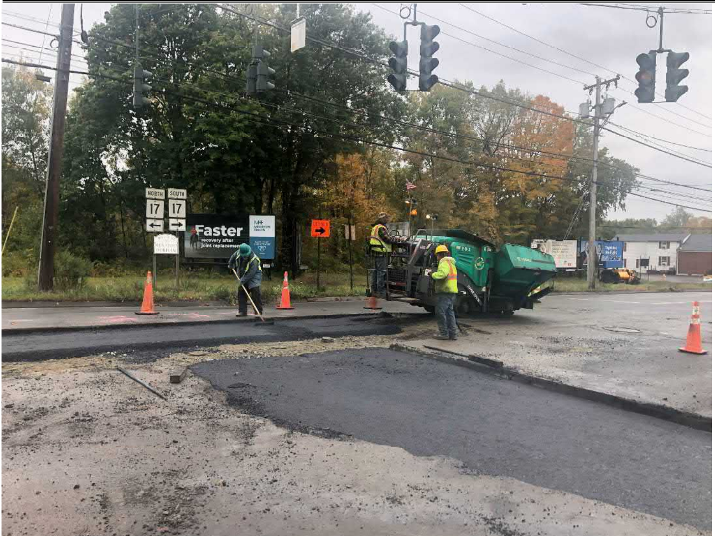
Picture 4: Intersection of Main Street and Route 147, where Ludlow is placing and compacting first lift of asphalt. This is the location where the USACE field engineer questioned Ludlow regarding the thickness of placed asphalt. View to the southeast.
