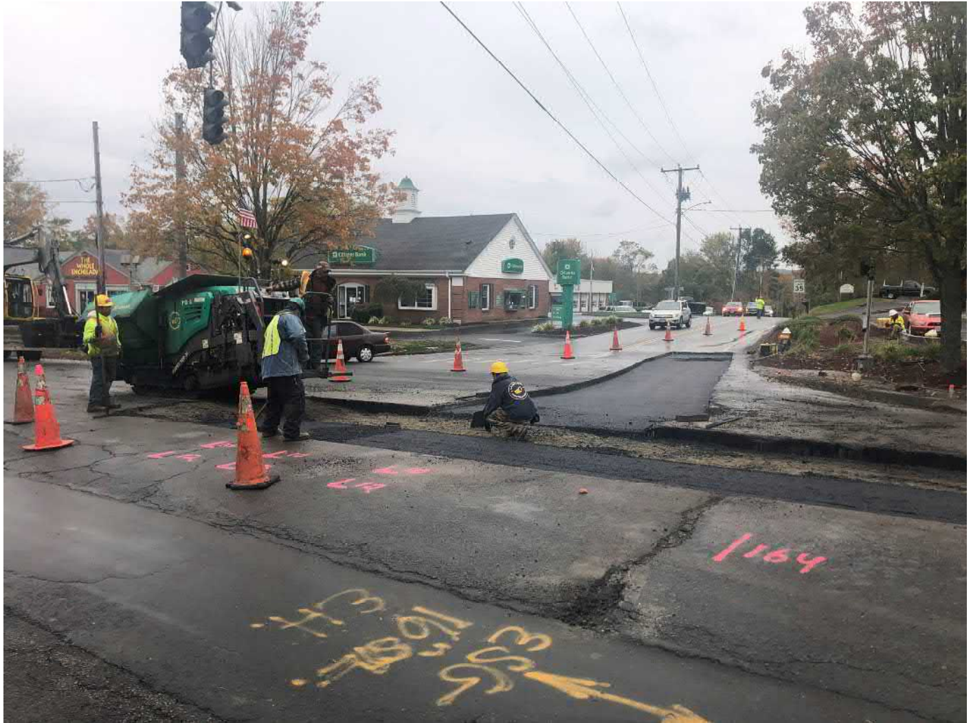
Picture 6: Overview of Route 147 permanent paving on trench cutbacks. View to the southwest.
