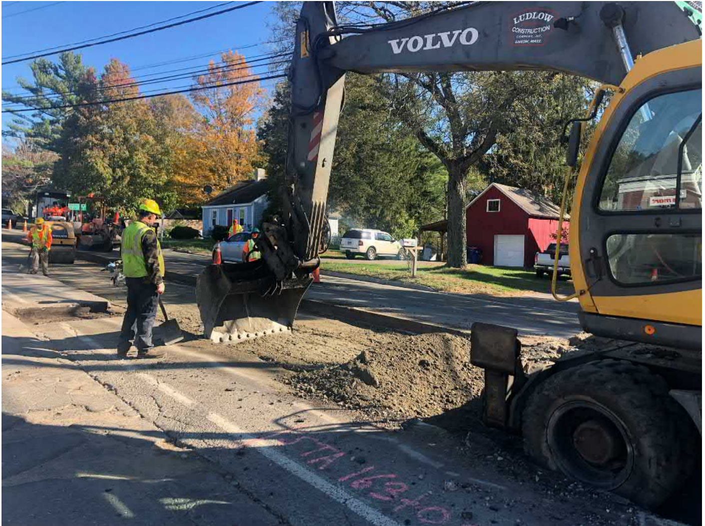
Picture 2: Ludlow grading and compacting 1.5" processed gravel between Stations 160+25 to 163+55 as they prepare to place permanent paving on the southbound lane of Main Street, Durham. View to the northeast.
