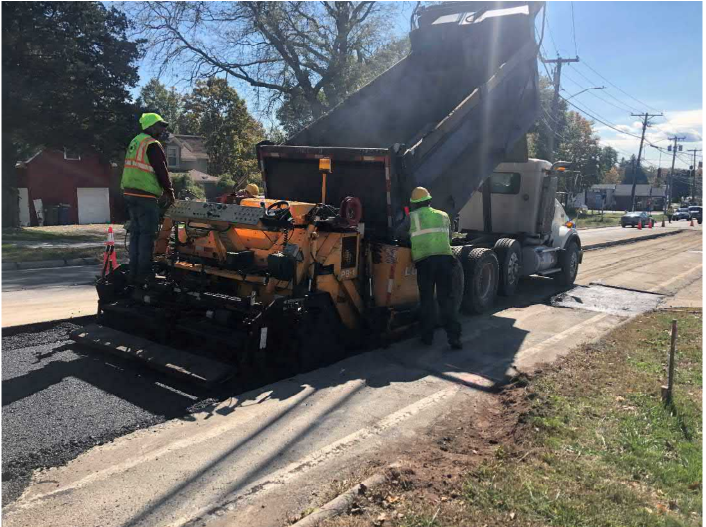
Picture 7: Ludlow placing and compacting the first of three 3" lifts of asphalt between Stations 160+25 to 163+55 as they prepare to place permanent paving on the southbound lane of Main Street, Durham. View to the southeast.
