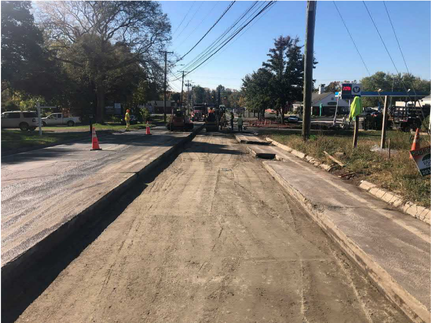
Picture 4: Ludlow stripping back asphalt as they prepare to place permanent paving between Stations 160+25 to 163+55 the southbound lane of Main Street, Durham. View to the south.
