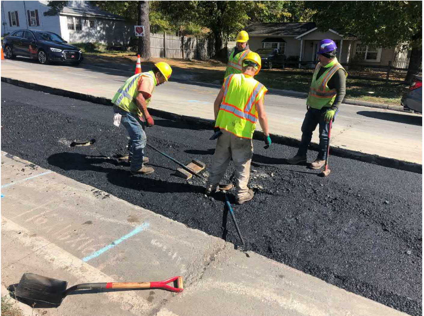
Picture 6: Ludlow raising a road box during permanent paving at trench cutbacks between Stations 157+25 and 160+25 on the southbound lane of Main Street, Durham. View to the east.
