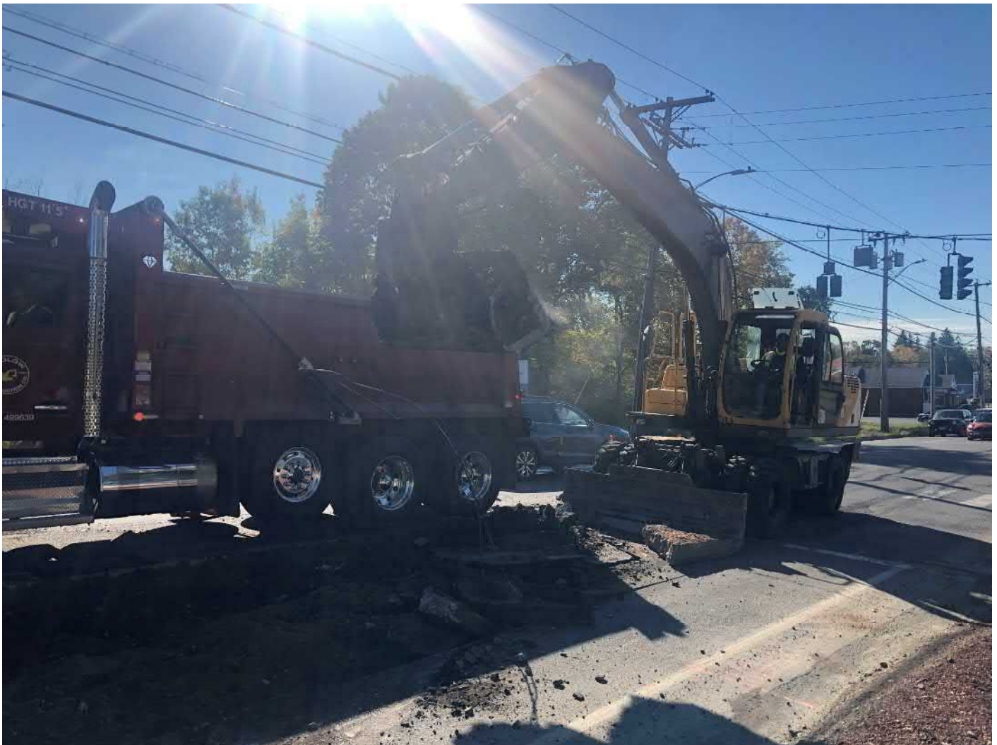
Picture 1: Ludlow stripping back asphalt as they prepare to place permanent paving between Stations 160+25 to 163+55 the southbound lane of Main Street, Durham. View to the southeast.
