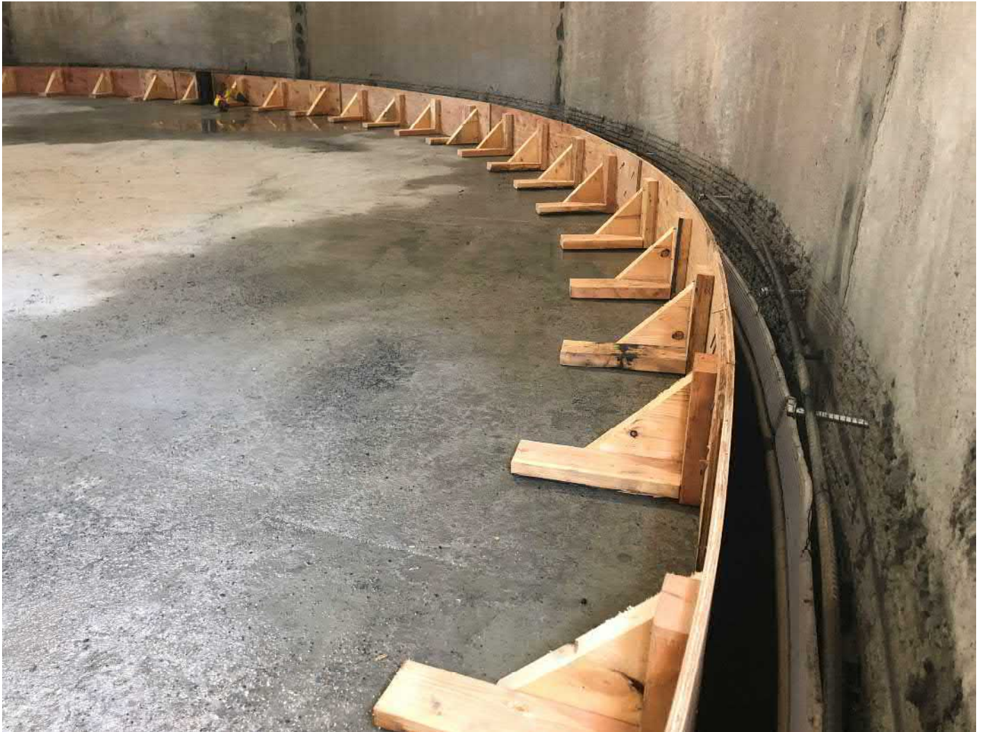
Picture 8: Concrete form for the C.I.P. cove on the inside of the water tank. Water tank work zone located to the east of the Shared Access Driveway, Middletown.
