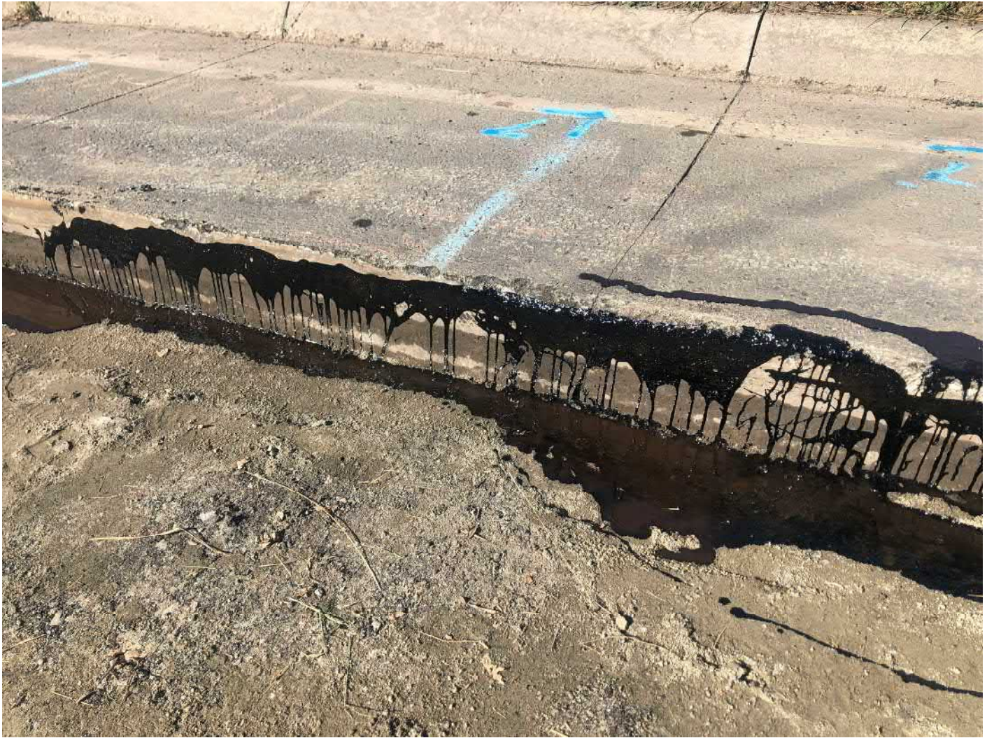
Picture 3: Tack coat that Ludlow has placed on the edges of cut pavement between Stations 160+25 to 163+55 as they prepare to place permanent paving on the southbound lane of Main Street, Durham. View to the west.
