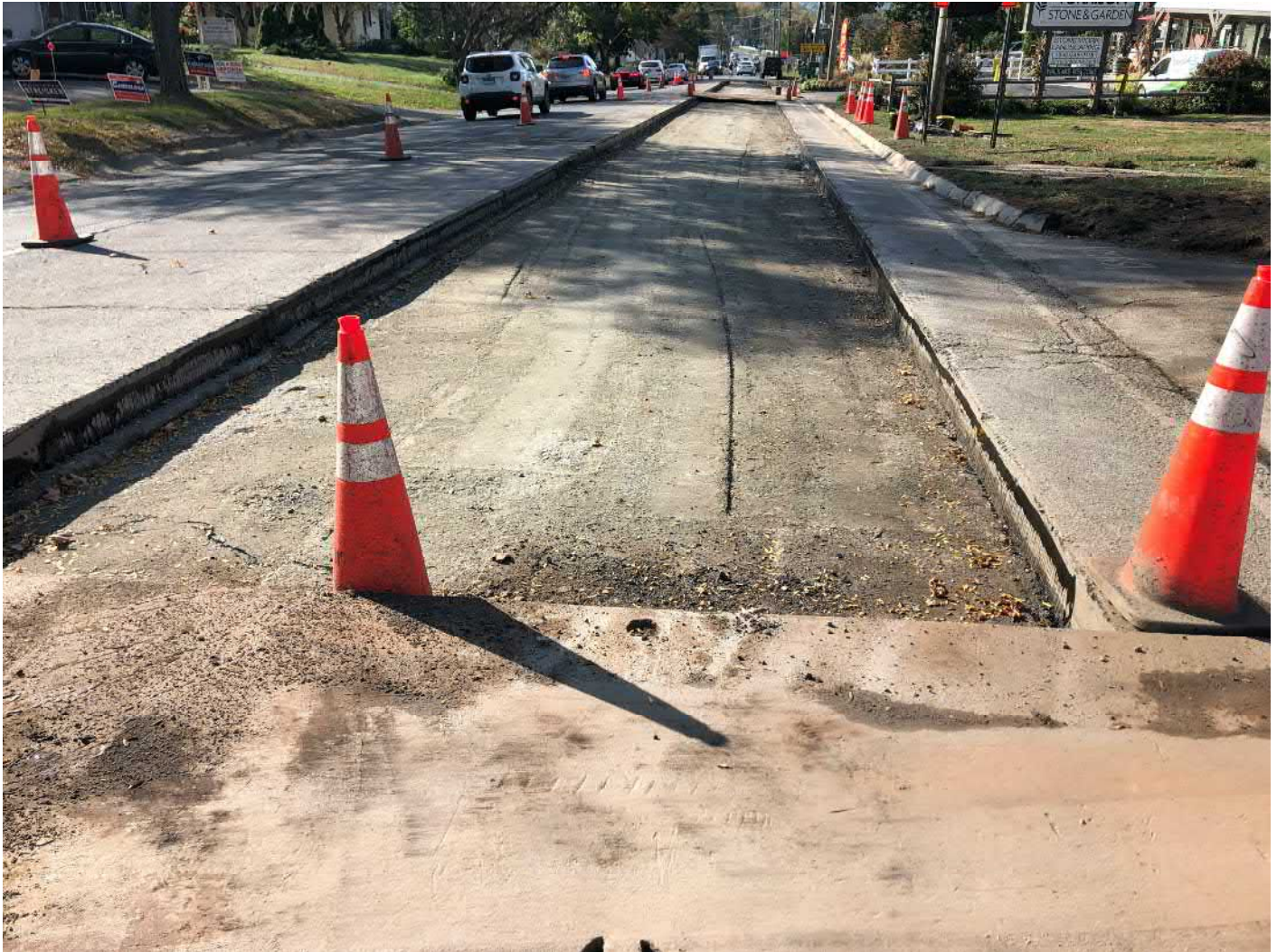
Picture 5: Ludlow has asphalt removed from trench cutback work zone and has compacted 1.5” processed gravel as they prepare to place permanent paving on the southbound lane of Main Street, Durham. View to the southeast.
