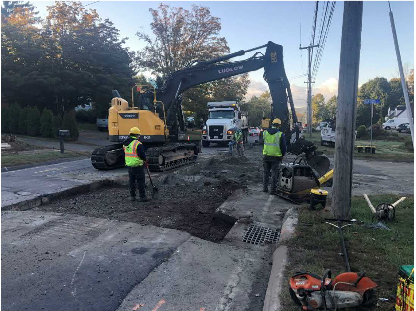
Picture 2: Ludlow stripping back asphalt as they prepare to place permanent paving on the southbound lane of Main Street, Durham from Stations 151+35 to 154+25. View to the south.
