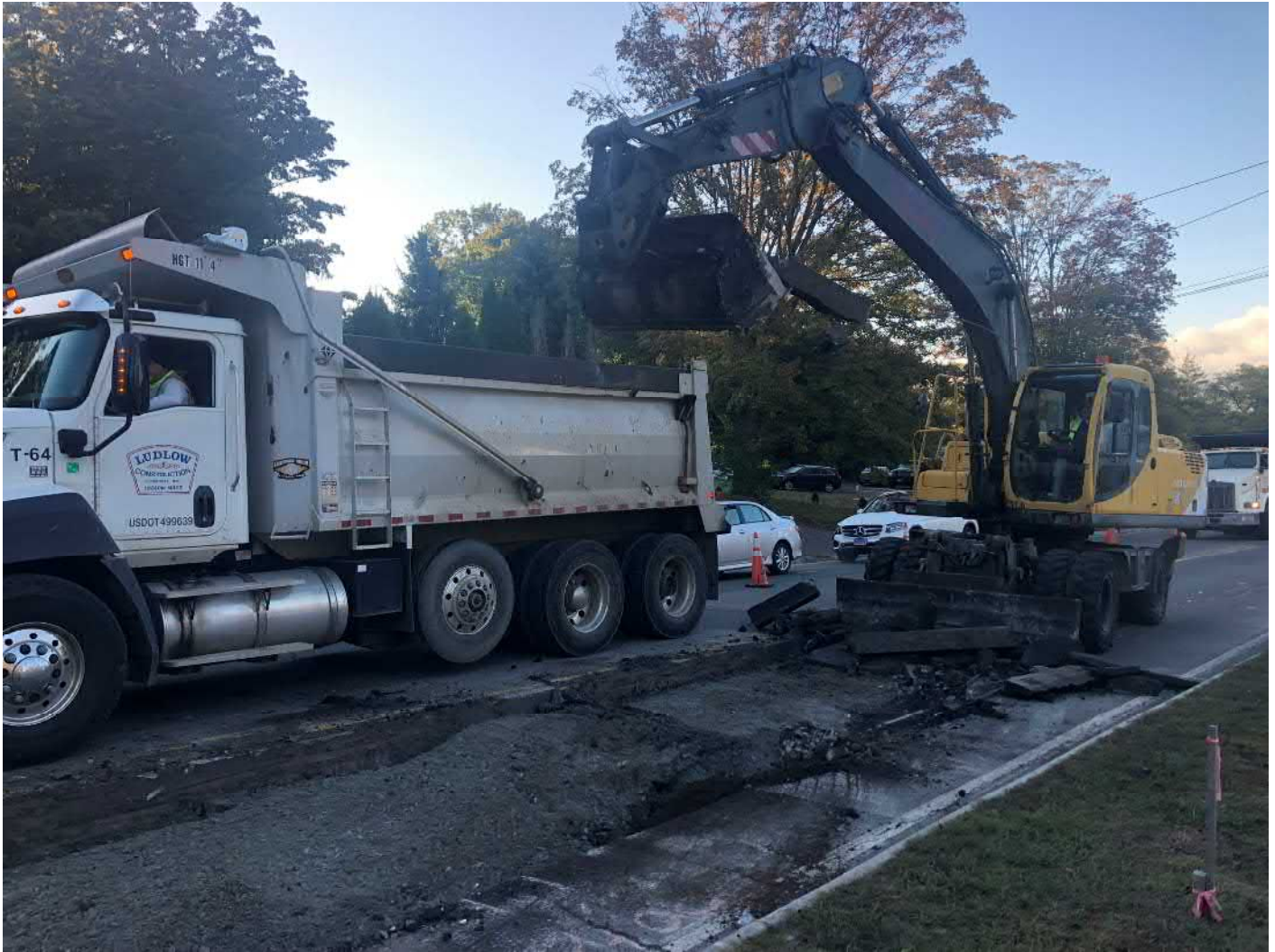
Picture 4: Ludlow loading asphalt and concrete into a dump truck as they strip back asphalt for permanent paving on the southbound lane of Main Street, Durham from Stations 151+35 to 154+25. View to the southeast.
