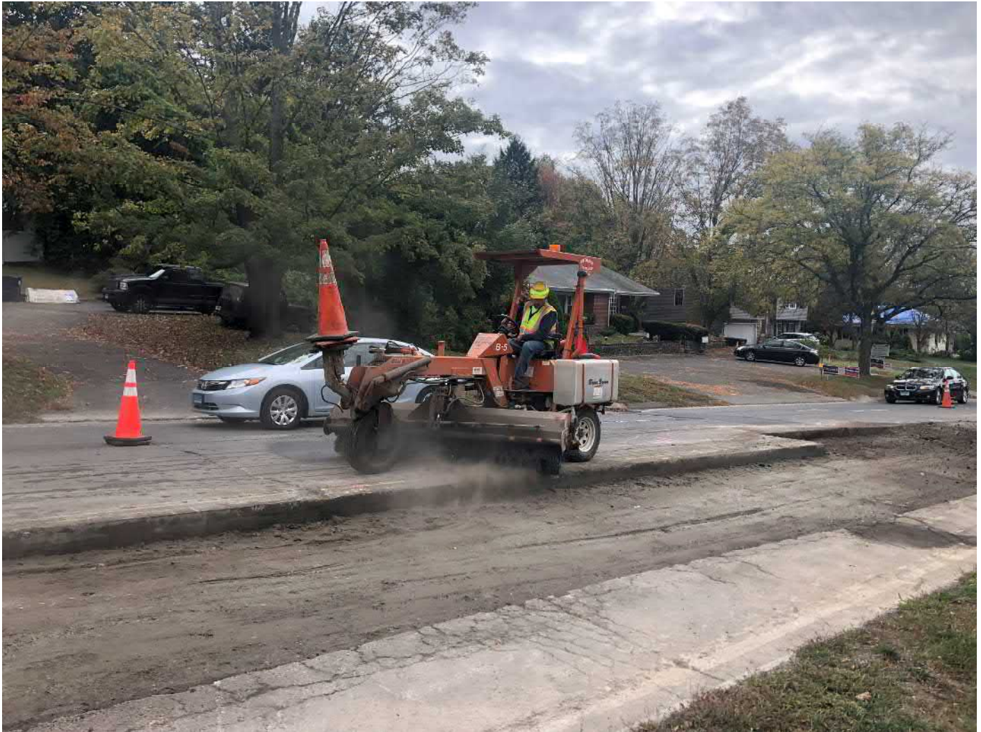
Picture 7: Ludlow cleaning work zone with the Broce Broom between Stations 151+35 to 154+25 as they prepare to place permanent paving on the southbound lane of Main Street, Durham. View to the southeast.
