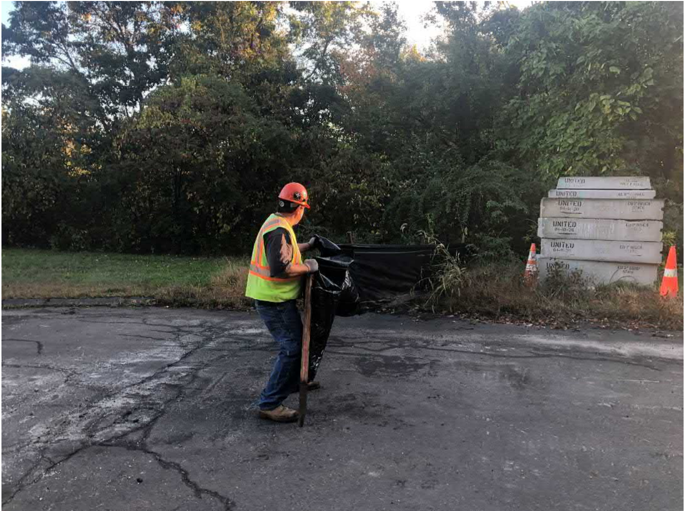
Picture 1: Ludlow removing silt fence from the Talcott Ridge Drive cul-de-sac and down along the Shared Access Driveway. View to the north.
