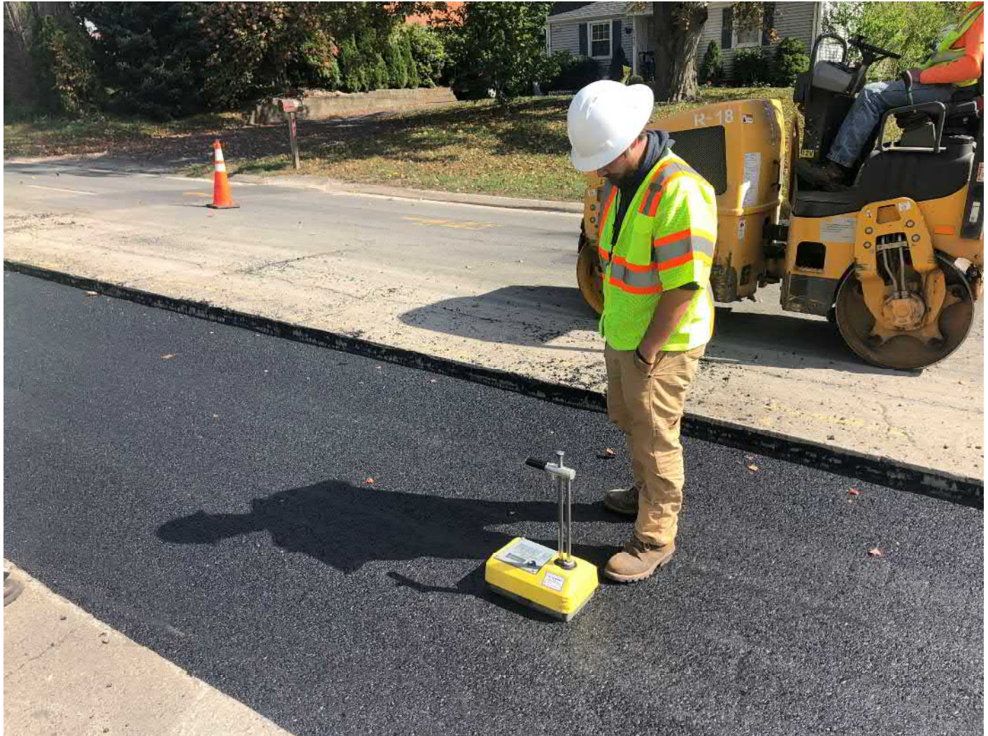
Picture 8: JTC is collecting compaction data from freshly placed and rolled asphalt between Stations 151+35 to 154+25 on the southbound lane of Main Street, Durham. View to the northeast.
