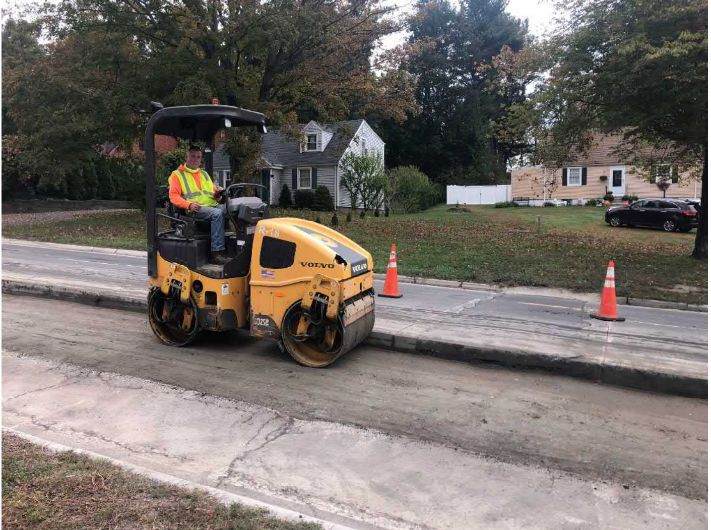
Picture 6: Ludlow is compacting 1.5" processed gravel as they prepare to place permanent paving on the southbound lane of Main Street, Durham from Stations 151+35 to 154+25. View to the east.
