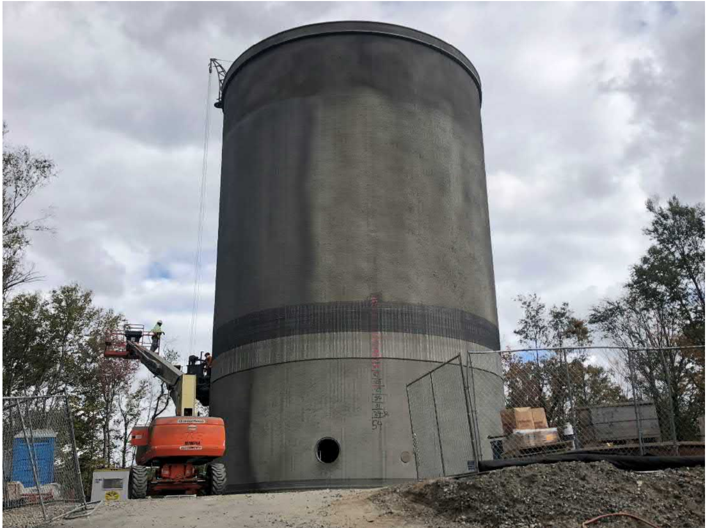
Picture 10: DN Tanks wrapping prestressed wire around the sides of the water tank. Water tank work zone located to the east of the Shared Access Driveway, Middletown. View to the east.
