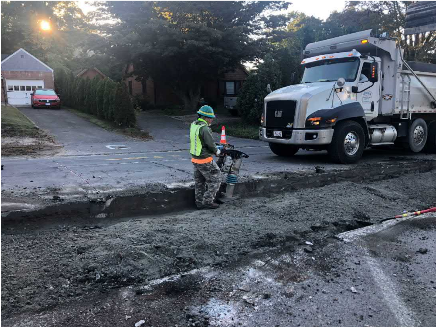
Picture 3: Ludlow using a Jumping Jack to compact 1.5" processed gravel along the edge of cut pavement as they prepare to place permanent paving on the southbound lane of Main Street, Durham from Stations 151+35 to 154+25. View to the southeast.
