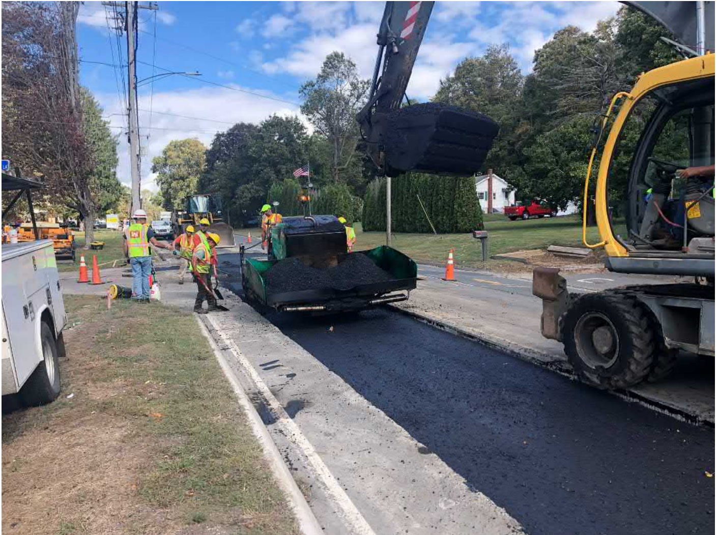
Picture 9: Ludlow placing the second of three 3" lifts of asphalt as part of permanent paving activities on the southbound lane of Main Street, Durham from Stations 151+35 to 154+25. View to the north.
