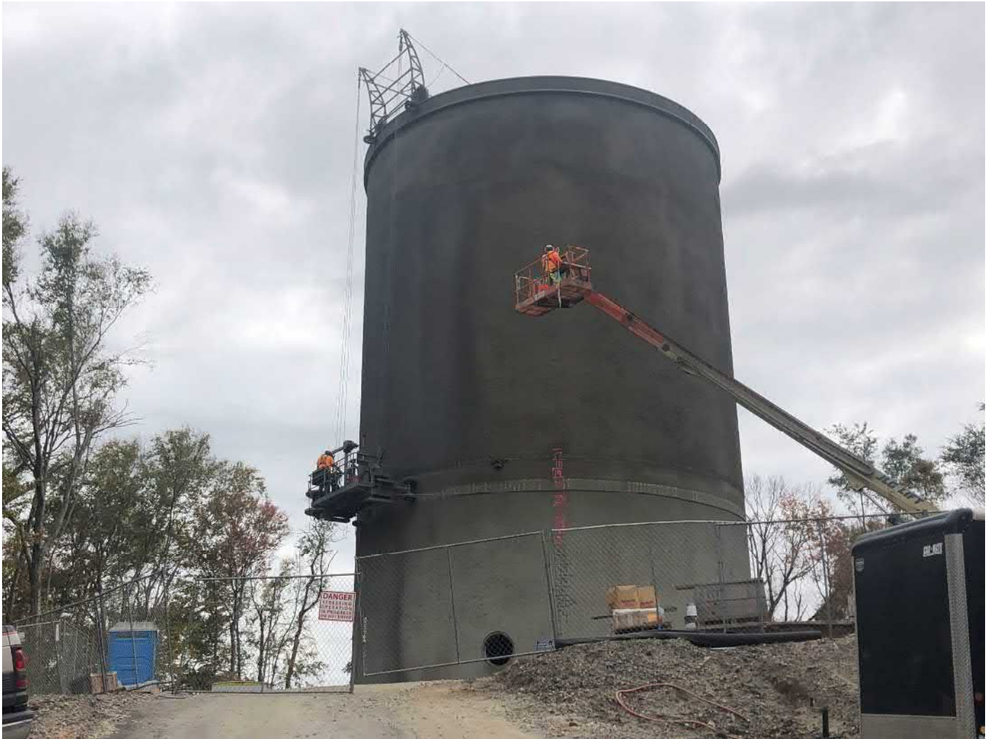
Picture 5: DN Tanks wrapping prestressed wire around the sides of the water tank. Water tank work zone located to the east of the Shared Access Driveway, Middletown. View to the east.
