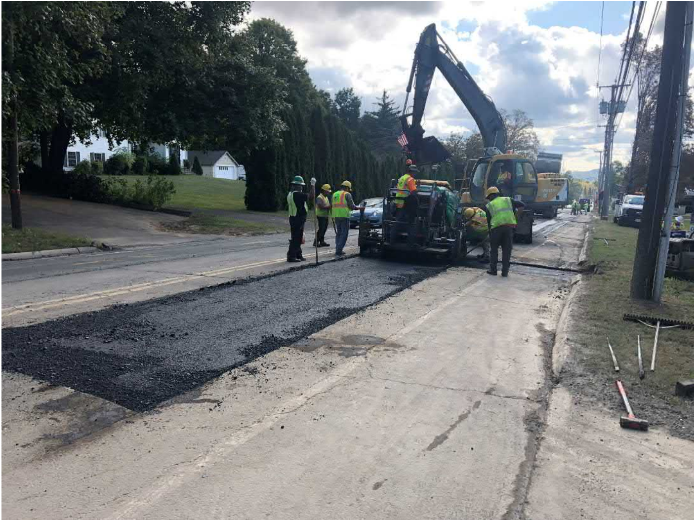
Picture 9: Ludlow placing the second of three 3" lifts of asphalt as part of permanent paving activities on the southbound lane of Main Street, Durham from Stations 148+65to 151+35. View to the southeast.
