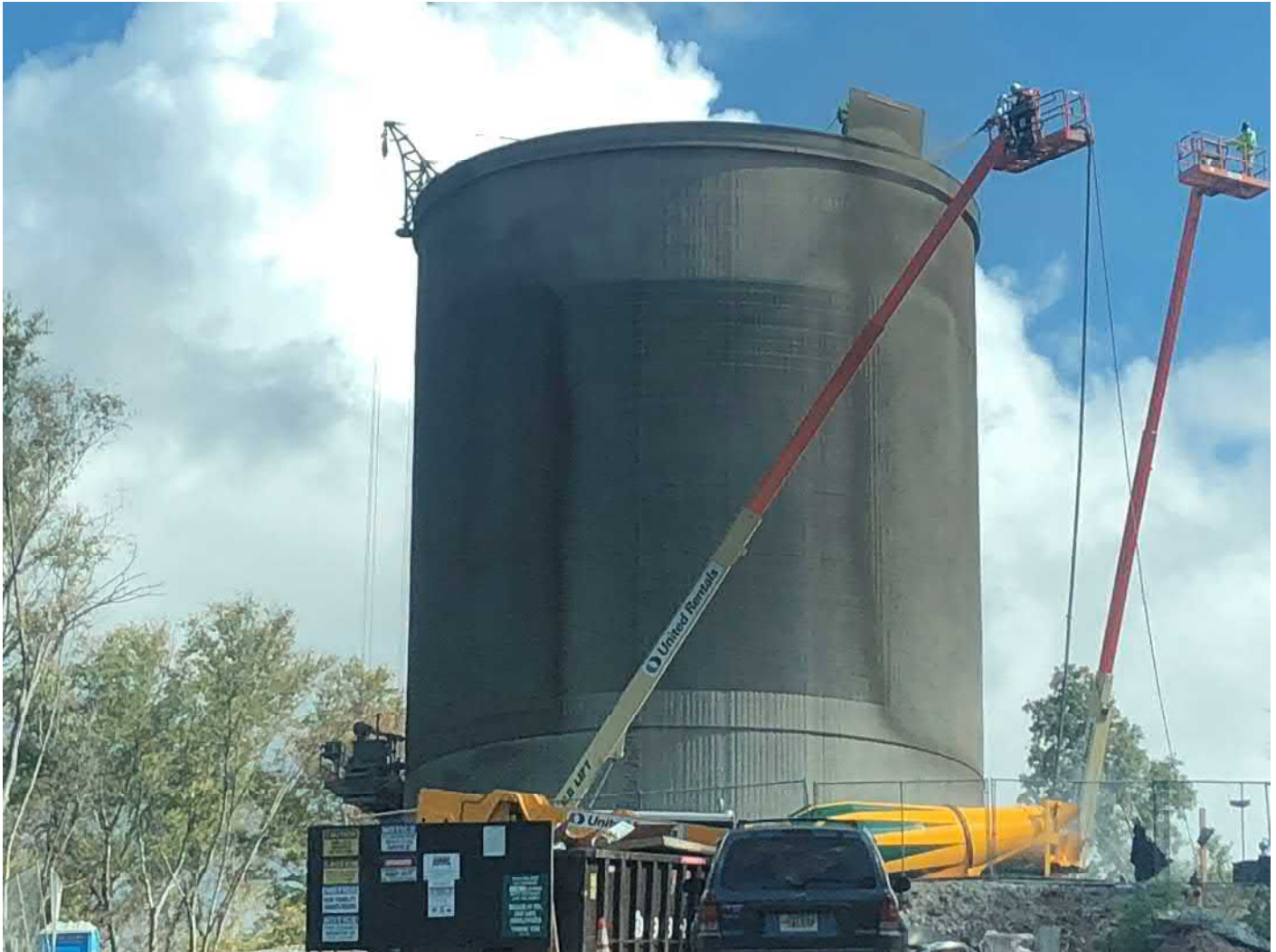
Picture 8: DN Tanks applying shotcrete to the dome rim of the water tank. Water tank work zone located to the east of the Shared Access Driveway, Middletown. View to the east.
