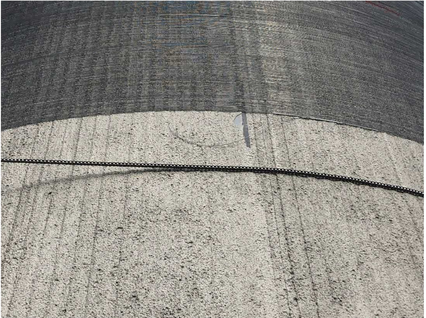
Picture 4: One of the two spots on the steel diaphragm where shotcrete has chipped away, revealing bare metal. DN Tanks later applied fresh shotcrete to these two areas. Water tank work zone, east of the Shared Access Driveway, Middletown. View to the north.
