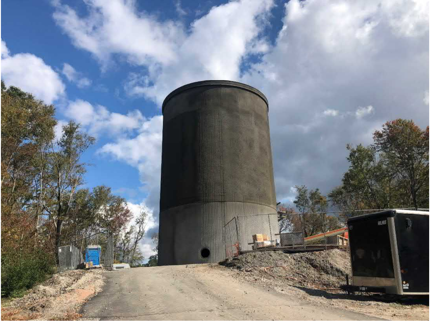
Picture 11: Overview of the water tank after DN Tanks applied shotcrete today. Water tank work zone located to the east of the Shared Access Driveway, Middletown. View to the east.
