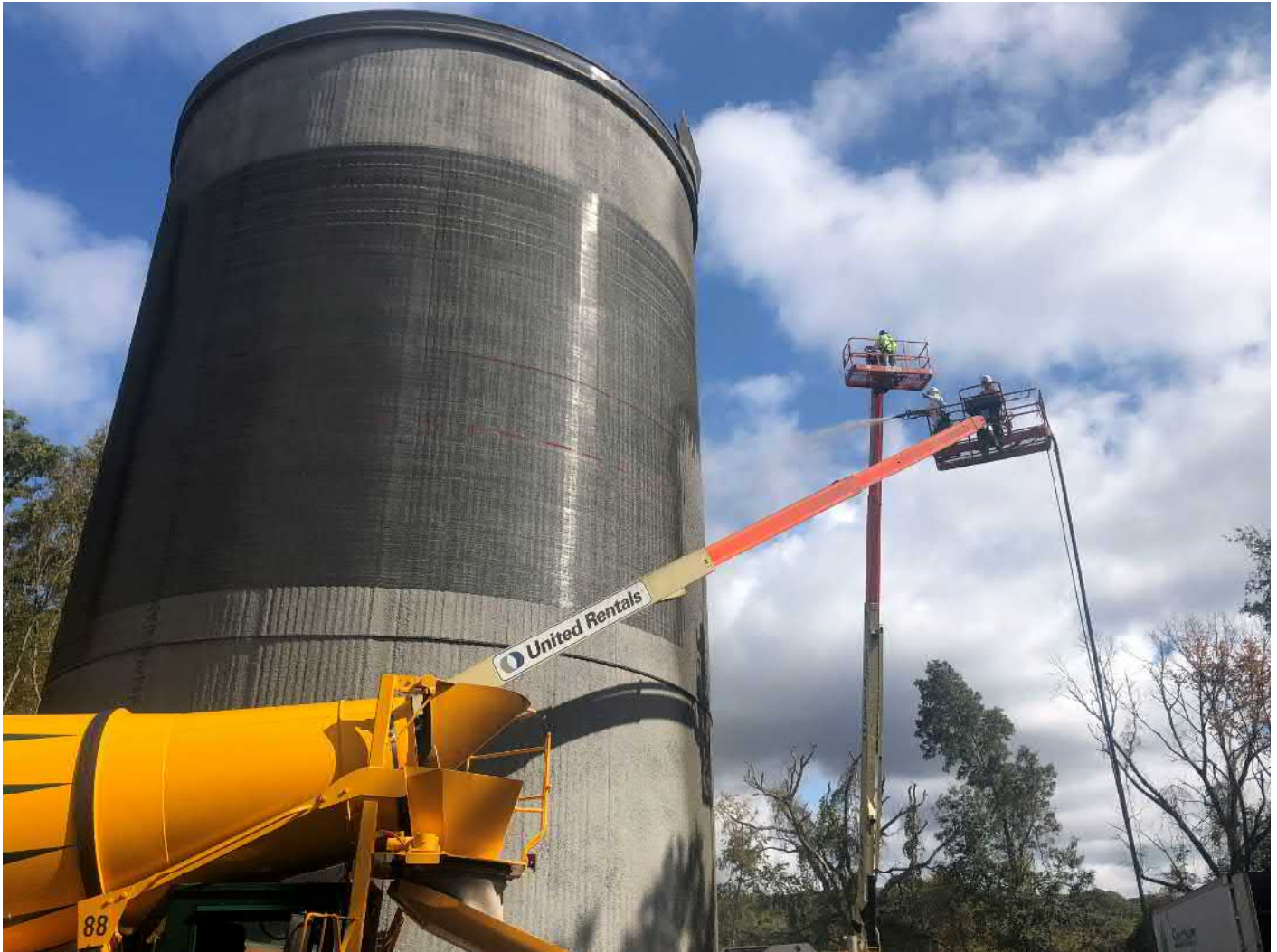
Picture 7: DN Tanks applying shotcrete to the side of the water tank. Water tank work zone located to the east of the Shared Access Driveway, Middletown. View to the east.
