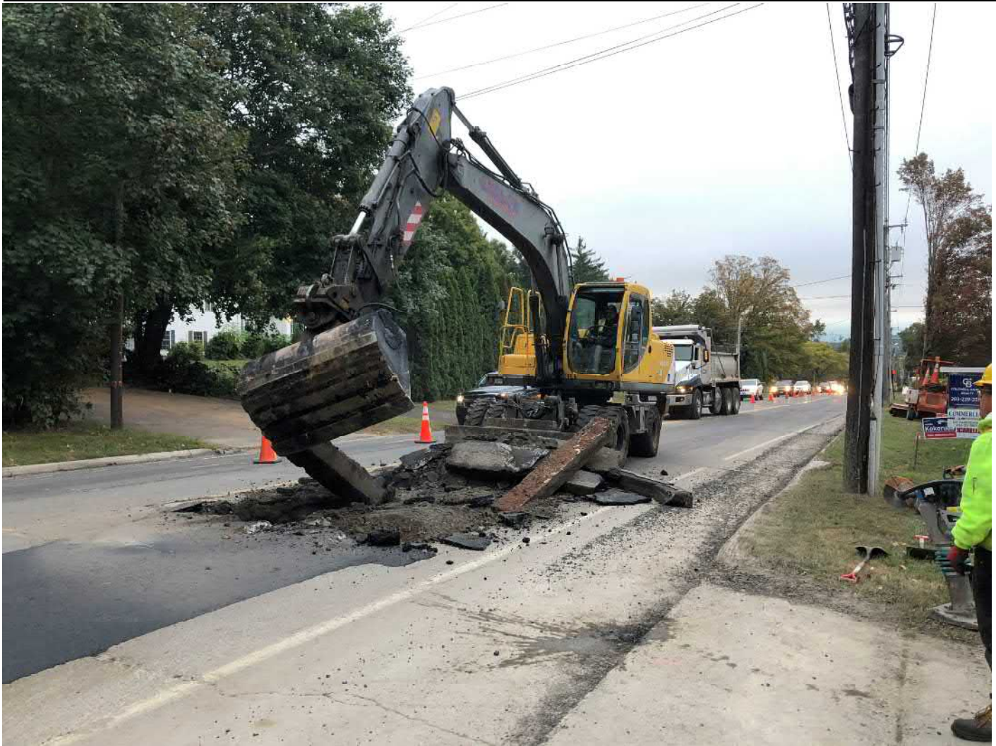
Picture 2: Ludlow stripping back asphalt as they prepare to place permanent paving on the southbound lane of Main Street, Durham from Stations 148+65 to 151+35. View to the southeast.
