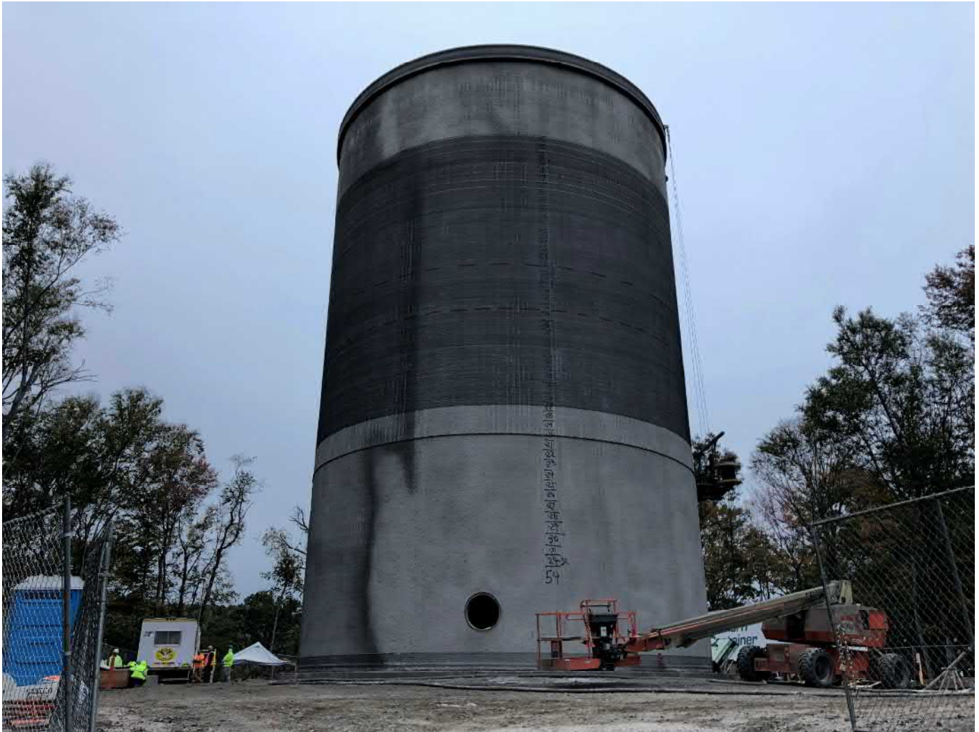
Picture 1: Water tank and the prestressed wire that has been wrapped around the sides of the tank. This is the tank before shotcrete was applied over the wire today. Water tank work zone, east of the Shared Access Driveway, Middletown. View to the east.
