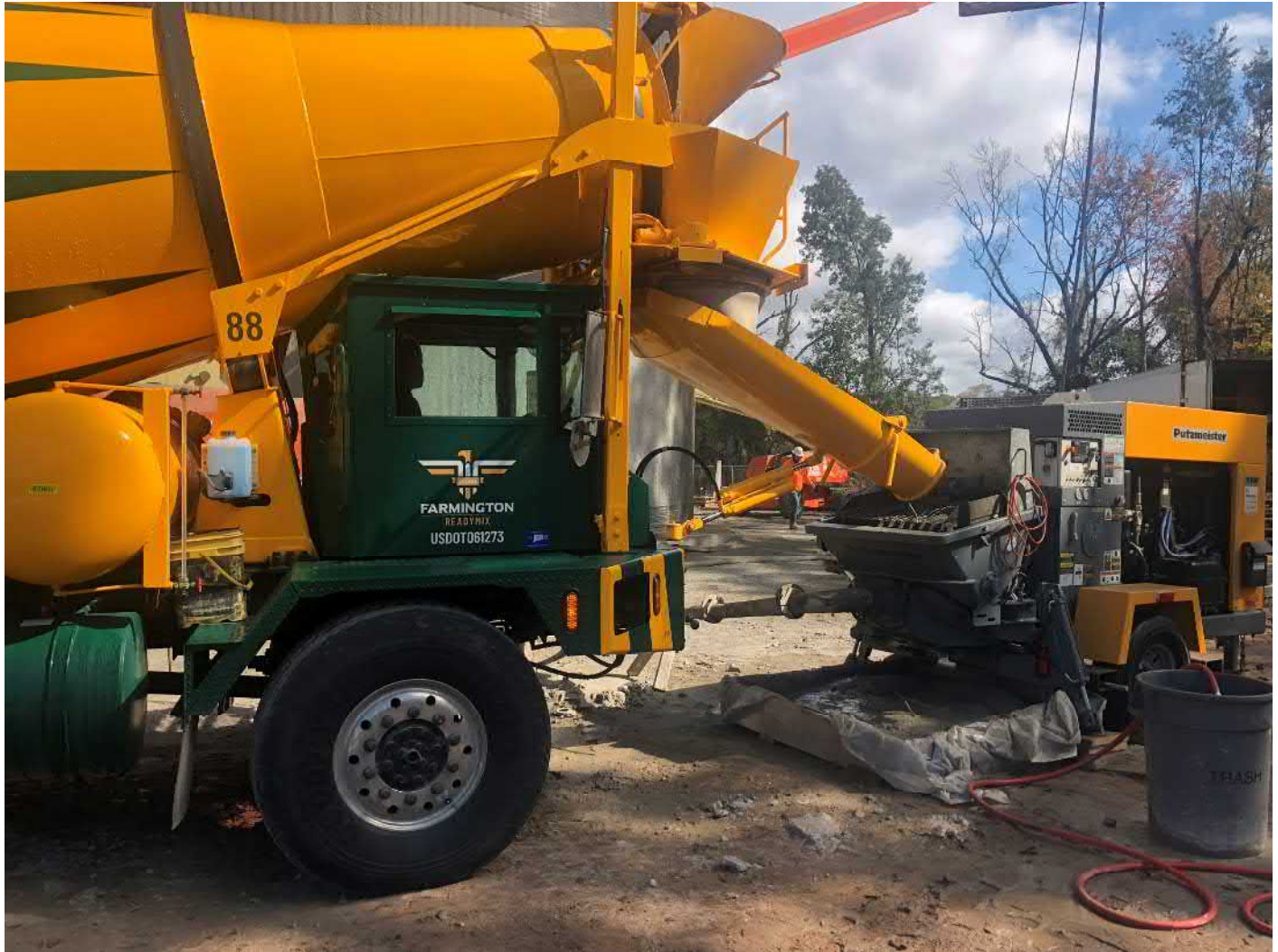
Picture 6: The third of three trucks of shotcrete about to start transferring shotcrete into pumper/mixer. Water tank work zone located to the east of the Shared Access Driveway, Middletown. View to the east.
