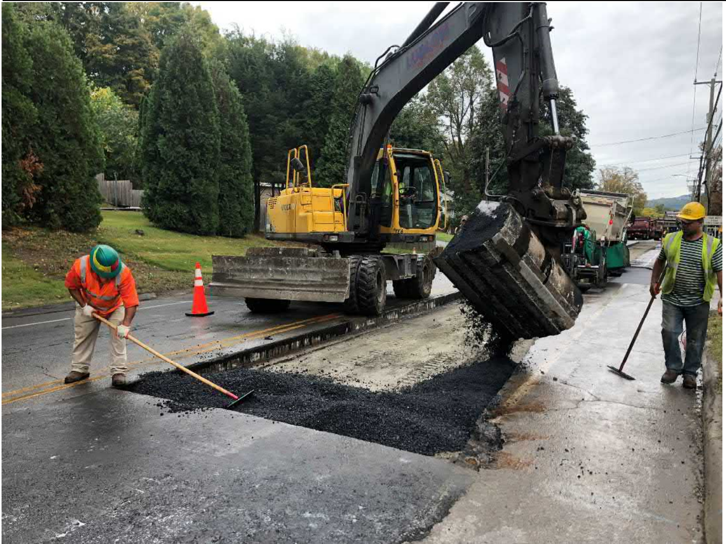
Picture 4: Ludlow placing first of three 3” lifts of asphalt on the southbound lane of Main Street, Durham from Stations 143+00 to 146+30. View to the southeast.
