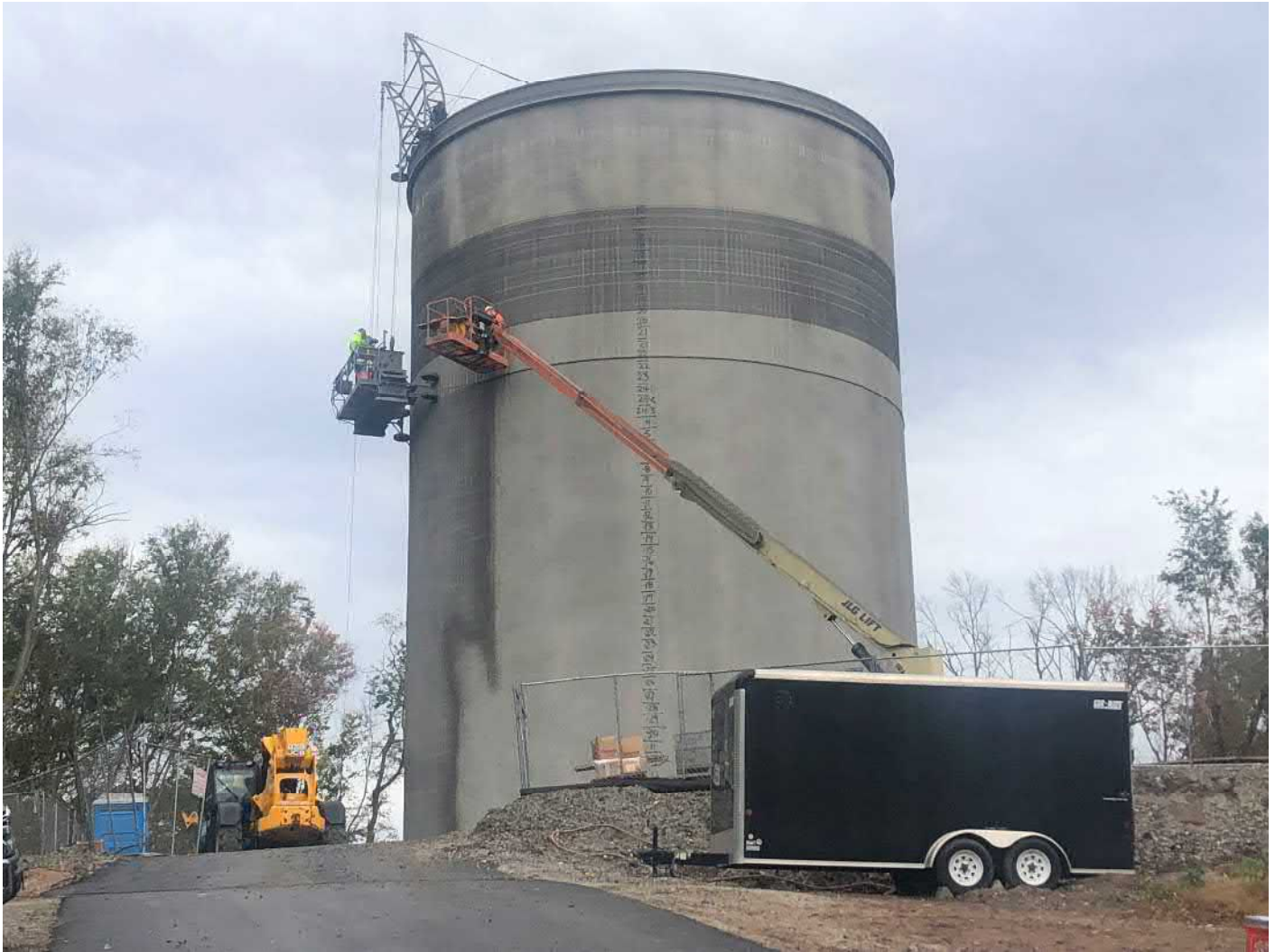
Picture 5: DN Tanks wrapping prestressed wire around the sides of the water tank from 47.5' to 58'. Water tank work zone, east of the Shared Access Driveway, Middletown. View to the northeast.
