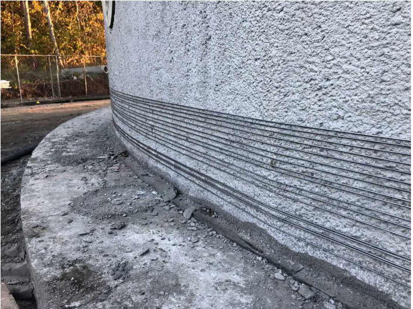
Picture 1: DN Tanks has wrapped prestressed wire around the sides of the water tank at the bottom. Water tank work zone, east of the Shared Access Driveway, Middletown. View to the northeast.
