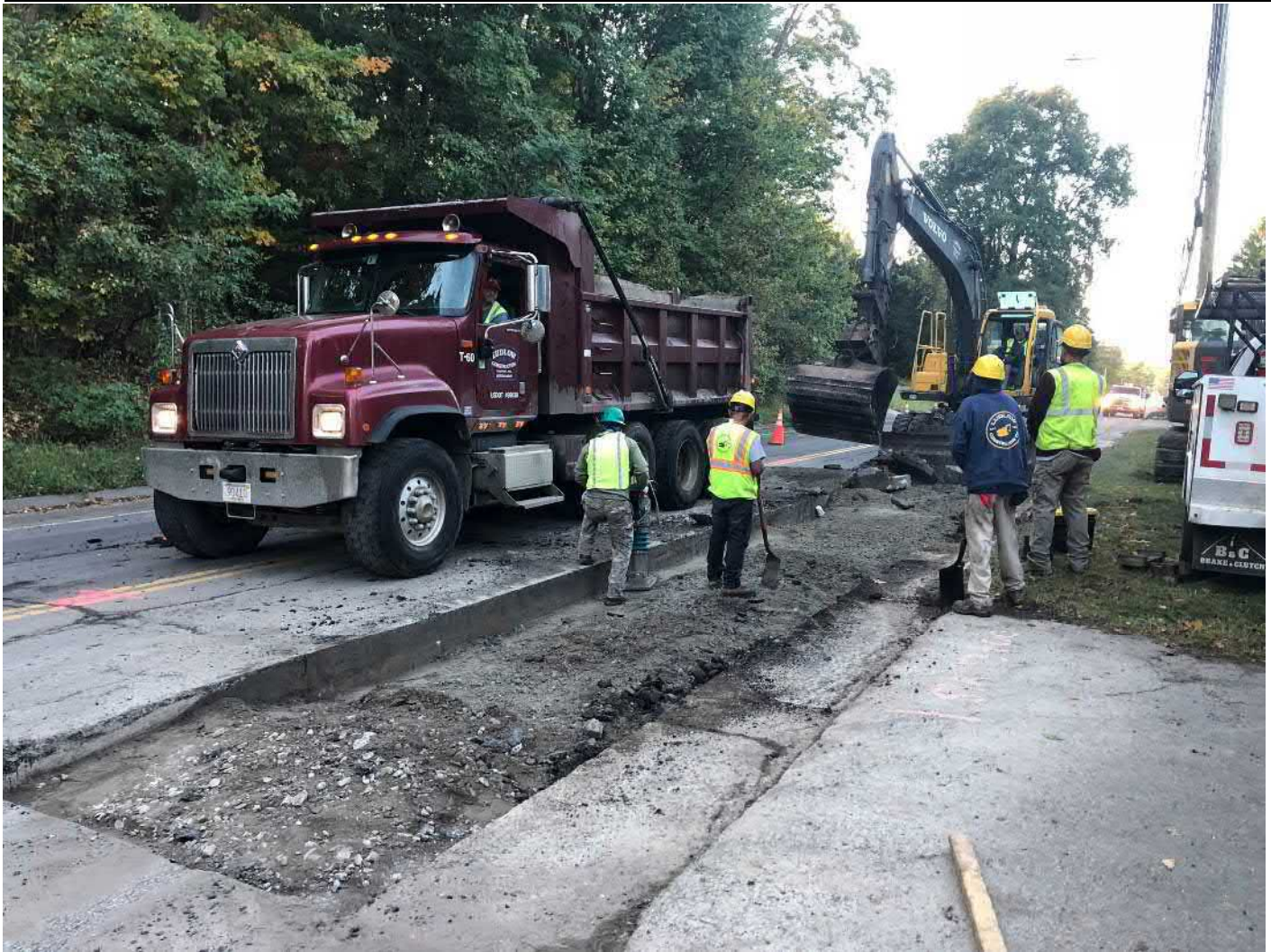
Picture 2: Ludlow stripping back asphalt as they prepare to place permanent paving on the southbound lane of Main Street, Durham from Stations 143+00 to 146+30. View to the south.
