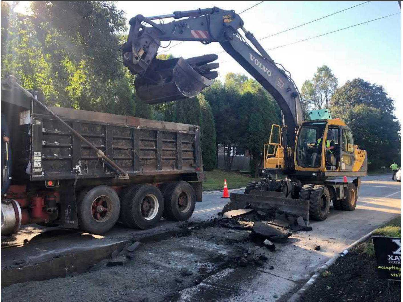
Picture 4: Ludlow stripping back asphalt as they prepare to place permanent paving on the southbound lane of Main Street, Durham from Stations 143+00 to 146+30. View to the southeast.
