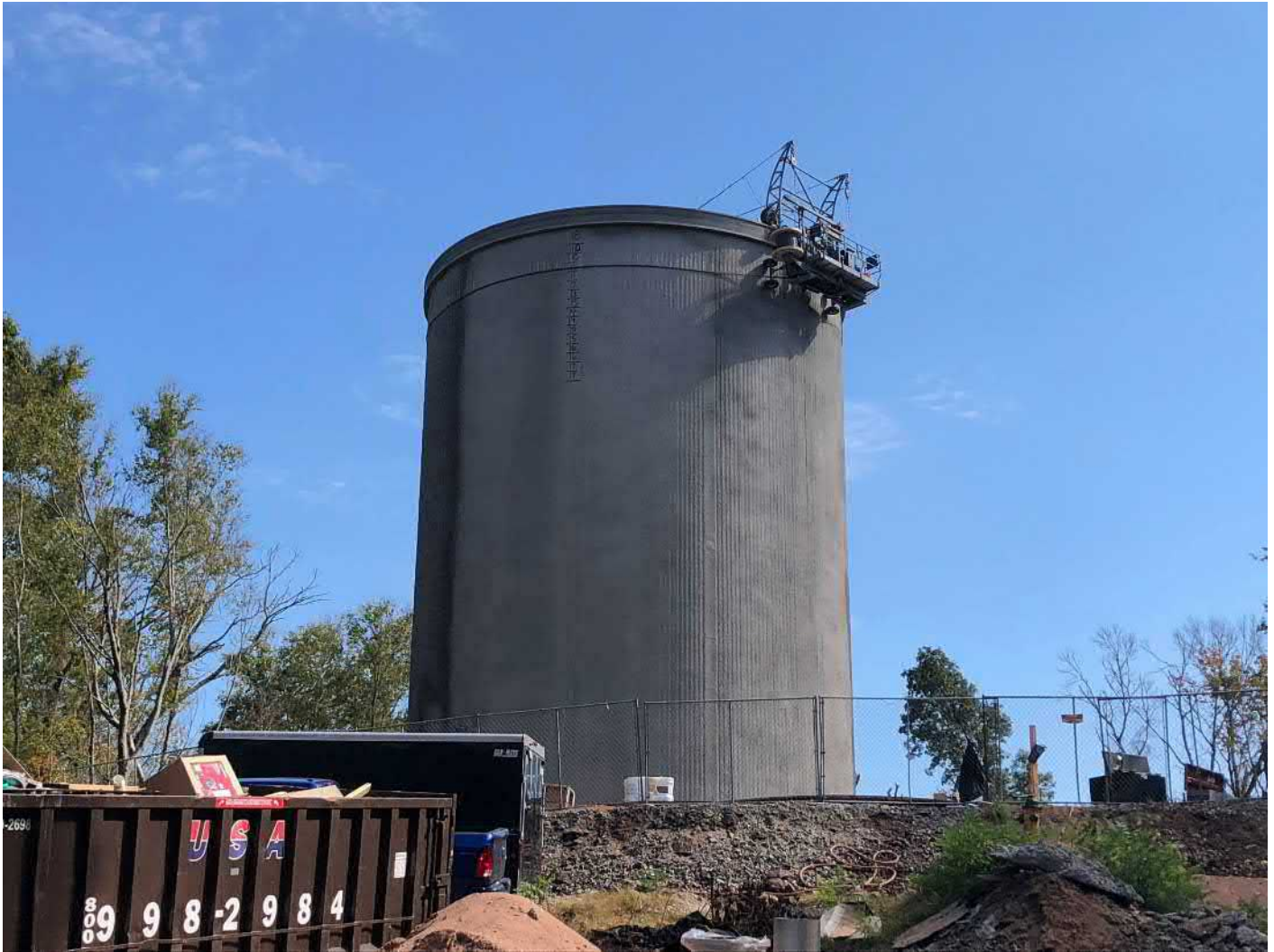
Picture 5: DN Tanks preparing to wrap prestressed wire around the sides of the water tank at the top of the tank. Water tank work zone, east of the Shared Access Driveway, Middletown. View to the northeast.
