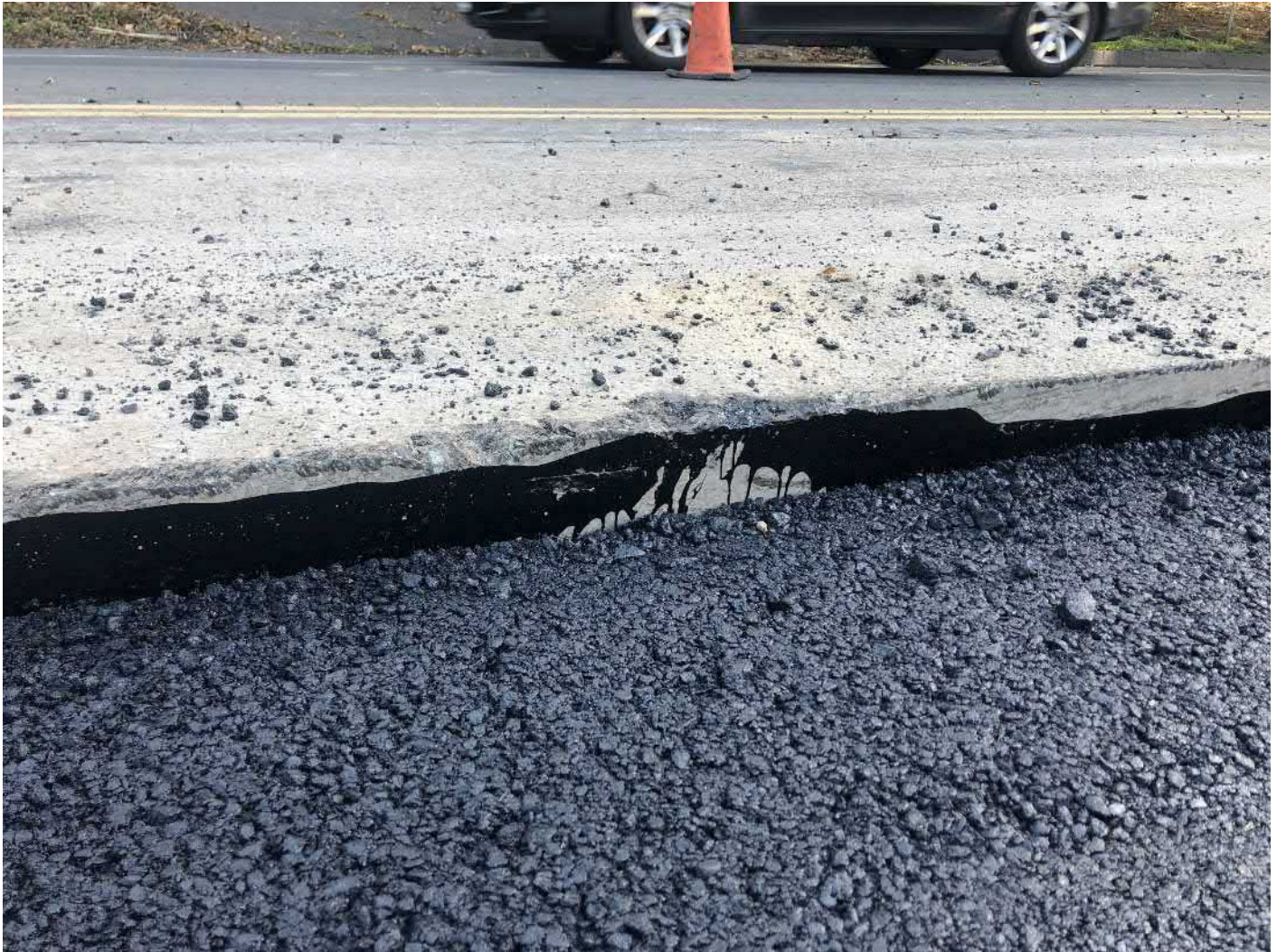
Picture 8: Tack coat applied to the sides of cut pavement as part of trench cutback paving activities on the southbound lane of Main Street, Durham from Stations 143+00 to 146+30.
