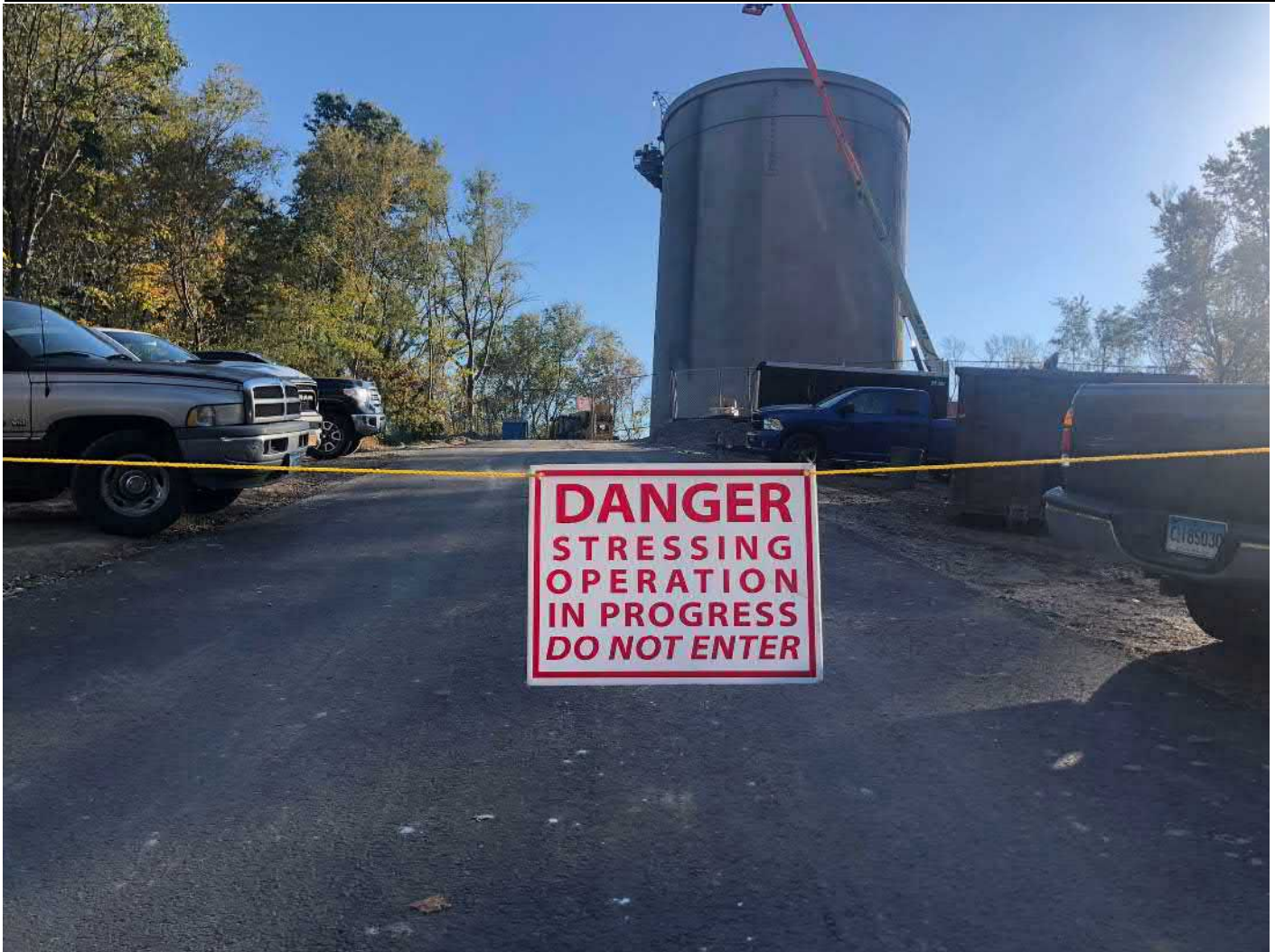
Picture 3: DN Tanks placed warning sign near the water tank work zone, east of the Shared Access Driveway, Middletown as they wrapped prestressed wire around the tank. View to the east.
