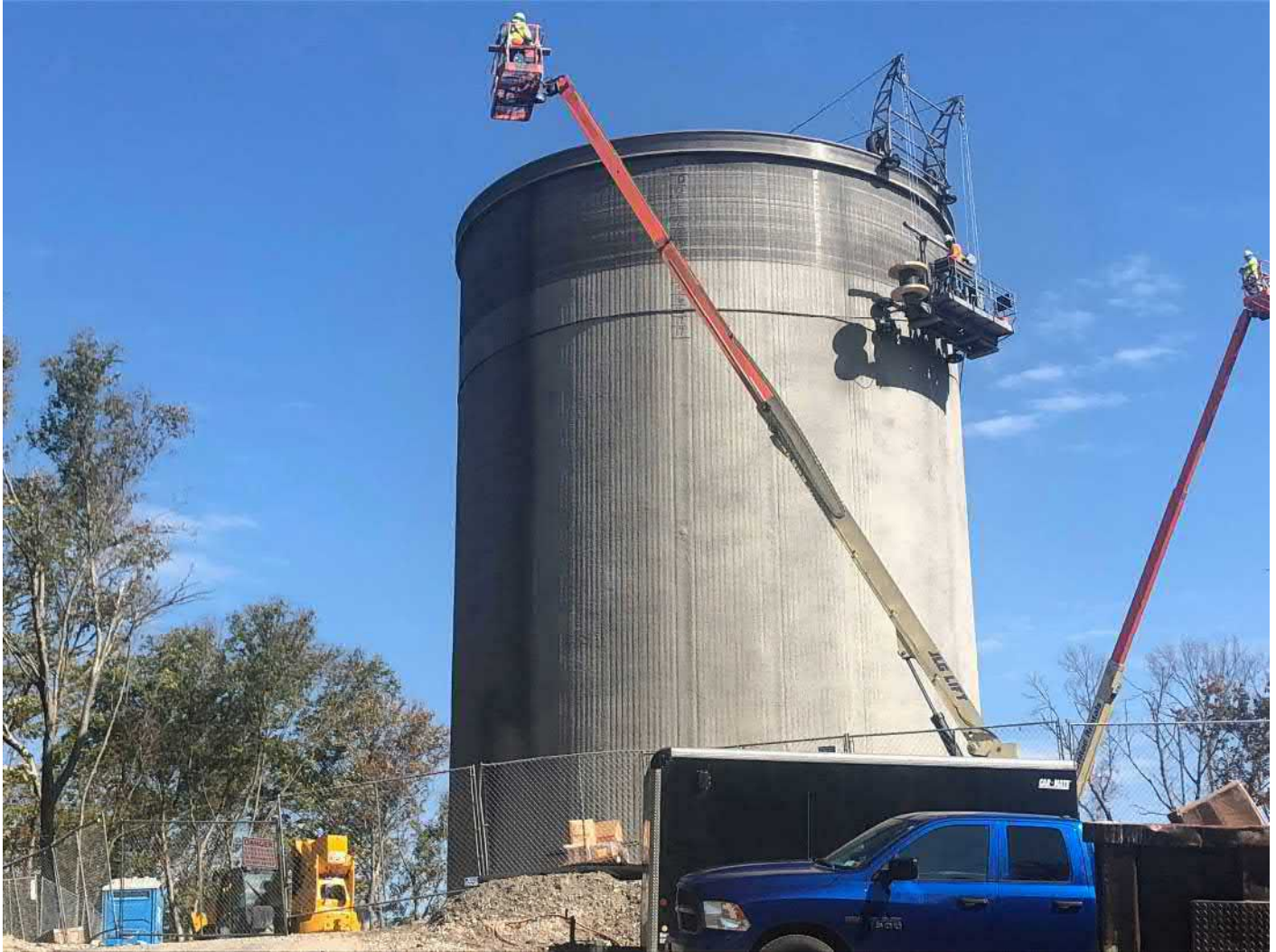
Picture 6: DN Tanks wrapping prestressed wire around the sides of the water tank at the top of the tank. Water tank work zone, east of the Shared Access Driveway, Middletown. View to the northeast.
