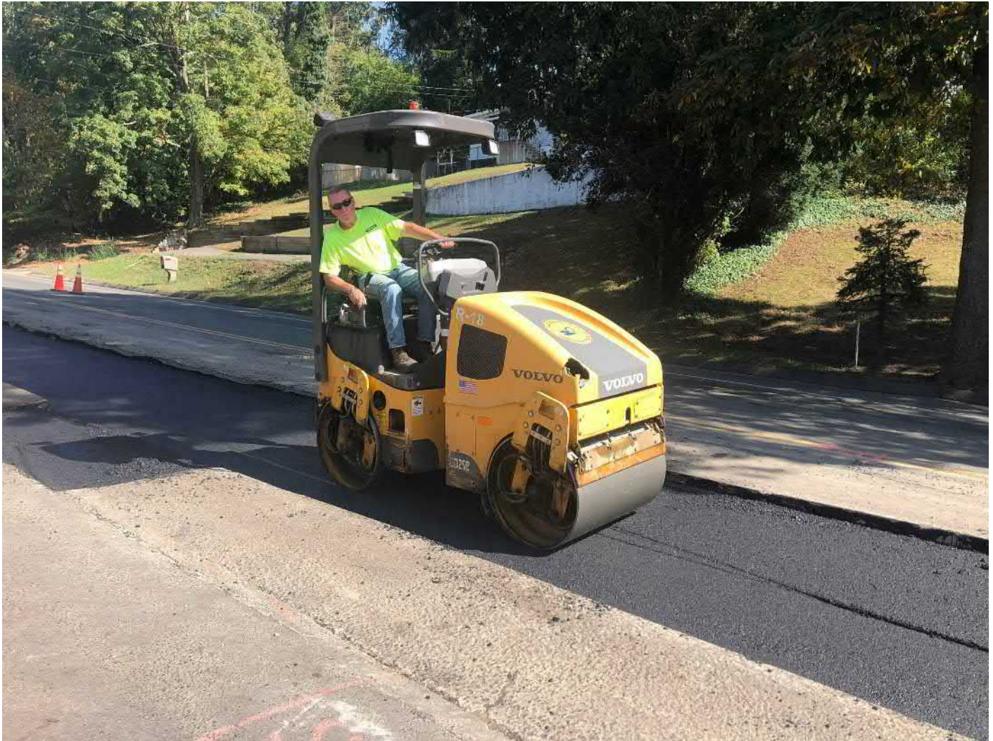
Picture 9: Ludlow compacting second lift of asphalt as part of trench cutback paving activities on the southbound lane of Main Street, Durham from Stations 143+00 to 146+30. View to the northeast.
