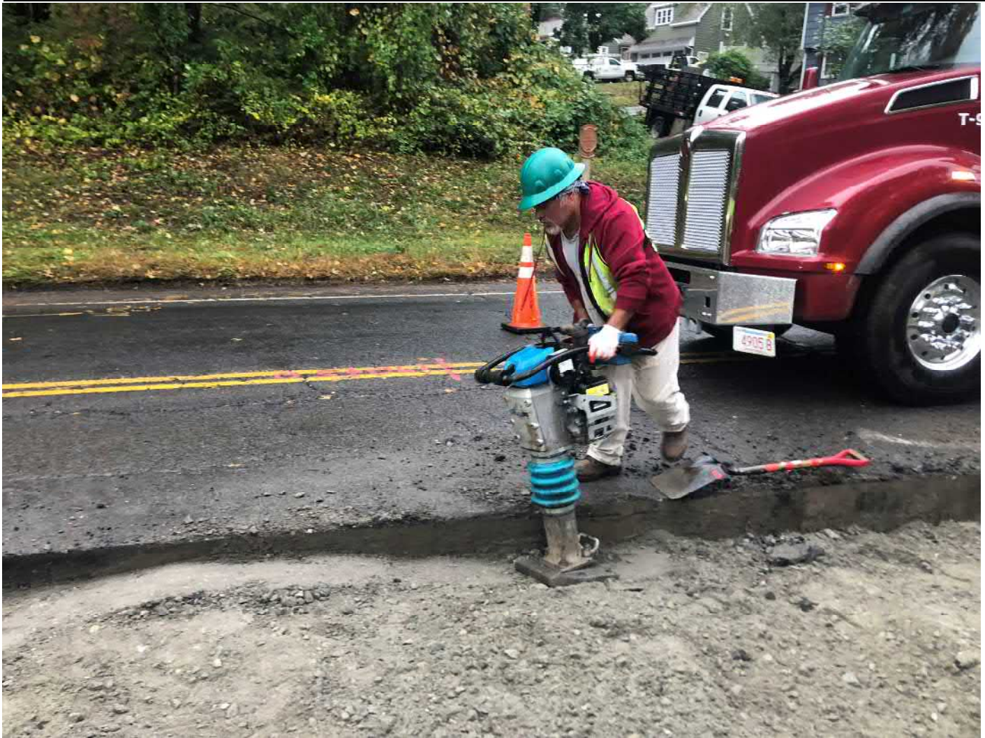
Picture 2: Ludlow compacting 1.5" processed gravel as they prepare to place permanent paving on the southbound lane of Main Street, Durham from Stations 140+50 to 143+00. View to the south.
