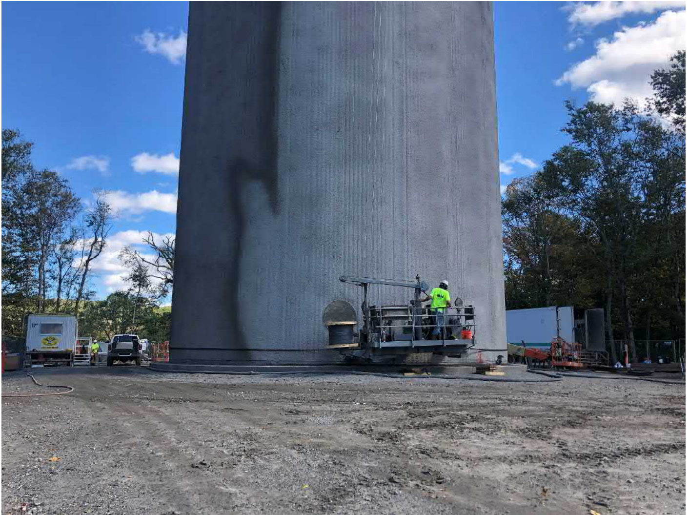
Picture 7: DN Tanks begins to wrap prestressed wire around the sides of the water tank. Water tank work zone, east of the Shared Access Driveway, Middletown. View to the east.
