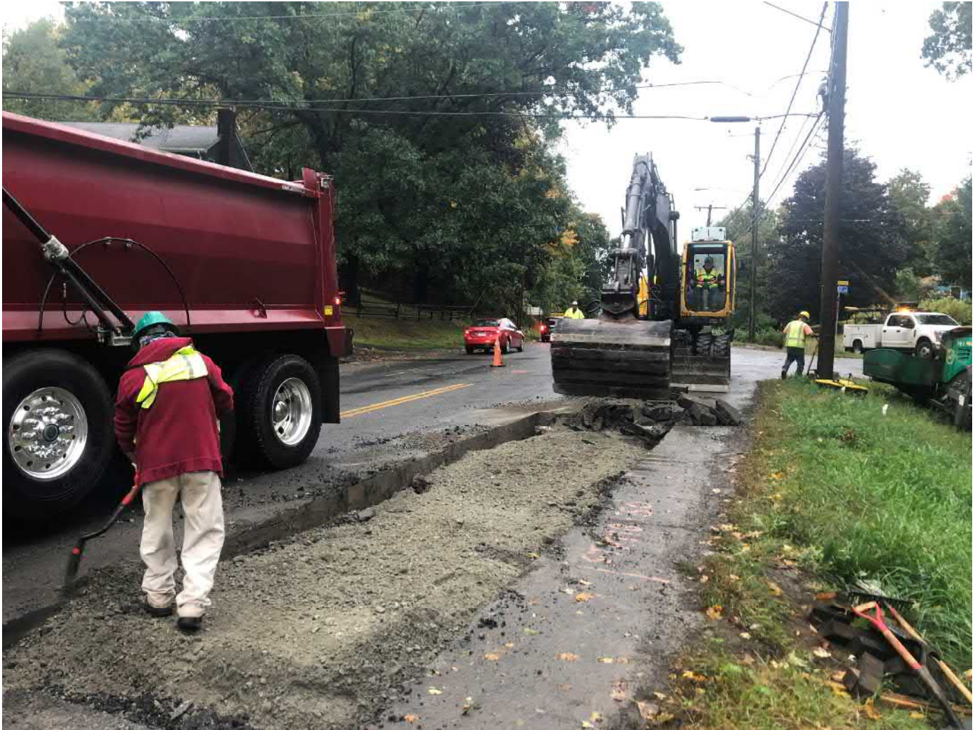
Picture 1: Ludlow in the process of stripping asphalt from trench overcuts as they prepare to place permanent paving on the southbound lane of Main Street, Durham from Stations 140+50 to 143+00. View to the south.
