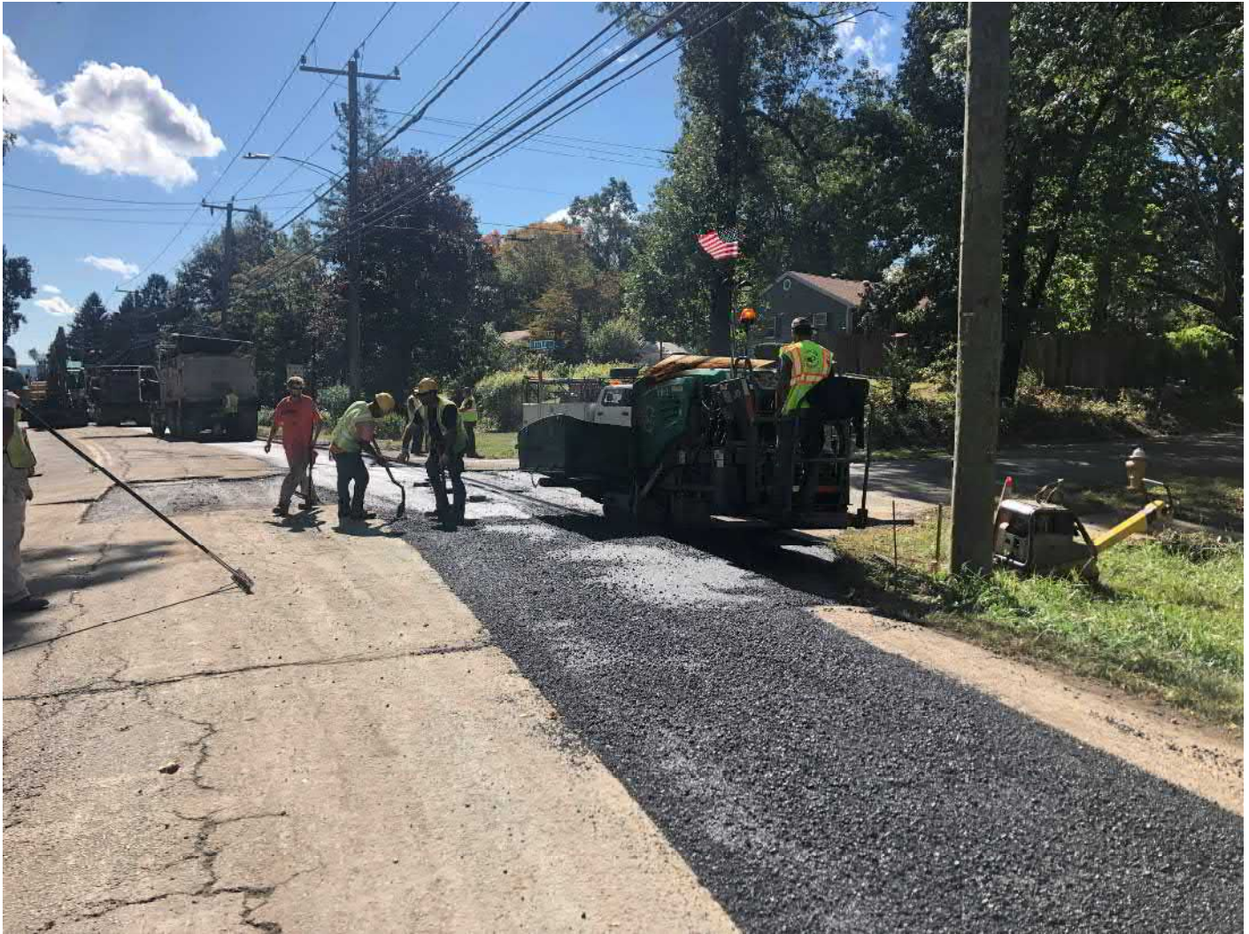
Picture 6: Ludlow placing and compacting the third of three 3" lifts of asphalt on the southbound lane of Main Street, Durham from Stations 140+50 to 143+00. View to the south.
