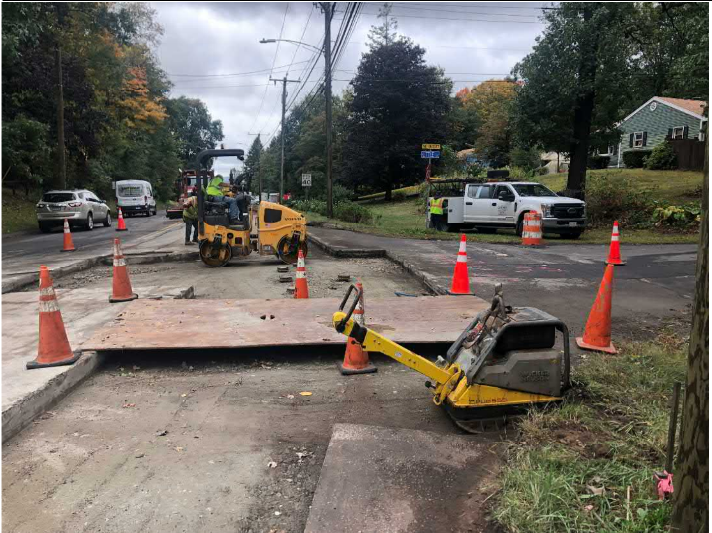
Picture 4: Ludlow compacting 1.5" processed gravel as they prepare to place permanent paving on the southbound lane of Main Street, Durham from Stations 140+50 to 143+00. View to the south.
