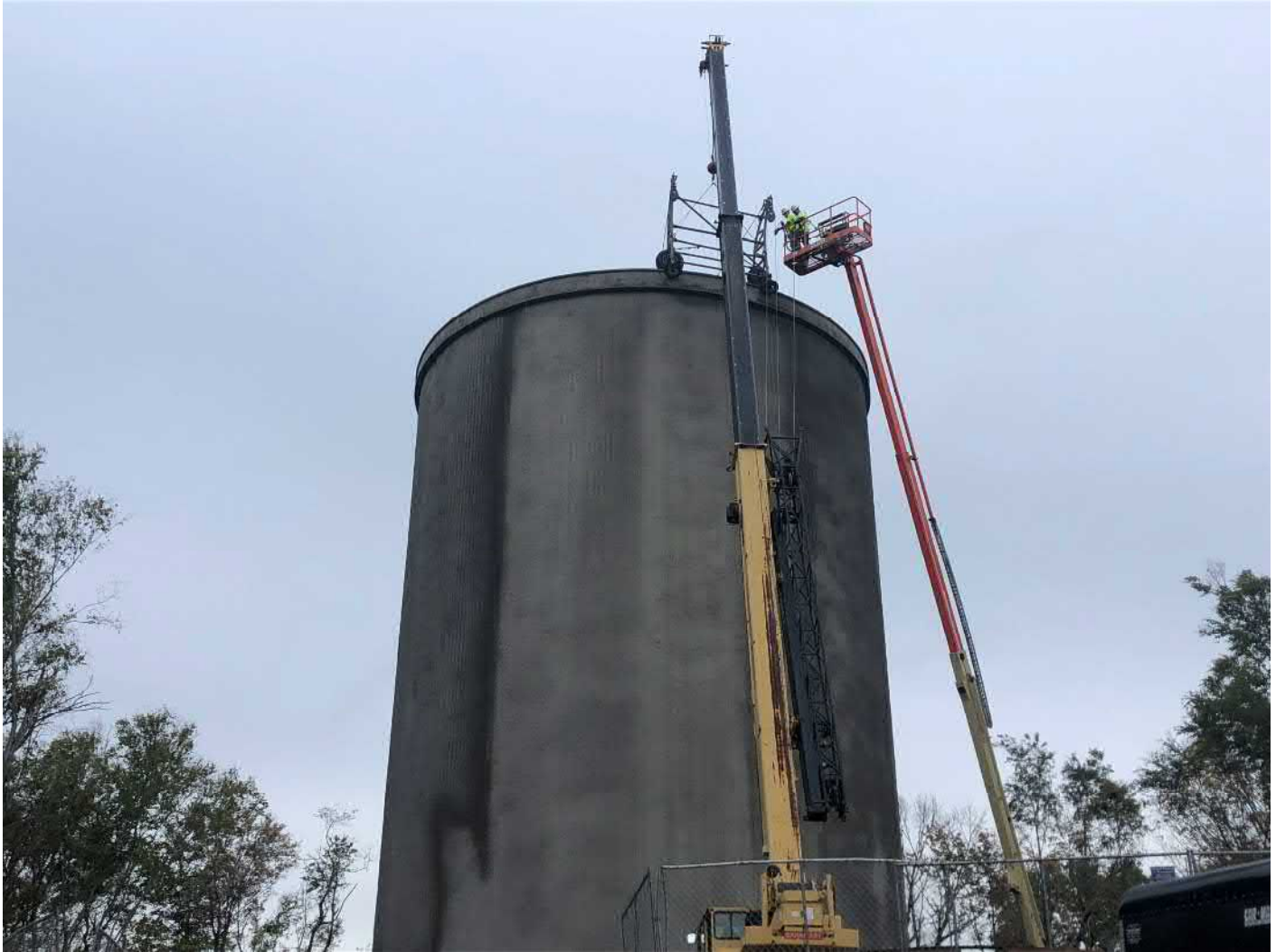
Picture 3: DN Tanks setting up to wrap prestressed wire around the sides of the water tank. Water tank work zone, east of the Shared Access Driveway, Middletown. View to the east.
