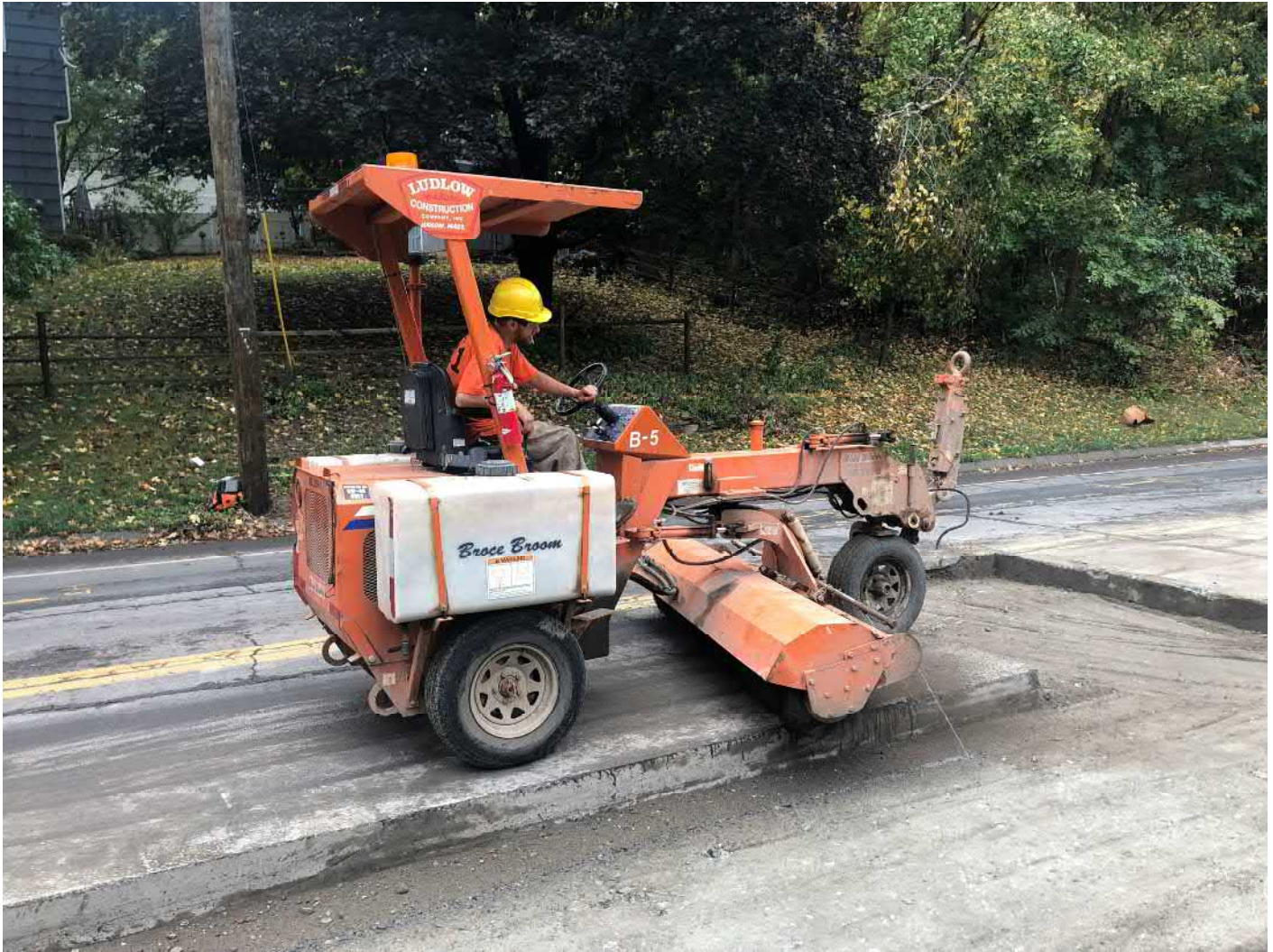
Picture 5: Ludlow using a Broce Broom to clean up the work zone as they prepare to place permanent paving on the southbound lane of Main Street, Durham from Stations 140+50 to 143+00. View to the southeast.
