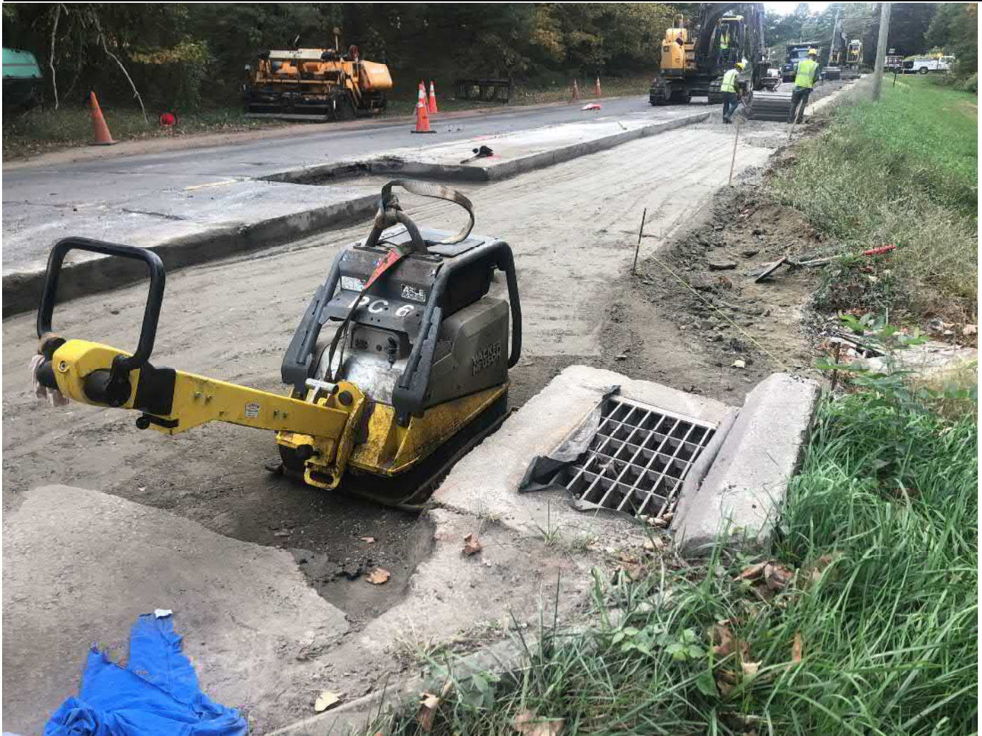
Picture 4: Ludlow in the process of stripping asphalt from trench overcuts as they prepare to place permanent paving on the southbound lane of Main Street, Durham from Stations 136+96 to 140+50. View to the south.
