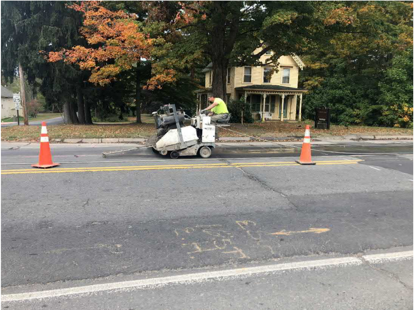
Picture 3: Veilleux saw cutting pavement on the southbound lane of Main Street, Durham at Station 175+00. View to the west.
