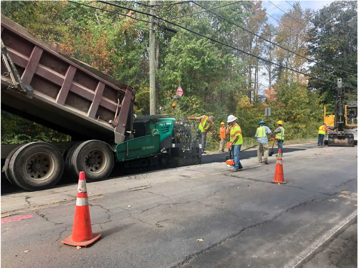
Picture 9: Ludlow placing the third of three 3" lifts of asphalt between Stations 136+95 and 140+50 as part of trench cutback paving activities on the southbound lane of S. Main Street, Middletown. View to the northwest.
