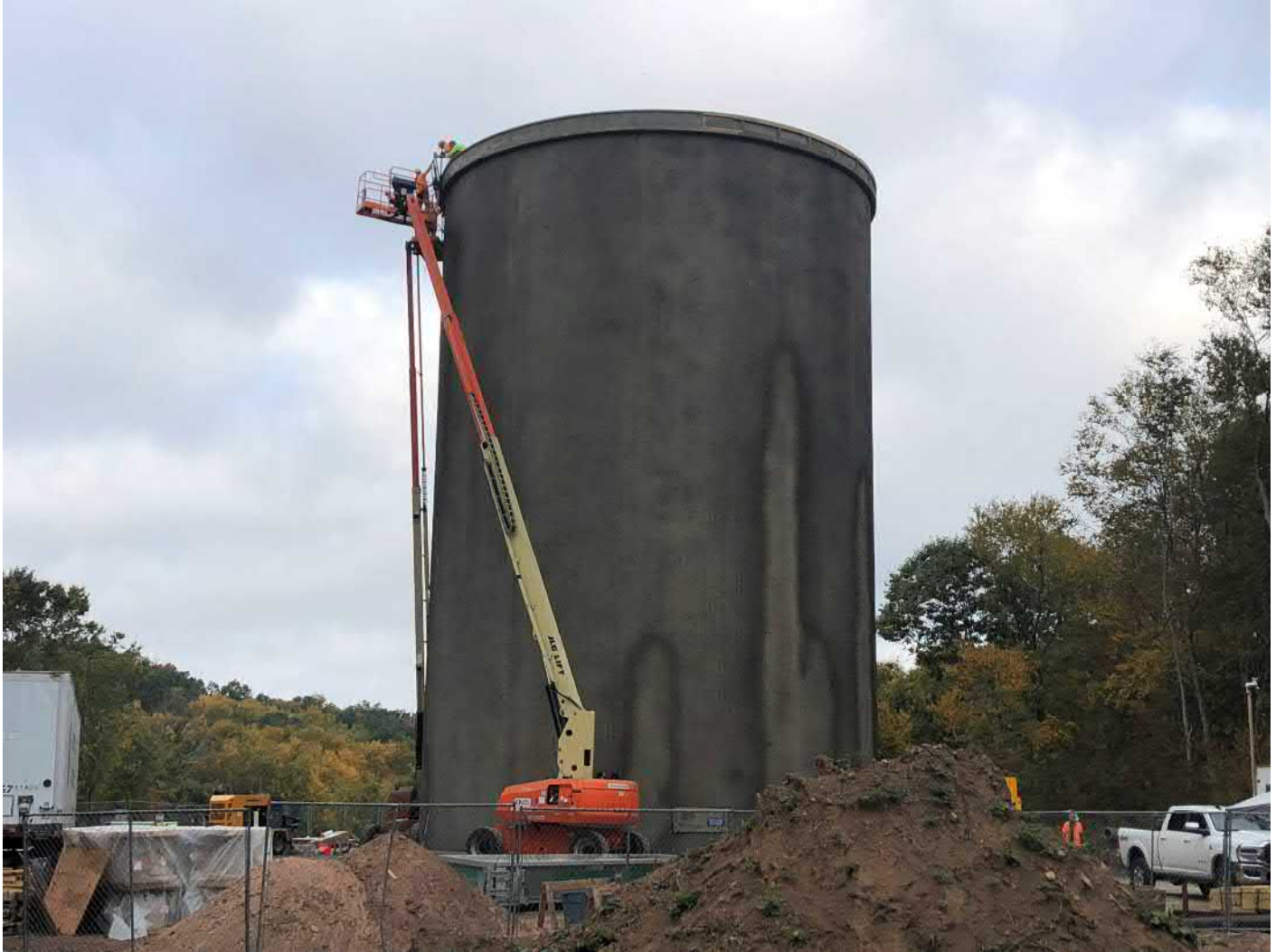
Picture 1: DN Tanks removing dome rim form from the top of the water tank, which was coated with shotcrete yesterday. Water tank work zone, east of the Shared Access Driveway, Middletown. View to the west.
