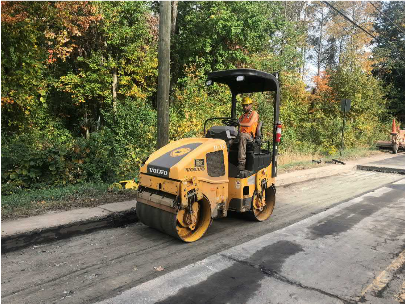
Picture 5: Ludlow compacting 1.5" processed gravel as they prepare to place permanent paving on the southbound lane of Main Street, Durham from Stations 136+96 to 140+50. View to the northwest.
