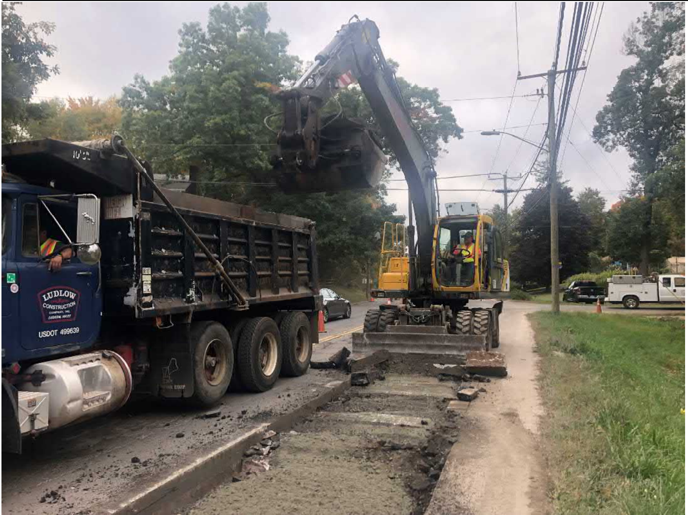
Picture 6: Ludlow stripping asphalt from trench overcuts as they prepare to place permanent paving on the southbound lane of Main Street, Durham from Stations 136+96 to 140+50. View to the south.
