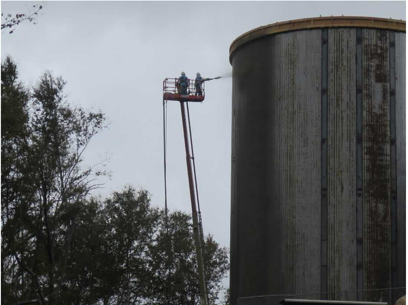
Picture 2: Applying coat of sprayed concrete mix on northwest side of tank wall. View to the east.
