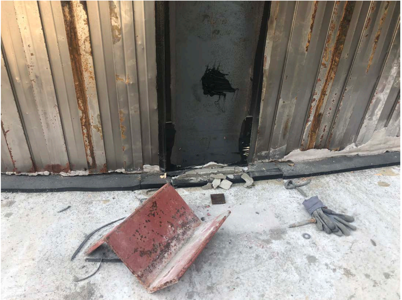
Picture 4: Brace removed from the toe of a slot panel on the water tank a day after grout was poured. Water tank work zone, east of the Shared Access Driveway, Middletown.
