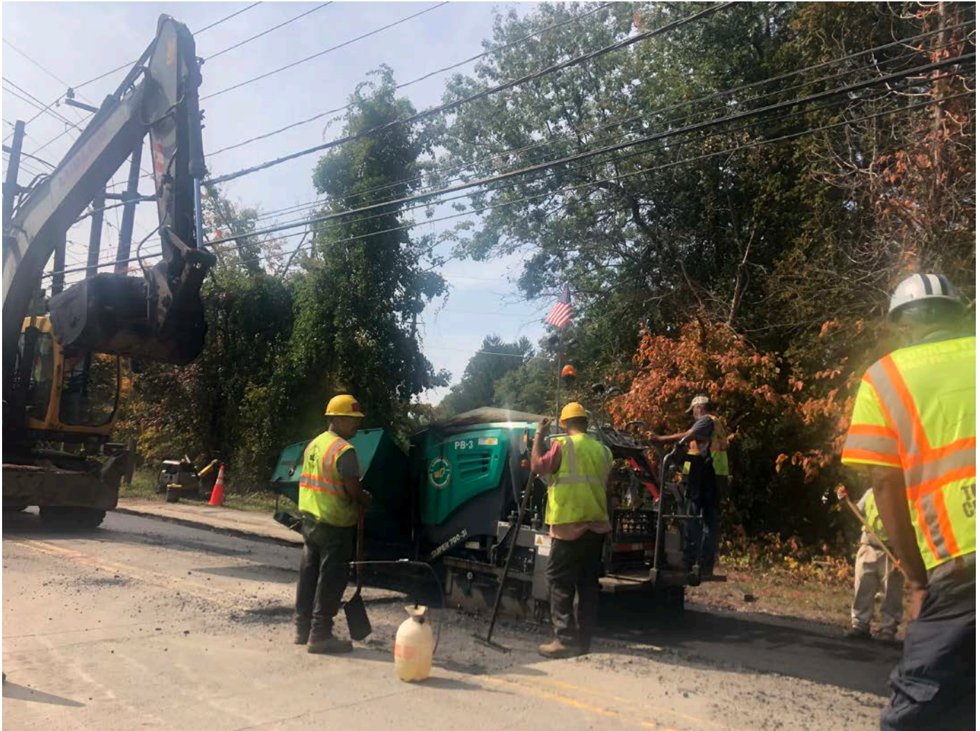
Picture 3: Ludlow placing the third of three 3" lifts of asphalt between Stations 130+00 and 134+00 as part of trench cutback paving activities on the southbound lane of S. Main Street, Middletown. View to the southwest.
