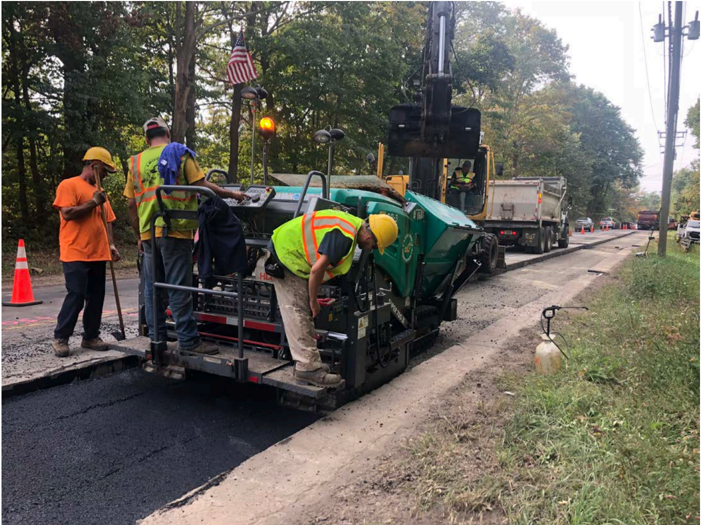
Picture 9: Ludlow placing the first of three 3" lifts of asphalt between Stations 126+00 and 130+00 as part of trench cutback paving activities on the southbound lane of S. Main Street, Middletown. View to the south.
