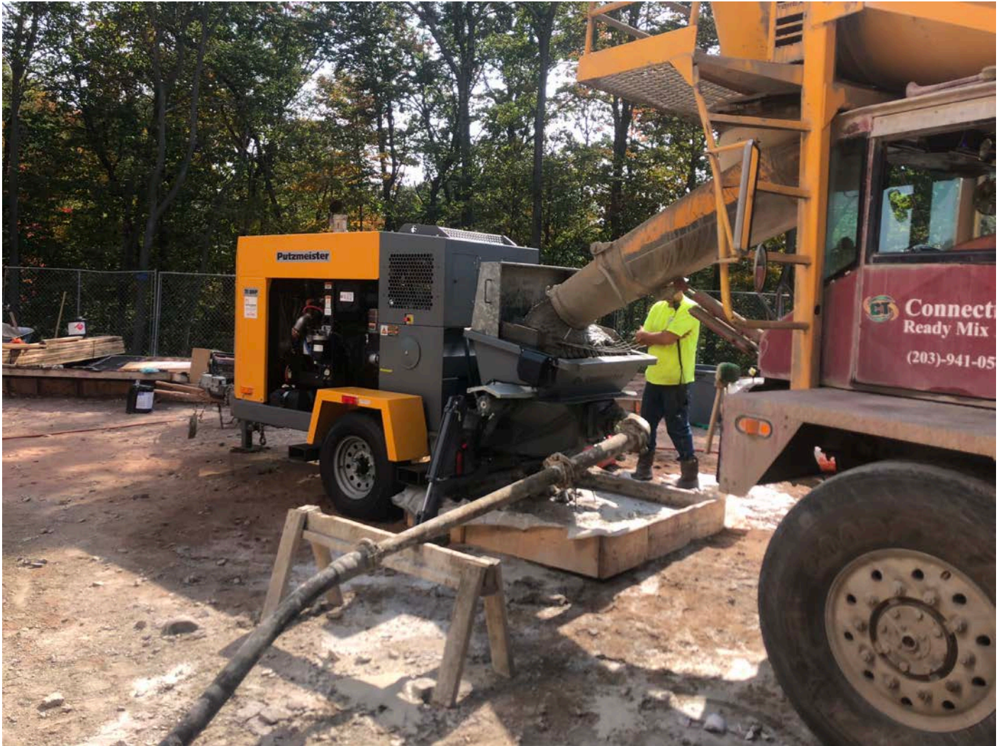
Picture 7: CT Ready Mix pumping concrete into a pump trailer that, in turn, is pumping concrete to the top of the water tower for a dome pour. Water tank work zone east of the Shared Access Driveway, Middletown. View to the south.
