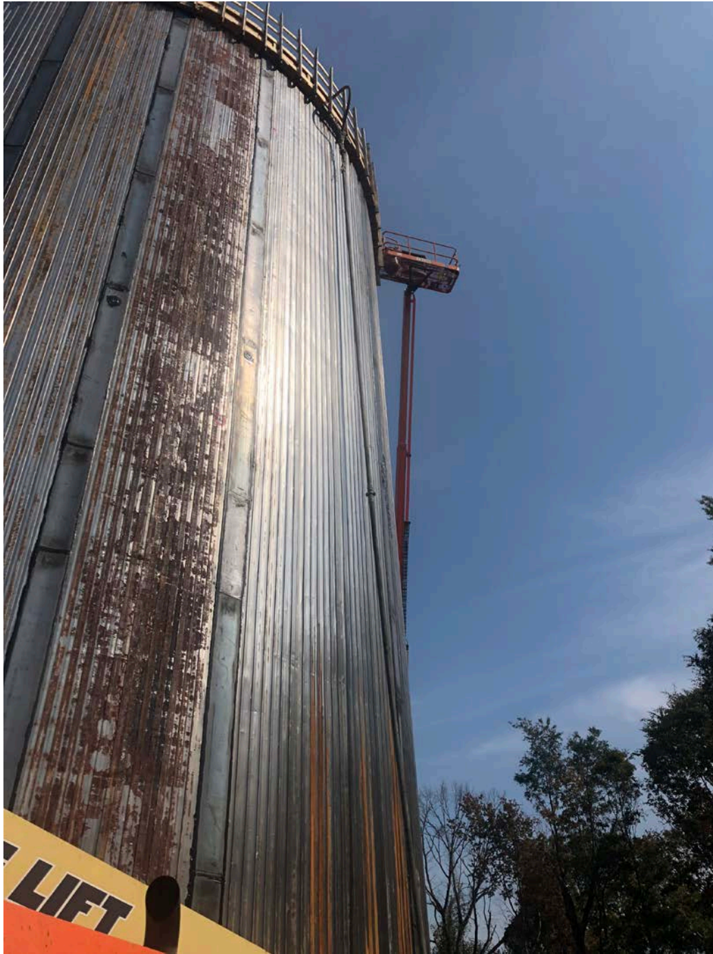
Picture 6: Hose run up the side of the water tank that was used in pumping concrete to top of the water tank today. Water tank work zone east of the Shared Access Driveway, Middletown. View to the southeast.
