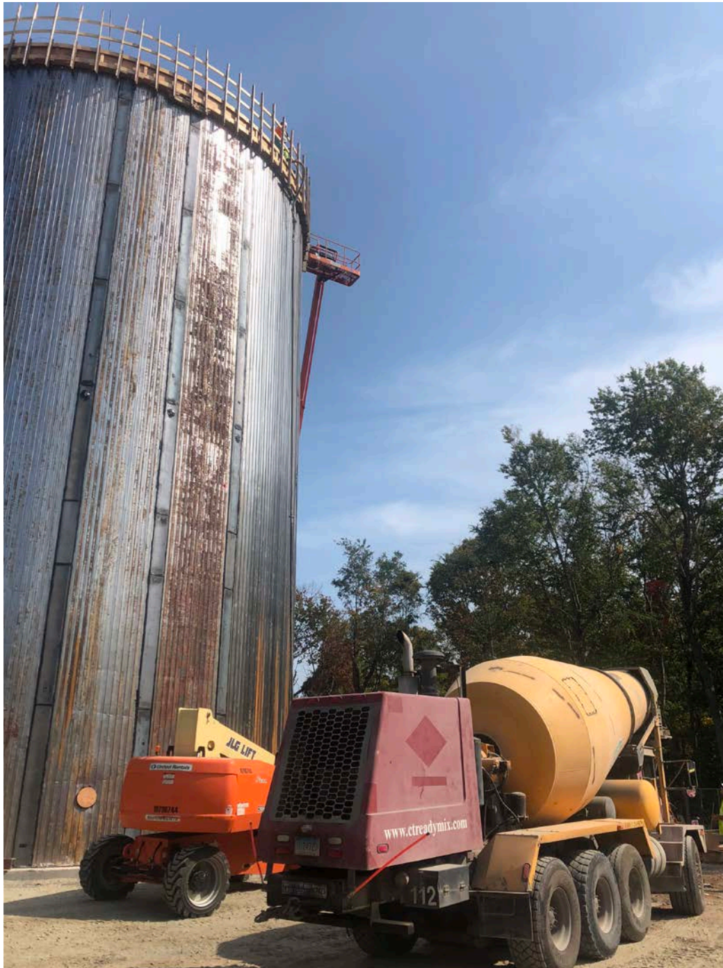
Picture 8: Overview of concrete being pumped to the top of the water tower for a dome pour. Water tank work zone east of the Shared Access Driveway, Middletown. View to the southeast.
