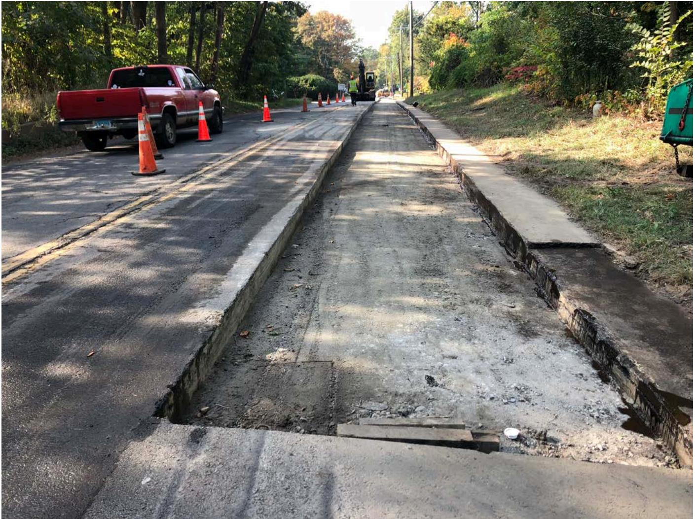
Picture 1: Ludlow removing pavement from the trench cutback zone on the southbound lane of S. Main Street, Middletown where they will pave later today. View to the south.
