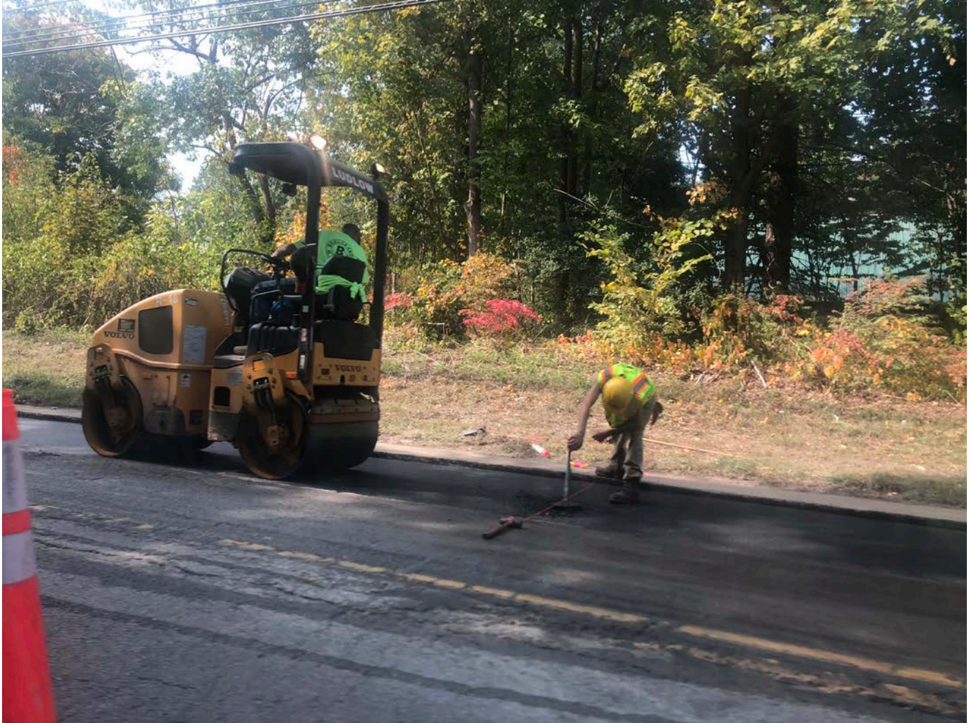
Picture 2: Ludlow raising a road box as they compact pavement between Stations 130+00 and 134+00 on the southbound lane of S. Main Street, Middletown. View to the southwest.
