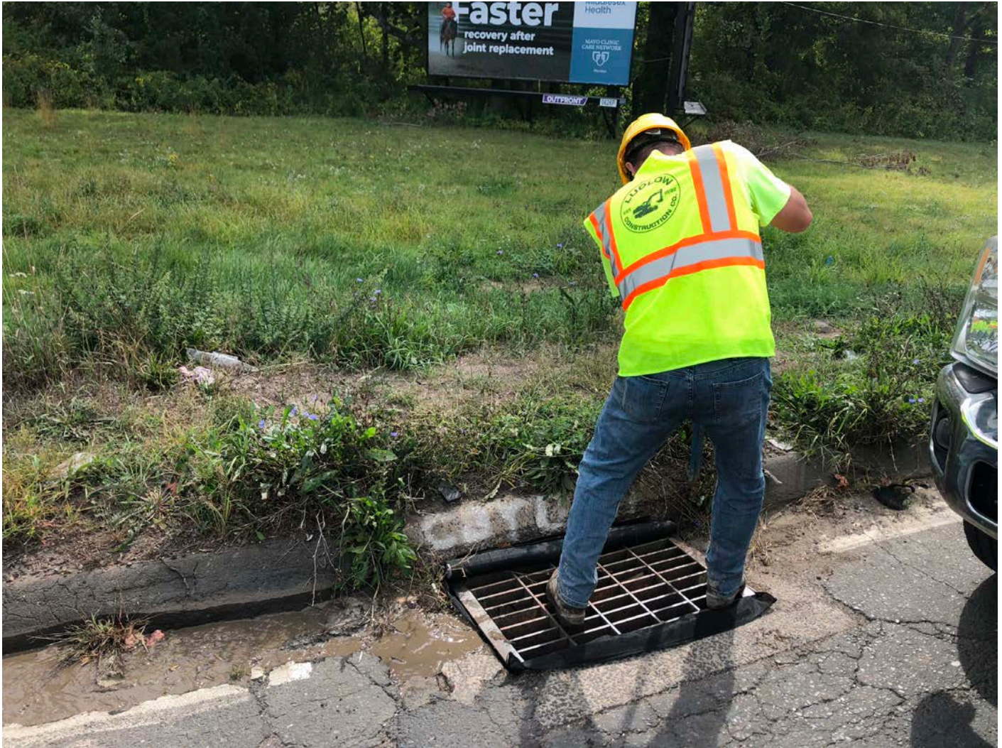
Picture 7: Ludlow installing a silt sock on the catch basin located at Station 164+30 on the northbound lane of Main Street, Durham. View to the north.
