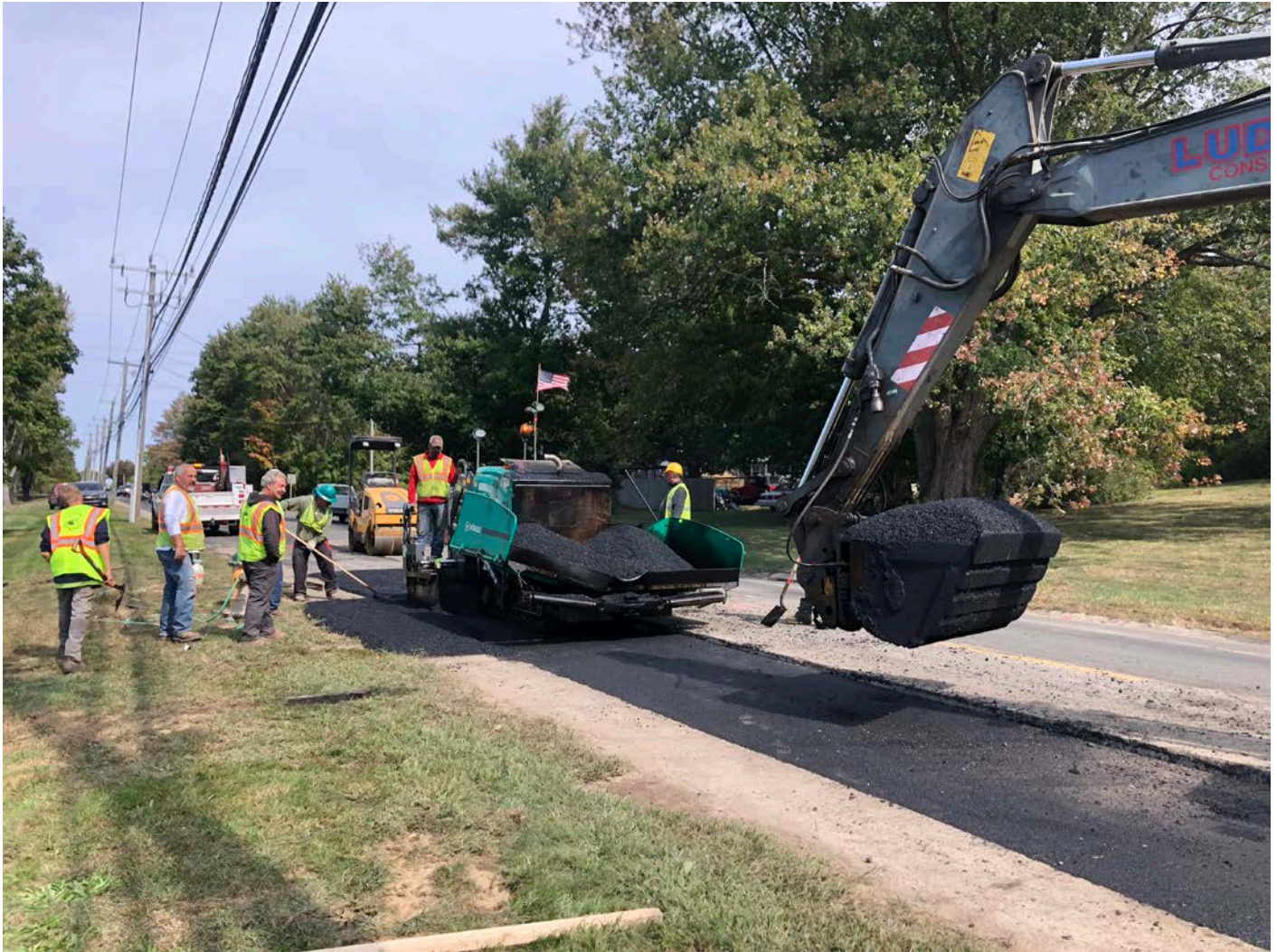
Picture 5: Ludlow placing the third of three 3” lifts of asphalt as part of trench cutback activities on S. Main Street in Middletown. View to the northeast.
