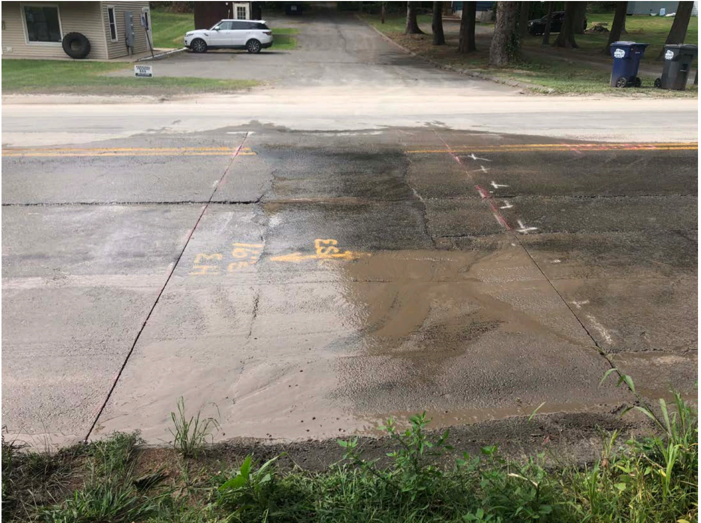
Picture 10: Freshly cut curb stop cutback at Station ~146+50 on Main Street, Durham. View to the west.
