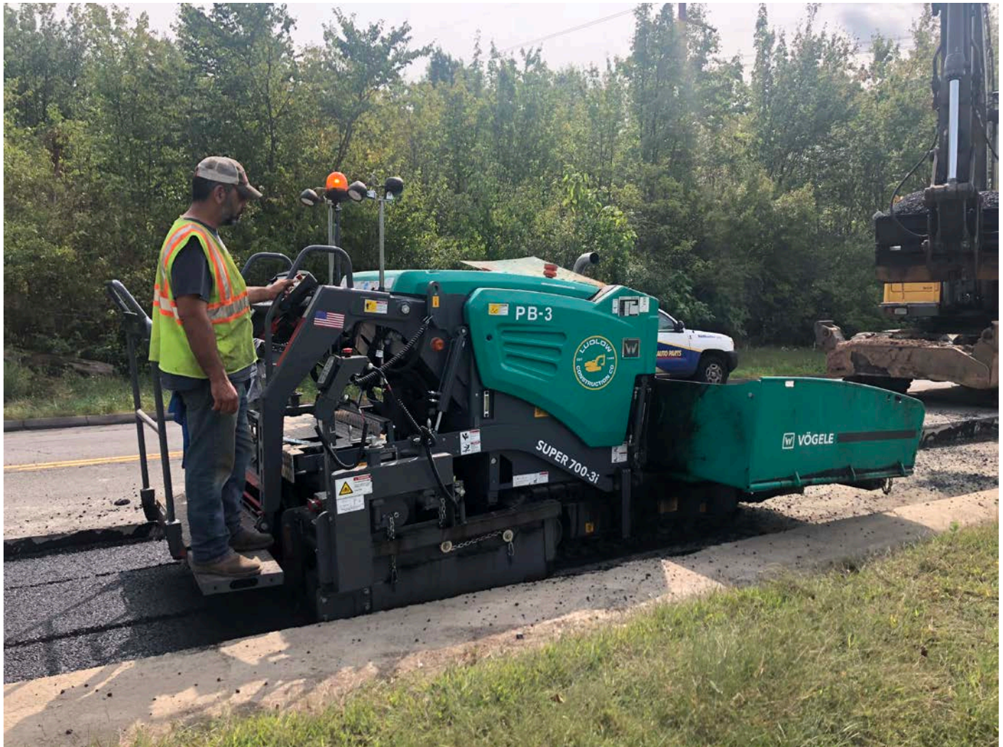
Picture 8: Ludlow placing the first of three 3" lifts of asphalt at the trench cutbacks on S. Main Street in Middletown. Station 109+50. View to the east.
