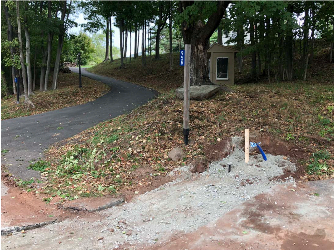
Picture 4: Curb stop that was installed at Station 909+00 (95R Maple Avenue, Durham). View to the northeast.
