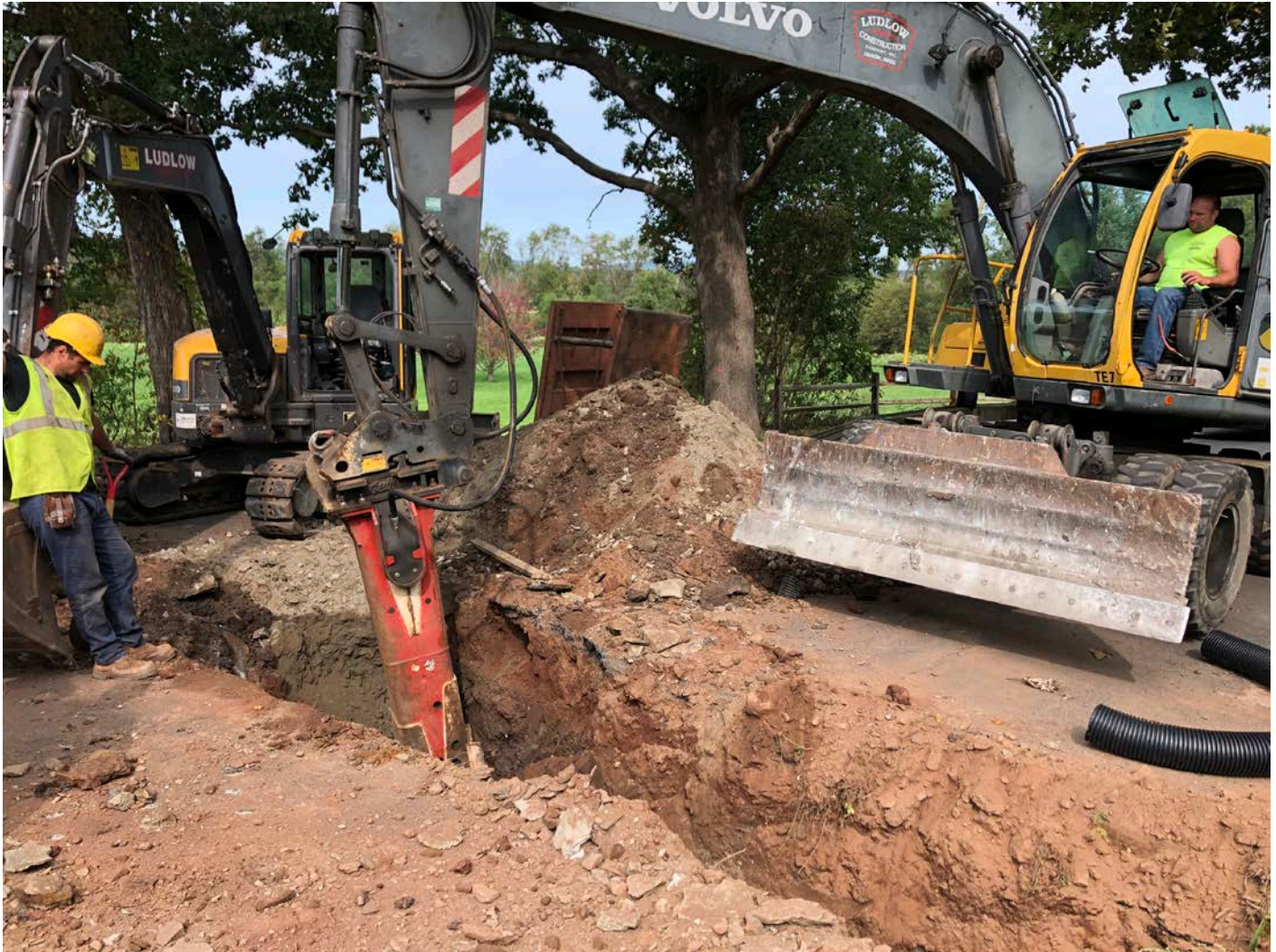
Picture 5: Ludlow hammering rock at Station 901+54 on Maple Avenue for the installation of a curb stop at 10 John's Way.
