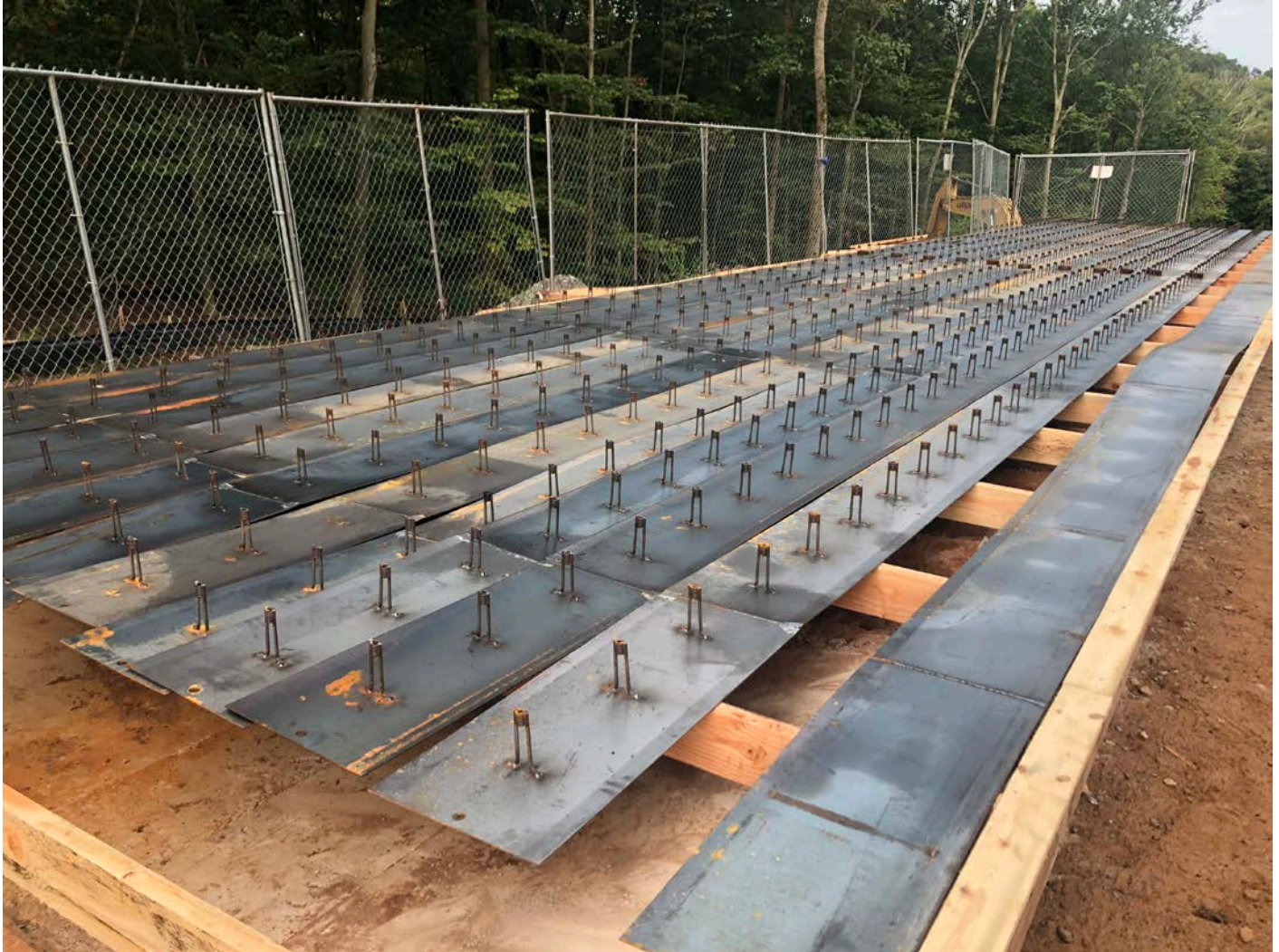
Picture 1: Slot panels laid out and welded together, waiting to be sandblasted. Water tank work zone, east of the Shared Access Road, Middletown. View to the west.
