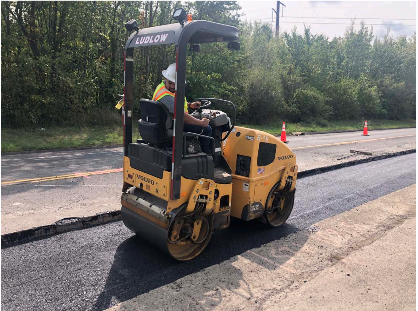
Picture 7: Ludlow rolling freshly-placed asphalt at the trench cutbacks on S. Main Street in Middletown. Station 109+50. View to the southeast.
