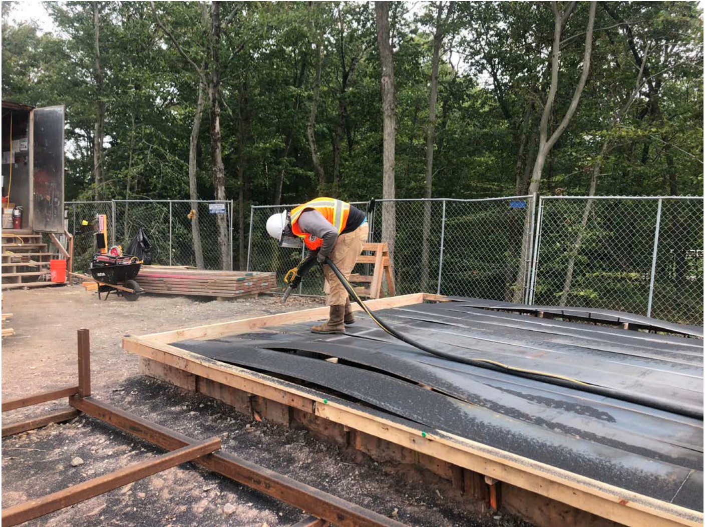
Picture 11: DN Tanks sandblasting slot panels. Water tank work zone, east of the Shared Access Driveway, Middletown. View to the southeast.
