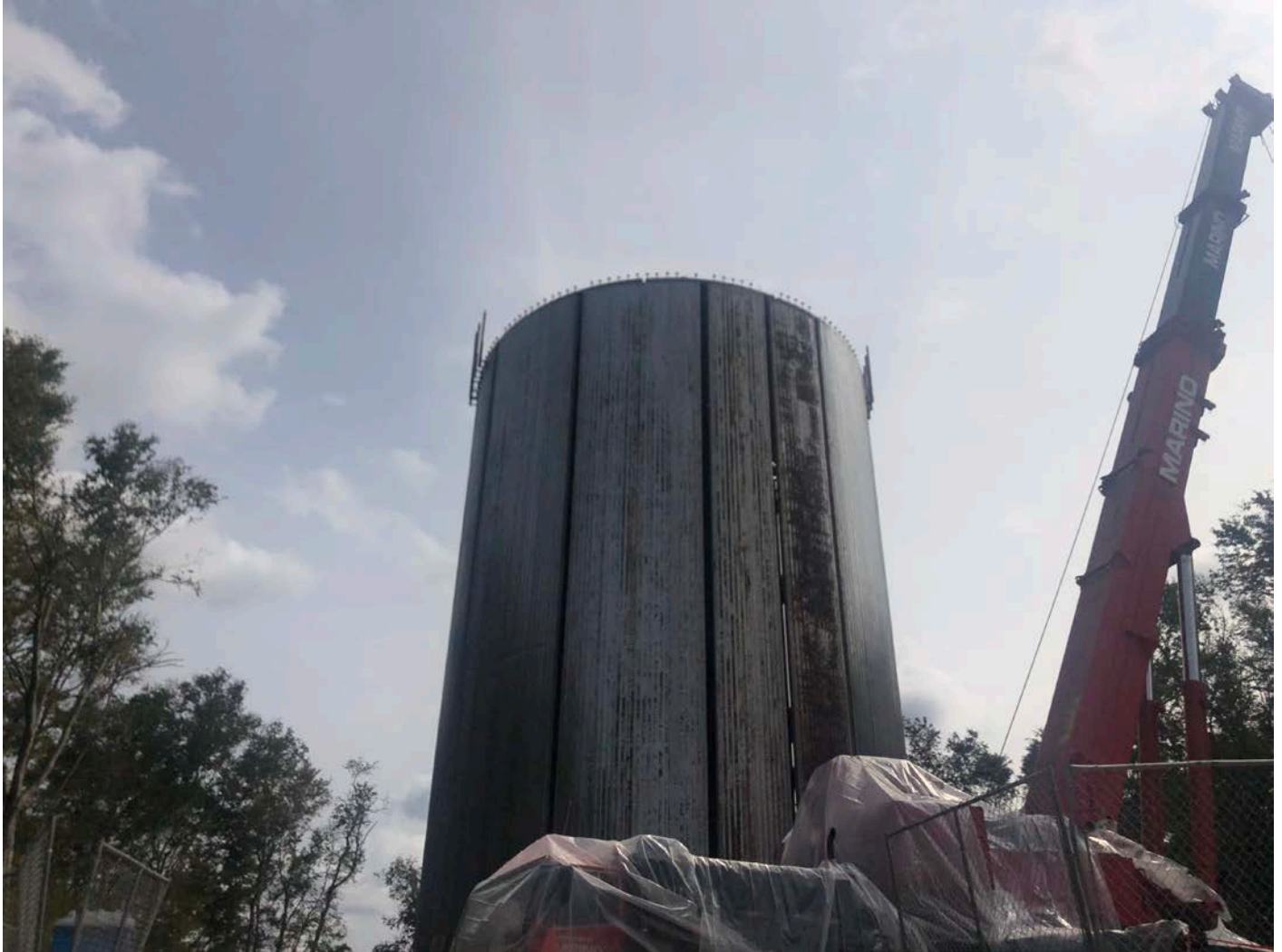
Picture 6: DN Tanks has started to install P-brackets at the top of the water tank. Water tank work zone, east of the Shared Access Driveway, Middletown. View to the east.
