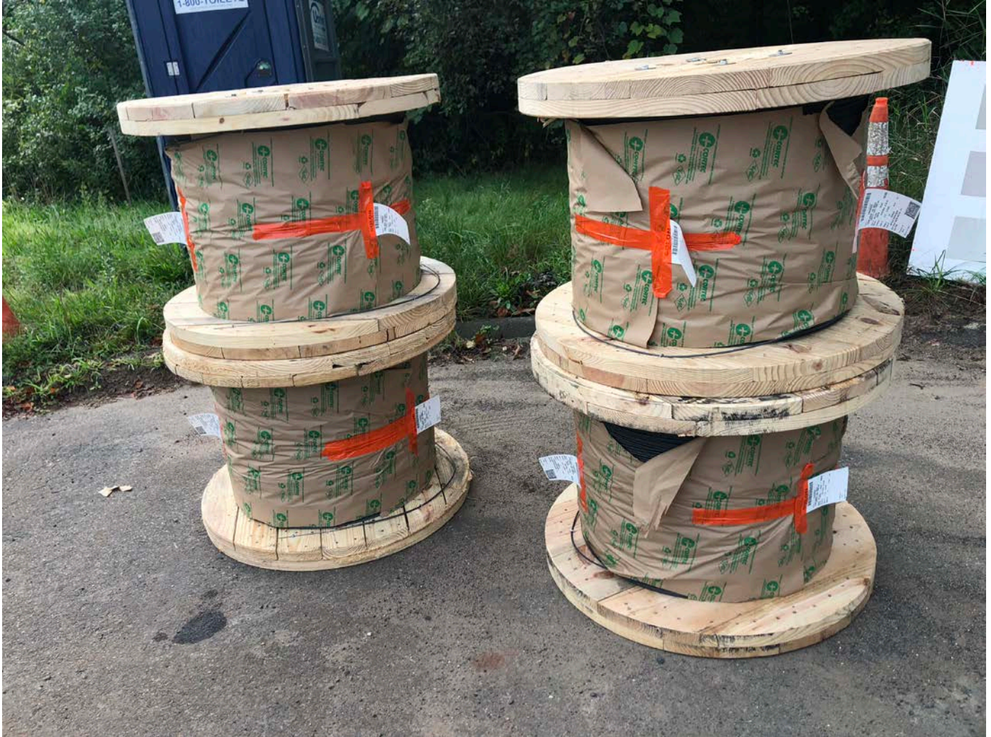
Picture 2: Prestressing wire that was delivered to the water tank work zone, east of the Shared Access Driveway, Middletown.
