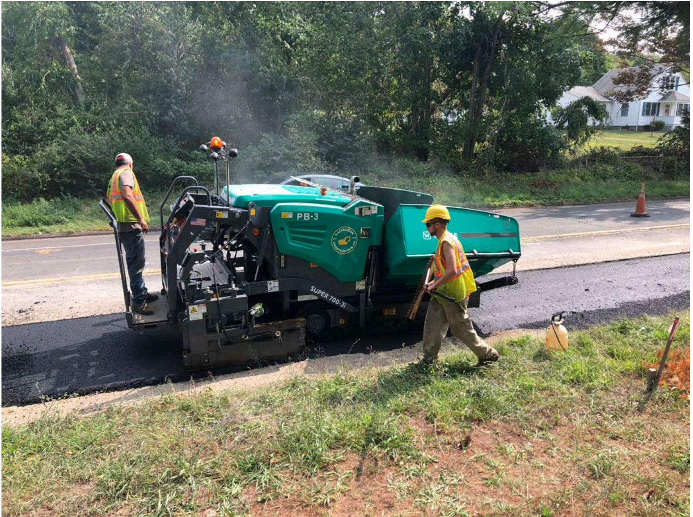
Picture 12: Ludlow placing third 3" lift of asphalt for the trench cutback repaving on S. Main Street, Middletown. View to the southeast.
