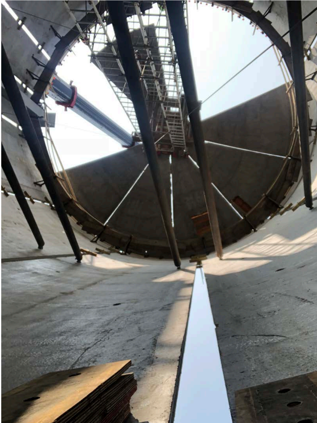
Picture 11: Marino holding the sixth dome panel in place for installation by DN Tanks. Water tank work zone, east of the Shared Access Driveway, Middletown.
