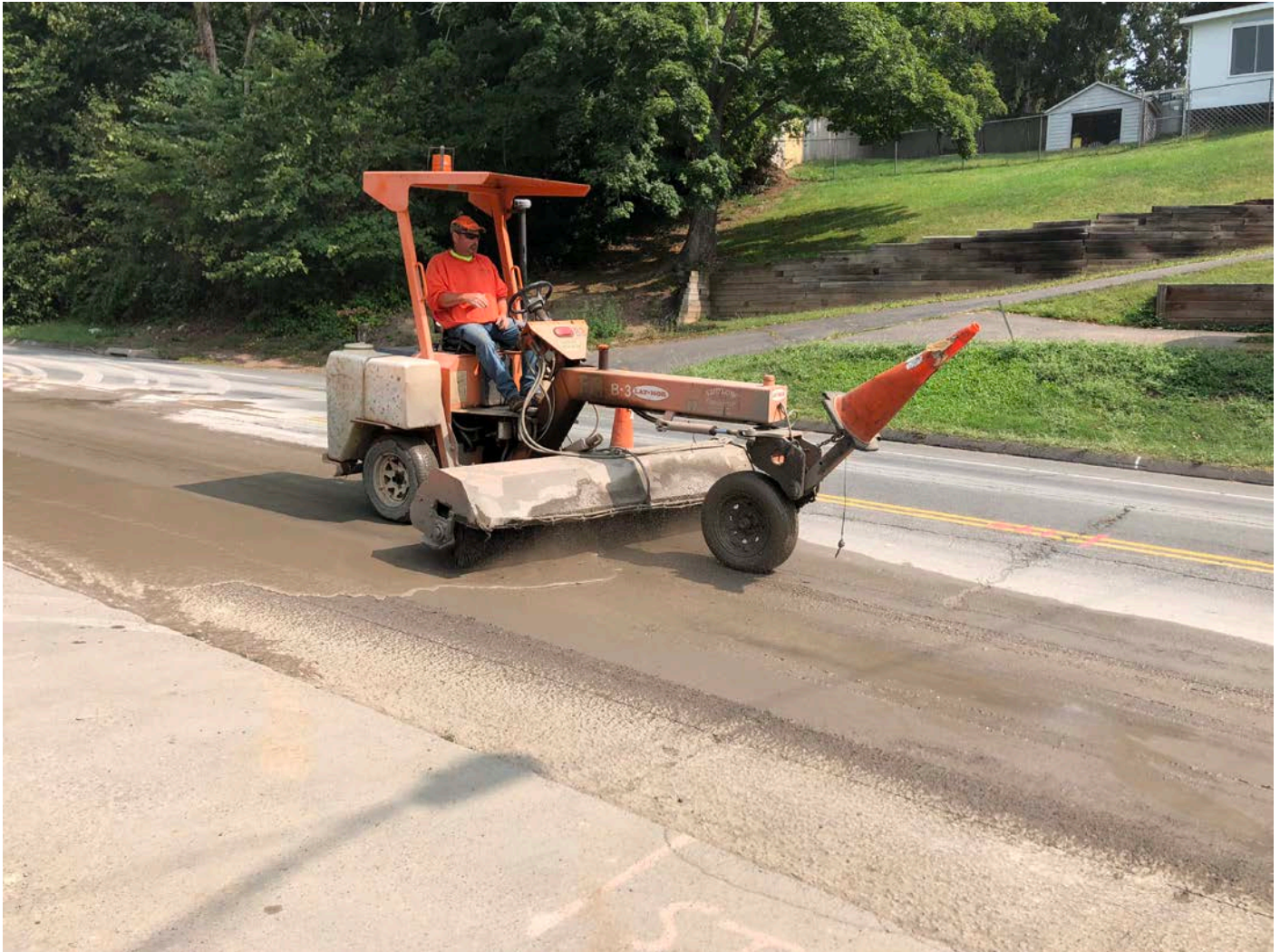
Picture 9: Ludlow using the Broce Broom to clean up after pavement saw cutting activities on the southbound lane of Main Street, Durham. Station 146+00. View to the northeast.
