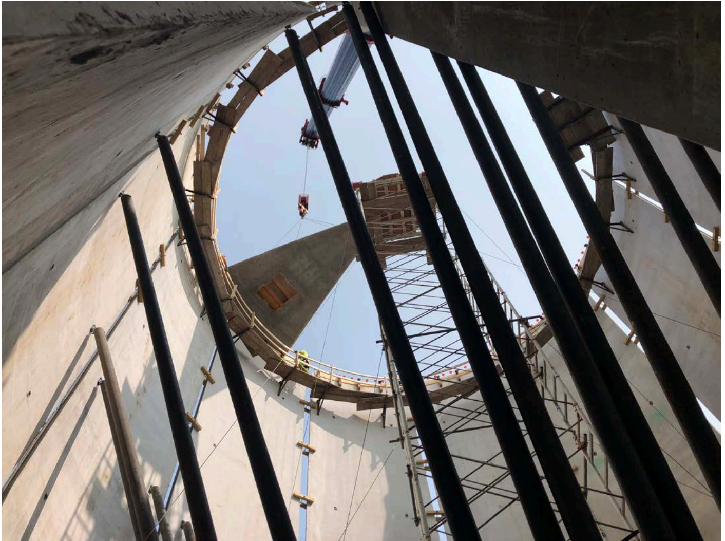
Picture 10: Marino holding the first dome panel in place for installation by DN Tanks. Water tank work zone, east of the Shared Access Driveway, Middletown.
