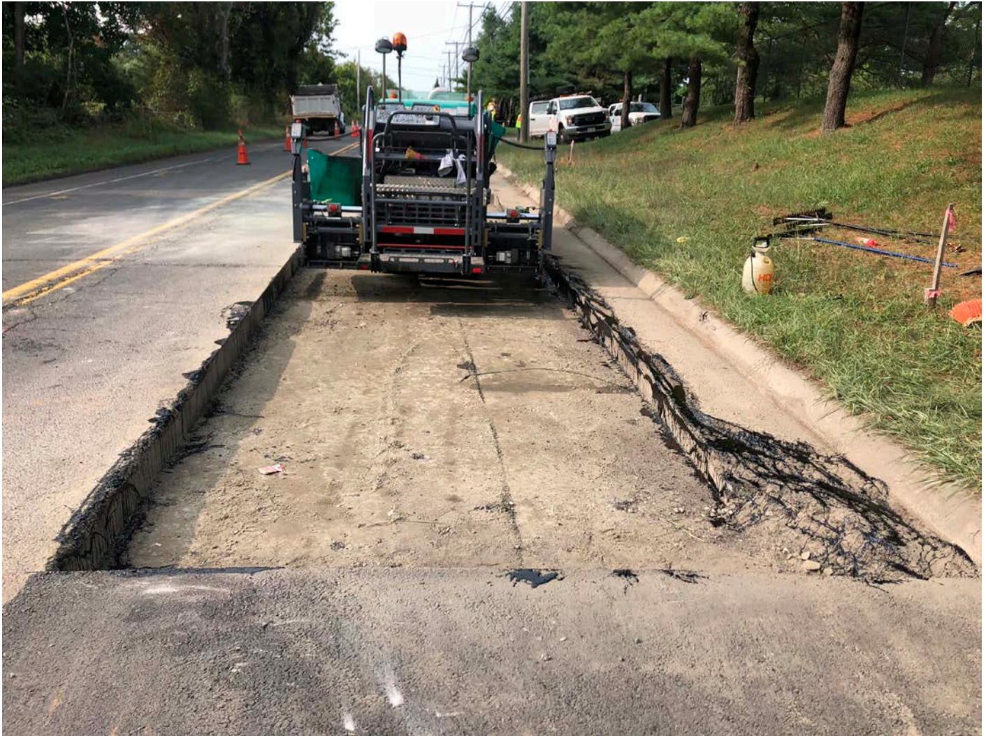
Picture 5: Tack coating applied to the cut edges of asphalt at the trench cutbacks that Ludlow repaved today from Stations 102+00 to 104+50 on S. Main Street, Middletown. View to the south.
