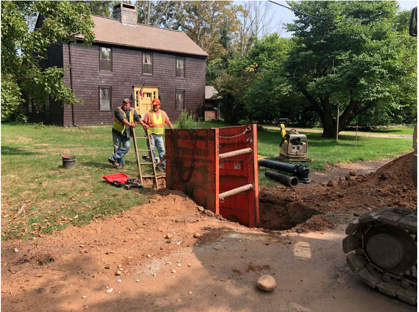
Picture 7: Ludlow installing a curb stop at Station 305+06 that will service 25 Talcott Lane, Durham. View to the northeast.
