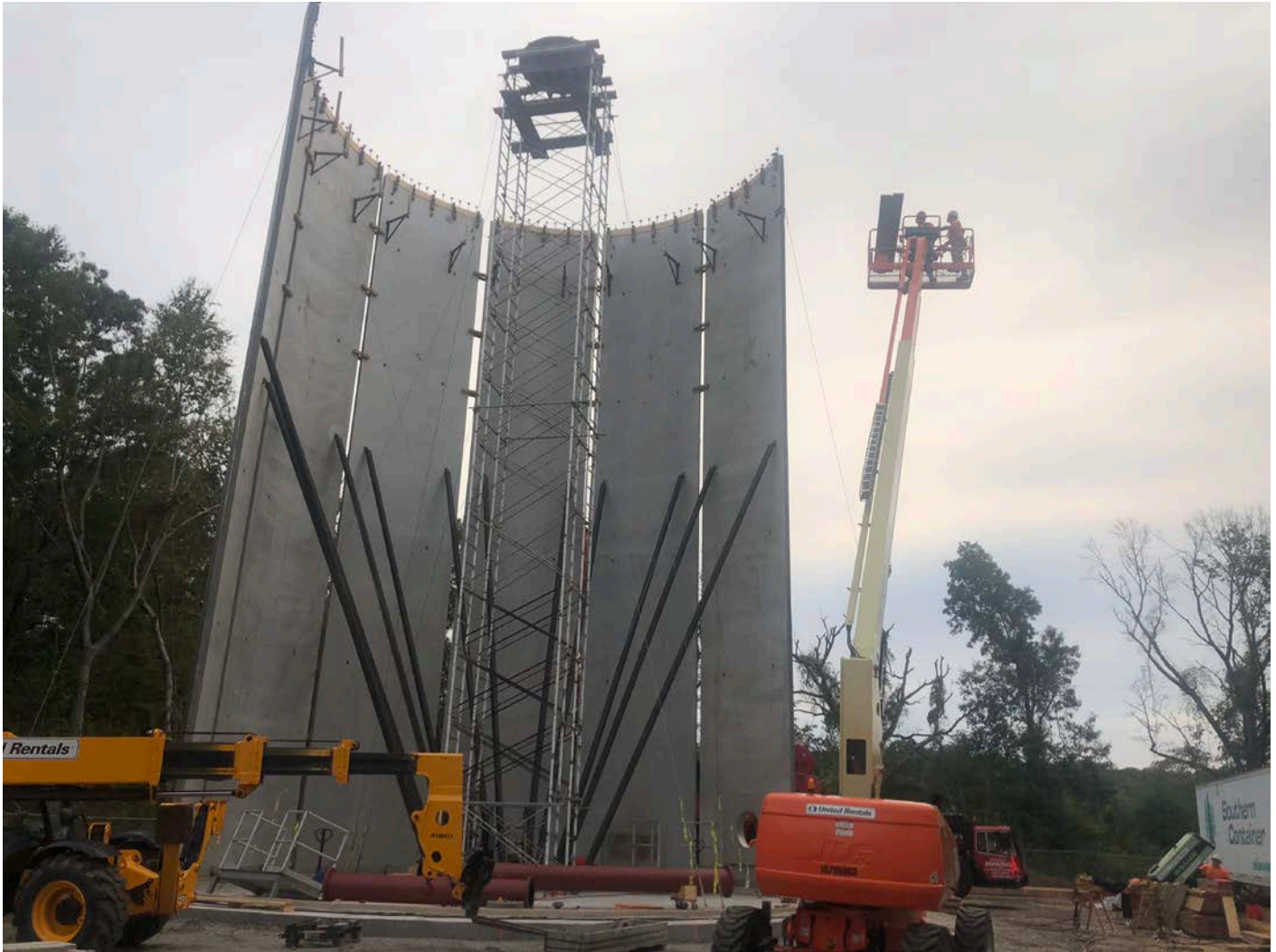
Picture 1: DN Tanks using lift boom to bring materials to the top of the center tower. Water tank work zone, east of the Shared Access Driveway, Middletown. View to the east.
