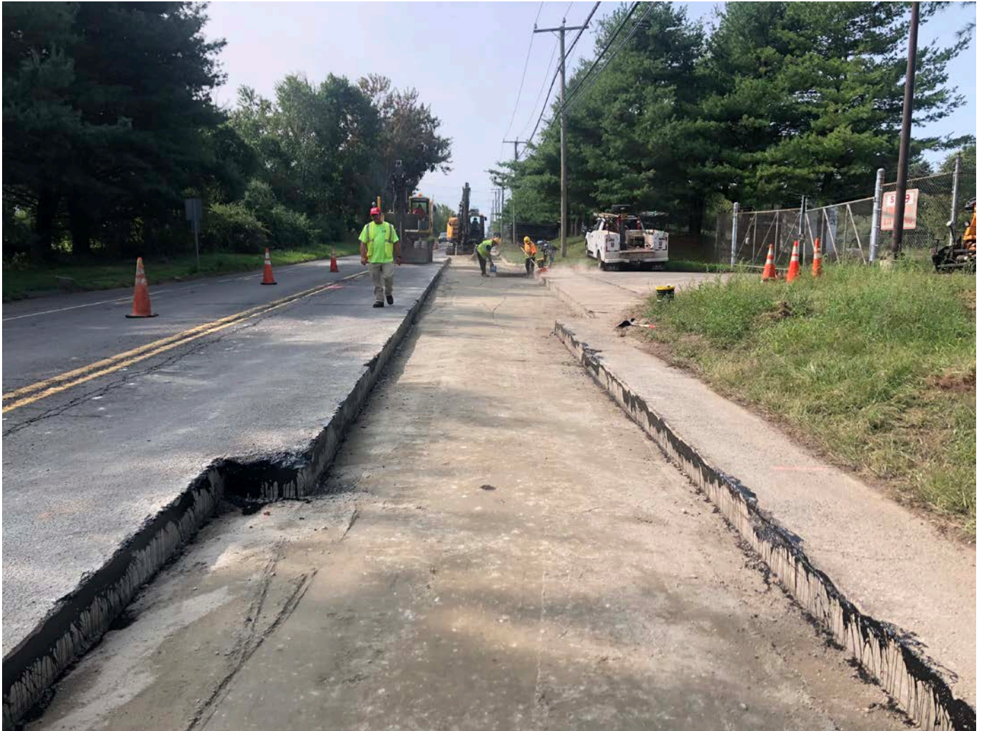
Picture 7: Ludlow applying tack coat to the edges of saw cut pavement as they prepare to repave trench cutbacks on S. Main Street, Middletown. View to the south.
