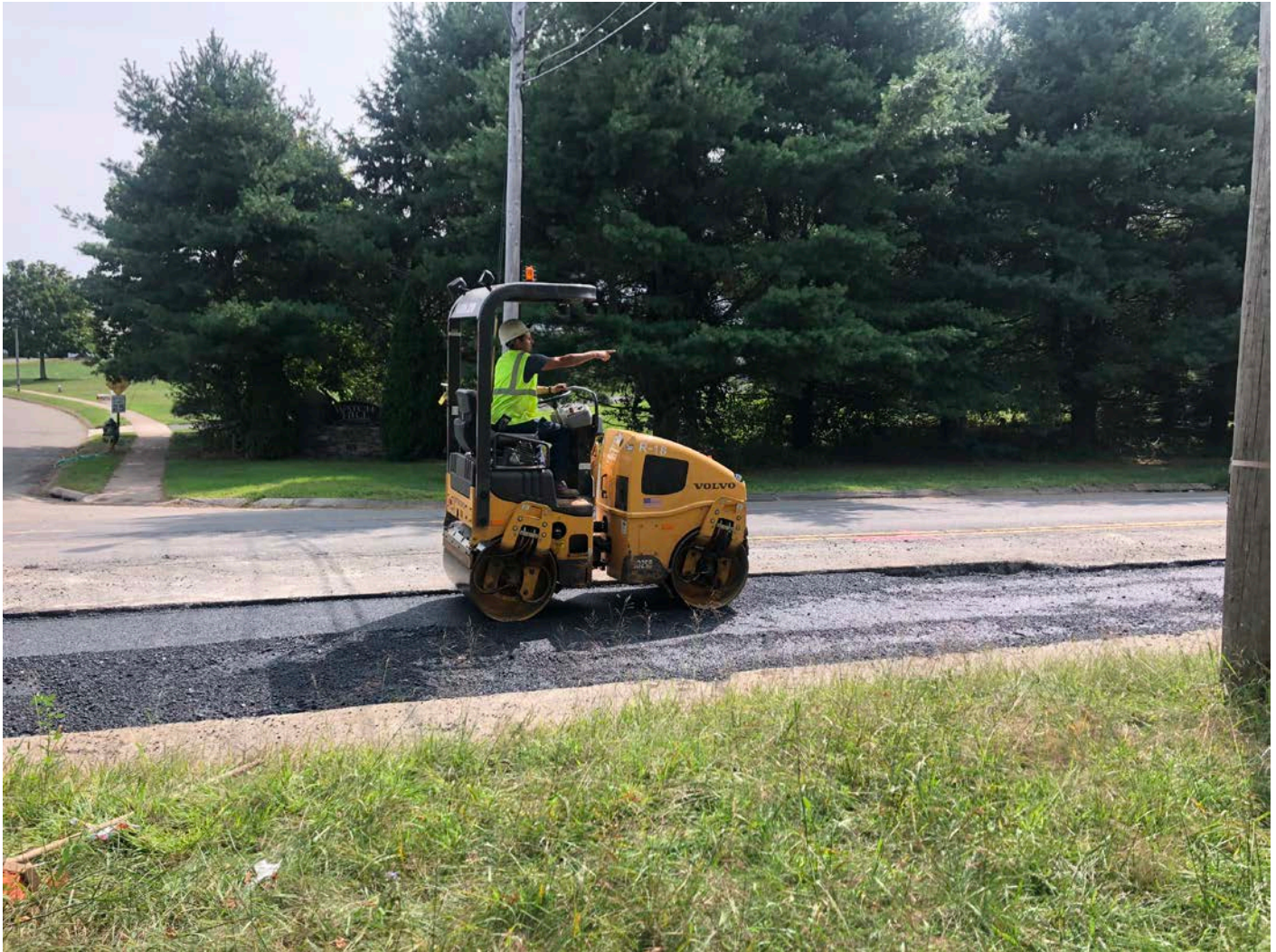
Picture 9: Ludlow compacting second of three 3" lifts of asphalt as they repave trench cutbacks on S. Main Street, Middletown. Station 100+00. View to the east.
