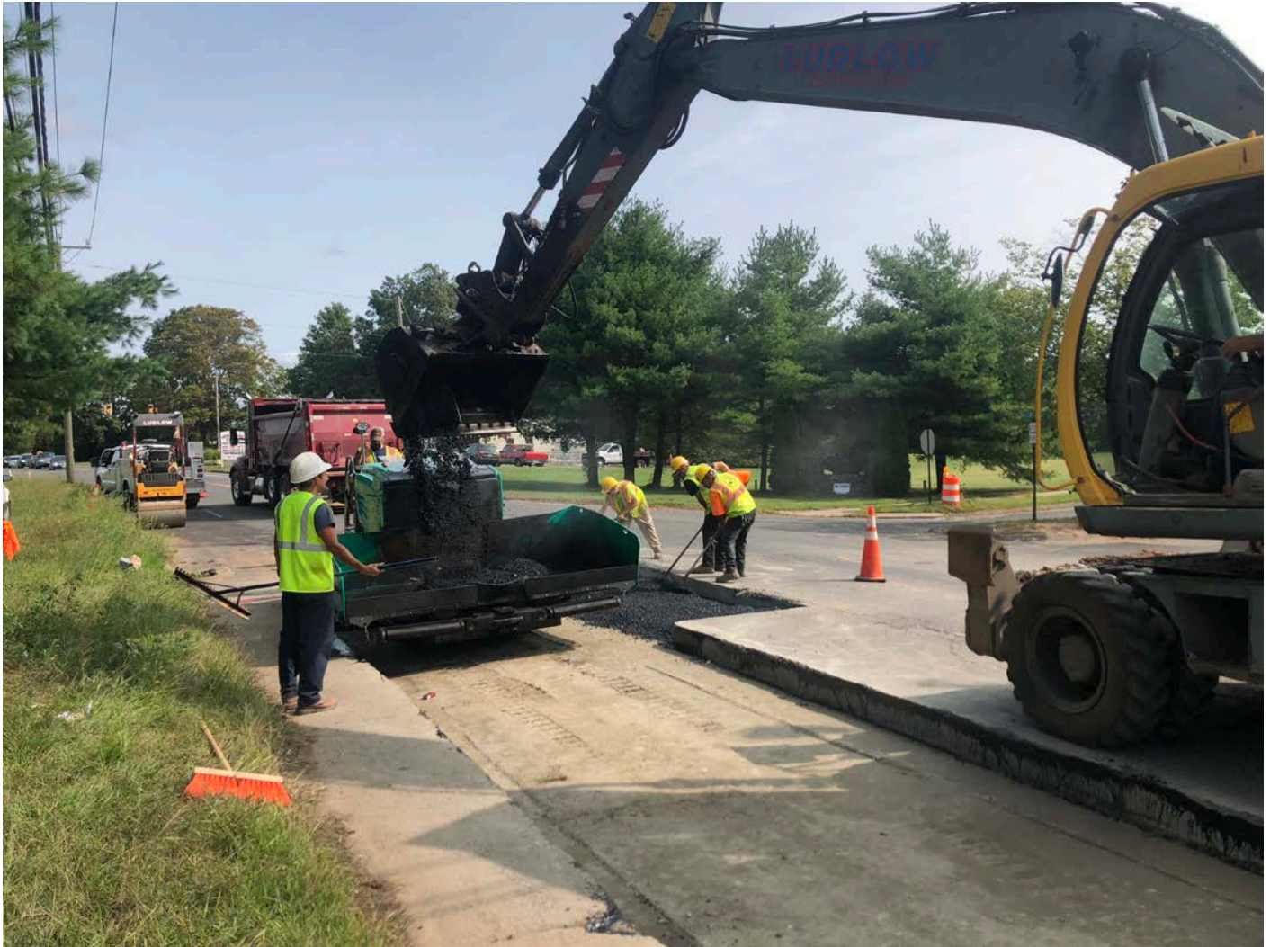
Picture 8: Ludlow placing the first of three 3" lifts of asphalt as they repave trench cutbacks on S. Main Street, Middletown. Station 100+00. View to the northeast.
