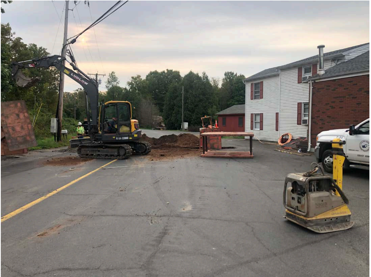
Picture 3: Ludlow excavating for the installation of a curb stop on Haddam Quarter Road, servicing 363 Main Street, Durham. View to the east.
