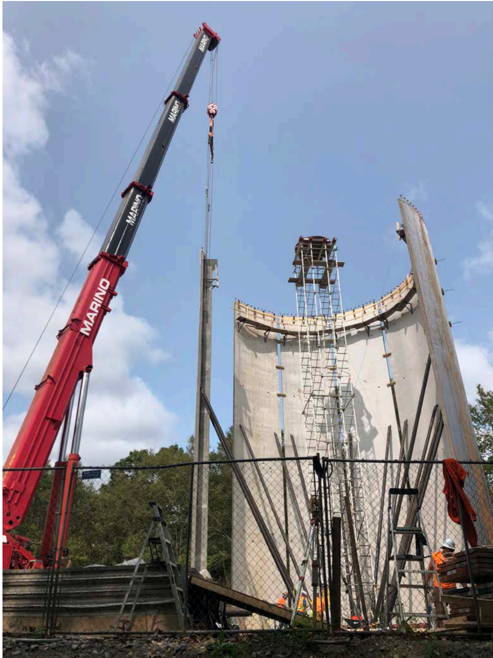
Picture 10: Marino lifting narrow water tank side panel into place for DN Tanks to secure it to the water tank base. Water tank work zone, east of the Shared Access Driveway, Middletown. View to the north.
