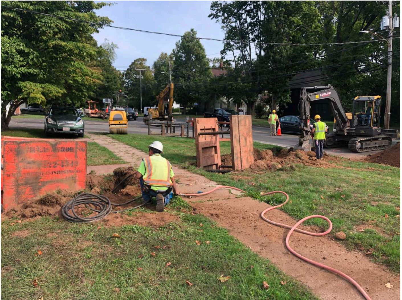
Picture 6: Ludlow installing a curb stop at Station 193+18 to provide service to 236 Main Street. Ludlow is using a pneumatic mole to advance a hole beneath the Town sidewalk for the placement of a 1" copper service line. View to the northeast.
