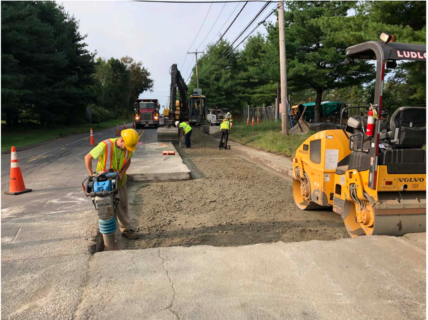
Picture 5: Ludlow compacting 1.5" processed gravel as they prepare to repave trench cutbacks on S. Main Street, Middletown. Station 100+00. View to the south.
