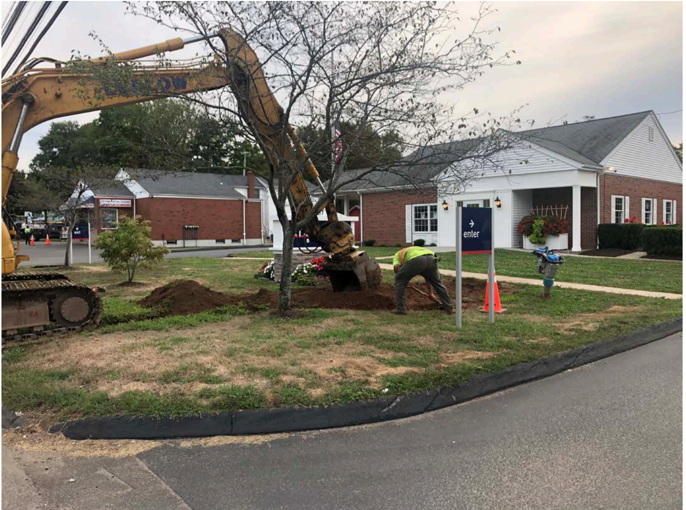
Picture 4: Ludlow excavating for the installation of a curb stop at Station 168+79 that will bring service to 357 Main Street, Durham. View to the southeast.
