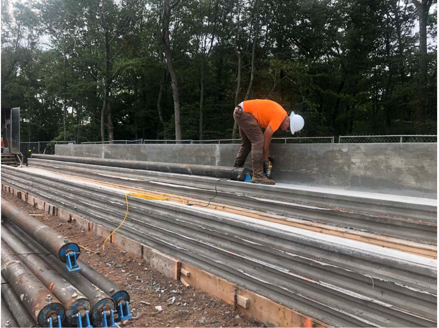
Picture 2: DN Tanks securing knee brace to narrow water tank side panel. Water tank work zone, east of the Shared Access Driveway, Middletown. View to the southeast.
