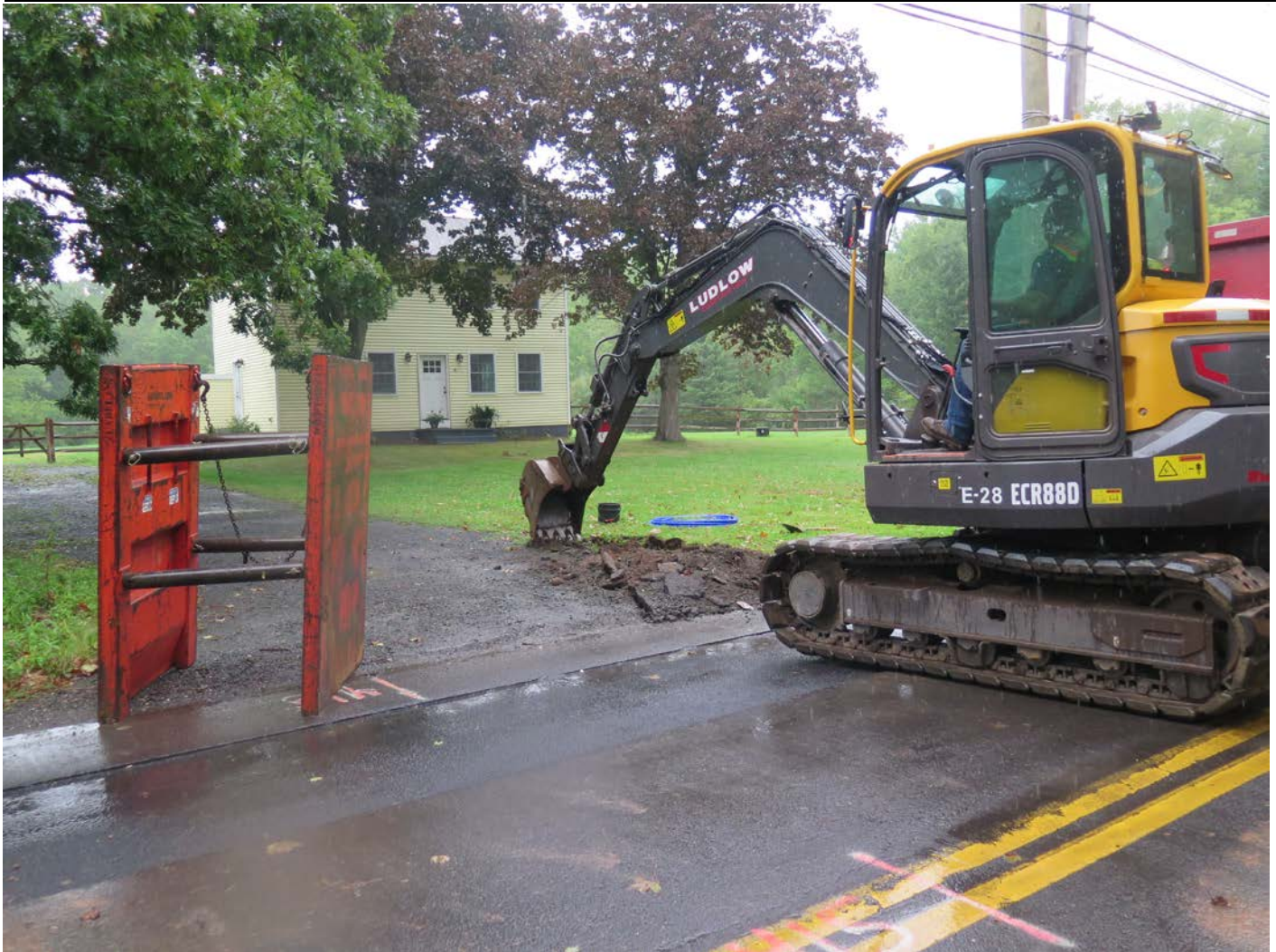
Picture 4: Excavating for curb stop at #78 Maiden Lane, Durham. View to the northeast.
