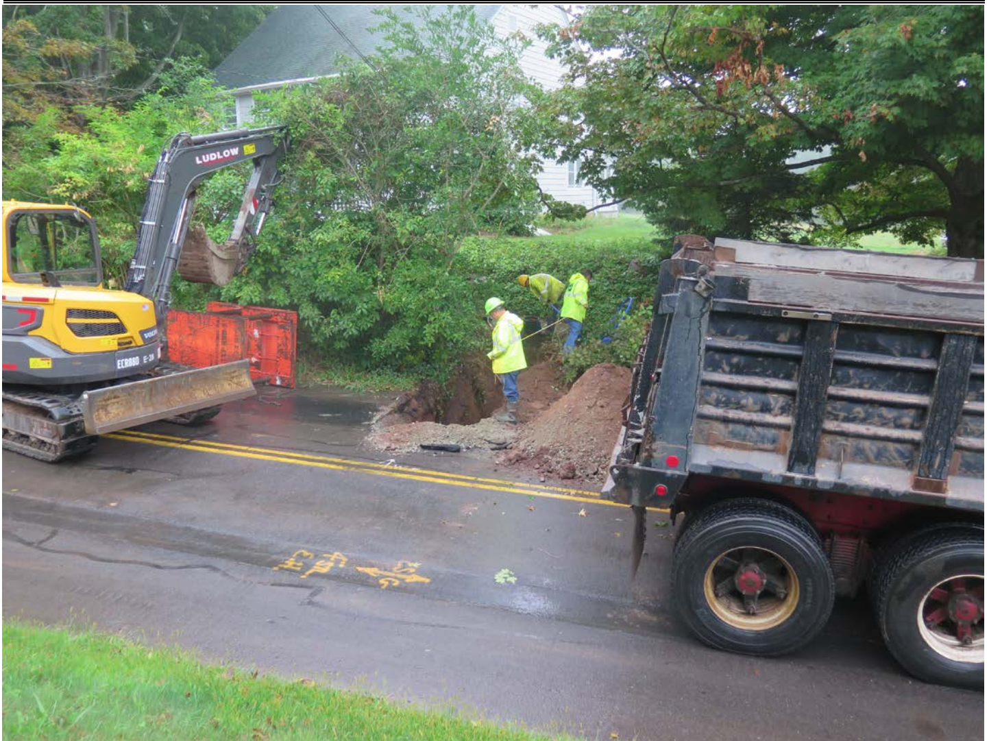
Picture 1: Installing curb stop at #36 Maiden Lane. View to the north.
