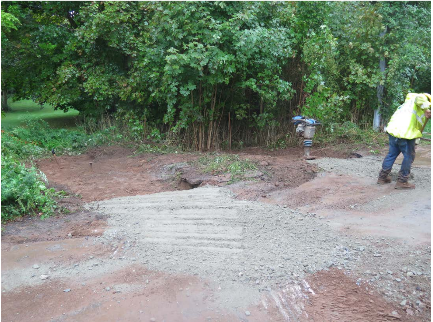
Picture 2: Backfilling curb stops at 212 and 212R Maple Avenue, Durham. View to the west.
