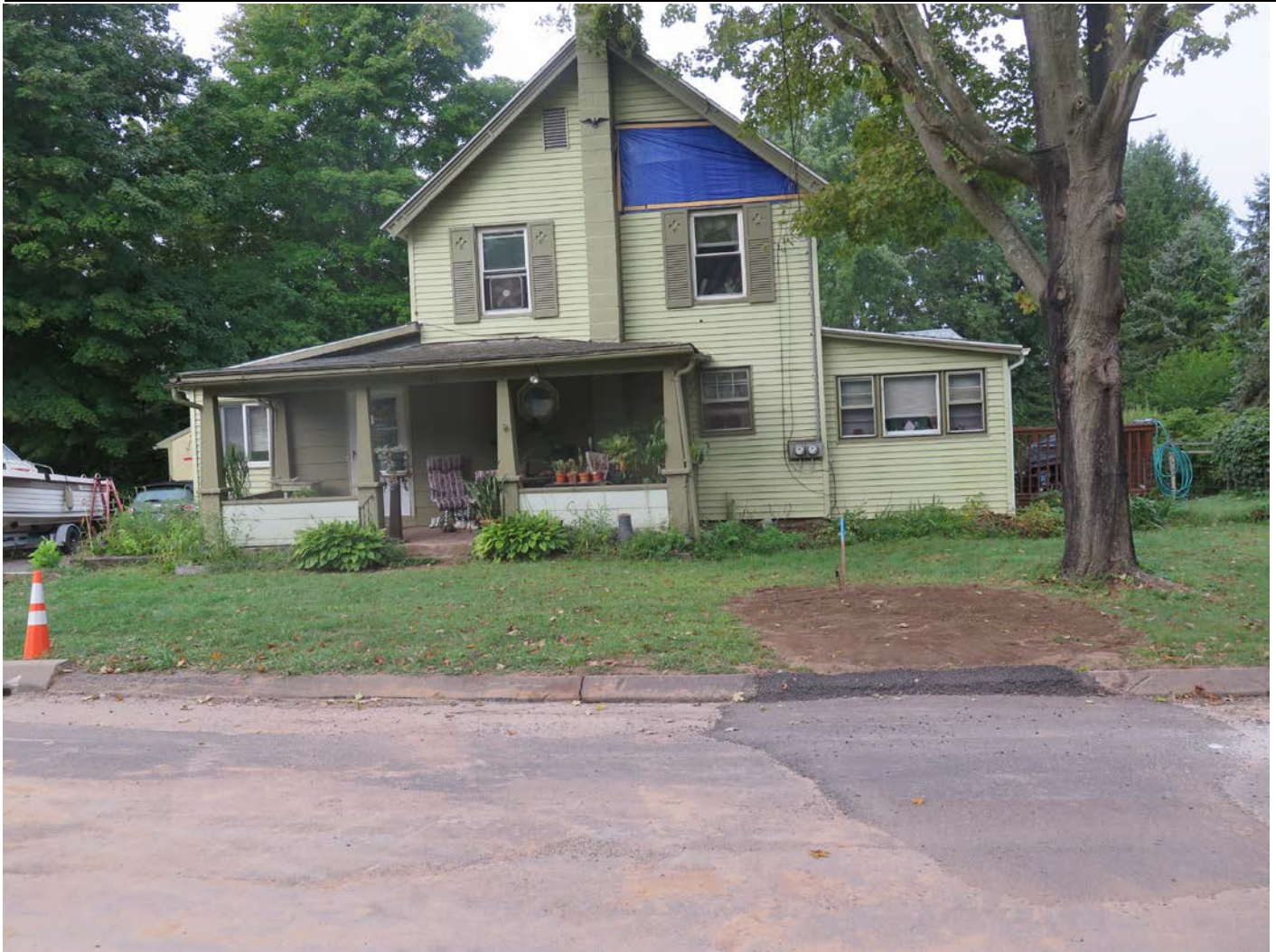
Picture 2: Curb stop completed at 176 Maple Avenue, Durham. View to the west.
